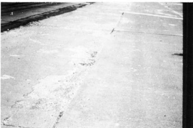
FIG. X2.46 High-Severity Scaling
