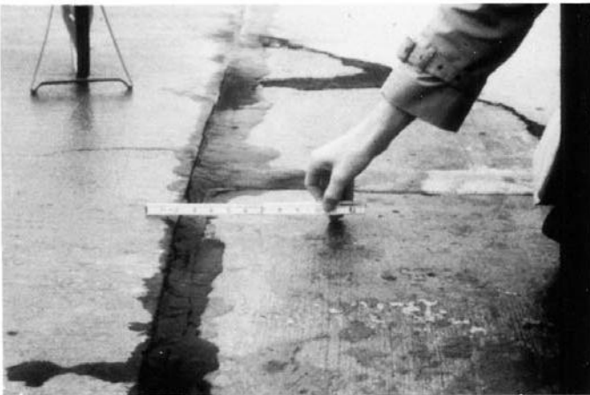
FIG. X2.50 Medium-Severity Settlement on Apron (> 1/2 in. (13 mm))
