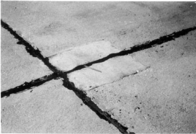
FIG. X2.28 Low-Severity Small Patch
