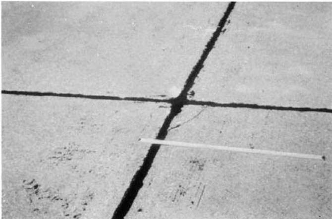
FIG. X2.68 Low-Severity Corner Spall
