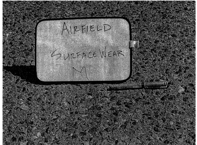
FIG. X1.80 Medium-Severity Weathering (Surface Wear)
