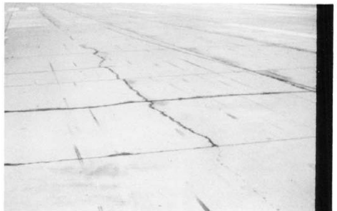
FIG. X2.53 Low-Severity Intersecting Cracks
