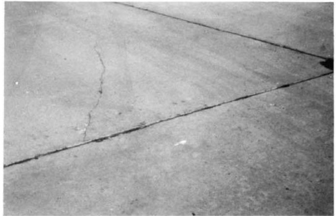
FIG. X2.11 Low-Severity Diagonal Crack
