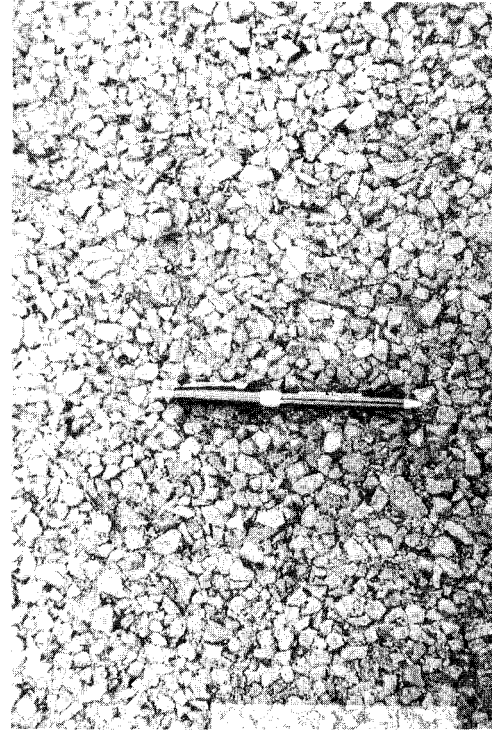
FIG. X1.61 Typical Porous Friction Course Surface with No Raveling
