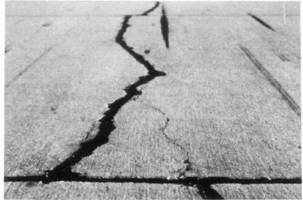
FIG. X2.16 High-Severity Longitudinal Cracks
