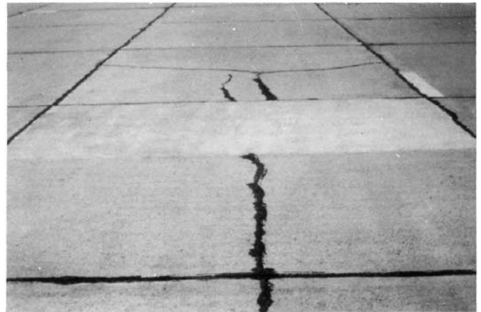
FIG. X2.34 Low-Severity Patch
