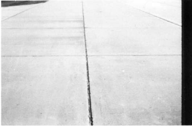
FIG. X2.40 Pumping (Note Stains on Pavement)
