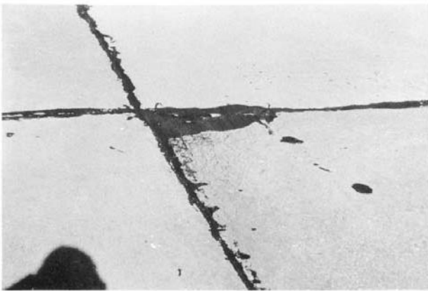
FIG. X2.19 Low-Severity "D" Cracking Approaching Medium Severity
