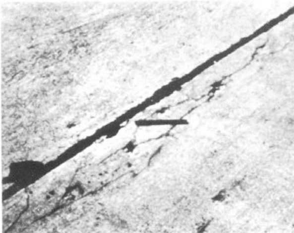
FIG. X2.20 Medium-Severity "D" Cracking
