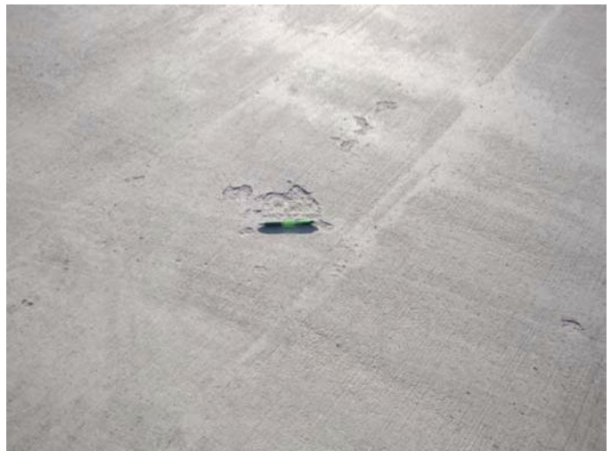
FIG. X2.44 Low-Severity Scaling
