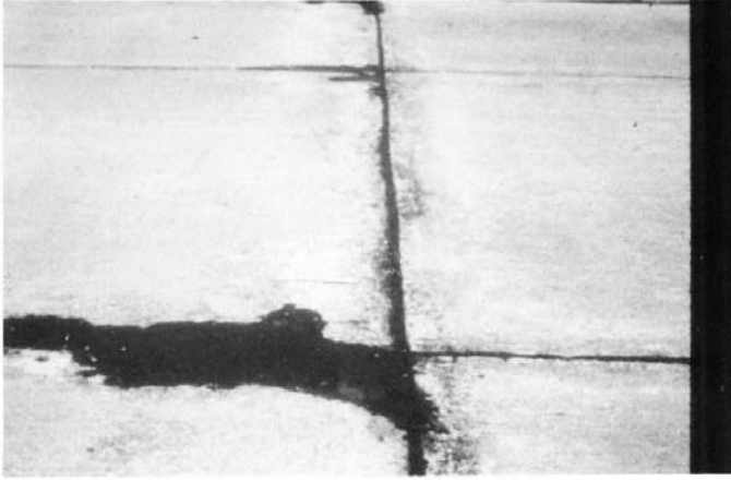
FIG. X2.45 Medium-Severity Scaling
