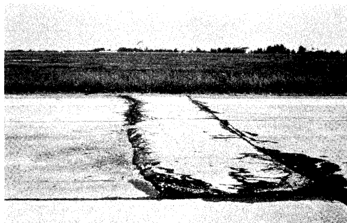
FIG. X2.2 Medium-Severity Blowup
