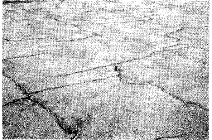
FIG. X1.17 Medium-Severity Block Cracking
