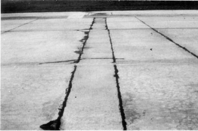
FIG. X2.35 Low-Severity Utility Cut
