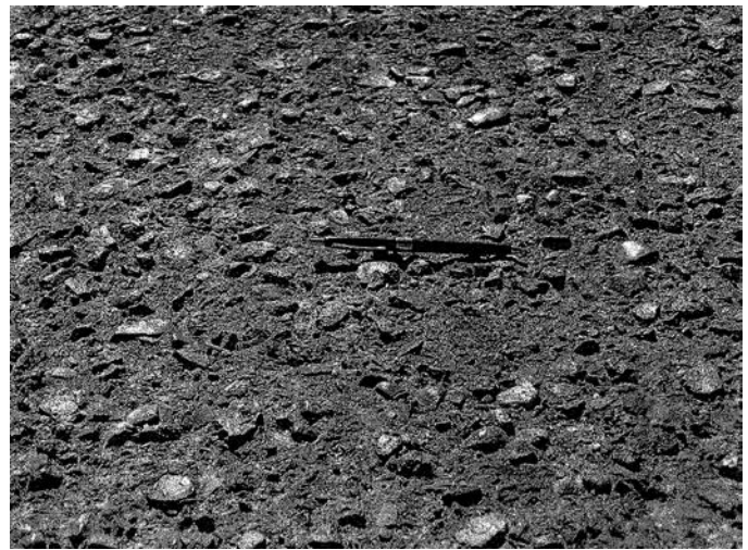
FIG. X1.81 High-Severity Weathering (Surface Wear)
