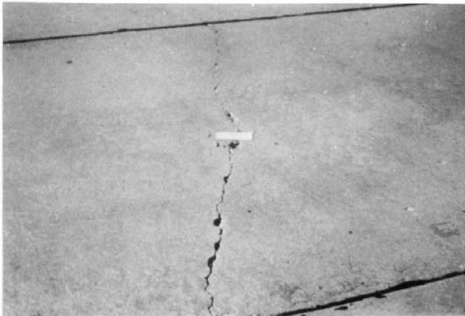
FIG. X2.14 Medium-Severity Transverse Crack
