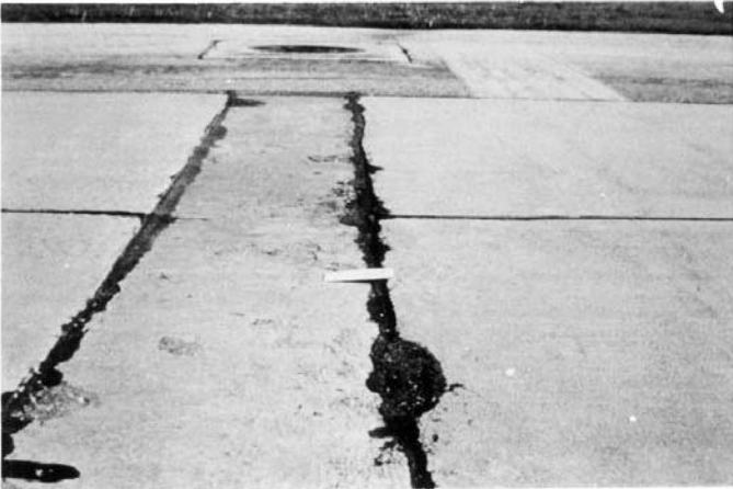
FIG. X2.36 Medium-Severity Utility Cut
