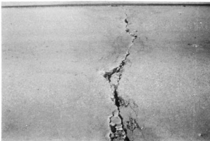
FIG. X2.15 High-Severity Crack
