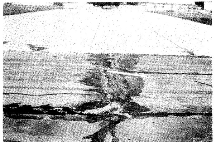
FIG. X1.78 High-Severity Swell
