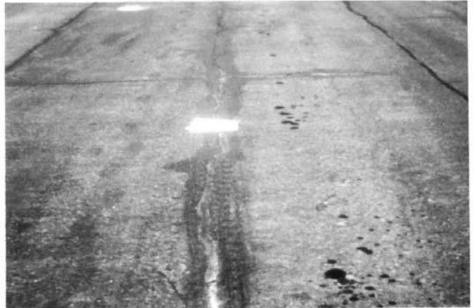
FIG. X1.40 Medium-Severity Longitudinal Crack (Note the Crack is Reflective But Not at the Joint of Slab)
