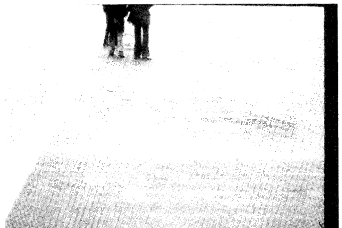
FIG. X1.46 Oil Spillage
