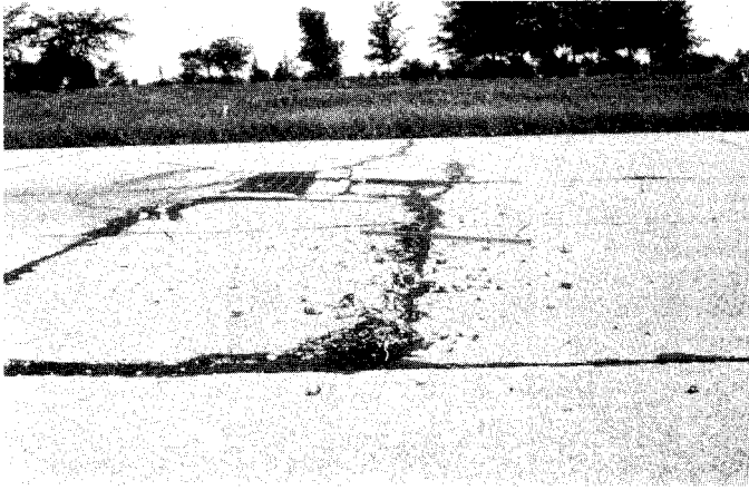
FIG. X2.1 Low-Severity Blowup
