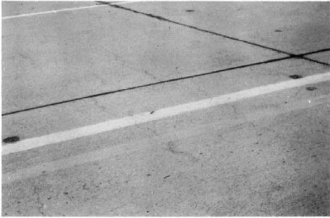
FIG. X2.59 Shrinkage Cracks
