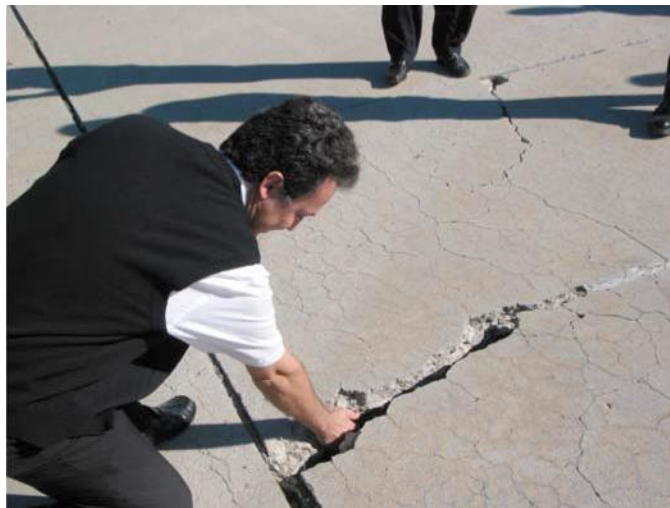
FIG. X2.76 High-Severity ASR
