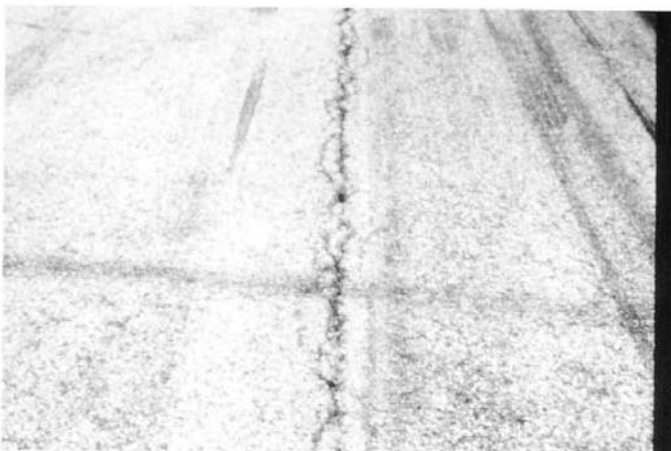
FIG. X1.39 Medium-Severity Longitudinal Construction Joint Crack
