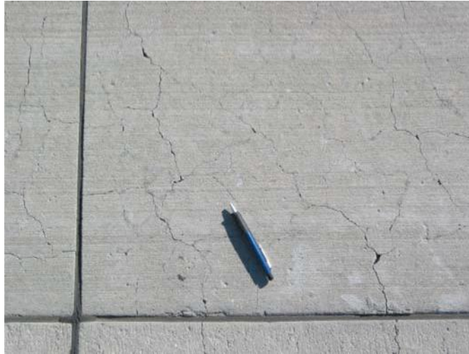
FIG. X2.75 Medium-Severity ASR
