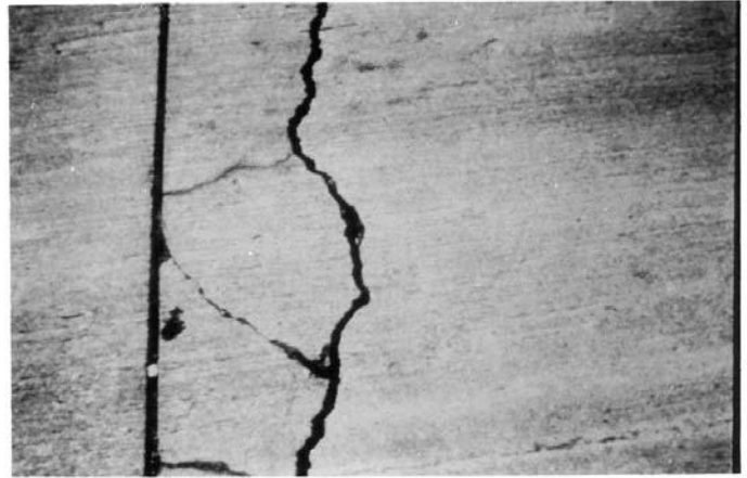
FIG. X2.64 Medium-Severity Joint Spall
