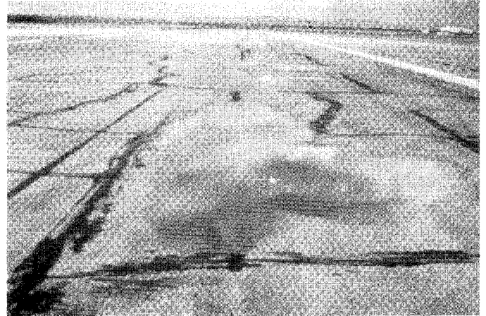
FIG. X1.27 High-Severity Depression (2 in. (50 mm))
