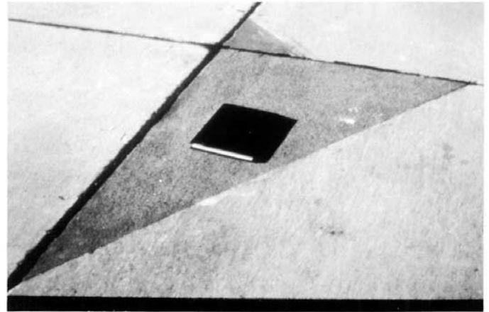
FIG. X2.33 Low-Severity Patch
