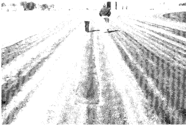
FIG. X1.48 Low-Severity Patch
