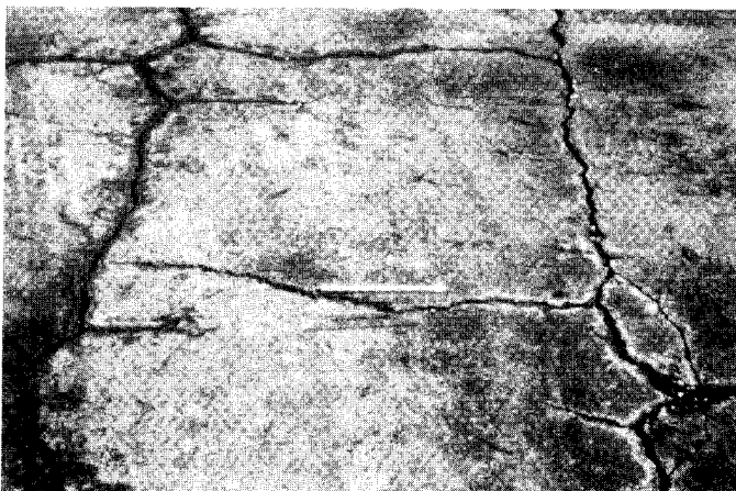
FIG. X1.16 Medium-Severity Block Cracking
