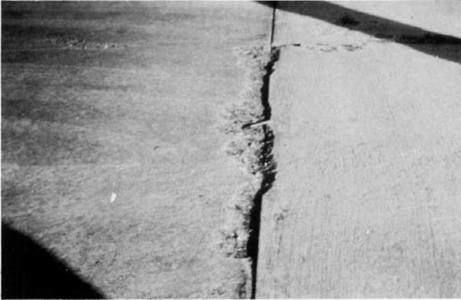
FIG. X2.67 High-Severity Joint Spall
