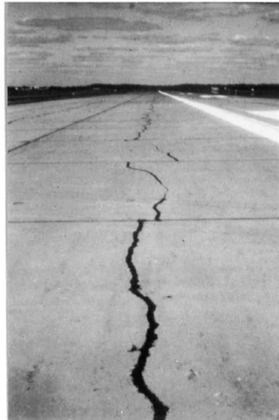
FIG. X2.12 Medium-Severity Longitudinal Crack
