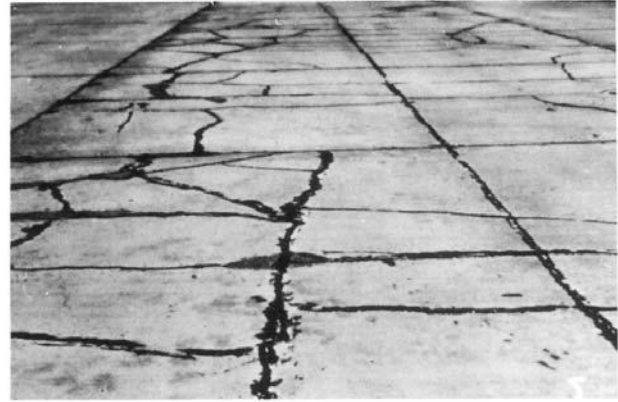
FIG. X2.57 Shattered Slab
