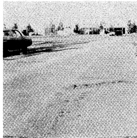
FIG. X1.77 High-Severity Swell
