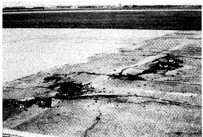
FIG. X1.72 High-Severity Shoving
