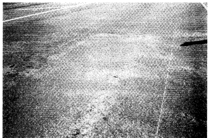
FIG. X1.22 Medium-Severity Corrugation
