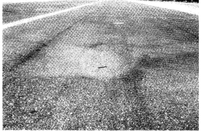
FIG. X1.26 Medium-Severity Depression
