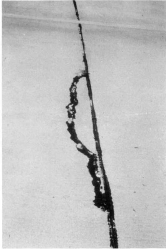
FIG. X2.62 Low-Severity Joint Spall
