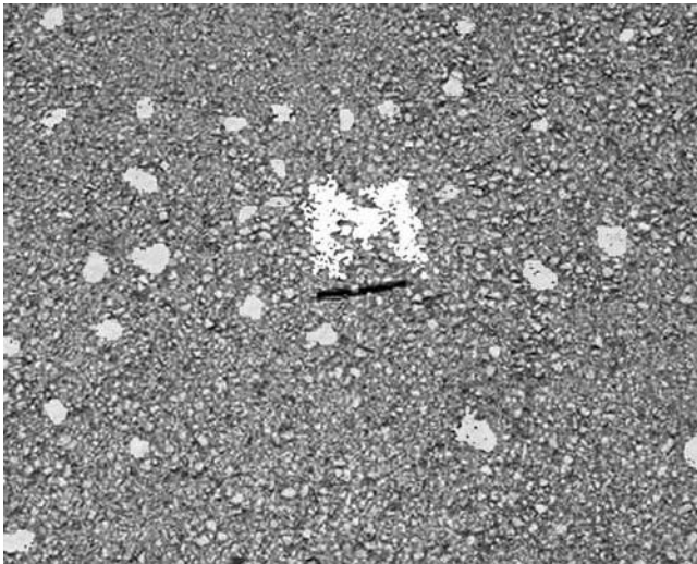
FIG. X1.56 Medium-Severity Raveling, Dense Mix
