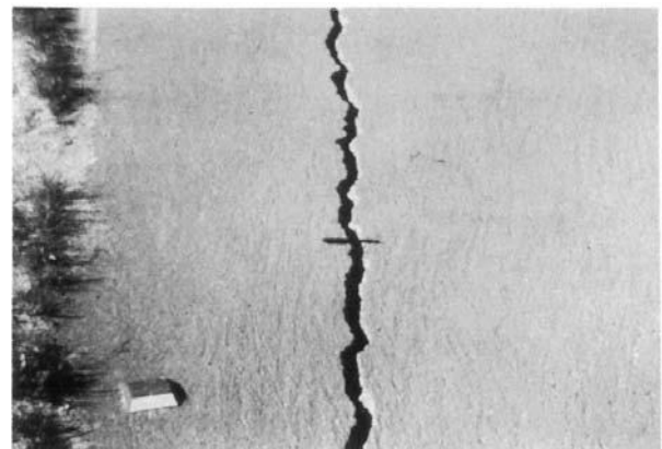
FIG. X2.17 High-Severity Crack
