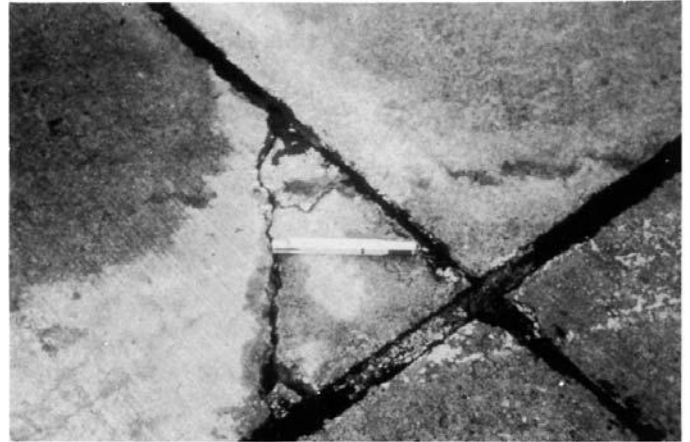
FIG. X2.70 Medium-Severity Corner Spall
