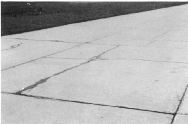
FIG. X2.56 Medium-Severity Intersecting Cracks
