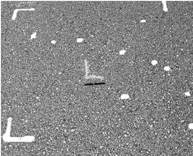
FIG. X1.55 Low-Severity Raveling, Dense Mix
