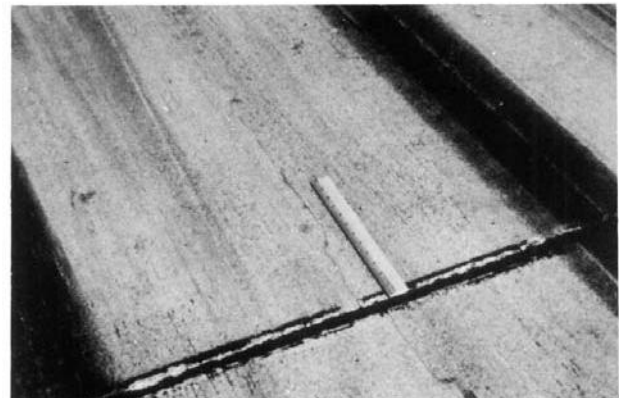
FIG. X2.58 Shrinkage Crack
