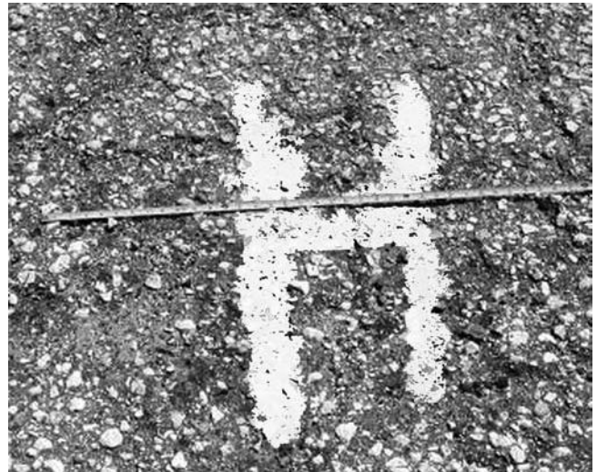
FIG. X1.57 High-Severity Raveling, Dense Mix
