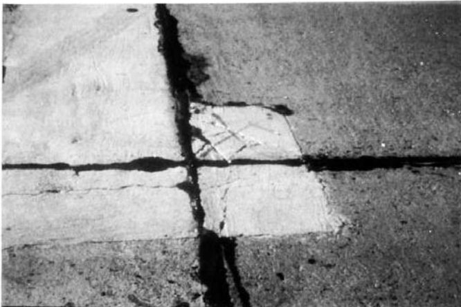
FIG. X2.31 Medium-Severity Small Patch
