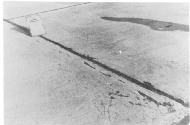
FIG. X2.22 High-Severity "D" Cracking
