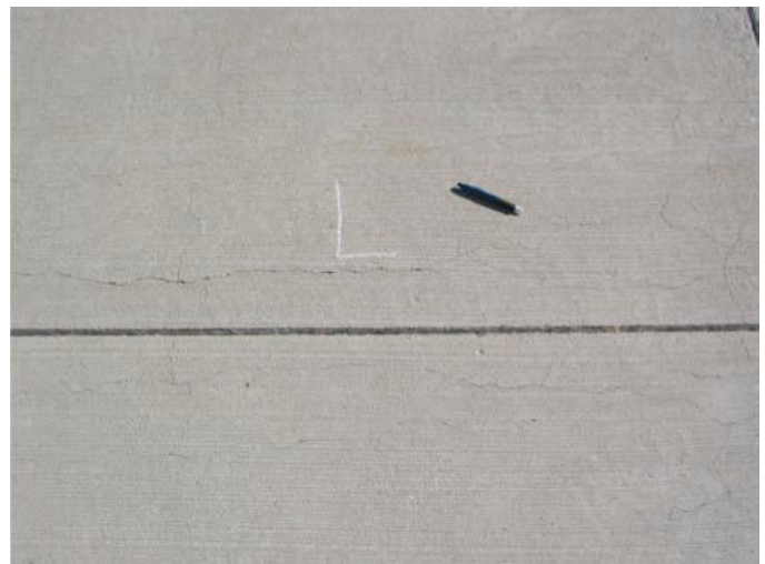
FIG. X2.74 Low-Severity ASR
