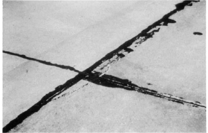
FIG. X2.69 Low-Severity Corner Spall
