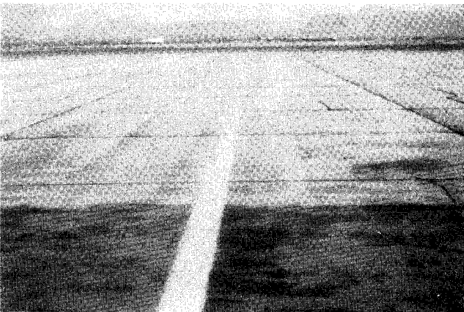
FIG. X1.30 Low-Severity Joint Reflection Cracking
