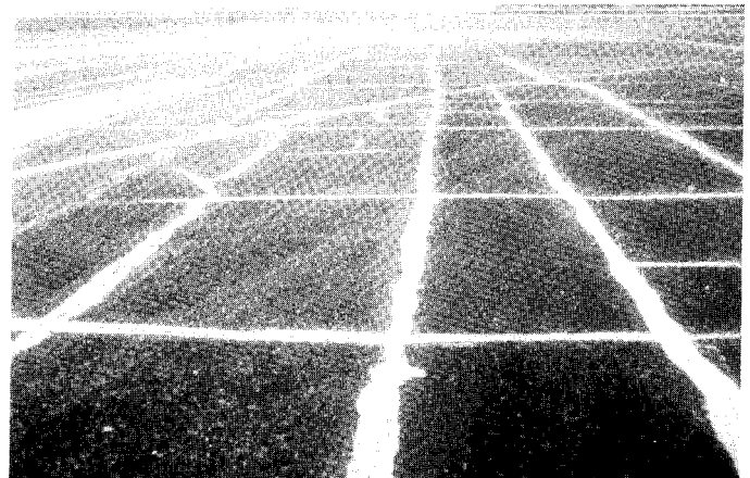
FIG. X1.13 Low-Severity Block Cracking, Filled Cracks
