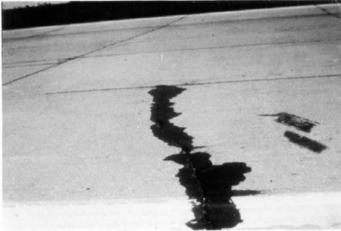
FIG. X2.13 Medium-Severity Transverse Crack
