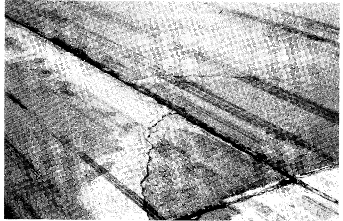
FIG. X2.7 Medium-Severity Corner Break
