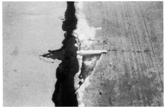
FIG. X2.65 Medium-Severity Joint Spall
