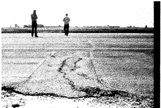
FIG. X1.52 High-Severity Patch
