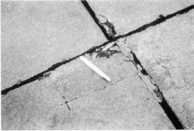
FIG. X2.30 Medium-Severity Small Patch
