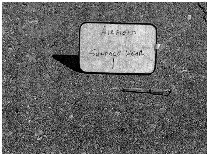
FIG. X1.79 Low-Severity Weathering (Surface Wear)
