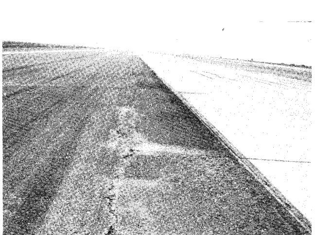
FIG. X1.41 Medium-Severity Longitudinal Crack
