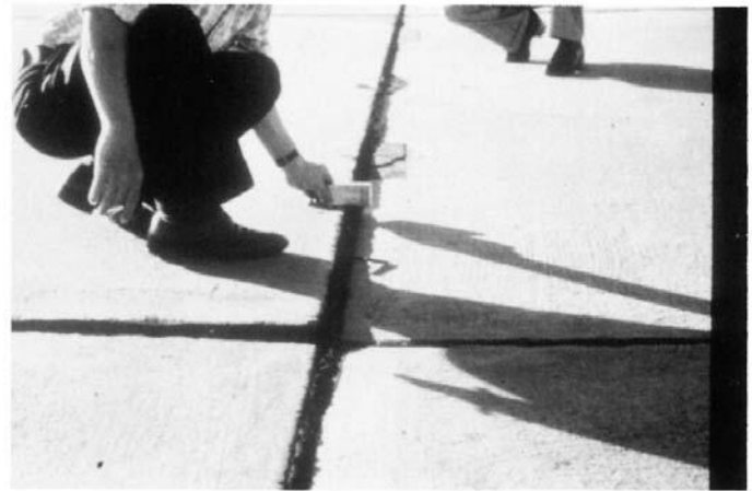
FIG. X2.52 High-Severity Settlement
