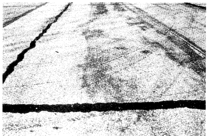
FIG. X1.31 Low-Severity Joint Reflection Cracking, Filled Crack
