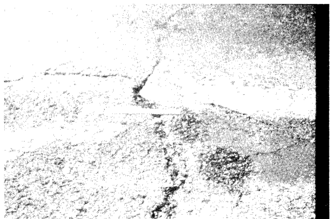
FIG. X1.42 High-Severity Longitudinal Crack
