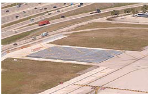
EMAS bed at Fort Lauderdale–Hollywood International Airport (above) and close-up view (right).
