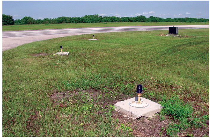
Taxiway edge lights, above, must meet the standards indicated in Chapter 14-60 of the Florida Administrative Code.
