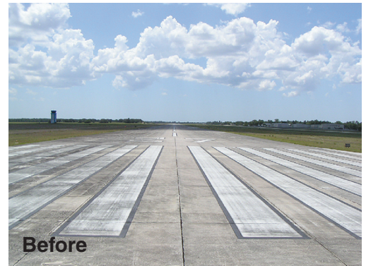
Above and left: Before and after photos of algae removal and runway cleaning performed by Hi-Lite Airfield Services at Hernando County Airport.
