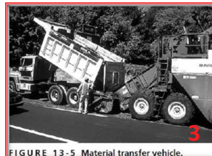
FIGURE 13-5 Material transfer vehicle.
