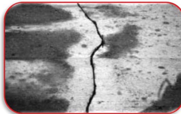
A freshly sawed crack.
