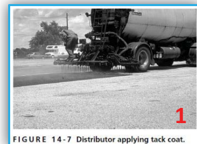
FIGURE 14-7 Distributor applying tack coat.
