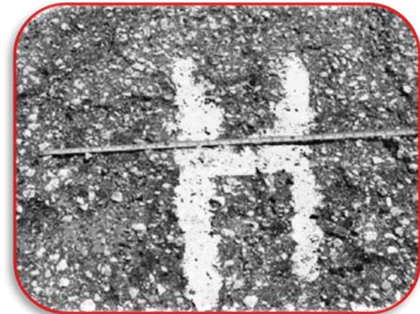
High-Severity Raveling, Dense Mix
