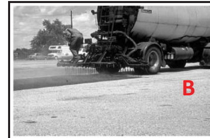
FIGURE 14-7 Distributor applying tack coat.
