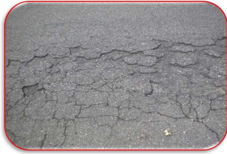
Irregularities in the asphalt surface
