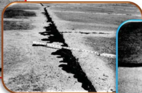
Medium-severity settlement on apron >1/2 in.
