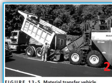
FIGURE 13-5 Material transfer vehicle.
