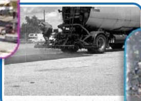
FIGURE 14-7 Distributor applying tack co
