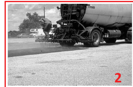
FIGURE 14-7 Distributor applying tack coat.
