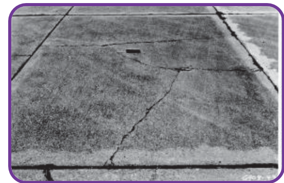
Medium-severity intersecting cracks 85
