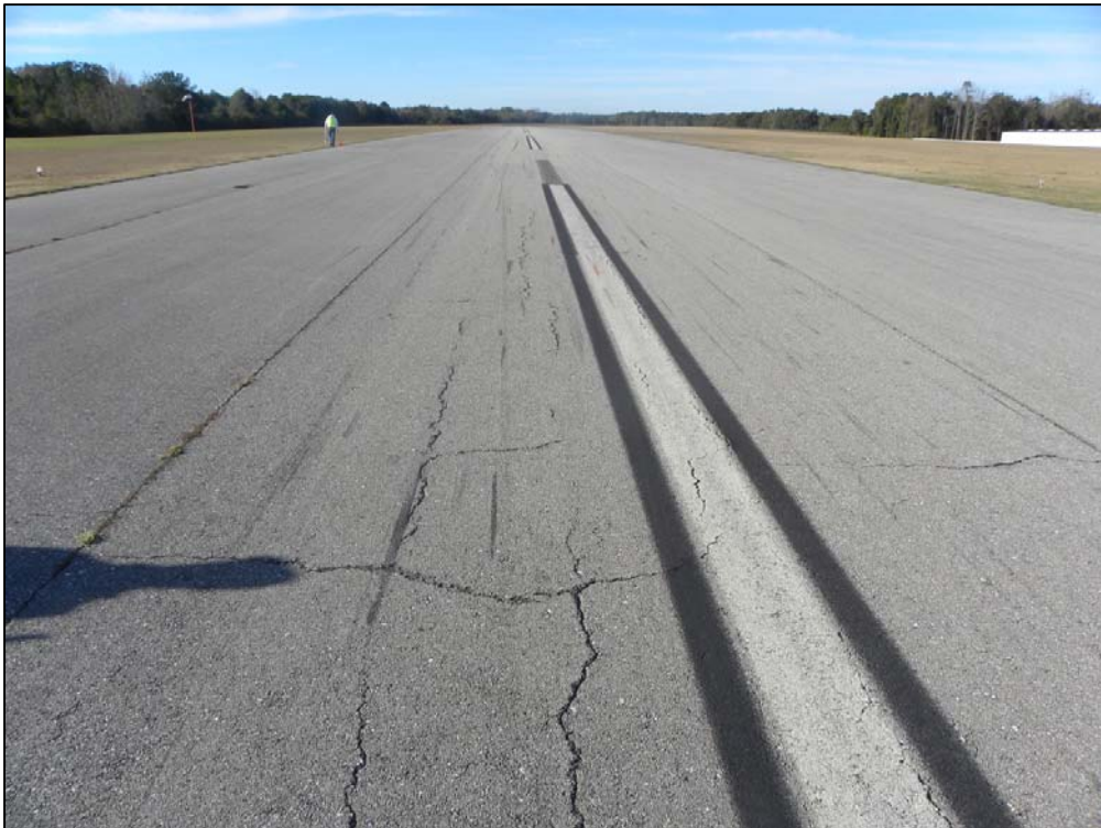
Runway 14-32, Section 6105, Sample Unit 144 – Medium severity (43) Block Cracking, medium severity (48) Longitudinal and Transverse Cracking, low and medium severity (52) Weathering and Raveling
