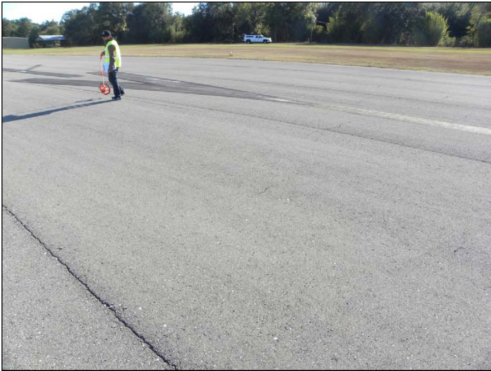
Runway 14-32, Section 6105, Sample Unit 154 – Low severity (52) Weathering and Raveling, low severity (48) Longitudinal and Transverse Cracking
