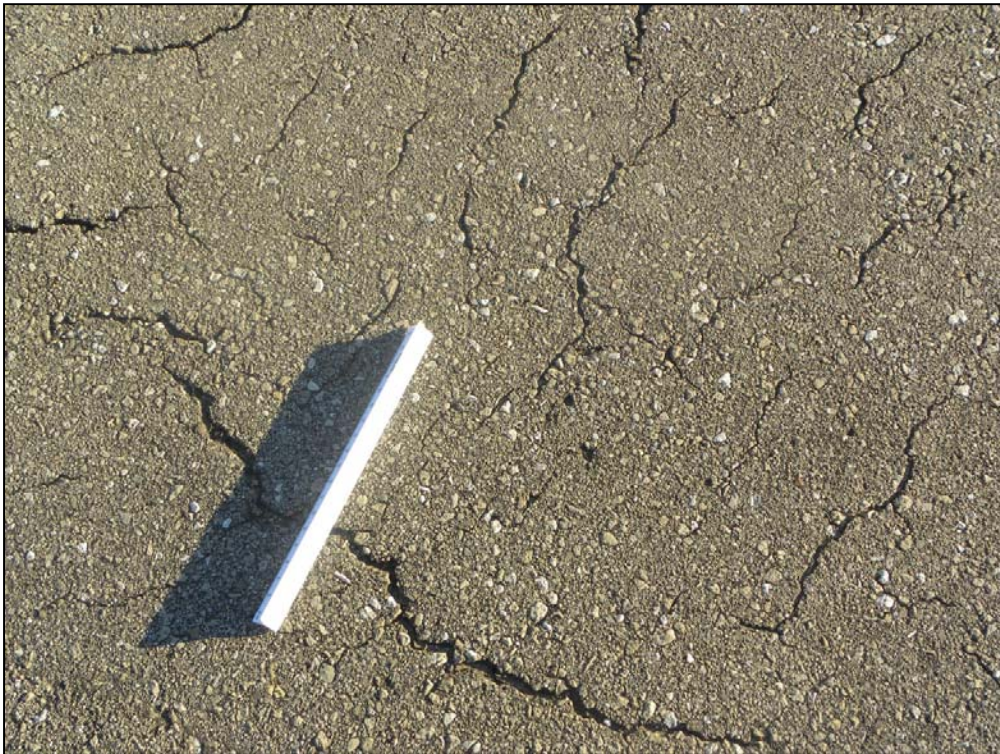
Taxiway Hangars, Section 125, Sample Unit 202 – Low severity (52) Weathering and Raveling, low severity (48) Longitudinal and Transverse Cracking
