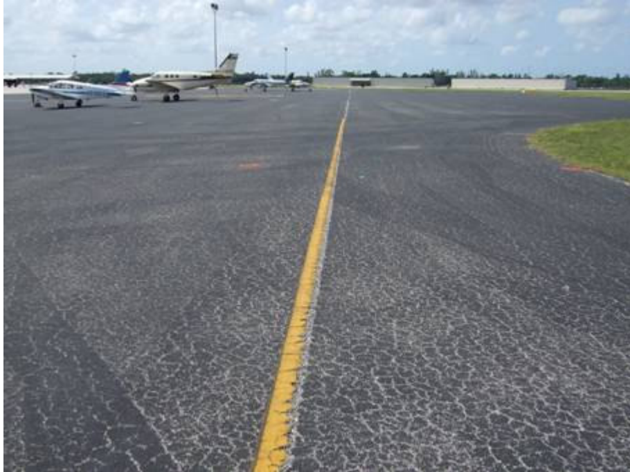
AP GA Section 4215 SU 408: Medium Severity Weathering (September 17, 2007)
