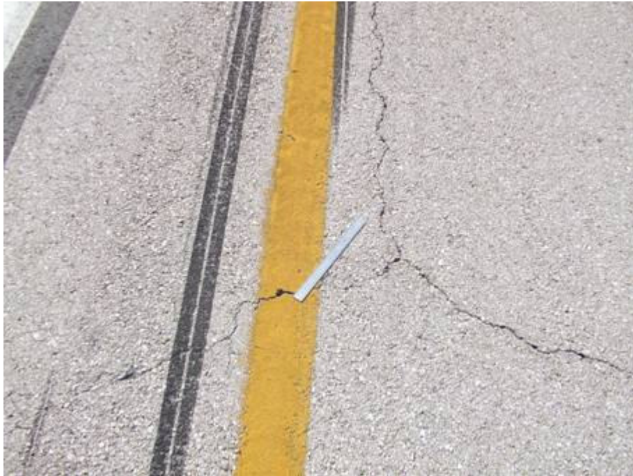
RW 14-32 Section 6215 SU 342: Low Severity L/T Cracking (September 17, 2007)
