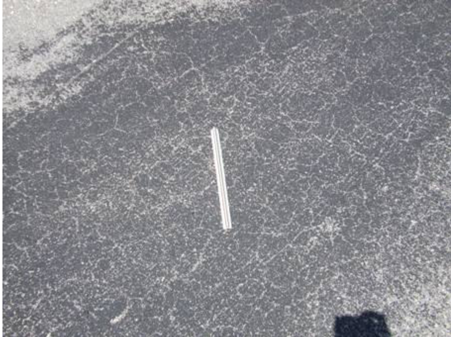
AP CONN Section 4105 SU 400: Medium Severity Weathering (September 17, 2007)
