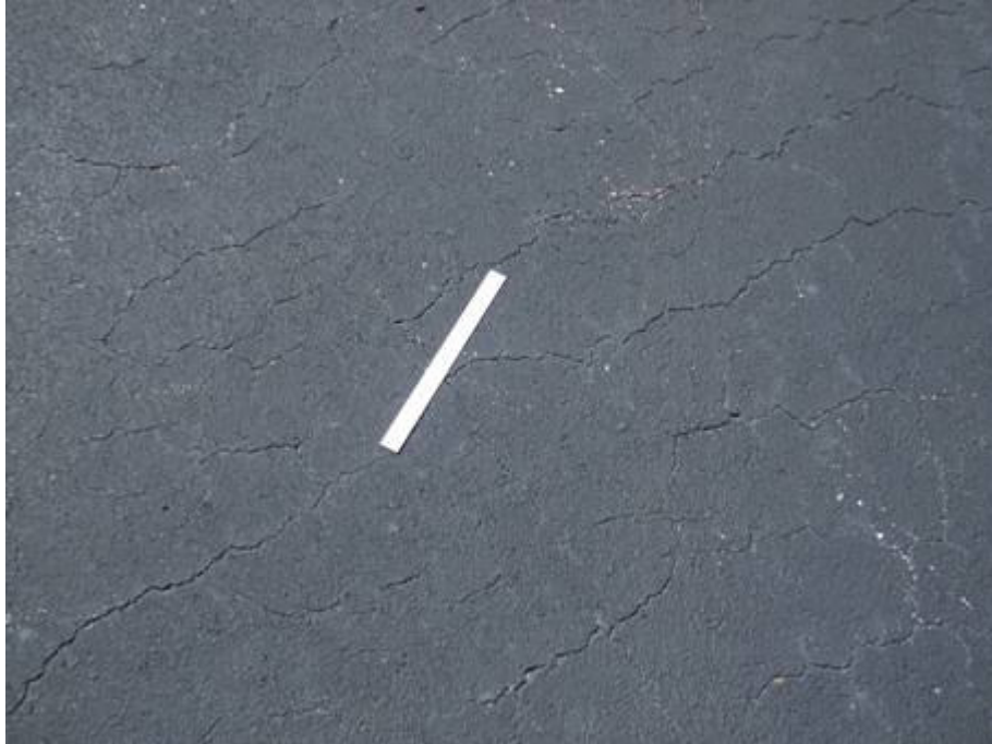
AP W Section 4605 SU 300: Low Severity Weathering (September 17, 2007)
