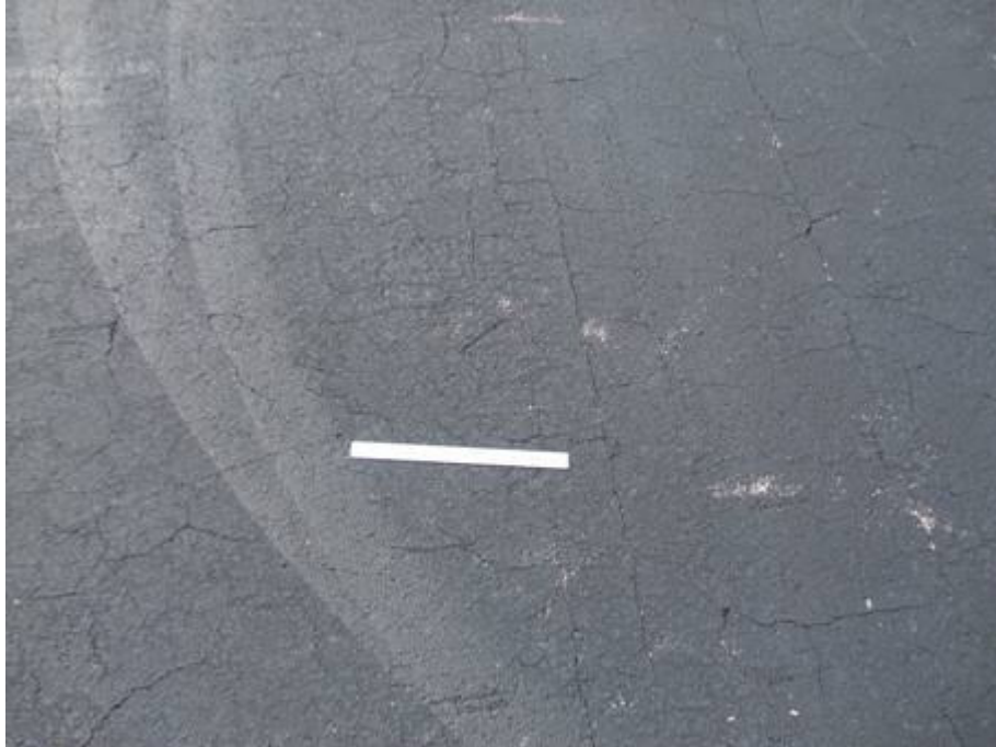
AP SW Section 4305 SU 201: Low Severity Weathering (September 17, 2007)
