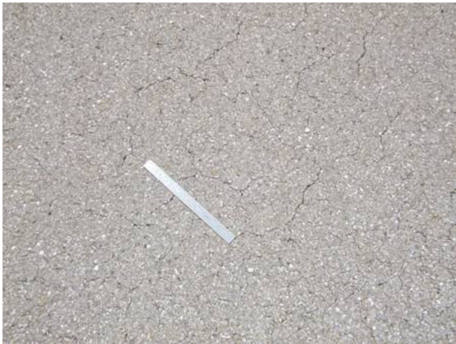
TW B Section 235 SU 101: Low Severity Weathering (September 17, 2007)
