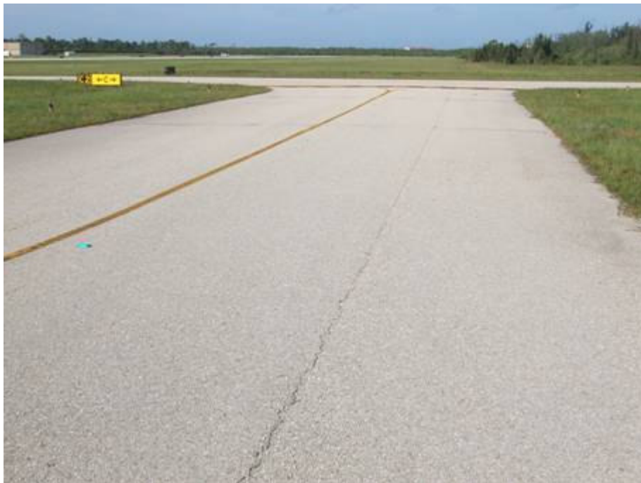
TW C-2 Section 335 SU 300: Medium Severity L/T Cracking (September 17, 2007)
