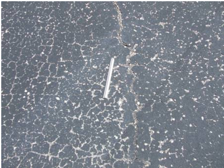
AP CONN Section 4110 SU 707: Medium Severity Weathering (September 17, 2007)
