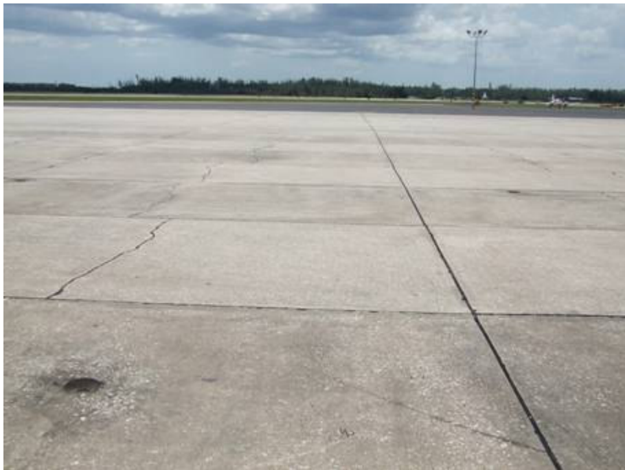
AP GA Section 4205 SU 600: Medium Severity Linear Cracking (September 17, 2007)
