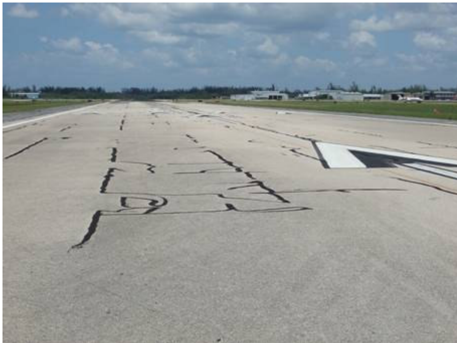
RW 14-32 Section 6230 SU 398: Low Severity L/T Cracking (September 17, 2007)
