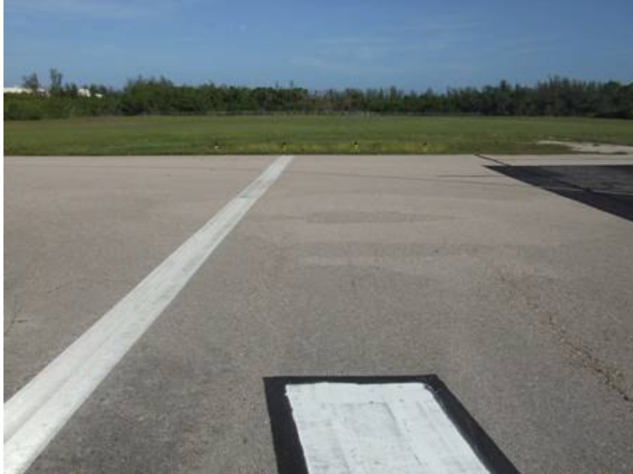
RW 14-32 Section 6204 SU 500: Low Severity L/T Cracking (September 17, 2007)
