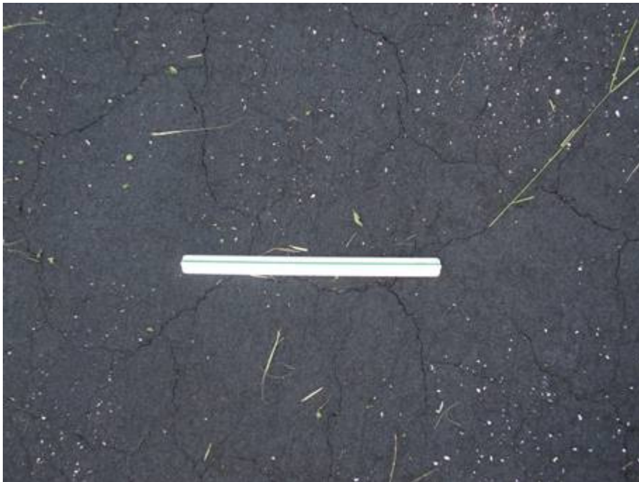
TW A-2 Section 120 SU 200: Low Severity Weathering (July 25, 2007)
