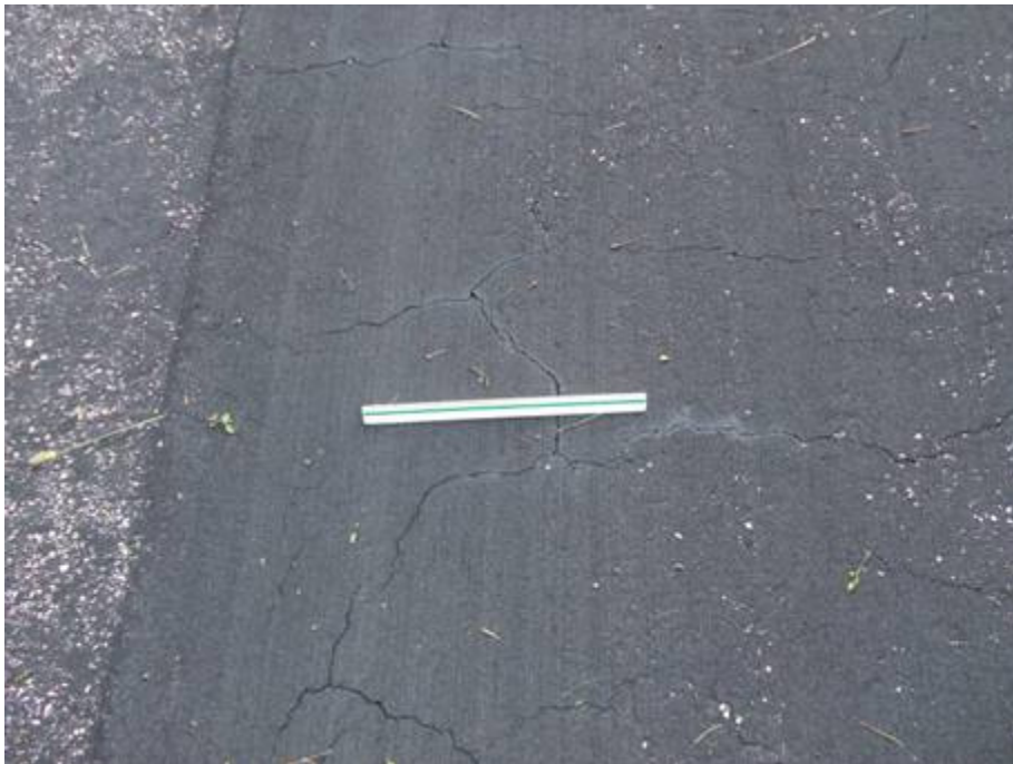
TW A-3 Section 125 SU 301: Low Severity Weathering (July 25, 2007)
