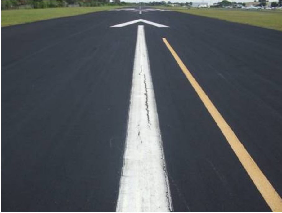
RW 16-34 Section 6110 SU 105: Low Severity L/T Cracking (July 25, 2007)
