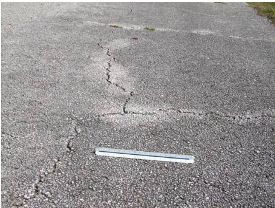
TW D Section 312 SU 303: Medium Severity L/T Cracking (October 16, 2007)
