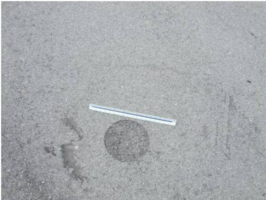
TW E Section 615 SU 602: Low Severity Core patch (October 16, 2007)
