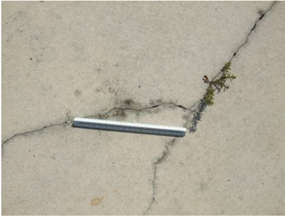
AP SE Section 4305 SU 603: Low Severity Linear Cracking (October 16, 2007)
