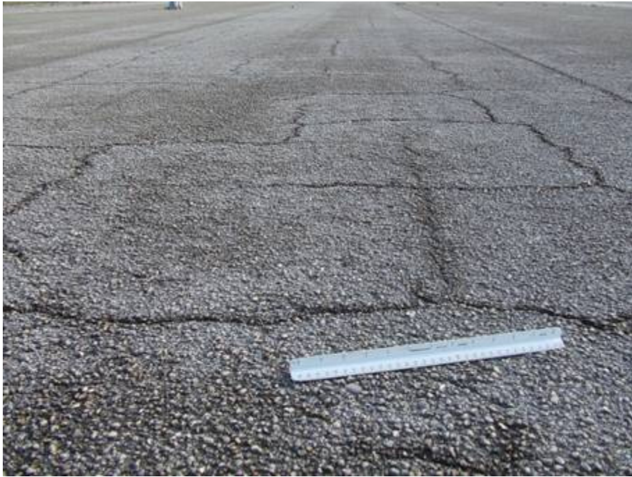
AP Center Section 4125 SU 306: Medium Severity Block Cracking (October 16, 2007)
