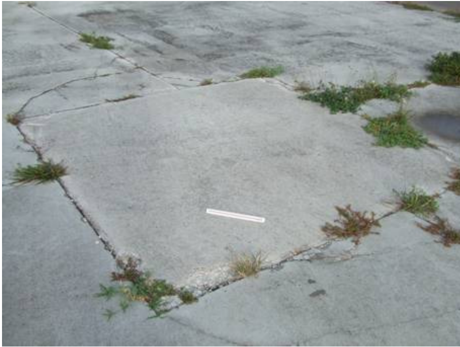
AP Center Section 4112 SU 400: Medium Severity Large Patch (October 16, 2007)
