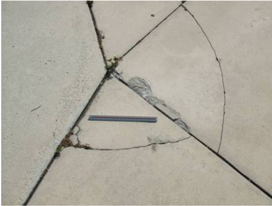
AP SE Section 4305 SU 603: Medium Severity Corner Break (October 16, 2007)
