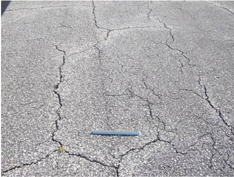
TW A Section 120 SU 402: Medium Severity Block Cracking (October 16, 2007)
