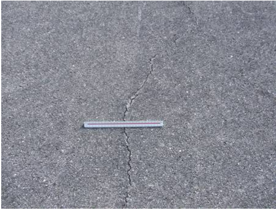
RW 9-27 Section 6120 SU 516: Low Severity L/T Cracking (October 16, 2007)
