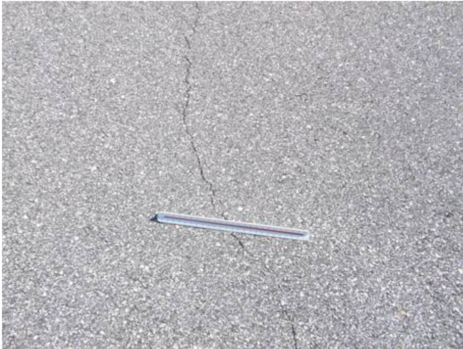
TW D Section 311 SU 301: Low Severity L/T Cracking (October 16, 2007)
