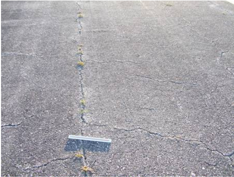
RW 9-27 Section 6110 SU 612: Low Severity Block Cracking (October 16, 2007)
