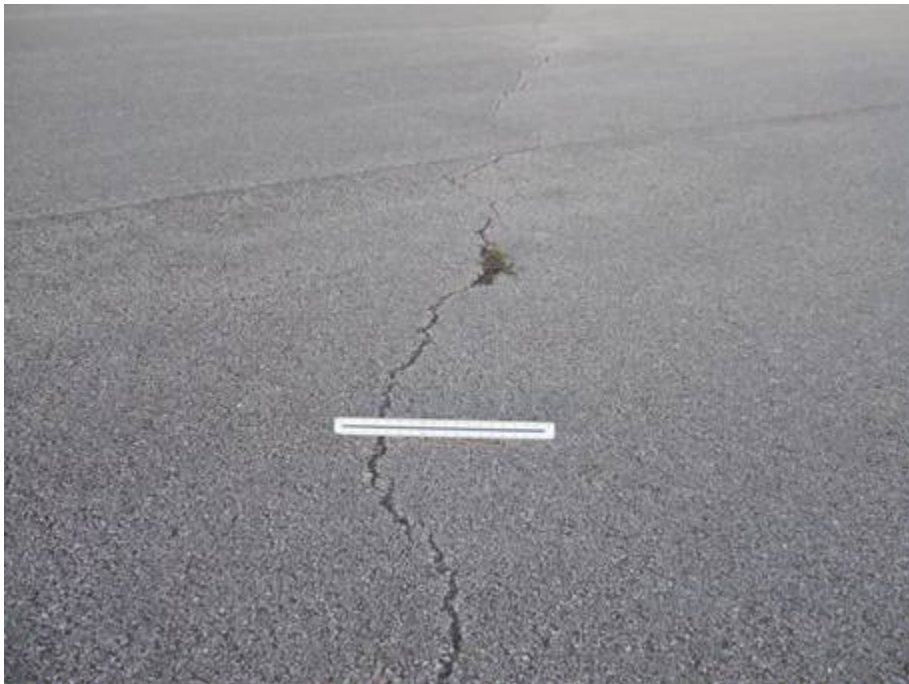
AP Center Section 4105 SU 402: Medium Severity L/T Cracking (October 16, 2007)
