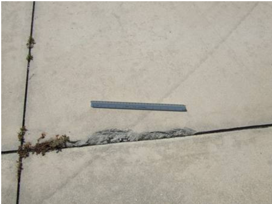
AP SE Section 4305 SU 603: Low Severity Joint Spalling (October 16, 2007)
