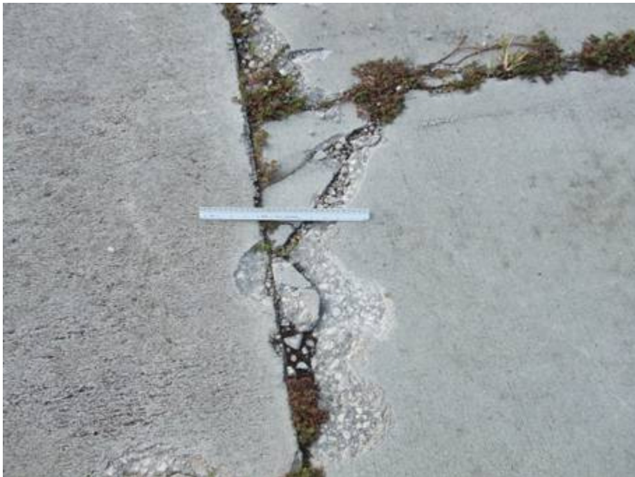
AP Center Section 4112 SU 400: High Severity Joint Spalling (October 16, 2007)
