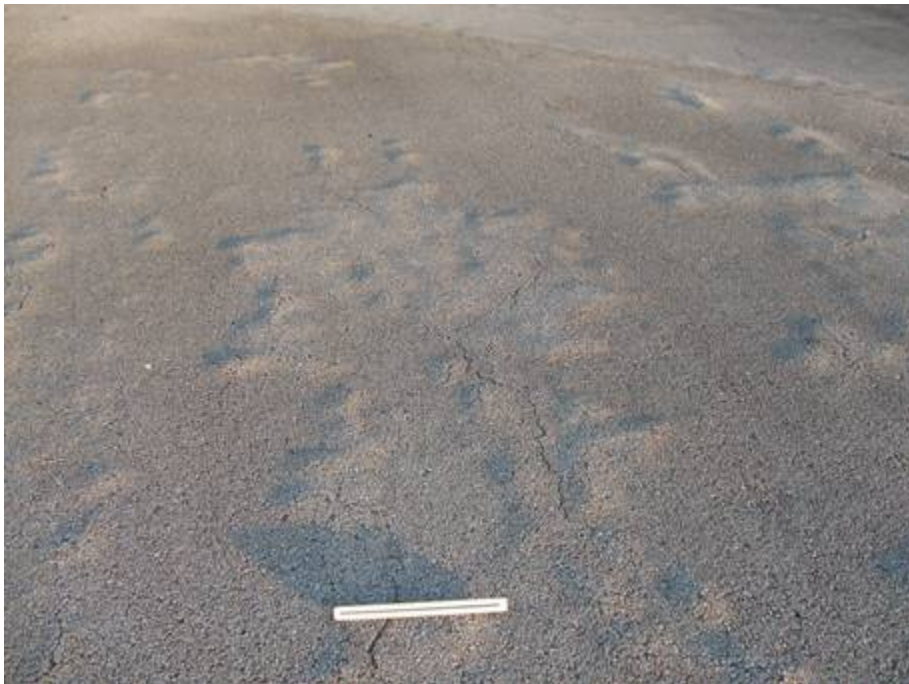
TW D Section 317 SU 331: Low Severity Swelling (October 16, 2007)
