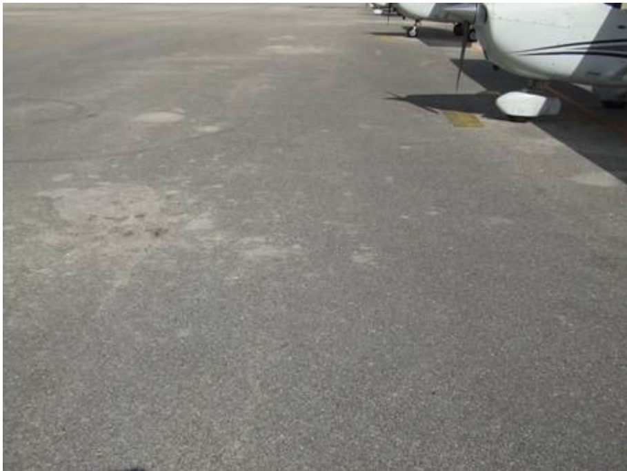
AP GA Section 4115 SU 460: Low Severity Weathering (October 10, 2007)
