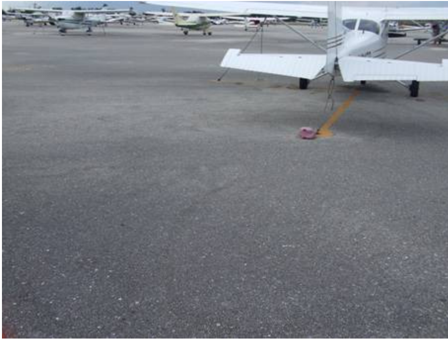
AP GA Section 4110 SU 457: Low Severity Weathering (October 10, 2007)
