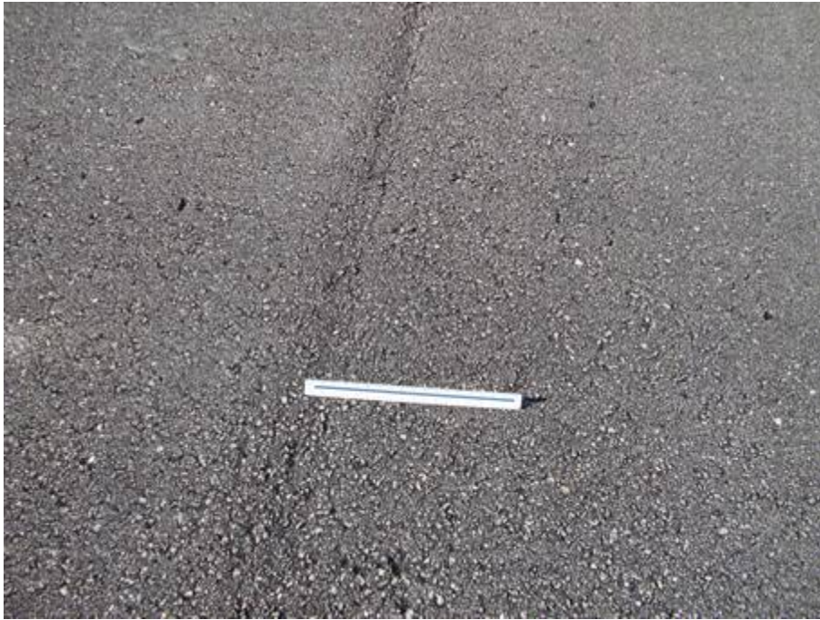
RW 3-21 Section 6305 SU 102: Low Severity Weathering (October 10, 2007)
