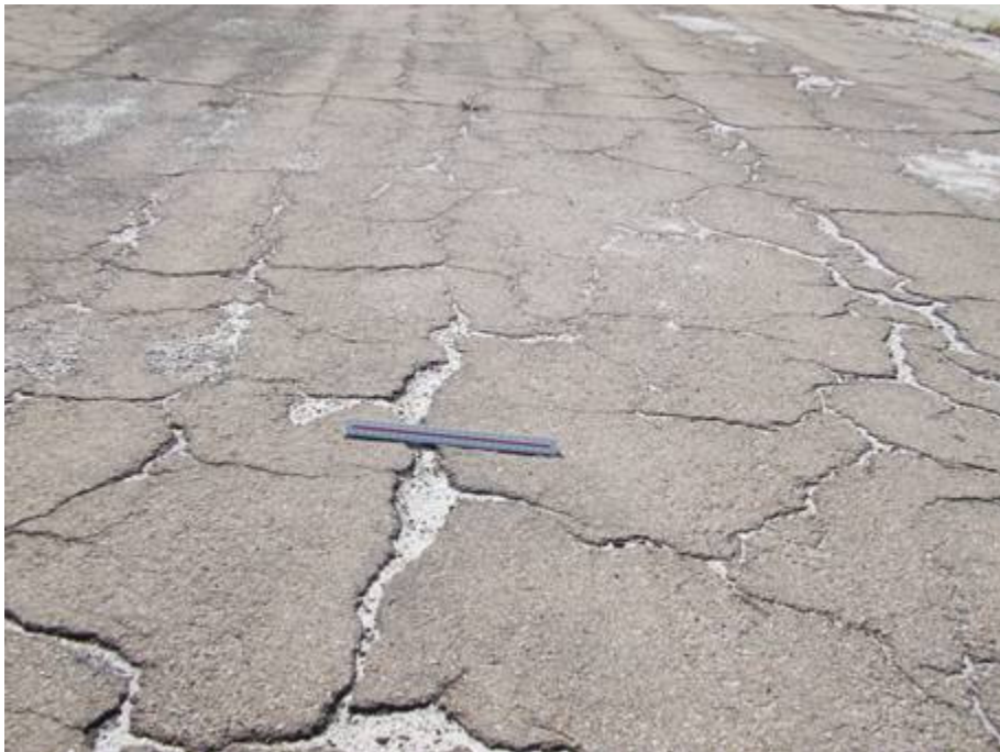
AP RU RW 15 Section 4405 SU 101: High Severity Block Cracking (October 10, 2007)
