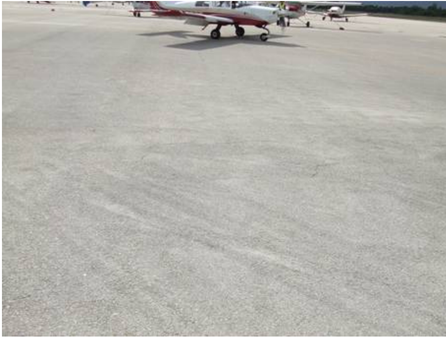
AP GA Section 4115 SU 609: Low Severity Weathering (October 10, 2007)
