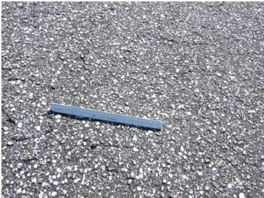
AP T-Hang Section 4205 SU 101: Low Severity Weathering (September 17, 2007)
