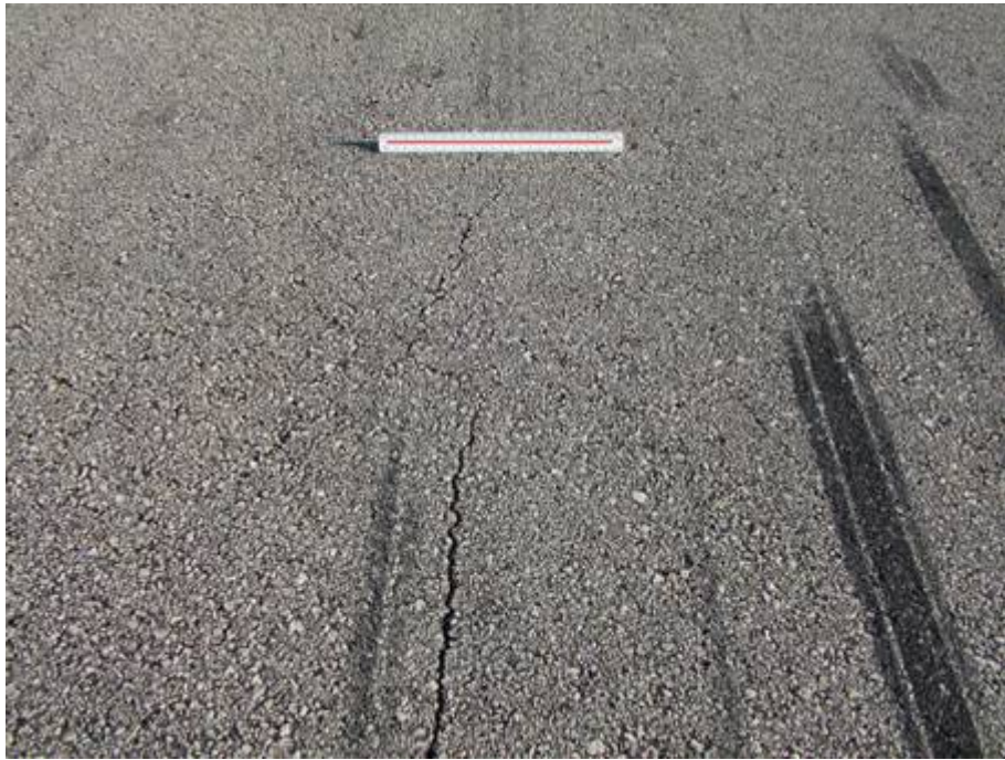
RW 17-35 Section 6105 SU 109: Low Severity L/T Cracking (September 17, 2007)
