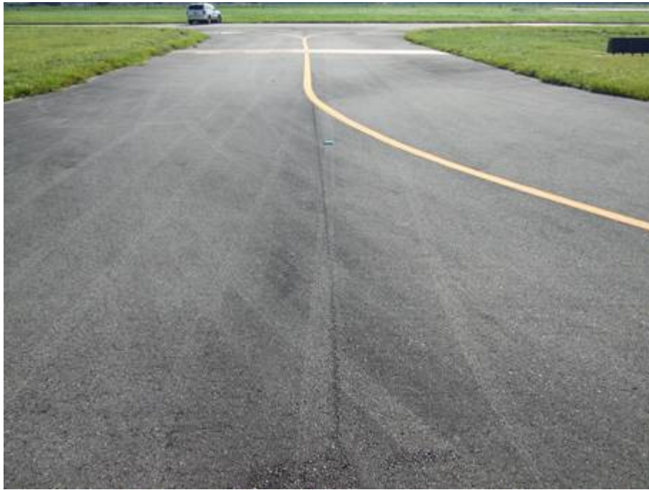
TW Section 125 SU 100: Low Severity L/T Cracking (September 17, 2007)
