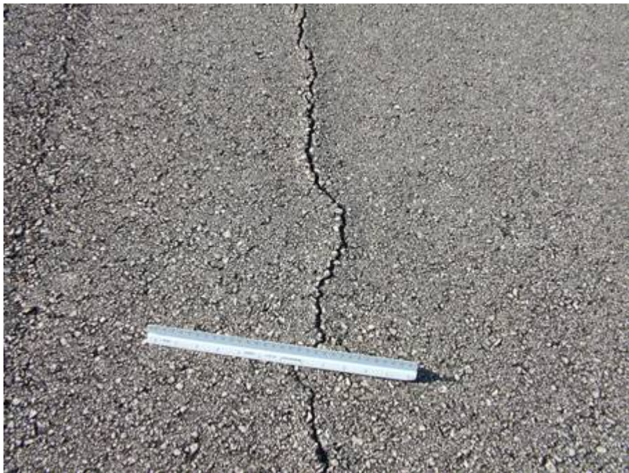
RW 17-35 Section 6110 SU 155: Low Severity L/T Cracking (September 17, 2007)
