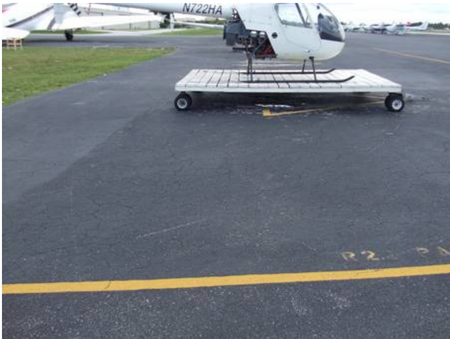
AP S Section 4120 SU 717: Low Severity Weathering (October 10, 2007)
