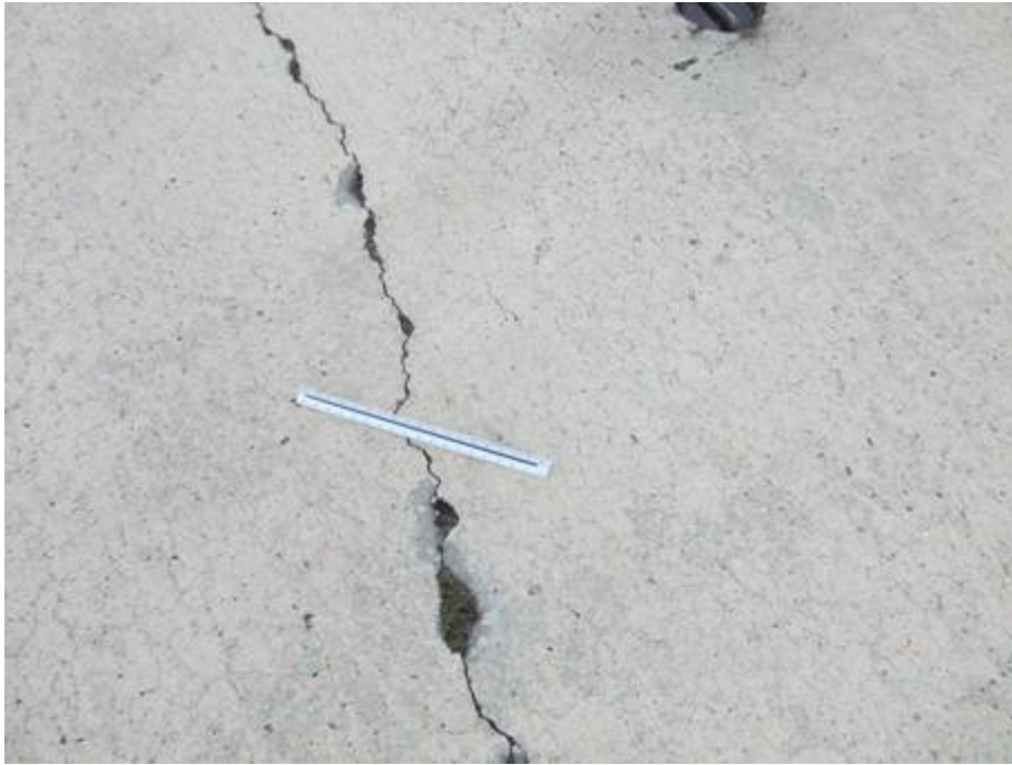
AP S Section 4130 SU 306: Medium Severity Linear Cracking (October 10, 2007)
