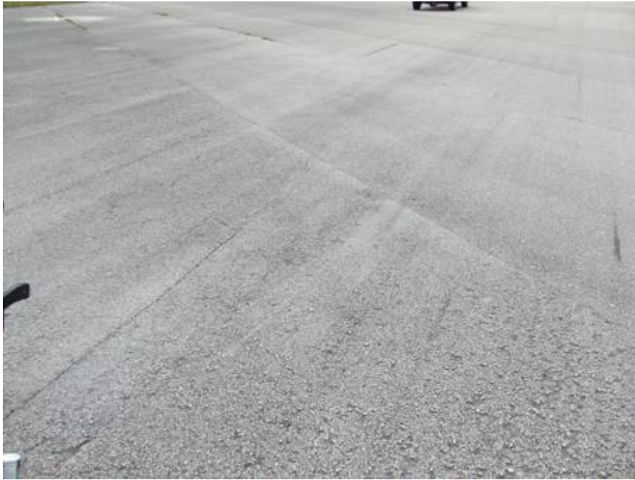
RW 15-33 Section 6315 SU 312: Low Severity Weathering and L/T Cracking (October 10, 2007)
