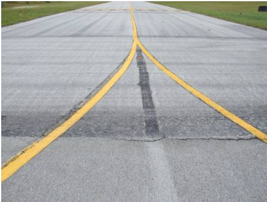
TW F Section 615 SU 612: Low Severity L/T Cracking (October 10, 2007)
