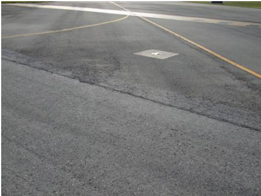
TW L Section 1205 SU 111: Low Severity L/T Cracking and Weathering (October 10, 2007)
