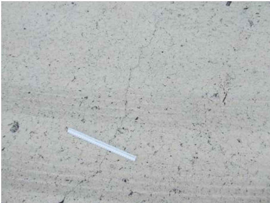
AP S Section 4130 SU 306: Shrinkage Cracking (October 10, 2007)
