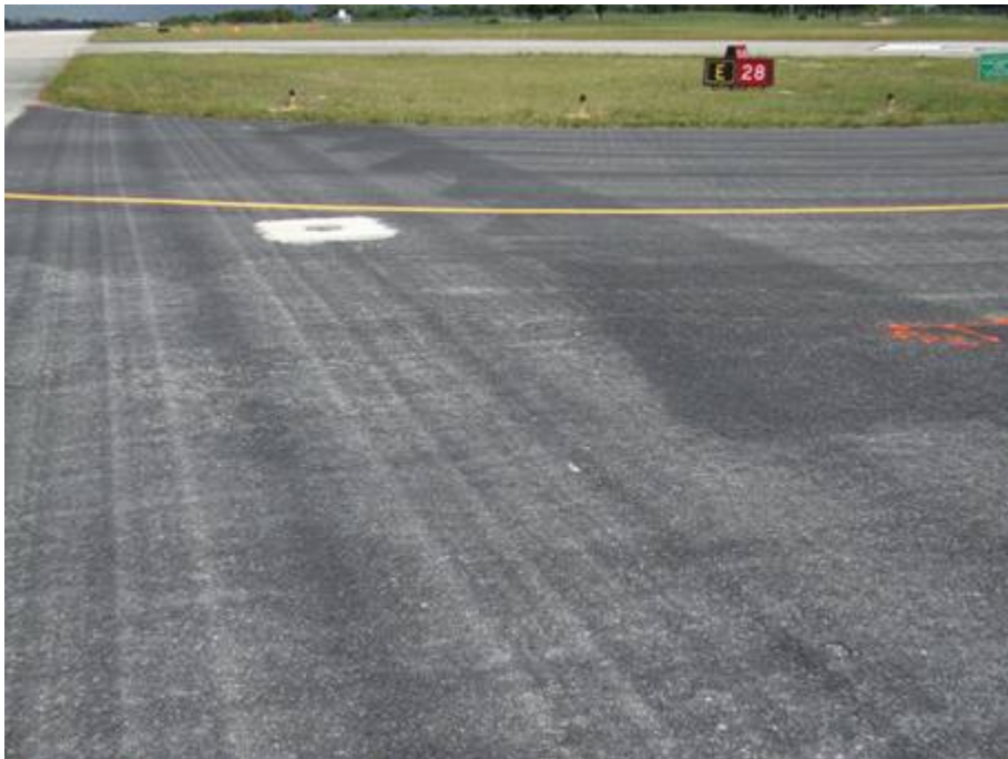
TW E Section 510 SU 502: Low Severity Weathering (October 10, 2007)
