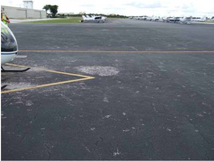
AP S Section 4115 SU 716: Medium Severity Weathering (October 10, 2007)
