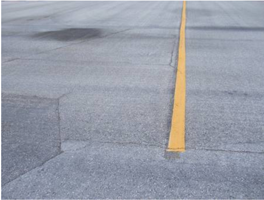
RW 6-24 Section 6211 SU 100: Low Severity L/T Cracking/Patching (October 10, 2007)
