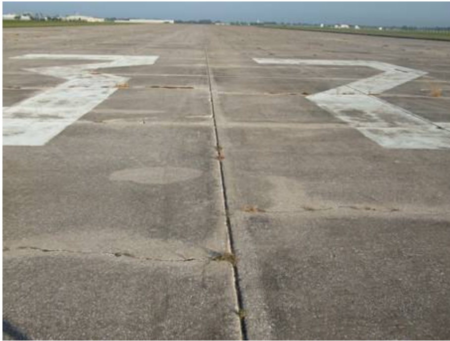
RW 14-32 Section 6205 SU 101: Low Severity Linear Cracking, High Severity Joint Seal Damage (September 17, 2007)
