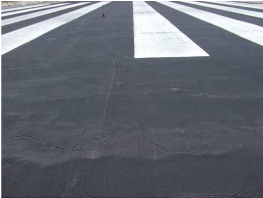
RW 18-36 Section 6105 SU 203: Low Severity Block Cracking (September 17, 2007)
