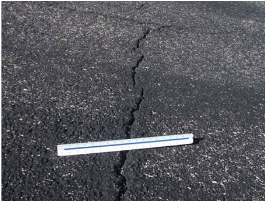
RW 14-32 Section 6210 SU 159: Medium Severity L/T Cracking (September 17, 2007)
