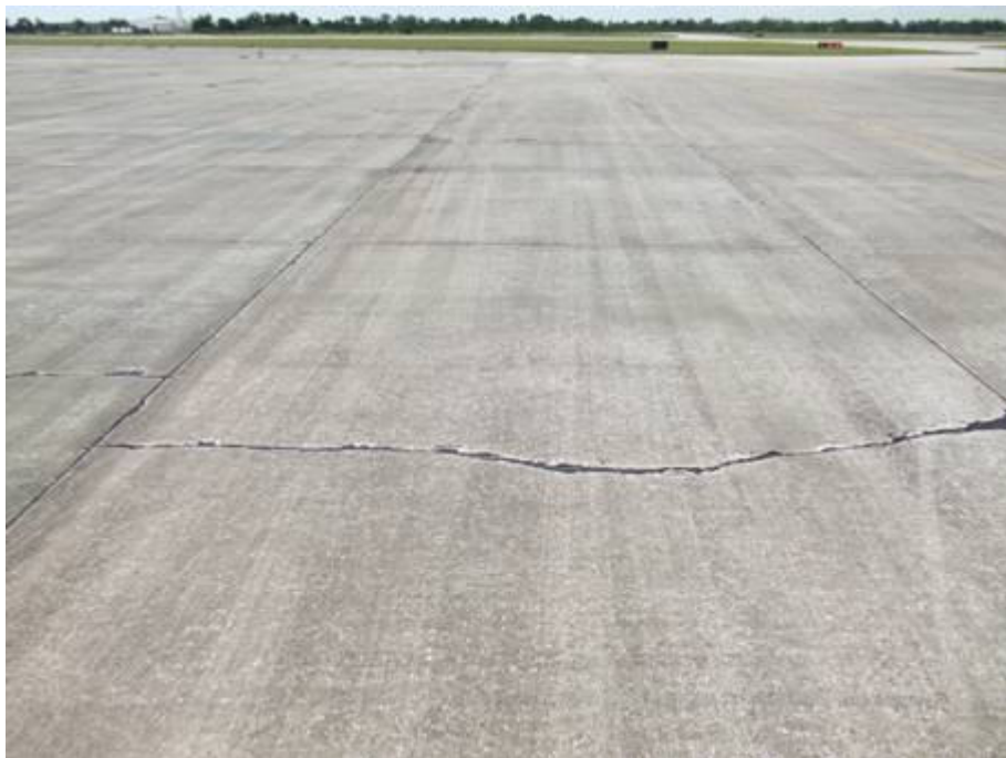
AP W Section 4105 SU 302: Medium Severity Linear Cracking (September 17, 2007)
