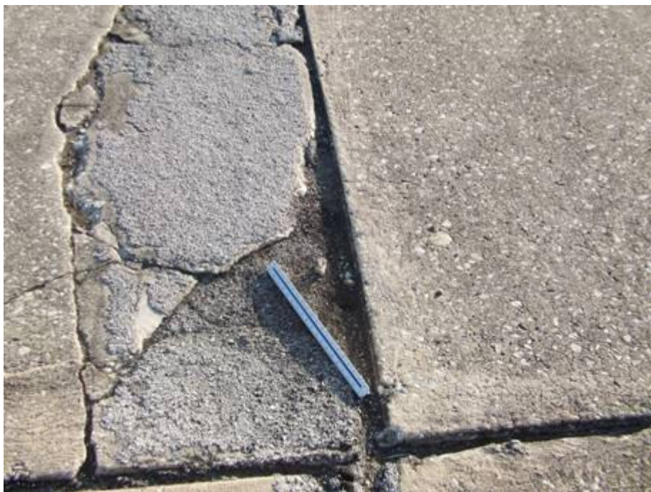
RW 14-32 Section 6205 SU 101: High Severity Corner Spall (September 17, 2007)
