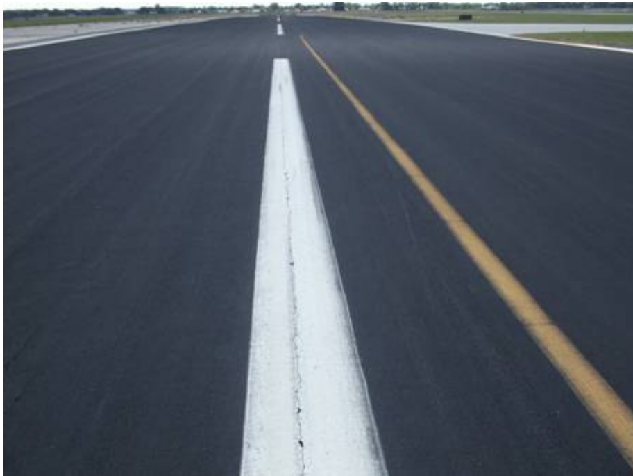
RW 18-36 Section 6105 SU 138: Low Severity L/T Cracking (September 17, 2007)
