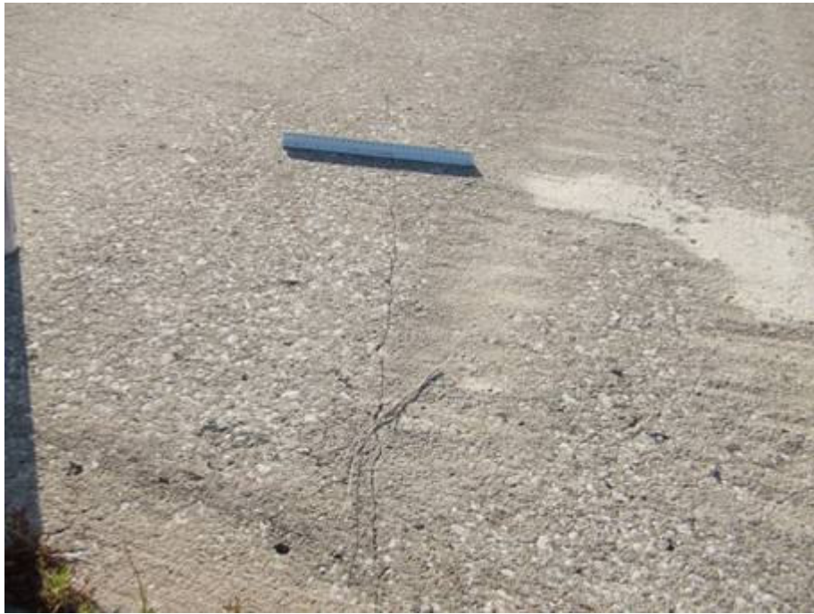
RW 14-32 Section 6205 SU 128: Shrinkage Cracking (Sept. 17, 2007)
