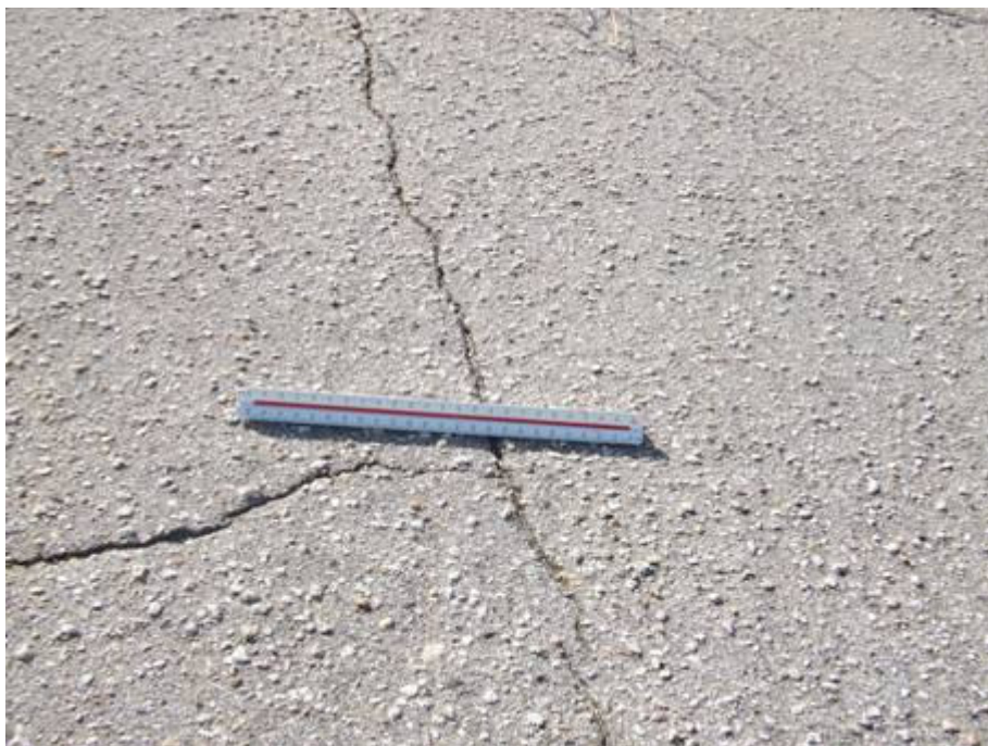
RW 14-32 Section 6215 SU 198: Medium Severity L/T Cracking, Low Severity Weathering (September 17, 2007)
