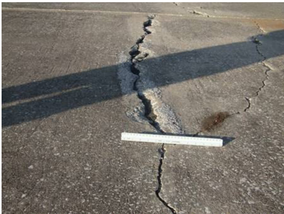
RW 14-32 Section 6205 SU 101: High Severity Linear Cracking (September 17, 2007)
