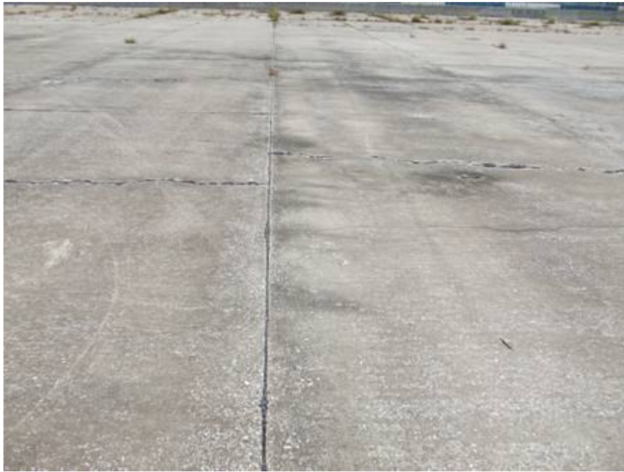
AP W Section 4105 SU 302: Low Severity Joint Seal Damage (September 17, 2007)
