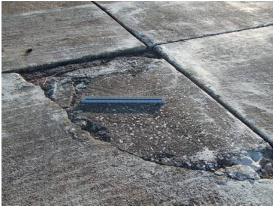
RW 14-32 Section 6205 SU 101: High Severity Corner Break (September 17, 2007)
