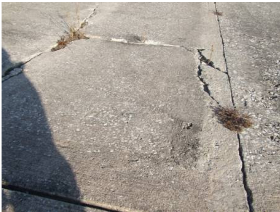
RW 14-32 Section 6205 SU 121: High Severity Shattered Slab (September 17, 2007)
