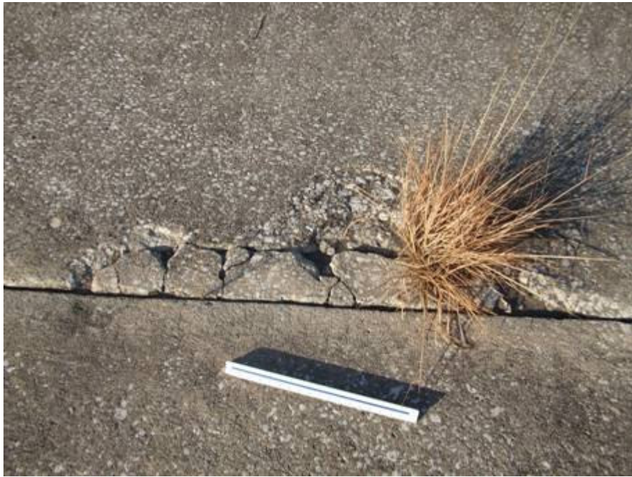
RW 14-32 Section 6205 SU 105: High Severity Joint Spall (September 17, 2007)
