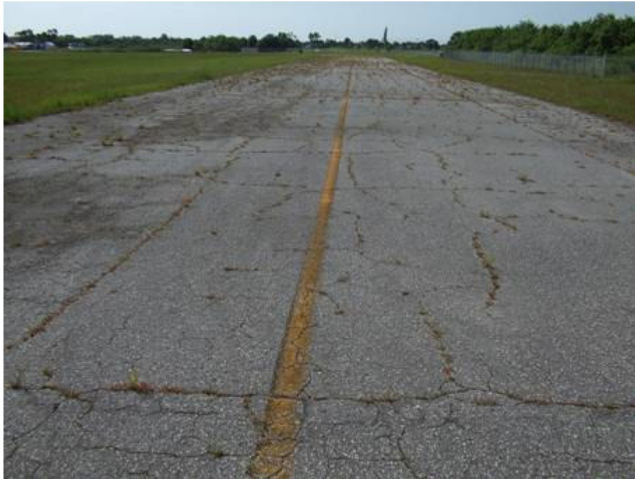
TW 2 Section 205 SU 200: Medium Severity Block Cracking (July 9, 2007)
