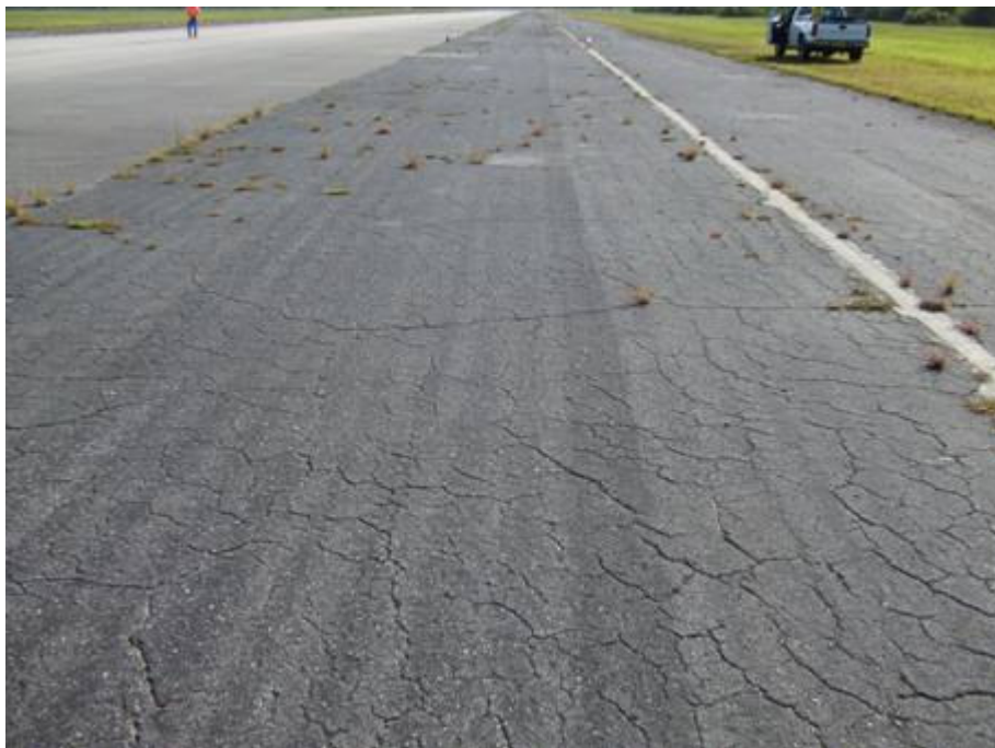
RW 4-22 Section 6210 SU 504: Medium Severity Block Cracking (July 9, 2007)
