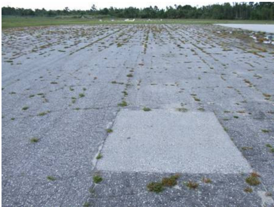
TW 4 Section 410 SU 435: Medium Severity Block Cracking (July 9, 2007)
