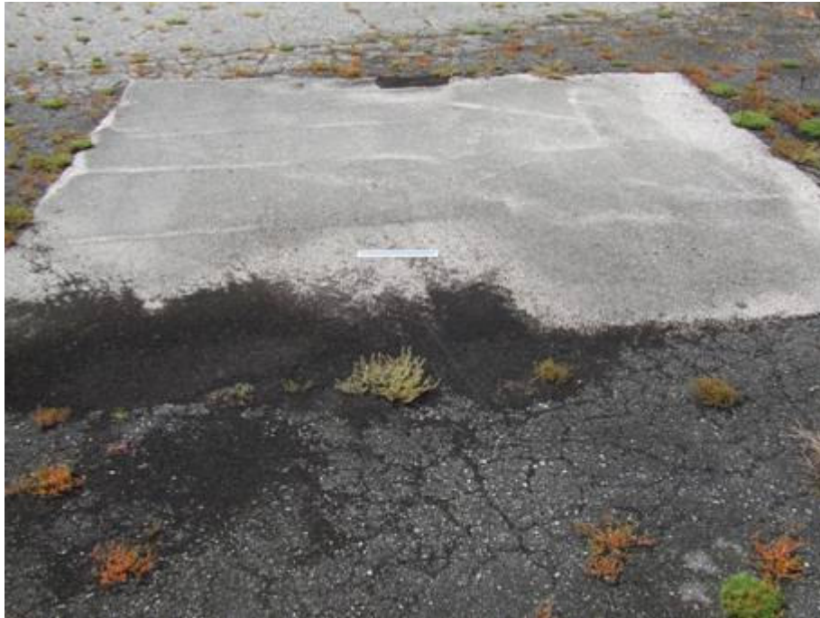
TW 3 Section 306 SU 101: Low Severity Patch (July 9, 2007)
