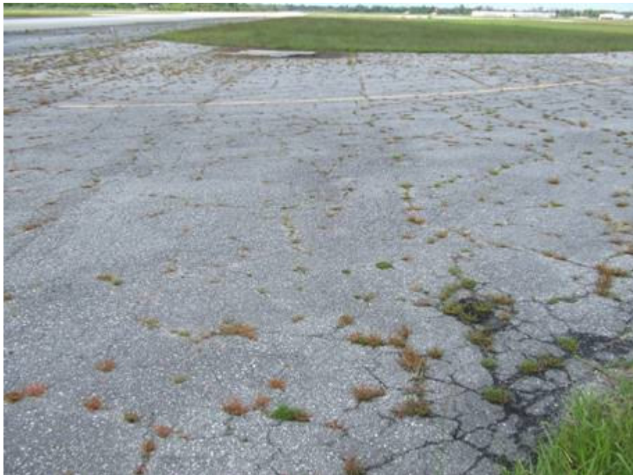
TW 3 Section 306 SU 101: Medium Severity Block Cracking (July 9, 2007)
