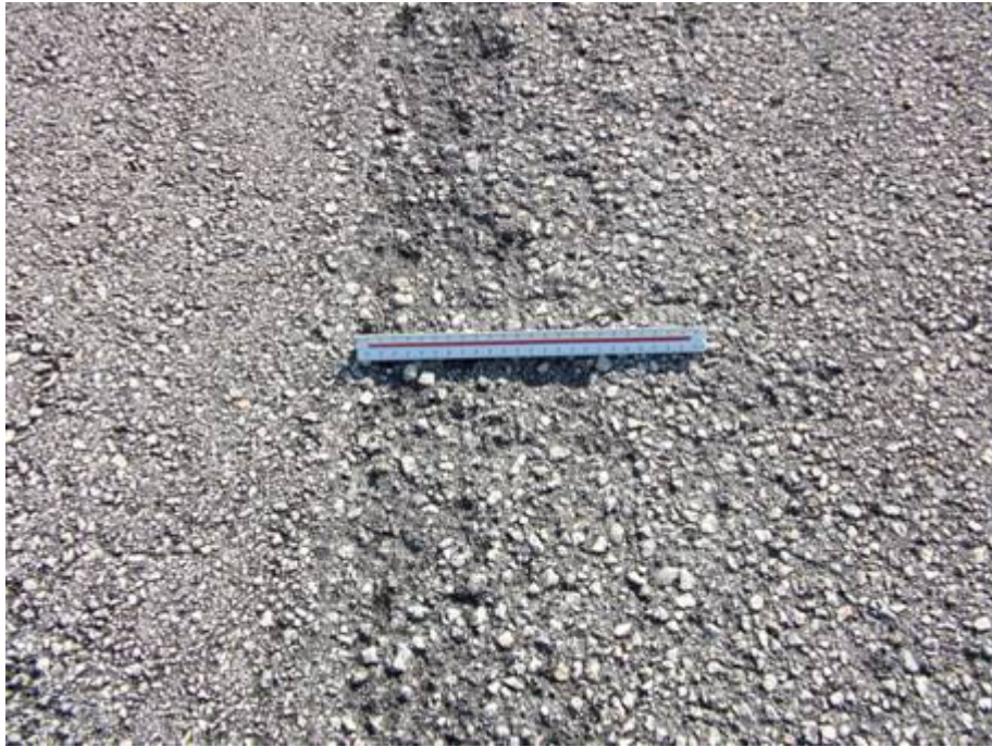
RW 4-22 Section 6205 SU 314: Medium Severity Weathering (July 9, 2007)
