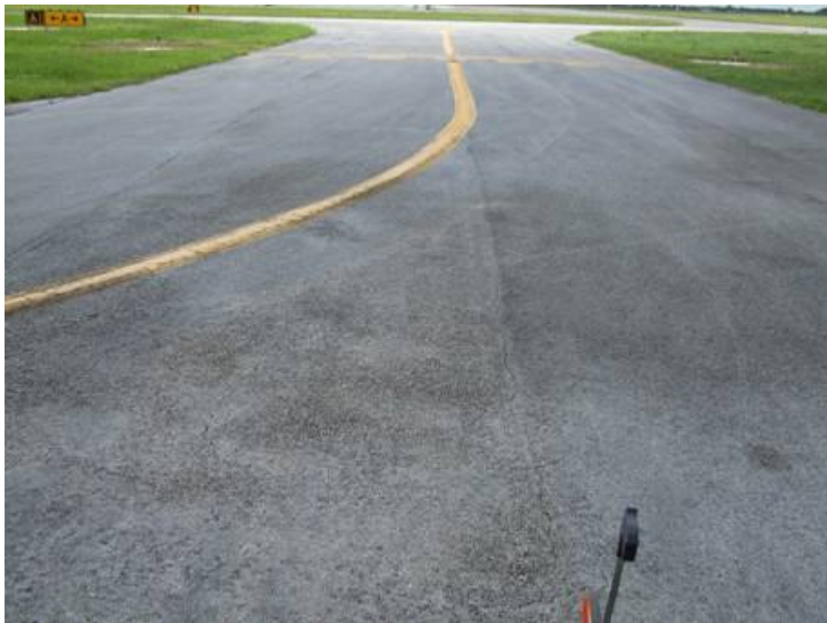
TW N Section 280 SU 300: Low Severity L/T Cracking (September 17, 2007)
