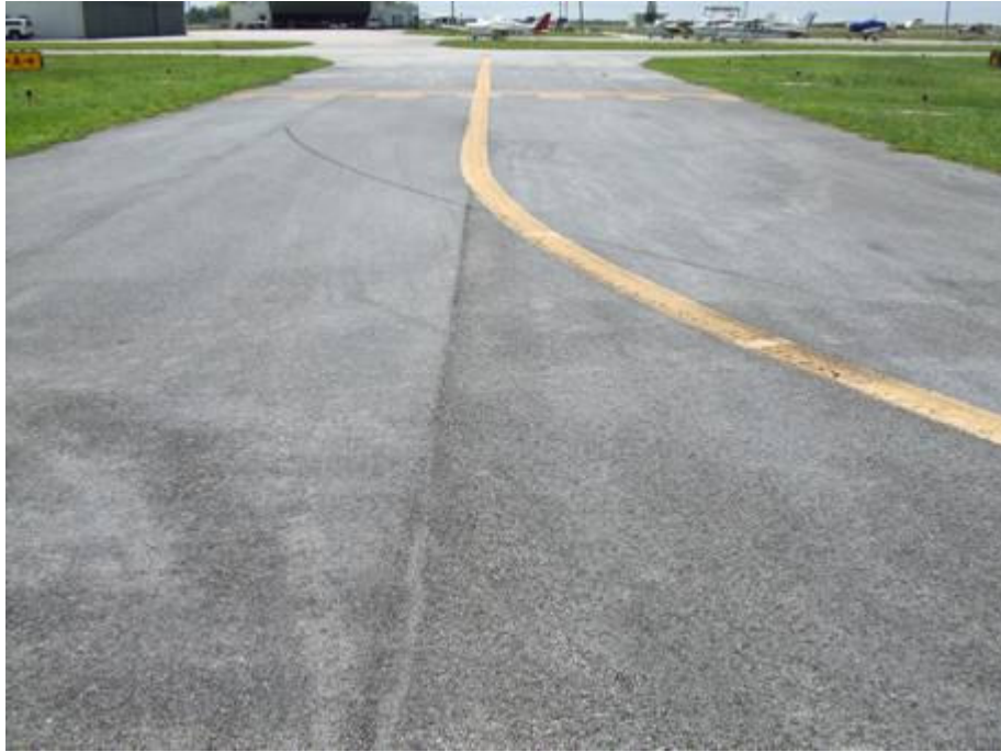
TW N Section 250 SU 301: Low Severity L/T Cracking (September 17, 2007)
