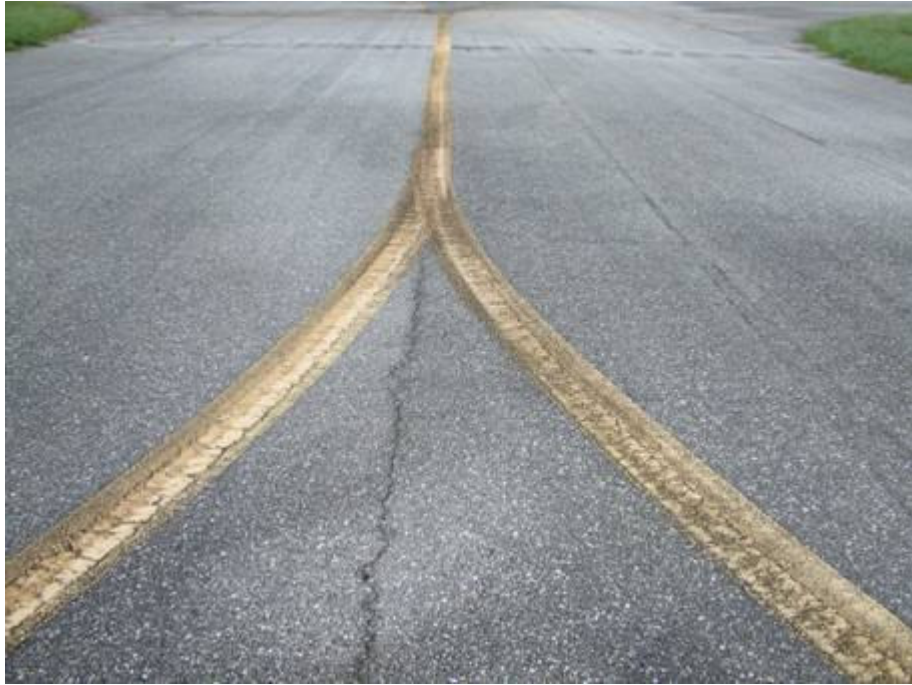
TW E Section 140 SU 401: Low Severity L/T Cracking (September 17, 2007)
