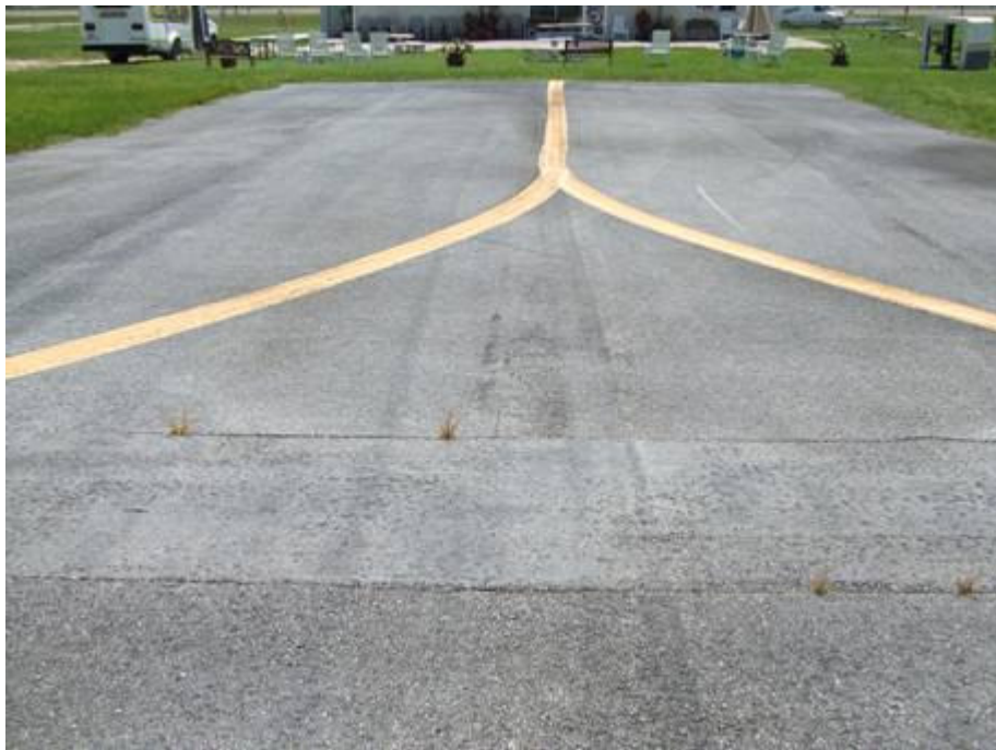
TW N Section 295 SU 500: Low Severity Patching (September 17, 2007)
