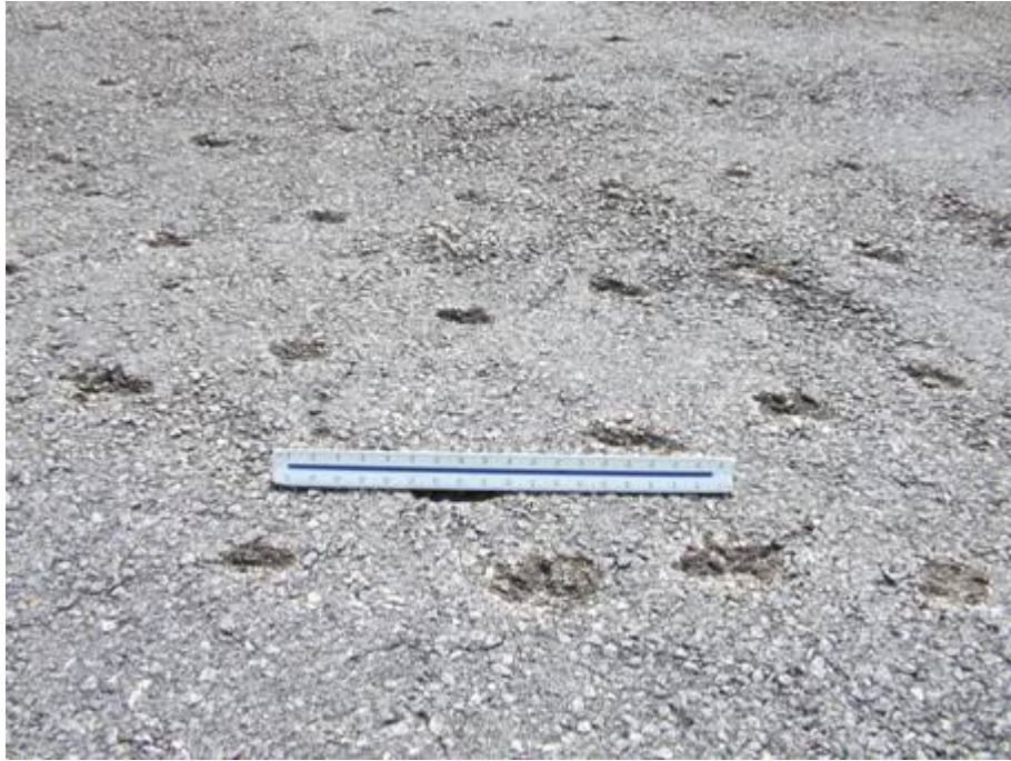
TW N Section 280 SU 300: Medium Severity Weathering (September 17, 2007)
