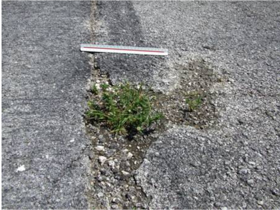
TW N Section 295 SU 500: High Severity Weathering (September 17, 2007)
