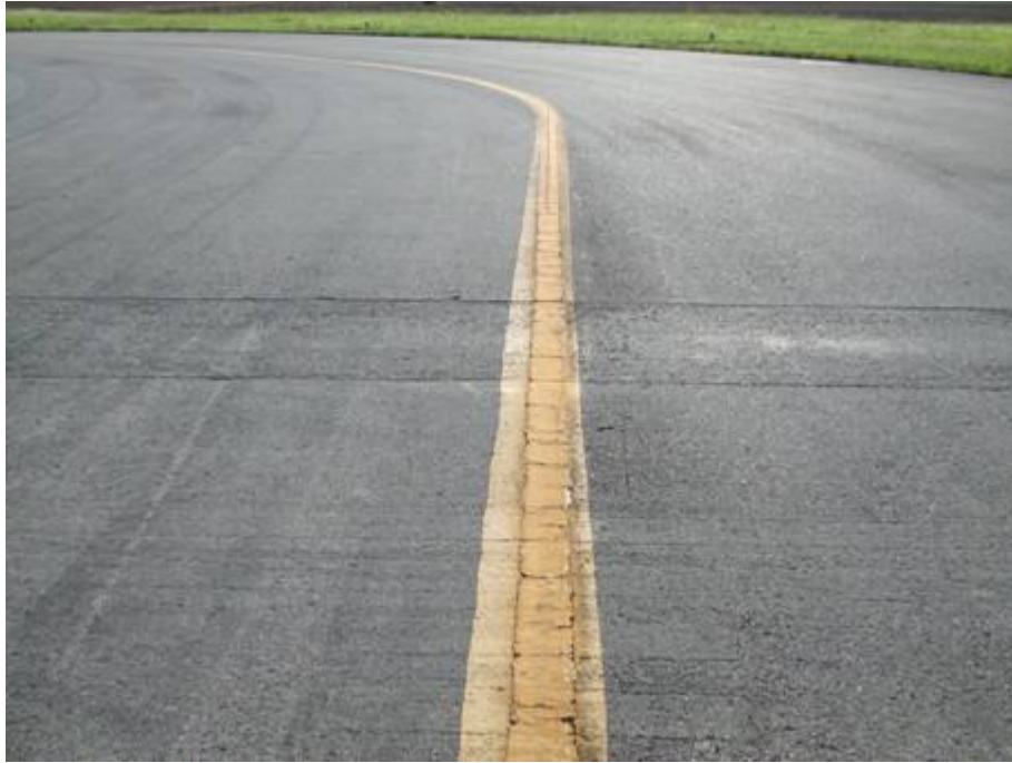
TW E Section 110 SU 202: Low Severity Patching (September 17, 2007)
