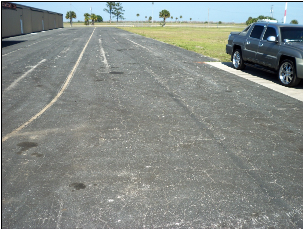
Apron, Section 4105, Sample Unit 150 – Low severity (43) Block Cracking, (49) Oil Spillage, low and medium severity (52) Weathering and Raveling
