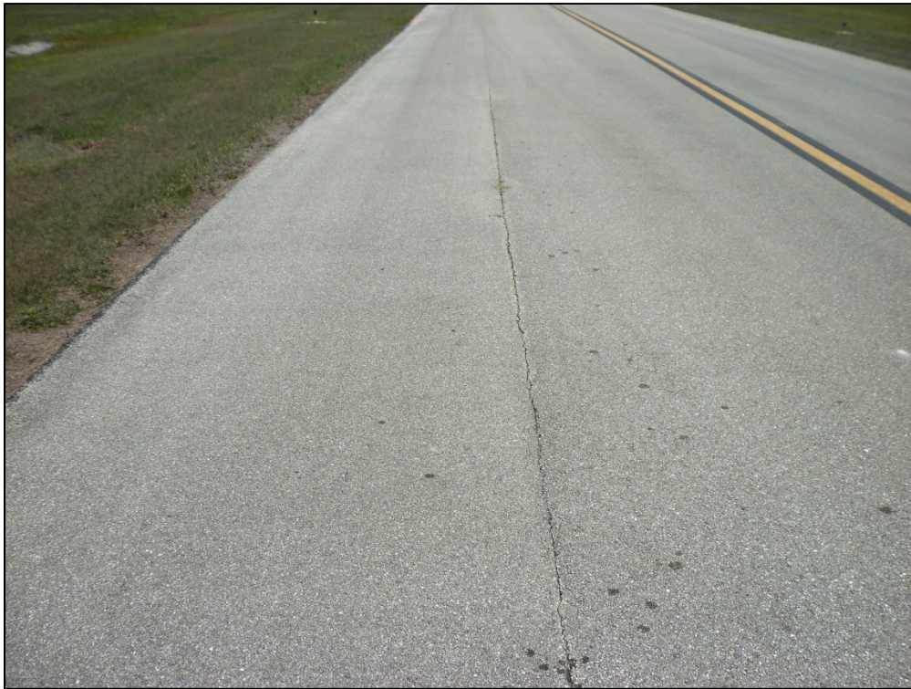
Taxiway Connector A1, Section 105, Sample Unit 102 – Low severity (48) Longitudinal and Transverse Cracking, low severity (52) Weathering and Raveling
