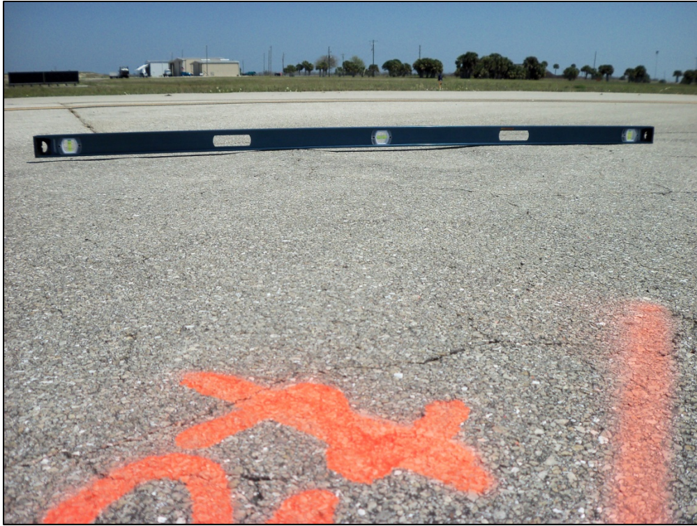
Taxiway Alpha, Section 103, Sample Unit 121 – Low severity (48) Longitudinal and Transverse Cracking, low severity (52) Weathering and Raveling, low severity (56) Swelling
