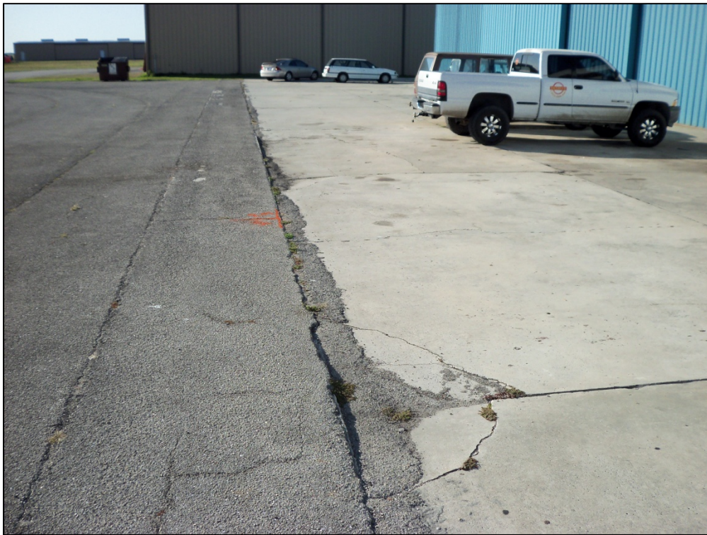
Apron, Section 4205, Sample Unit 100 – Low and medium severity (62) Corner Break, (63) LTD Cracking, (65) Joint Seal Damage, (70) Sealing/Map Cracking, (72) Shattered Slabs, (73) Shrinkage Cracks, (74) Joint Spalling, (75) Corner Spalling
