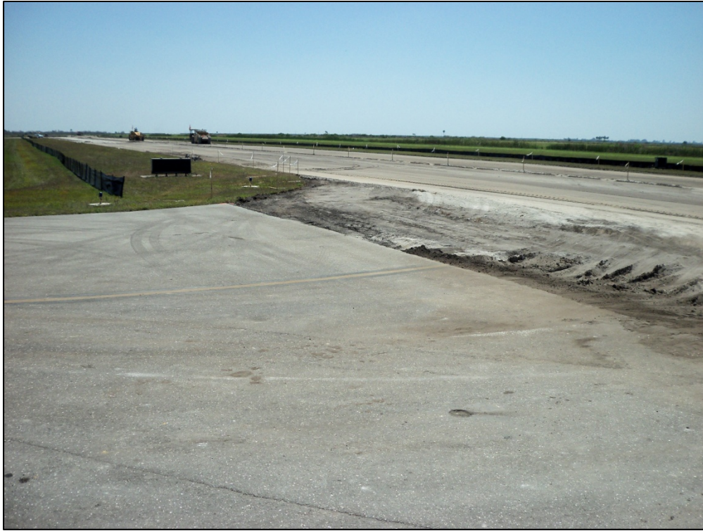
Taxiway Connector A2, Section 210, Sample Unit 100 – Low severity (48) Longitudinal and Transverse Cracking, (49) Oil Spillage, low severity (52) Weathering and Raveling
