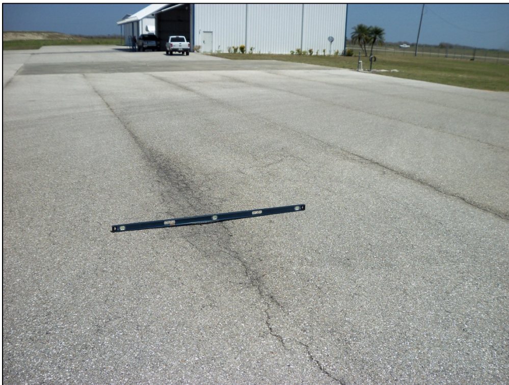
Apron NW, Section 4405, Sample Unit 305 – Low severity (43) Block Cracking, medium severity (45) Depression, low and medium severity (48) Longitudinal and Transverse Cracking, low and medium severity (52) Weathering and Raveling
