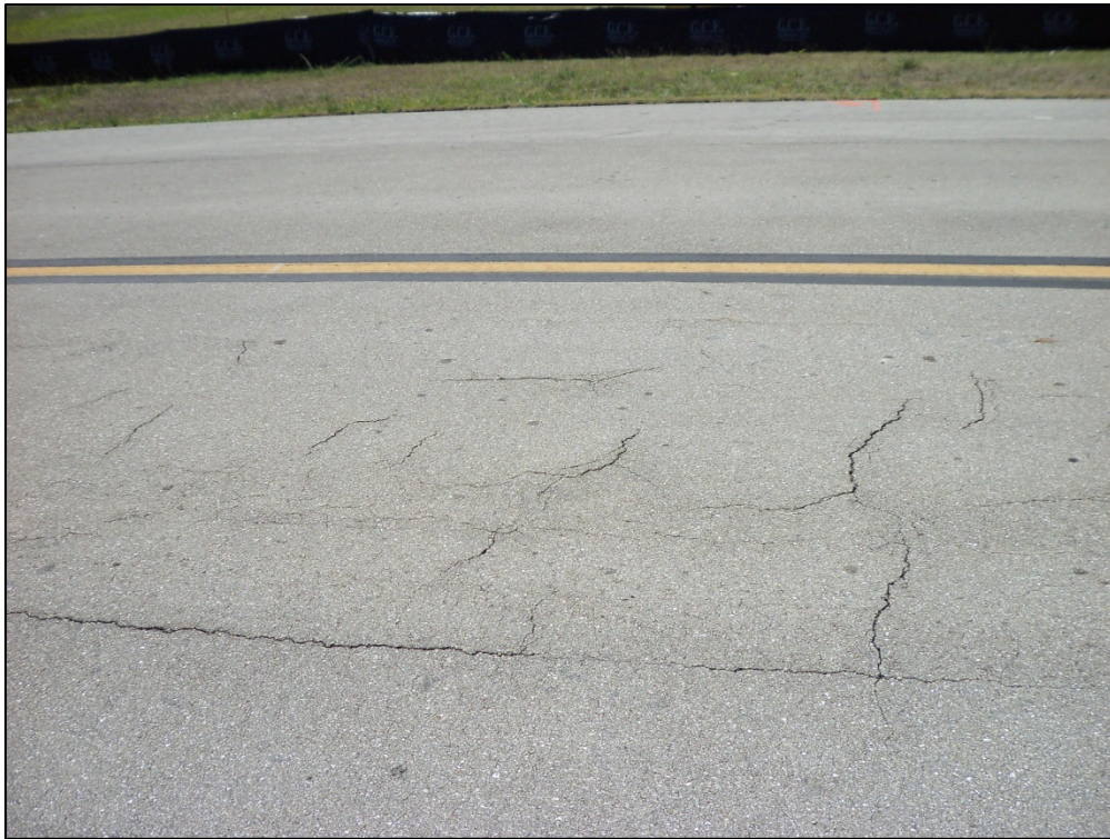
Taxiway Alpha, Section 120, Sample Unit 119 – Low severity (43) Block Cracking, low and medium severity (48) Longitudinal and Transverse Cracking, low severity (52) Weathering and Raveling
