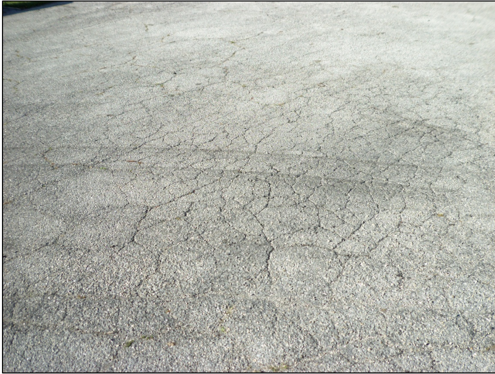
Apron, Section 405, Sample Unit 103 – Low and medium severity (43) Block Cracking, medium and high severity (52) Weathering and Raveling
