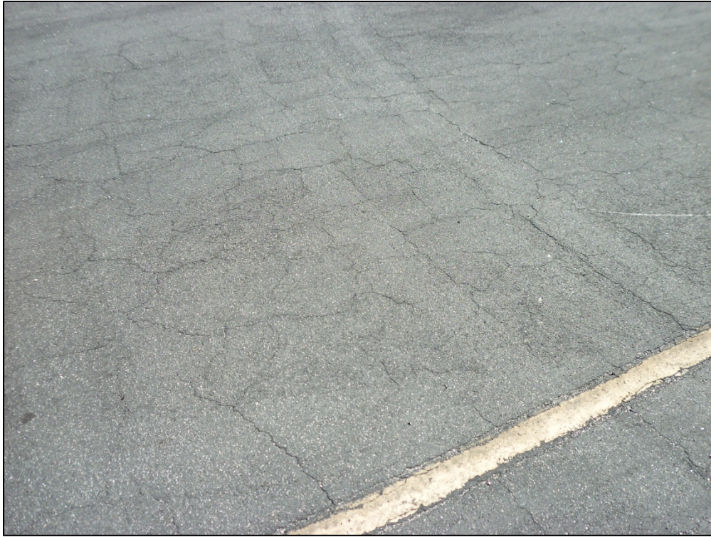
Apron, Section 4105, Sample Unit 402 – Low severity (50) Patch, low and medium severity (52) Weathering and Raveling
