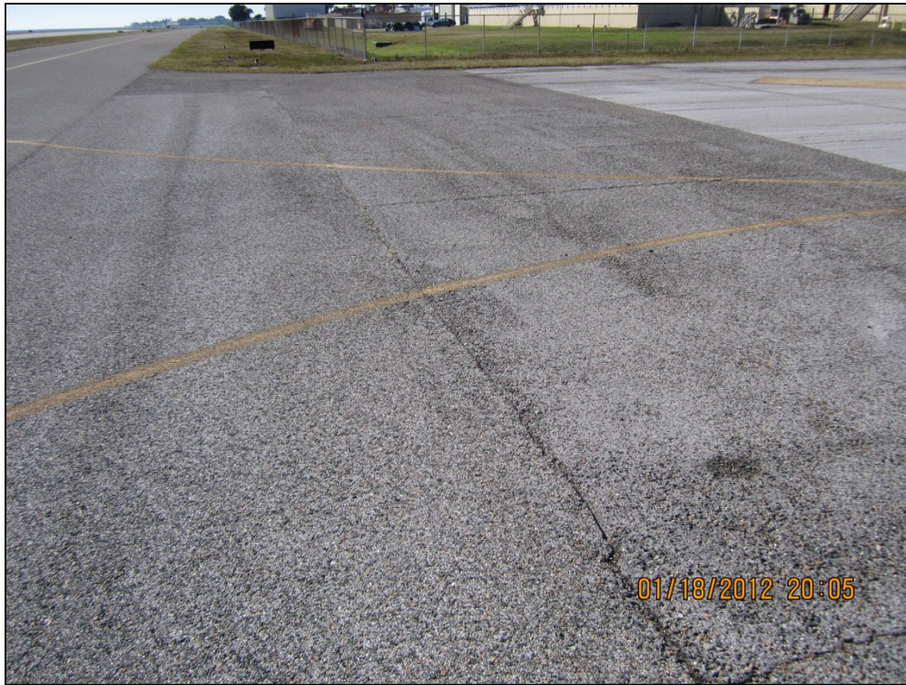
Taxiway Charlie, Section 301, Sample Unit 100 – Low and medium severity (48) Longitudinal and Transverse Cracking: low, medium and high severity (52) Weathering and Raveling
