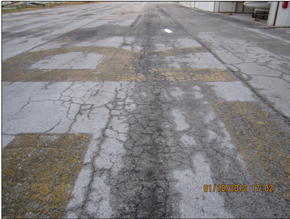
Taxiway Charlie, Section 305, Sample Unit 106 – Low severity (43) Block Cracking, medium severity (41) Alligator Cracking, low, medium and high severity (52) Weathering and Raveling
