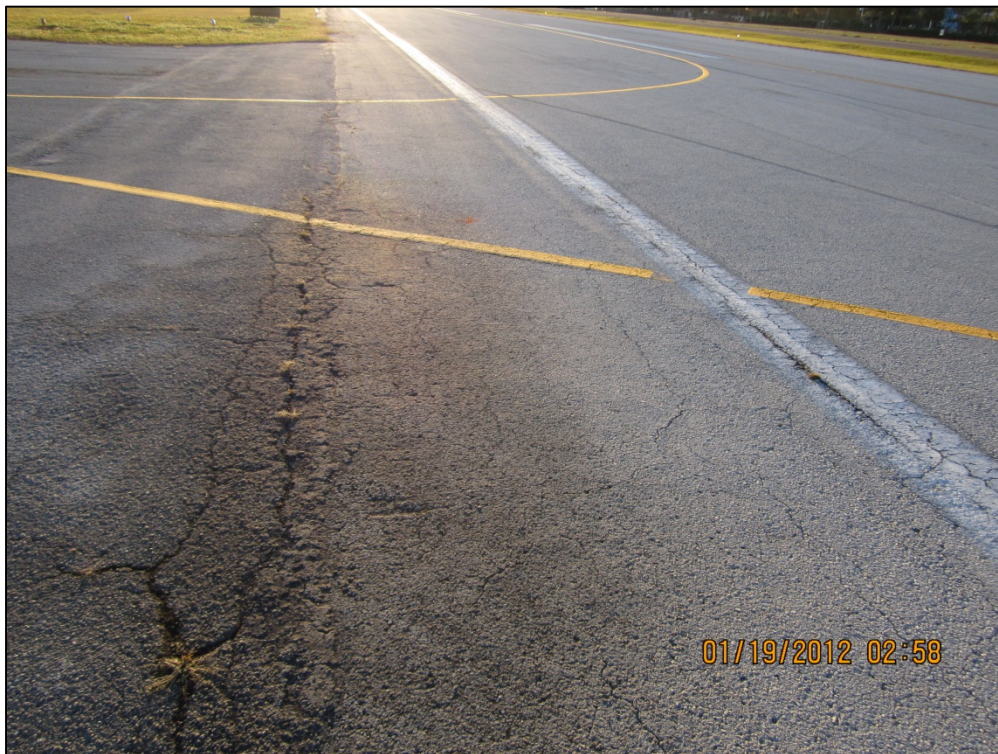
Taxiway A1, Section 609, Sample Unit 99 – Low severity (48) Longitudinal and Transverse Cracking, medium severity (45) Depression, low severity (52) Weathering and Raveling
