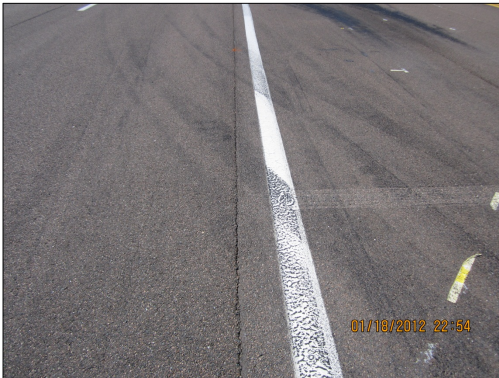
West Apron, Section 4210, Sample Unit 115 – Low severity (48) Longitudinal and Transverse Cracking
