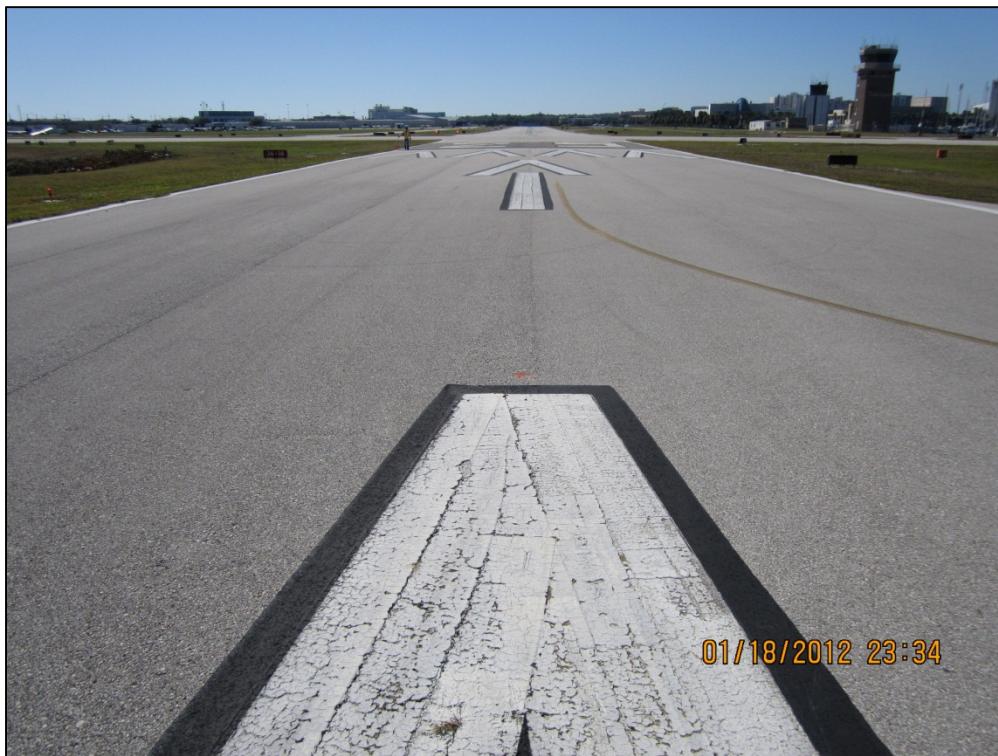
Runway 7-25, Section 6215, Sample Unit 101 – Low severity (48) Longitudinal and Transverse Cracking, low severity (52) Weathering and Raveling
