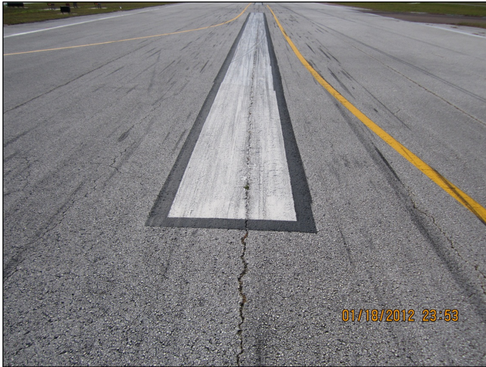
Runway 7-25, Section 6210, Sample Unit 114 – Low and medium severity (48) Longitudinal and Transverse Cracking, low severity (52) Weathering and Raveling
