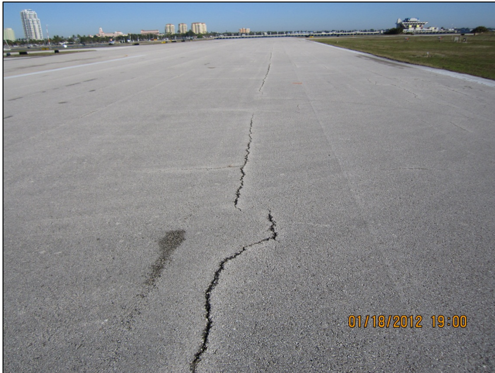
Runway 18-36, Section 6105, Sample Unit 335 – Low and medium severity (48) Longitudinal and Transverse Cracking, low severity (52) Weathering and Raveling
