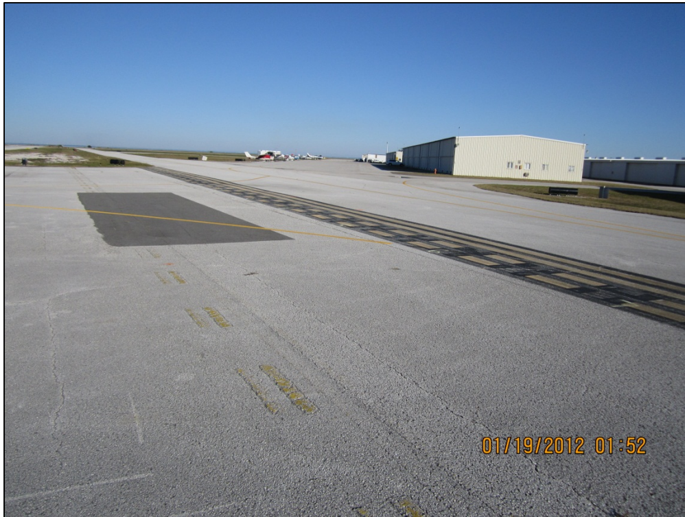
Taxiway Alpha, Section 310, Section 150 – Low and medium severity (48) Longitudinal and Transverse Cracking, medium severity (50) Patch, low severity (52) Weathering and Raveling
