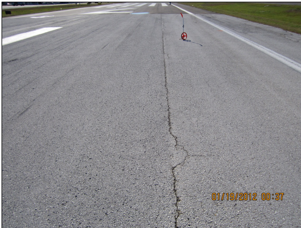
Runway 7-25, Section 6210, Sample Unit 155 – Low and medium severity (48) Longitudinal and Transverse Cracking, low severity (52) Weathering and Raveling
