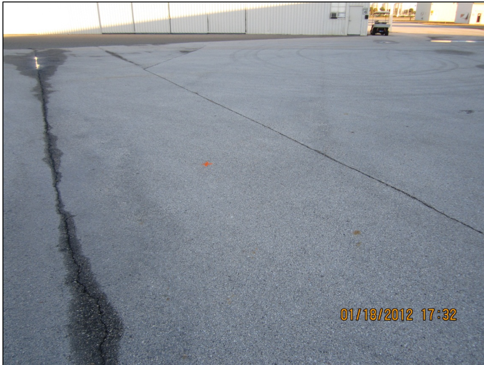
Southwest Apron, Section 4120, Sample Unit 211 – Low severity (48) Longitudinal and Transverse Cracking, low severity (52) Weathering and Raveling
