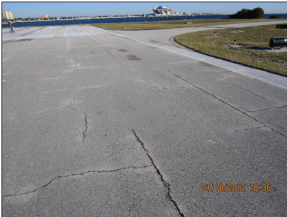
Runway 18-36, Section 6110, Sample Unit 552 – Low severity (48) Longitudinal and Transverse Cracking, low severity (43) Block Cracking, low severity (52) Weathering and Raveling
