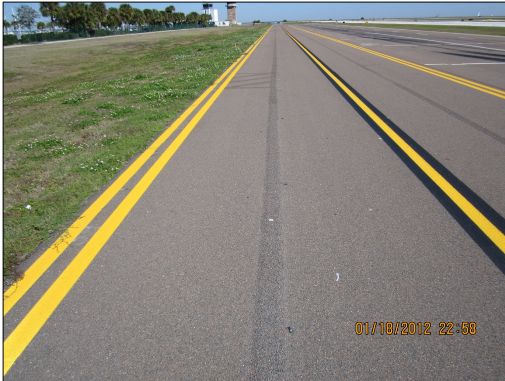
Taxiway Delta, Section 510, Sample Unit 232 – Low severity (52) Weathering and Raveling
