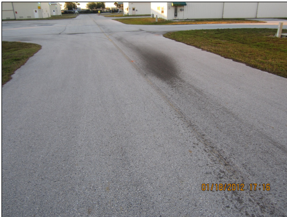
T-Hangars Apron, Section 4135, Sample Unit 154 – Low severity (48) Longitudinal and Transverse Cracking, (49) Oil Spillage, low severity (52) Weathering and Raveling
