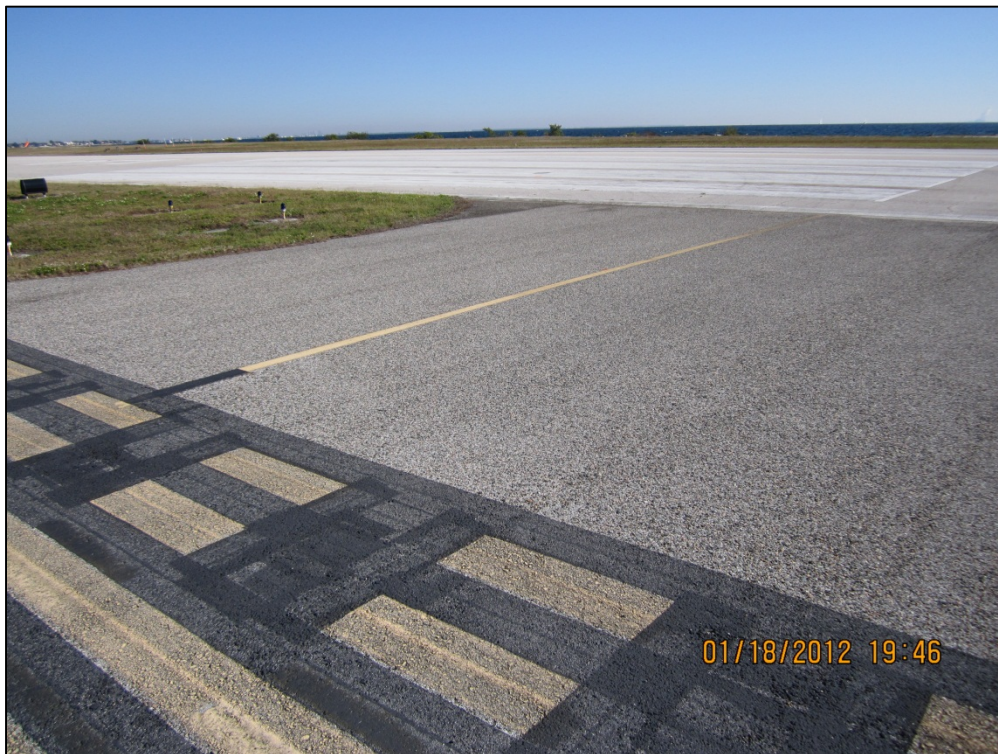
Taxiway Bravo, Section 250, Sample Unit 100 – Low and medium severity (52) Weathering and Raveling
