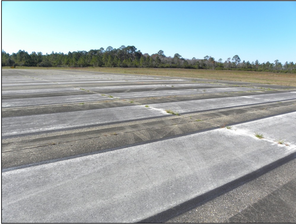
Runway 13-31, Section 6105, Sample Unit 384 – Low, medium and high severity (63) Longitudinal/Transverse/Diagonal Cracking, medium severity (65) Joint Seal Damage, low and medium severity (74) Joint Spalling
