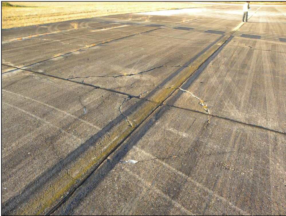
Taxiway B5, Section 335, Sample Unit 103 – Medium and high severity (62) Corner Spalling, low, medium and high severity (63) Longitudinal/Transverse/Diagonal Cracking, low severity (65) Joint Seal Damage, low severity (67) Patching, low and high severity (74) Joint Spalling
