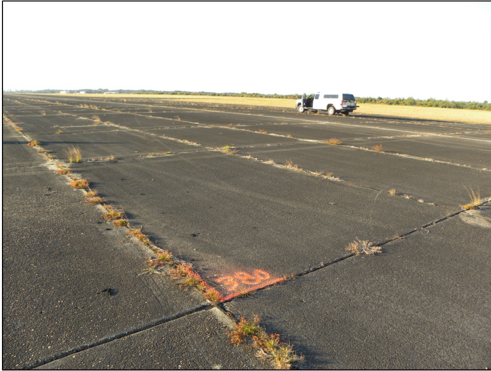
Runway 18-36, Section 6305, Sample Unit 380 – High severity (63) Longitudinal/Transverse/Diagonal Cracking, medium severity (65) Joint Seal Damage, low severity (66) Patching, low severity (74) Joint Spalling, low severity (75) Corner Spalling
