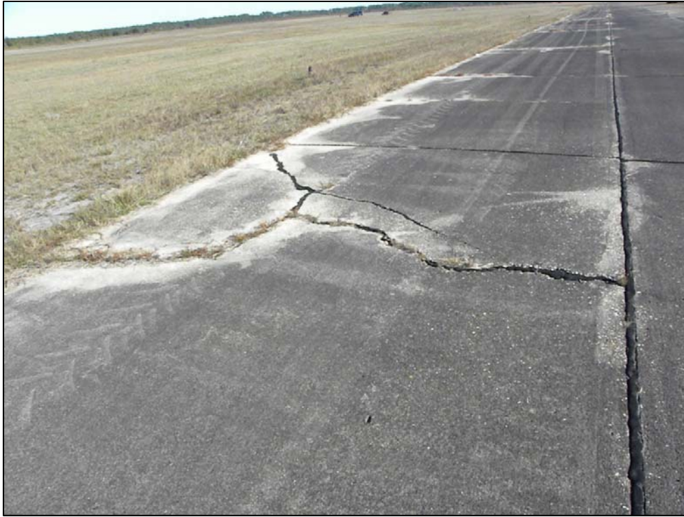
Apron, Section 4105, Sample Unit 166 – Medium and high severity (63) Longitudinal/Transverse/Diagonal Cracking, medium severity (65) Joint Seal Damage, low severity (66) Patching, high severity (72) Shattered Slab, (73) Shrinkage Cracking, medium severity (74) Joint Spalling, low severity (75) Corner Spalling
