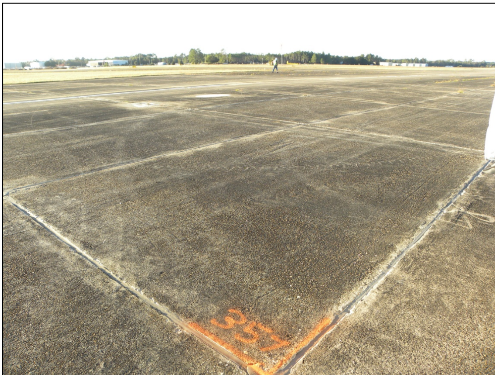
Runway 6-24, Section 6205, Sample Unit 357 – High severity (63) Longitudinal/Transverse/Diagonal Cracking, low severity (65) Joint Seal Damage, low severity (74) Joint Spalling, low severity (75) Corner Spalling
