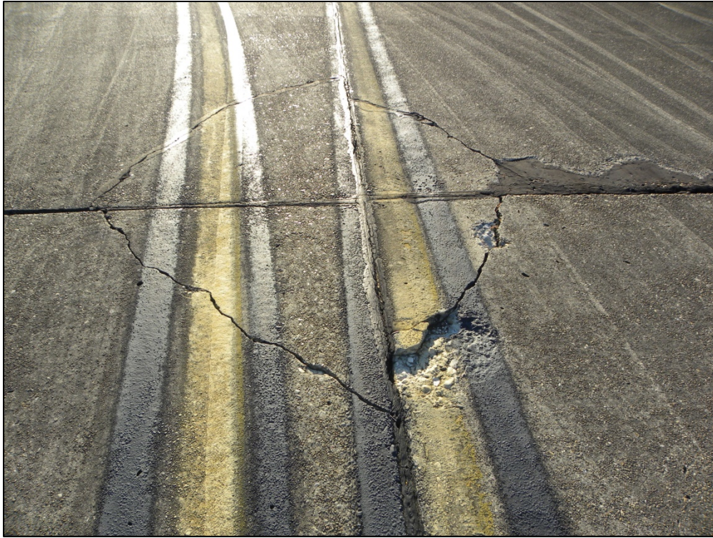
Taxiway A4, Section 230, Sample Unit 103 – High severity (62) Corner Break, high severity (63) Longitudinal/Transverse/Diagonal Cracking, low severity (65) Joint Seal Damage, low, medium and high severity (74) Joint Spalling, medium severity (75) Corner Spalling
