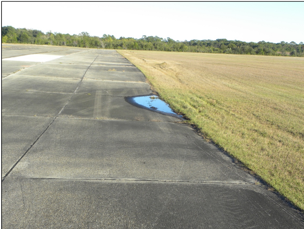
Taxiway A5, Section 210, Sample Unit 202 – Medium severity (65) Joint Seal Damage, high severity (71) Settlement or Faulting, medium severity (75) Corner Spalling
