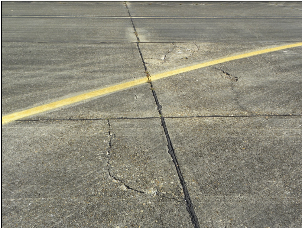
Apron, Section 4105, Sample Unit 214 – Medium and high severity (62) Corner Break, medium and high severity (63) Longitudinal/Transverse/Diagonal Cracking, medium severity (65) Joint Seal Damage, (68) Popouts, low severity (74) Joint Spalling
