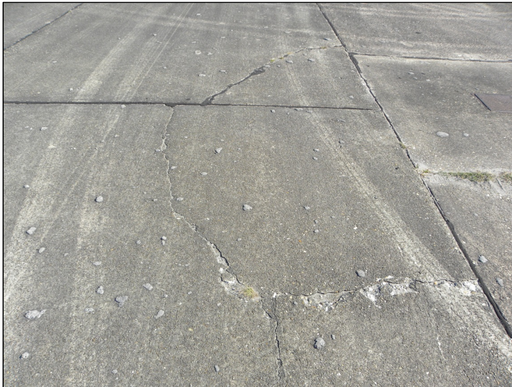
Apron, Section 4105, Sample Unit 360 – High severity (62) Corner Break, high severity (63) Longitudinal/Transverse/Diagonal Cracking, medium severity (65) Joint Seal Damage, low, medium and high severity (74) Joint Spalling, medium severity (75) Corner Spalling
