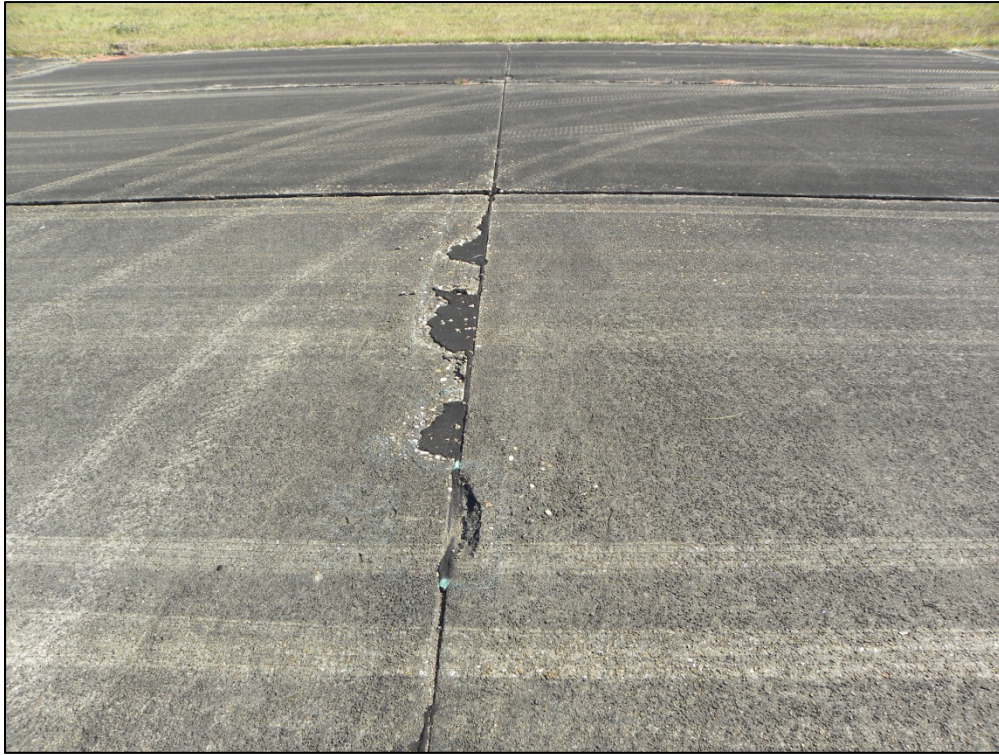
Taxiway Charlie, Section 105, Sample Unit 119 – Medium and high severity (65) Joint Seal Damage, low and high severity (74) Joint Spalling, medium severity (75) Corner Spalling
