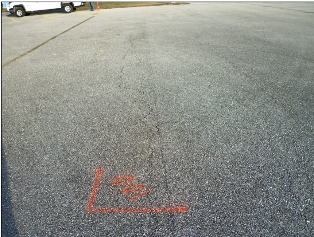
Apron, Section 4105, Sample Unit 100 – Low severity (52) Weathering and Raveling, low severity (48) Longitudinal and Transverse Cracking, and low severity (43) Block Cracking.
