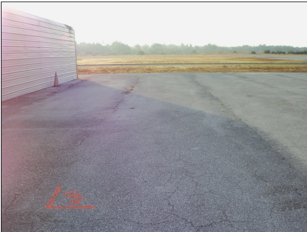
Apron, Section 4110, Sample Unit 401 – Low severity (52) Weathering and Raveling and low severity (43) Block Cracking.
