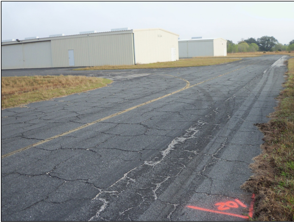
Taxiway Access to Hangars, Section 230, Sample Unit 102 – Medium severity (43) Block Cracking and medium severity (52) Weathering and Raveling.
