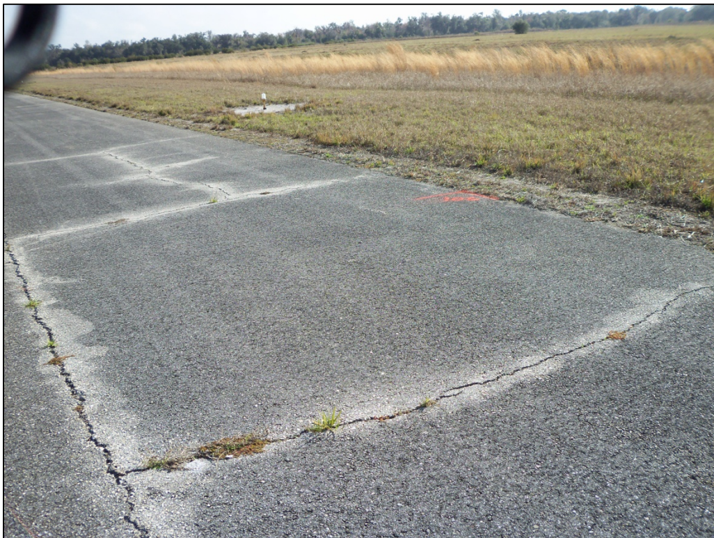
Runway 5-23, Section 6105, Sample Unit 106 – Medium severity (48) Longitudinal and Transverse Cracking, medium and high severity (52) Weathering and Raveling, and low severity (43) Block Cracking.
