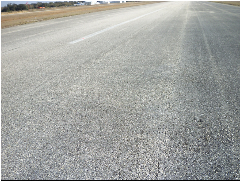
Runway 5-23, Section 6105, Sample Unit 106 – Low severity (48) Longitudinal and Transverse Cracking, medium and high severity (52) Weathering and Raveling, and low severity (43) Block Cracking.
