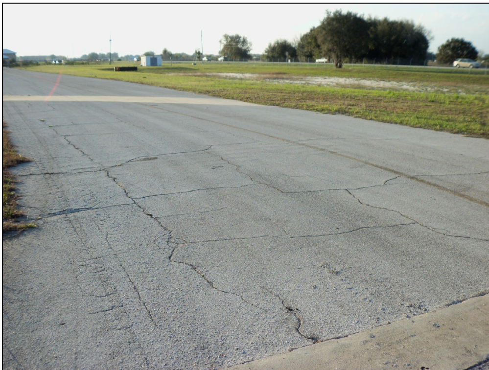
Taxiway Delta, Section 405, Sample Unit 101 – Medium severity (43) Block Cracking, low severity (50) Patch, low severity (52) Weathering and Raveling
