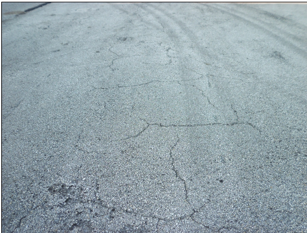
Apron, Section 4205, Sample Unit 300 – Low severity (43) Block Cracking, low severity (50) Patch, low and medium severity (52) Weathering and Raveling
