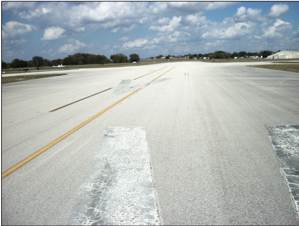
Runway 5-23, Section 6110, Sample Unit 158 – Low severity (48) Longitudinal and Transverse Cracking, low and medium severity (52) Weathering and Raveling
