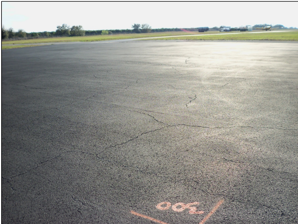
Apron, Section 4405, Sample Unit 300 – Low severity (43) Block Cracking, low severity (50) Patch, low severity (52) Weathering and Raveling
