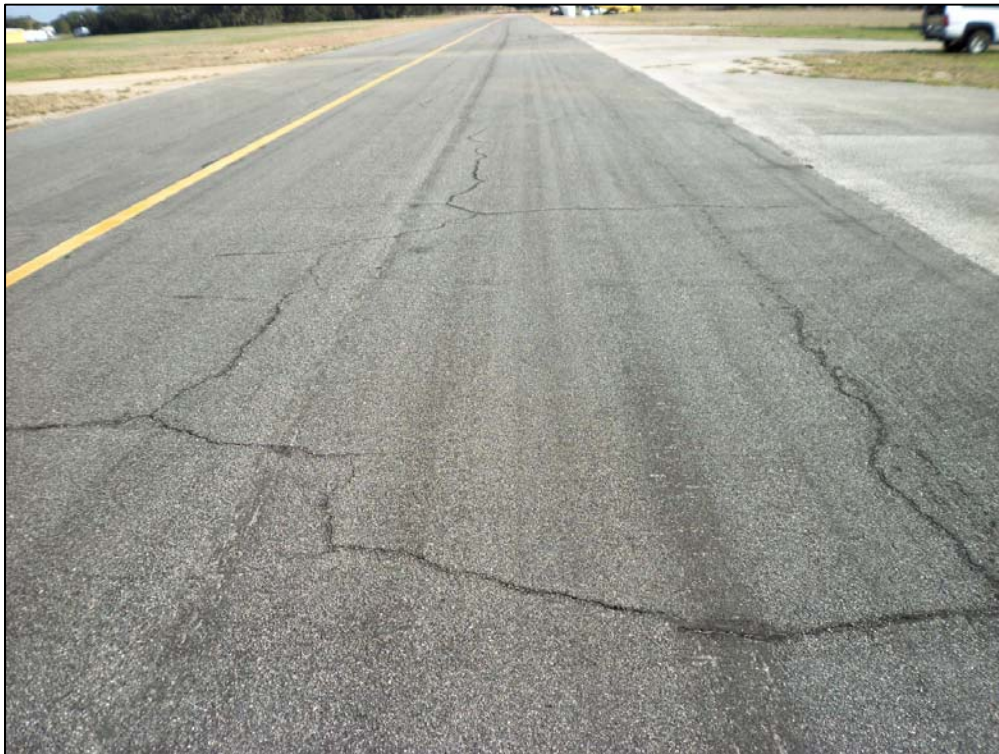
Taxiway Alpha, Section 115, Sample Unit 105 – Low severity (43) Block Cracking, low severity (48) Longitudinal and Transverse Cracking, low severity (52) Weathering and Raveling
