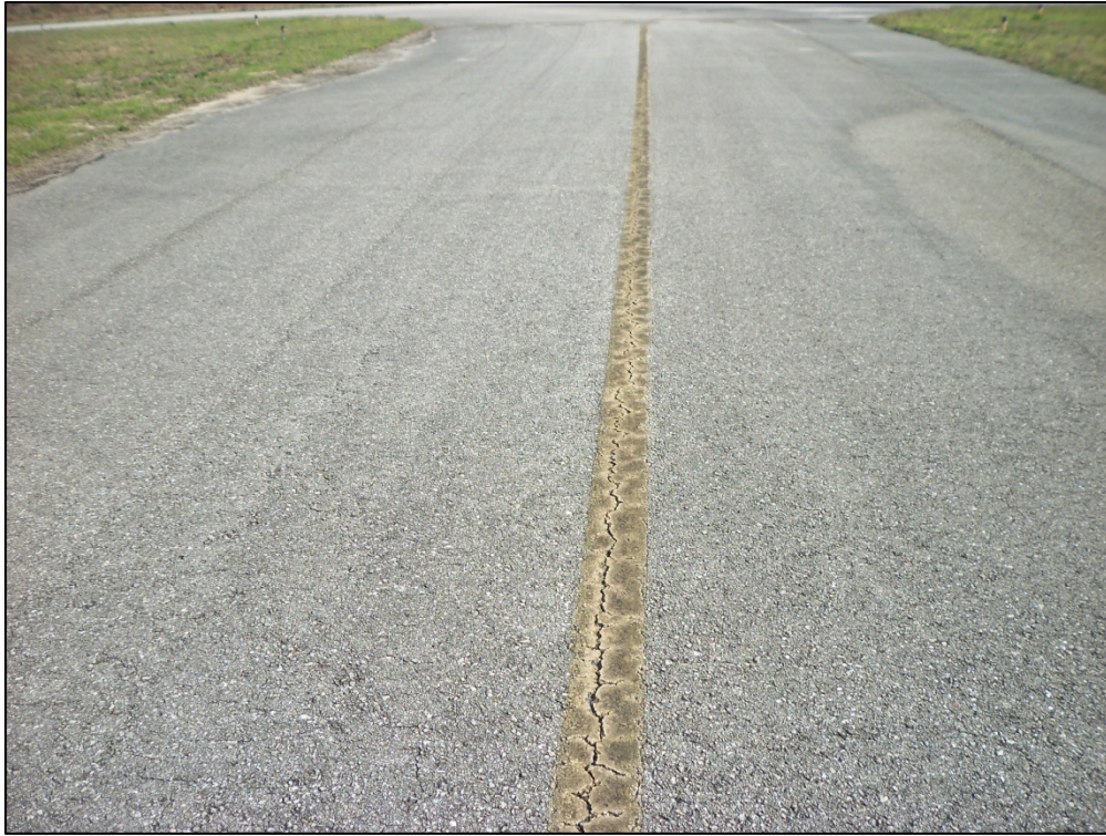
Taxiway Connector Delta, Section 415, Sample Unit 101 – Low severity (43) Block Cracking, low severity (48) Longitudinal and Transverse Cracking, low severity (52) Weathering and Raveling
