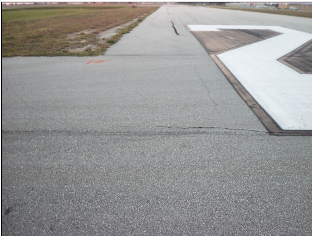
Runway 10-28, Section 6220, Sample Unit 100 – Low severity (48) Longitudinal and Transverse Cracking, low severity (52) Weathering and Raveling
