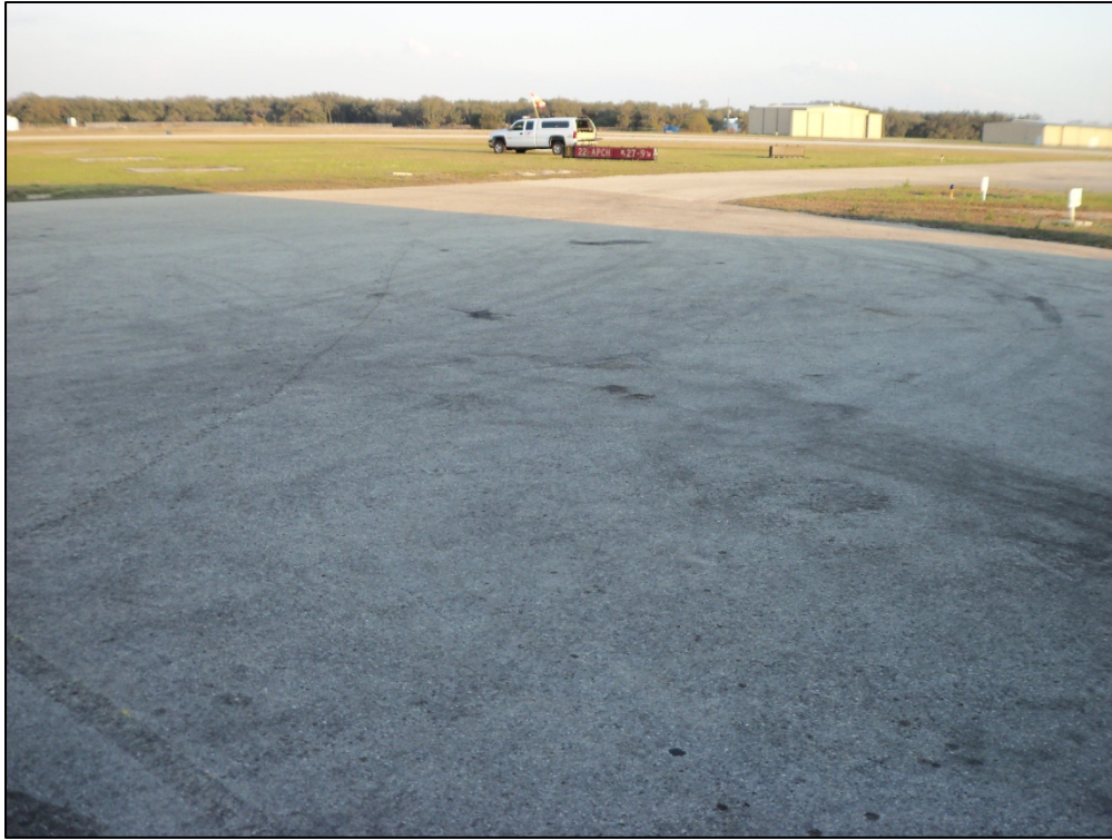
Apron, Section 4210, Sample Unit 102 – Low severity (43) Block Cracking, low severity (48) Longitudinal and Transverse Cracking, medium severity (52) Weathering and Raveling
