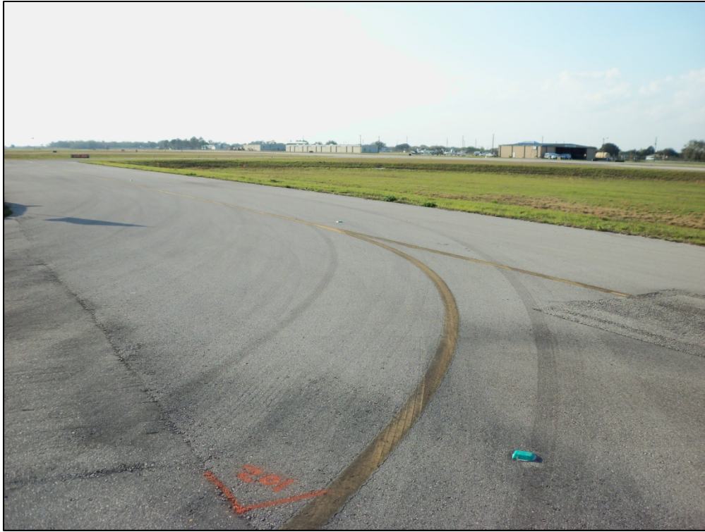
Taxiway 605, Section 605, Sample Unit 102 – Low severity (48) Longitudinal and Transverse Cracking, low severity (50) Patch, low severity (52) Weathering and Raveling
