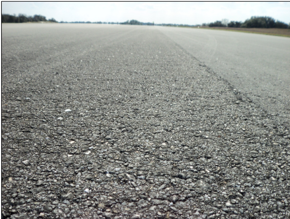
Runway 5-23, Section 6102, Sample Unit 99 – Low severity (48) Longitudinal and Transverse Cracking, low and medium severity (52) Weathering and Raveling
