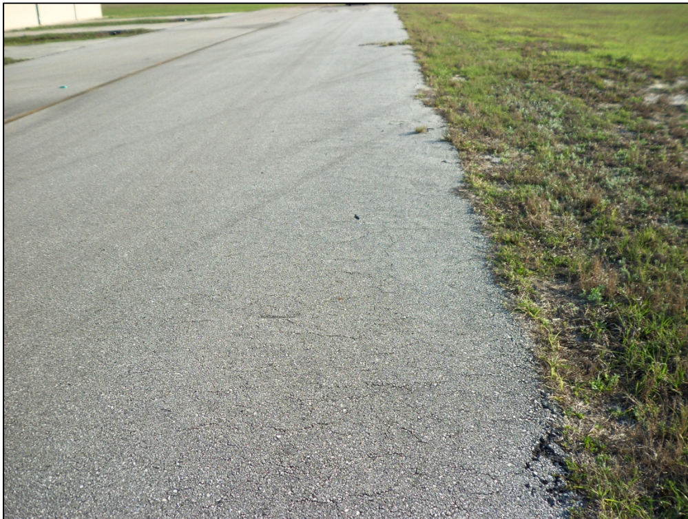
T-Hangar, Section 705, Sample Unit 402 – Low severity (43) Block Cracking, low severity (48) Longitudinal and Transverse Cracking, medium severity (50) Patch, low severity (52) Weathering and Raveling
