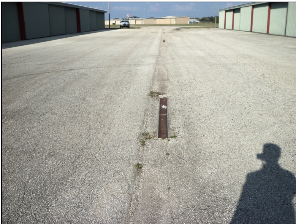
T-Hangar, Section 4305, Sample Unit 301 – Low severity Block Cracking, low severity (48) Longitudinal and Transverse Cracking, low severity (50) Patch, low and medium severity (52) Weathering and Raveling
