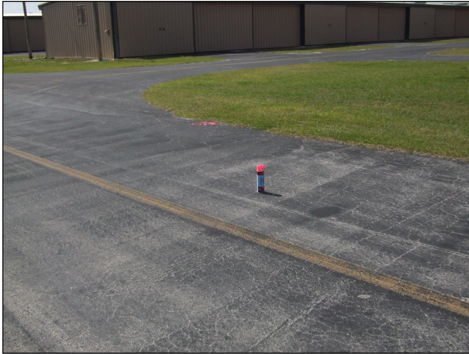
Runway 9R-27L, Section 6205, Sample Unit 329 – Low severity (41) Alligator Cracking, low and medium severity (43) Block Cracking, low severity (48) Longitudinal and Transverse Cracking, low and medium severity (52) Weathering and Raveling.
