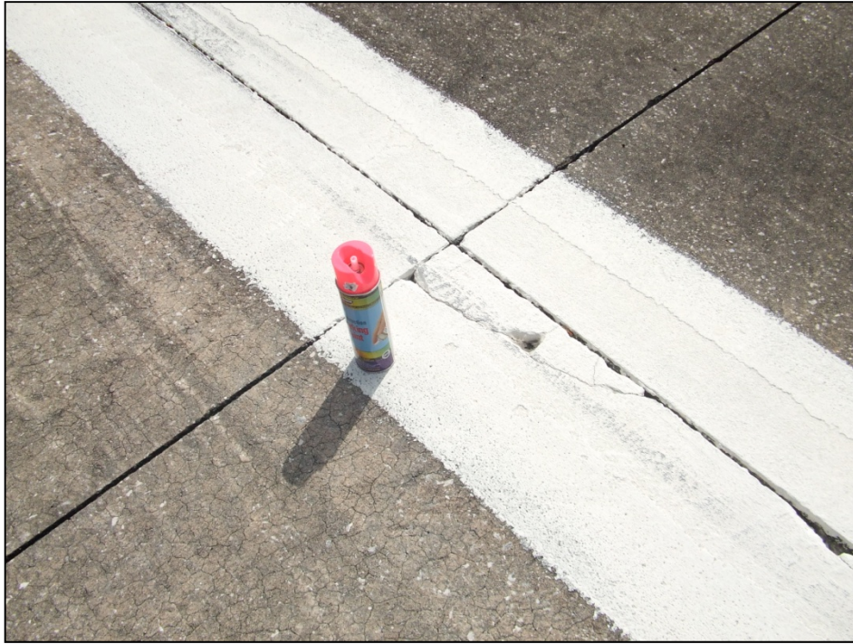
Runway 9R-27L, Section 6215, Sample Unit 382 – High severity (65) Joint Seal Damage, low severity (70) Scaling, low severity (73) Shrinkage Cracking, low and medium severity (74) Joint Spalling, low severity (75) Corner Spalling.
