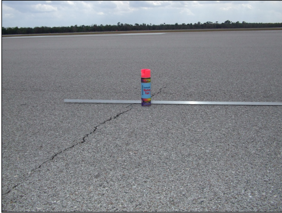
Runway 9L-27R, Section 6110, Sample Unit 104 – Low and medium severity (48) Longitudinal and Transverse Cracking, low severity (52) Weathering and Raveling, low severity (56) Swelling.
