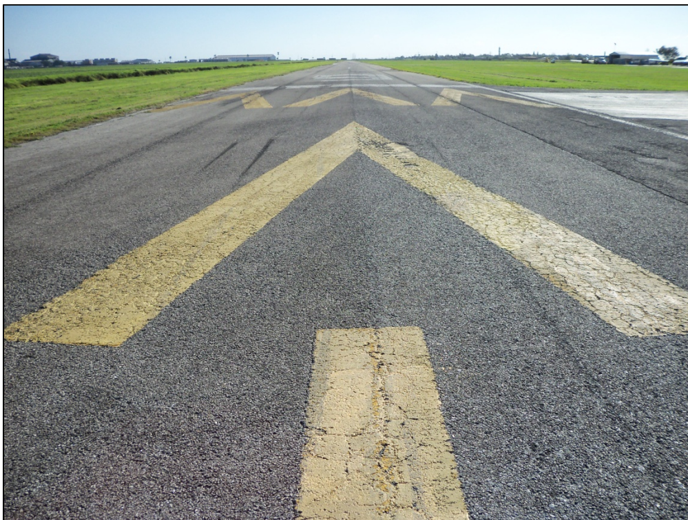
Runway 9-27, Section 6105, Sample Unit 101 – Low severity (43) Block Cracking, low, medium and high severity (52) Weathering and Raveling
