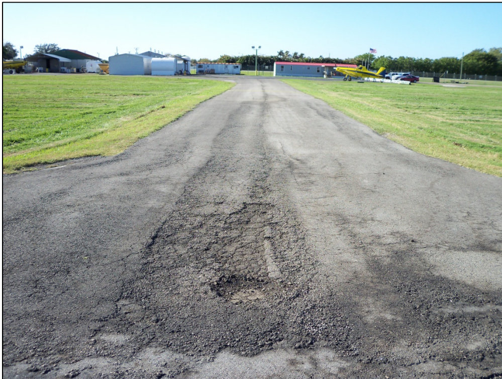
Taxiway, Section 115, Sample Unit 100 – Low severity (43) Block Cracking, low severity (48) Longitudinal and Transverse Cracking, low and high severity (52) Weathering and Raveling
