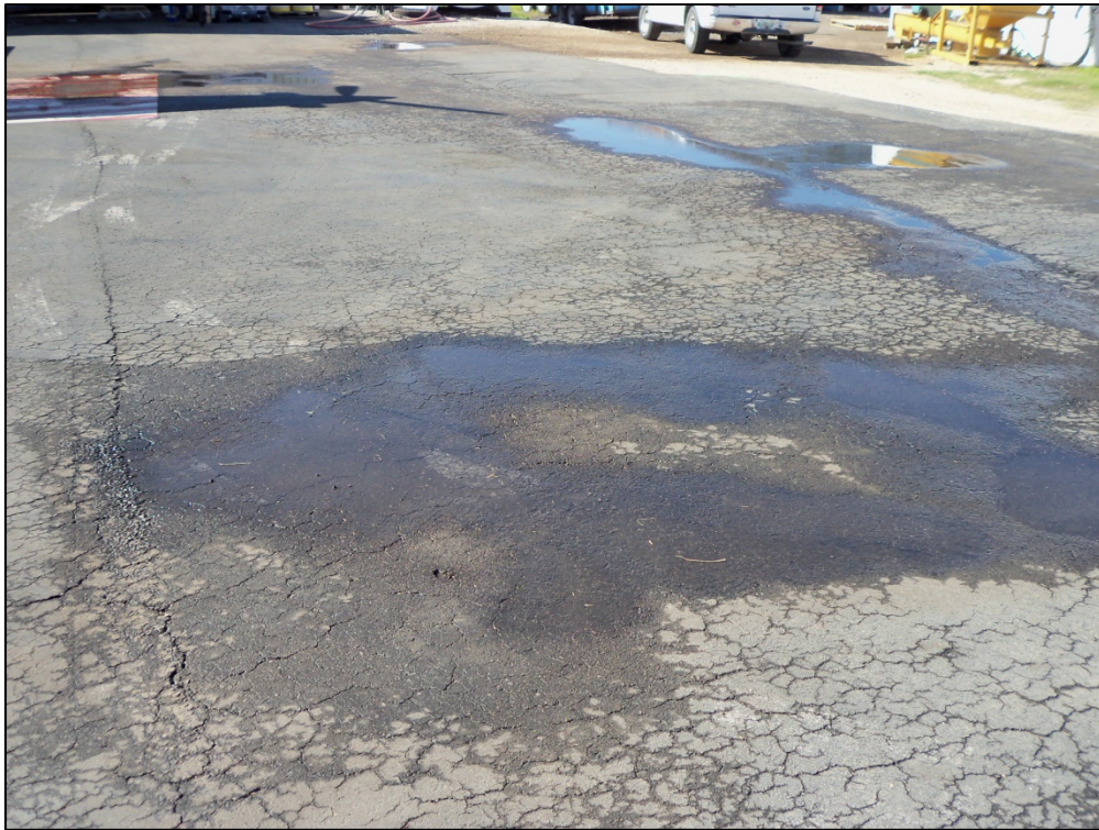
Apron, Section 4115, Sample Unit 100 – Low severity (43) Block Cracking, low severity (45) Depression, low severity (52) Weathering and Raveling
