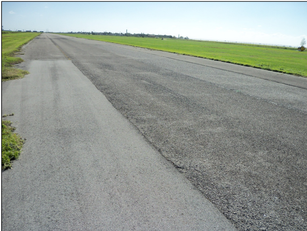
Runway 9-27, Section 6105, Sample Unit 109 – Low severity (48) Longitudinal and Transverse Cracking, low, medium and high severity (52) Weathering and Raveling
