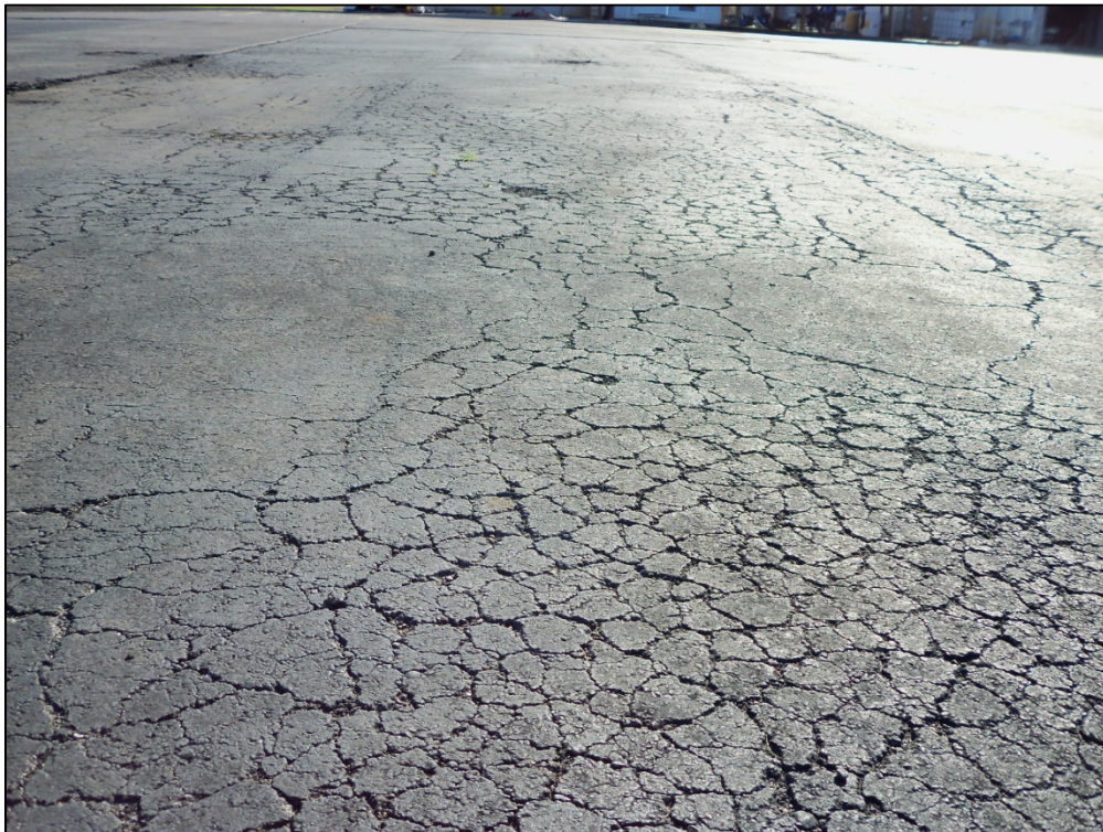
Apron, Section 4110, Sample Unit 100 – Medium severity (43) Block Cracking, low severity (48) Longitudinal and Transverse Cracking, (49) Oil Spillage, low and medium severity (52) Weathering and Raveling
