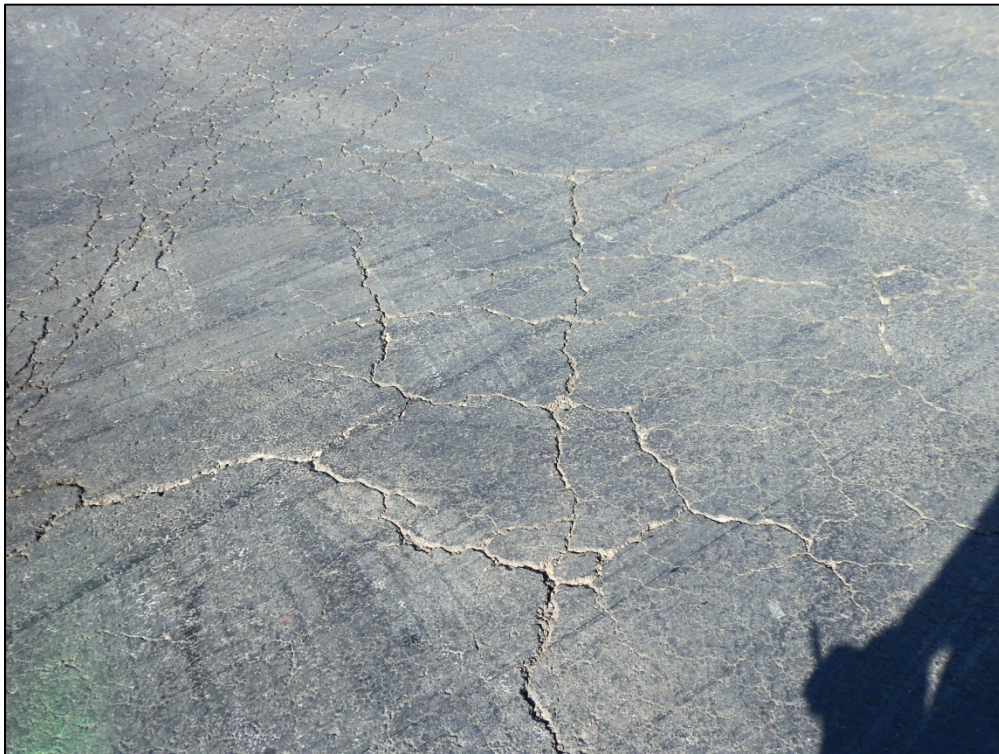
Apron, Section 4105, Sample Unit 200 – Low and medium severity (43) Block Cracking, low severity (48) Longitudinal and Transverse Cracking, (49) Oil Spillage, high severity (52) Weathering and Raveling
