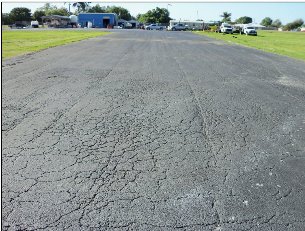
Taxiway, Section 105, Sample Unit 100 – Medium severity (43) Block Cracking, medium and high severity (52) Weathering and Raveling
