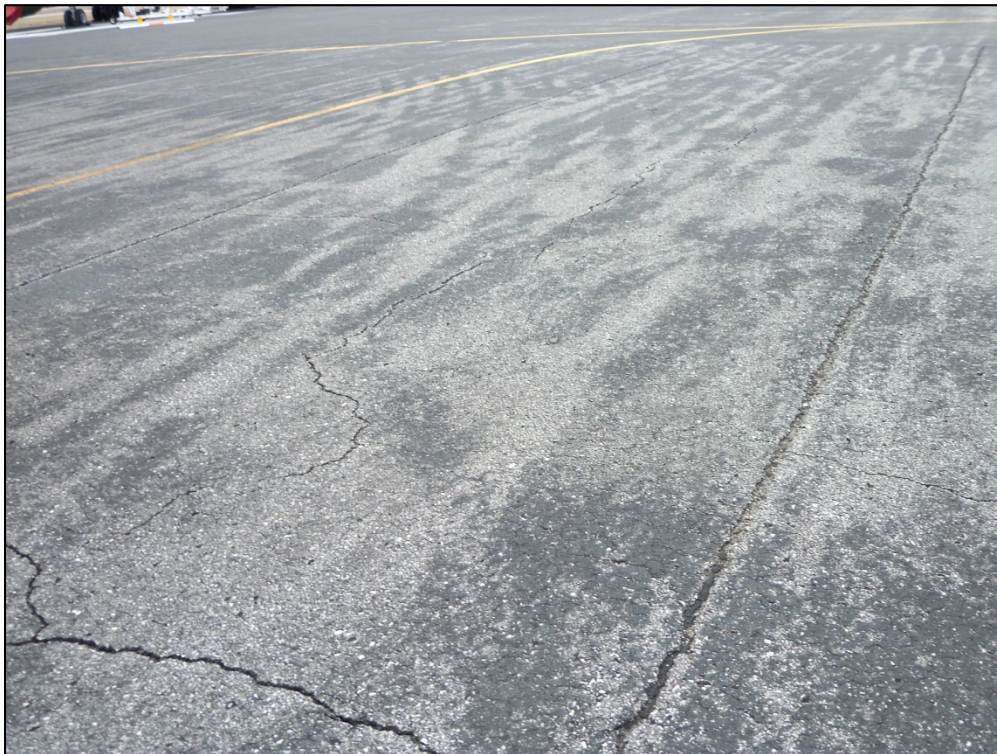
Apron, Section 4110, Sample Unit 501 – Medium severity (43) Block Cracking, low severity (48) Longitudinal and Transverse Cracking, medium severity (52) Weathering and Raveling
