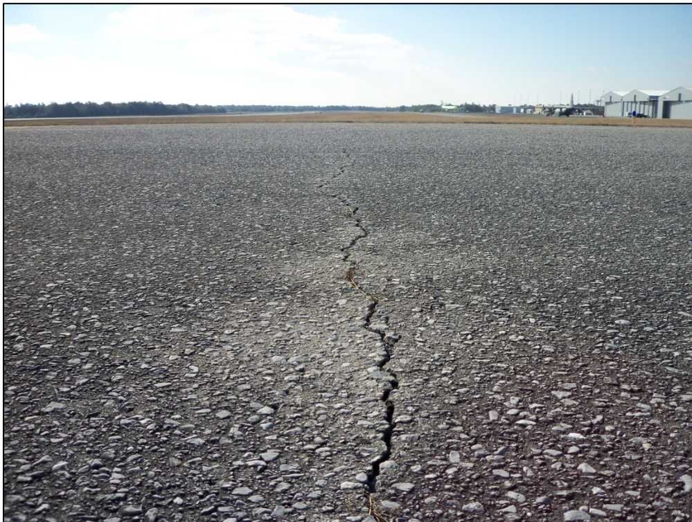
Taxiway A4, Section 110, Sample Unit 153 – Low severity (43) Block Cracking, low severity (48) Longitudinal and Transverse Cracking, low severity (52) Weathering and Raveling
