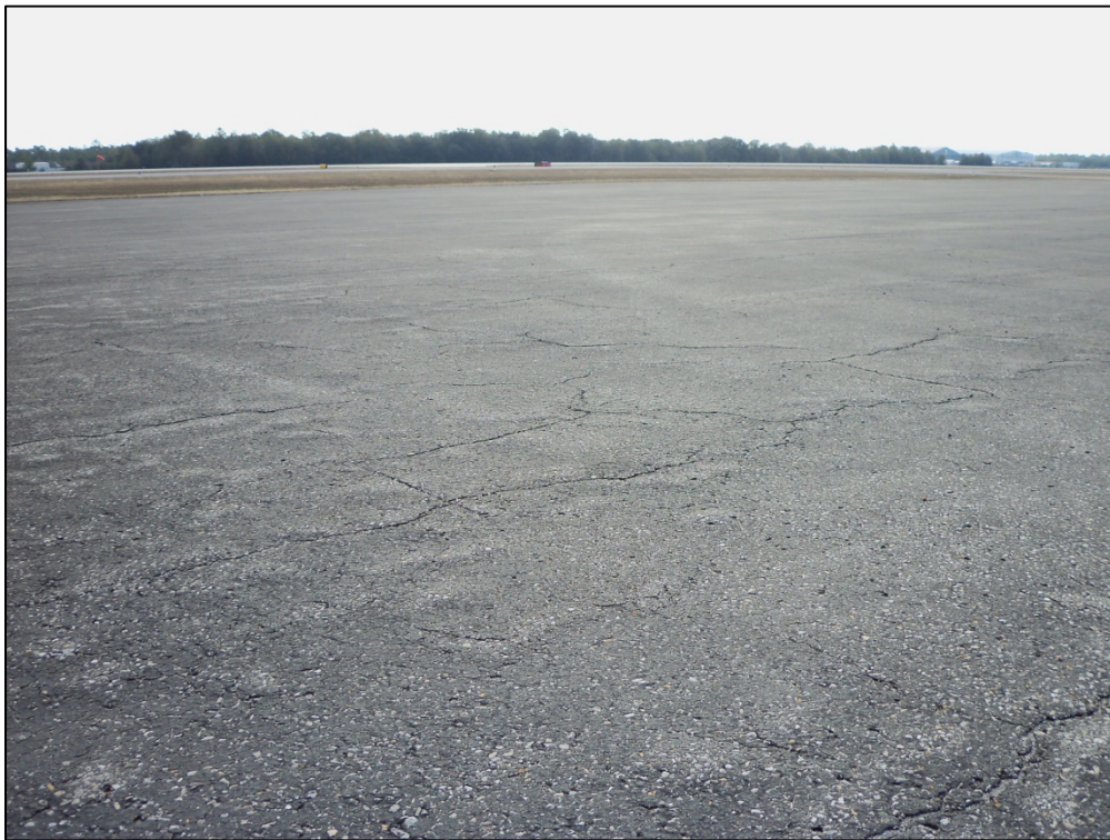
Apron, Section 4115, Sample Unit 312 – Medium severity (43) Block Cracking, medium severity (52) Weathering and Raveling
