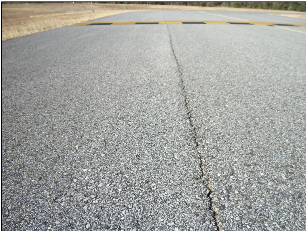
Taxiway, Section 105, Sample Unit 101 – Medium severity (43) Block Cracking, medium severity (52) Weathering and Raveling
