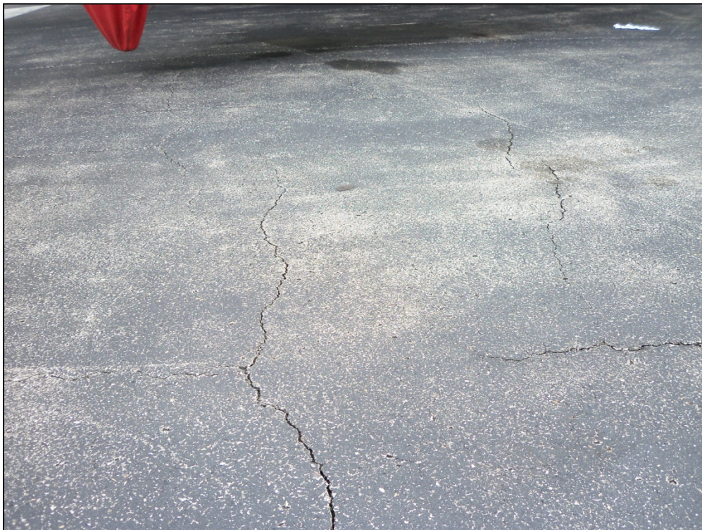
Apron, Section 4115, Sample Unit 200 – Medium severity (43) Block Cracking, high severity (48) Longitudinal and Transverse Cracking, (49) Oil Spillage, medium severity (52) Weathering and Raveling
