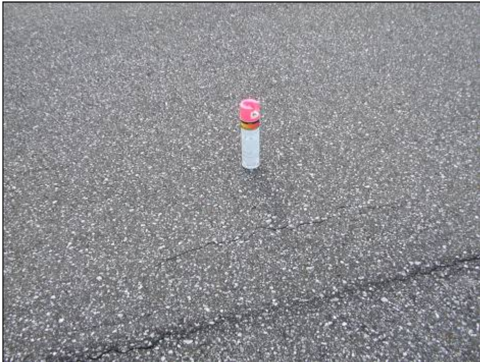
Runway 5-23 Section 6105, Sample Unit 139 – Low and medium severity (48) Longitudinal and Transverse Cracking, low severity (52) Weathering and Raveling, low severity (56) Swelling.
