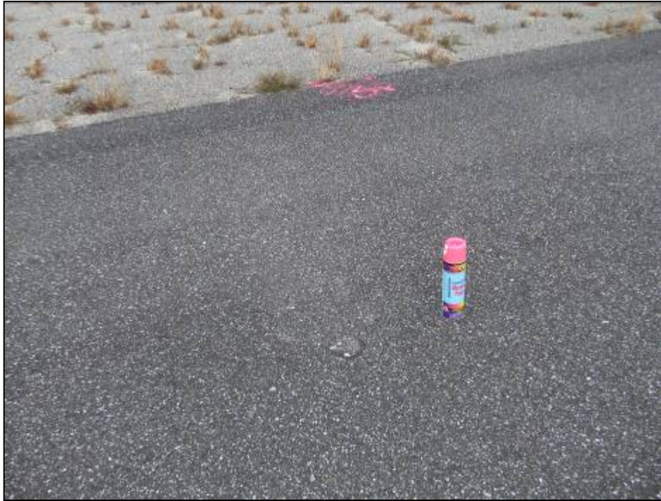
Runway 5-23 Section 6105, Sample Unit 115 – Low and medium severity (48) Longitudinal and Transverse Cracking, low severity (50) Patching, low severity (52) Weathering and Raveling.
