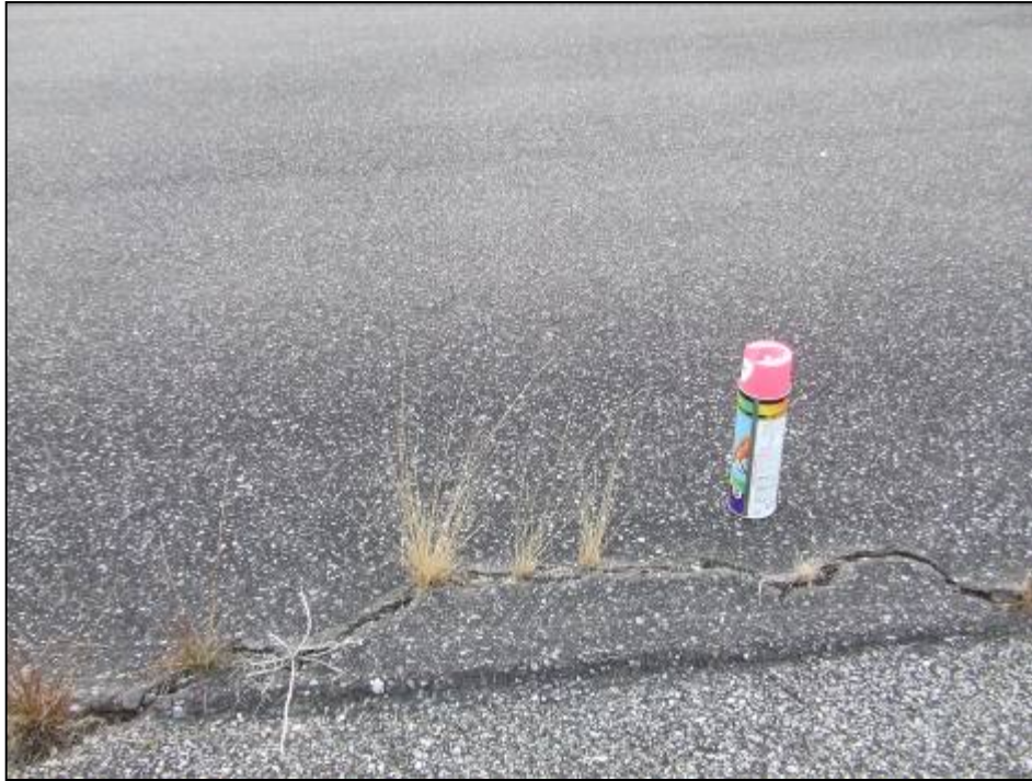
Runway 5-23 Section 6105, Sample Unit 175 – Low and medium severity (48) Longitudinal and Transverse Cracking, low severity (52) Weathering and Raveling.
