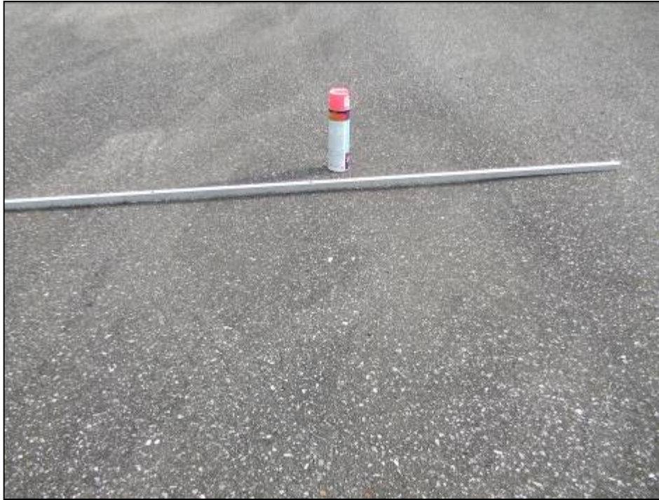
Apron Section 4105, Sample Unit 100 – Low severity (45) Depression, low severity (48) Longitudinal and Transverse Cracking, low severity (52) Weathering and Raveling, low severity (56) Swelling.
