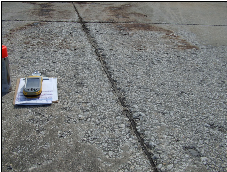
North Apron, Section 4110, Sample Unit 205 – Medium severity (70) Scaling
