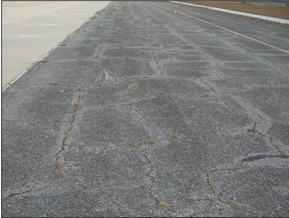
Taxiway Charlie, Section 315, Sample Unit 103 – High severity (43) Block Cracking and medium severity (52) Weathering and Raveling.
