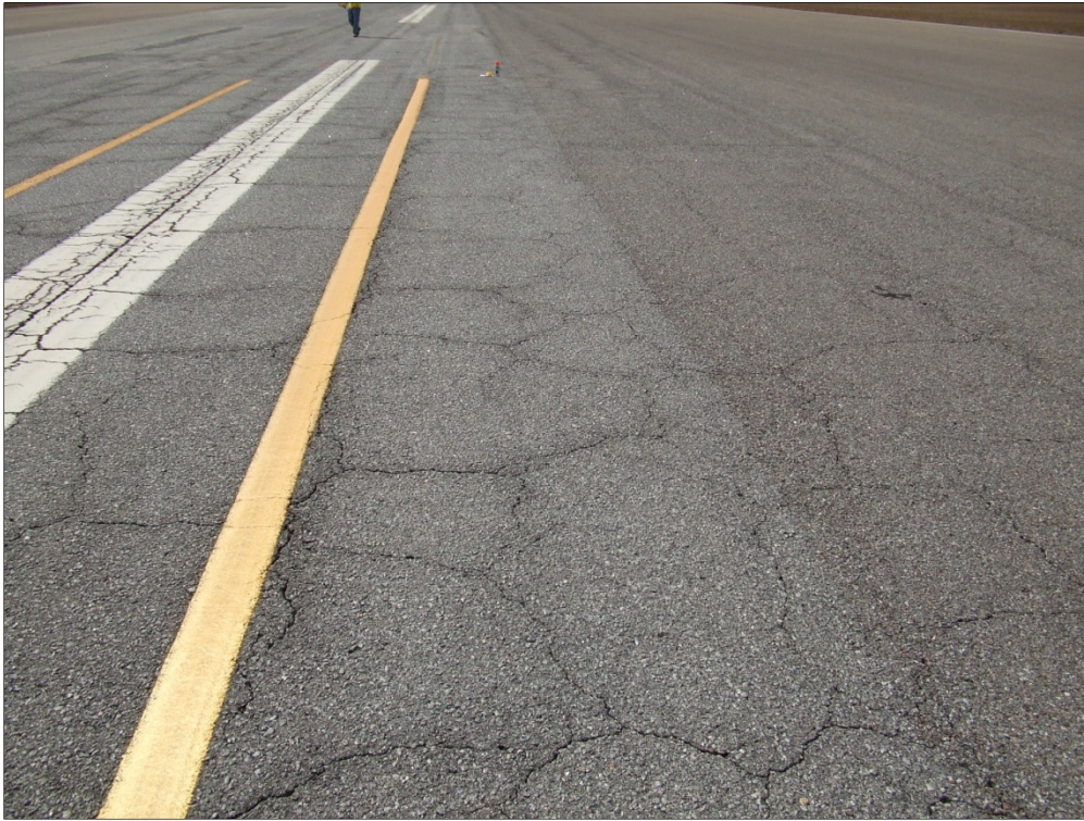
Runway 18R-36L, Section 6115, Sample Unit 348 – Low and moderate severity (43) Block Cracking and low severity (52) Weathering and Raveling.
