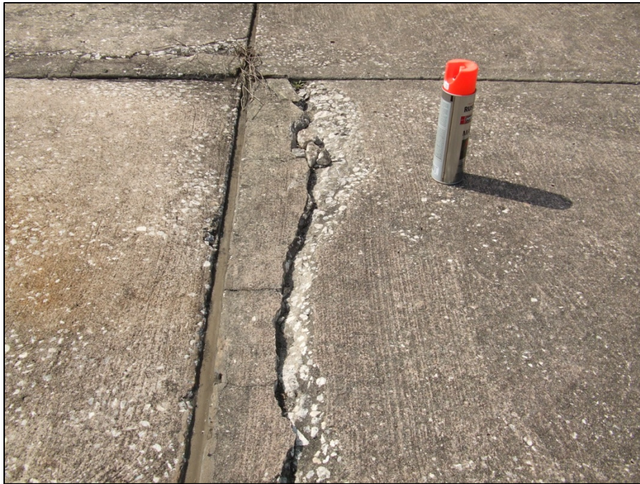
West Parking Apron, Section 4210, Sample Unit 206 – High severity (74) Joint Spalling, low severity (70) Scaling, and low severity (65) Joint Seal Damage.
