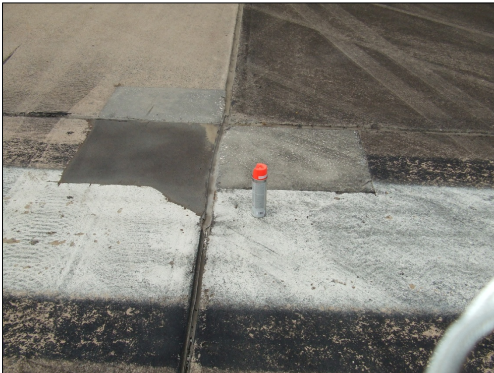
Runway 18R-36L, Section 6140, Sample Unit 482 – Low severity (67) Large Patch and low severity (70) Scaling.
