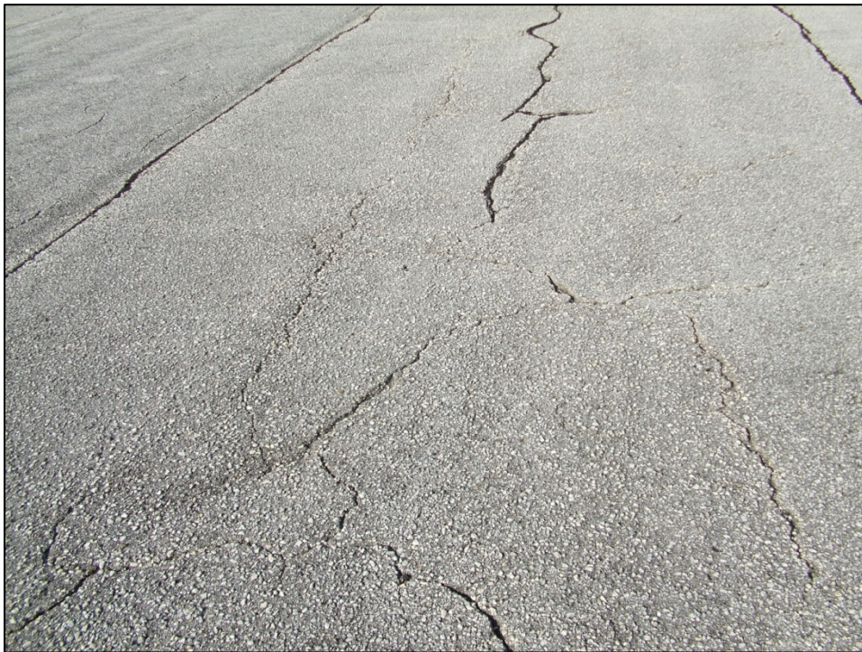
Runway 9L-27R, Section 6415, Sample Unit 527 – Low and medium severity (48) Longitudinal / Transverse Cracking and low severity (52) Weathering and Raveling
