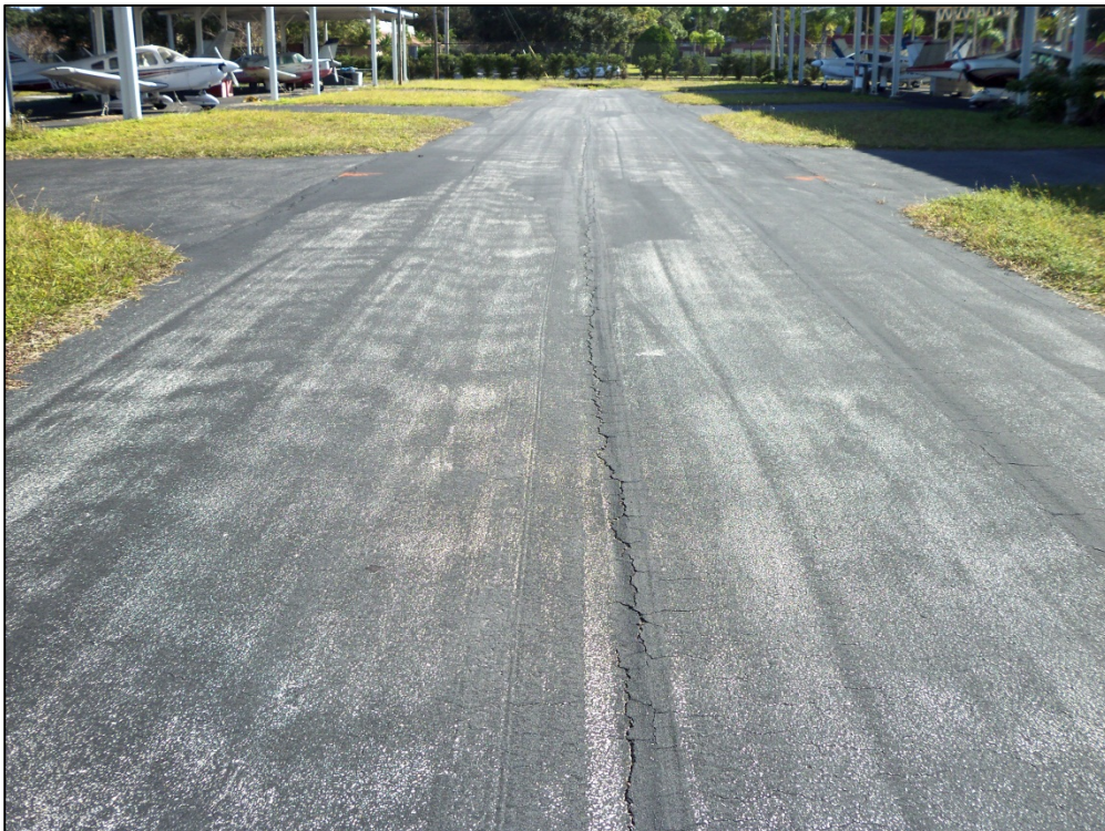
Apron T-Hangar, Section 4105, Sample Unit 201 – Low severity (48) Longitudinal and Transverse Cracking, (52) Raveling and Weathering
