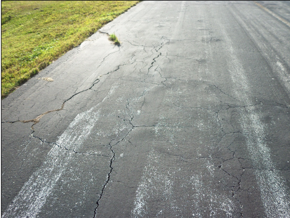
Taxiway Alpha, Section 105, Sample Unit 114 – Low severity (43) Block Cracking, High severity (48) Longitudinal and Transverse Cracking, Low severity (52) Raveling and Weathering
