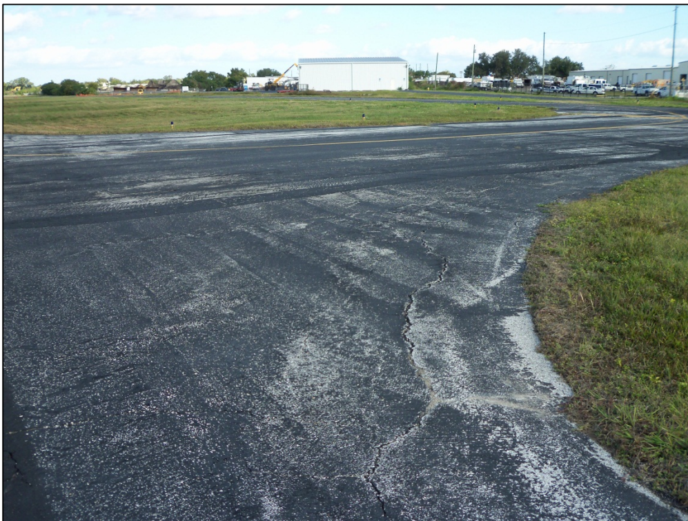
Taxiway Connector A-2, Section 120, Sample Unit 200 – Medium severity (48) Longitudinal and Transverse Cracking, (52) Raveling and Weathering
