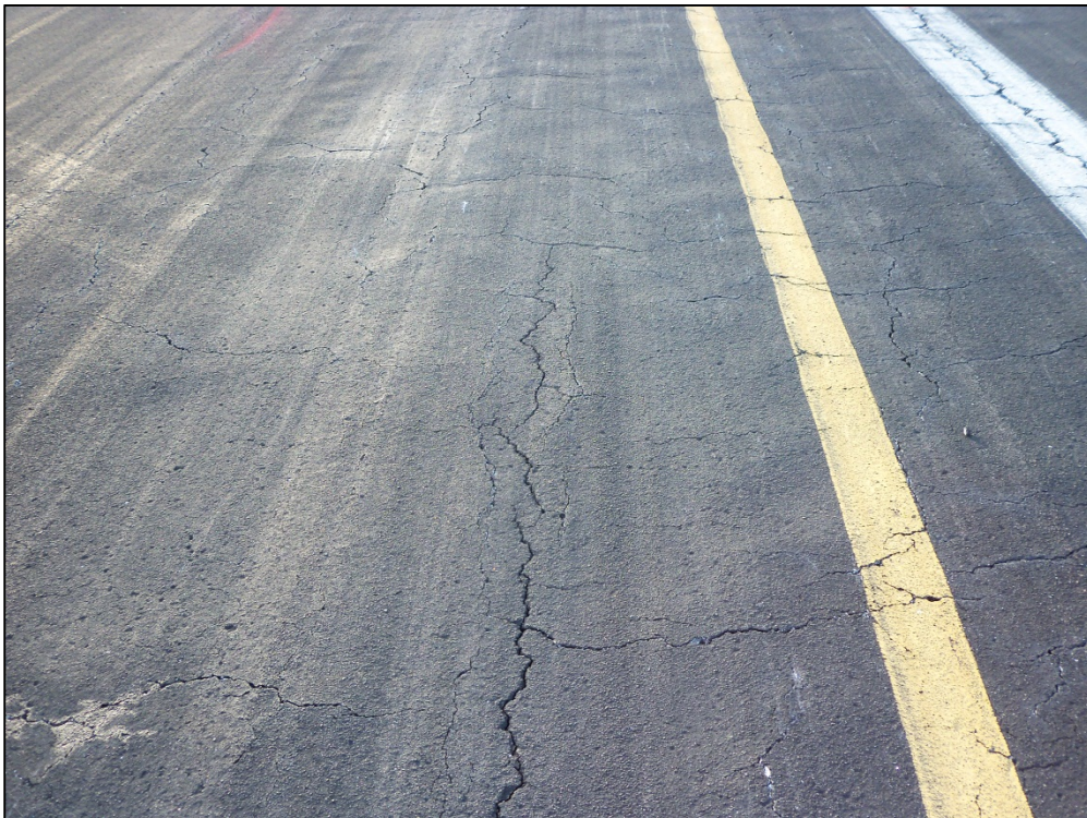
Runway 16-34, Section 6110, Sample Unit 155 – Low severity (43) Block Cracking, (48) Longitudinal and Transverse Cracking
