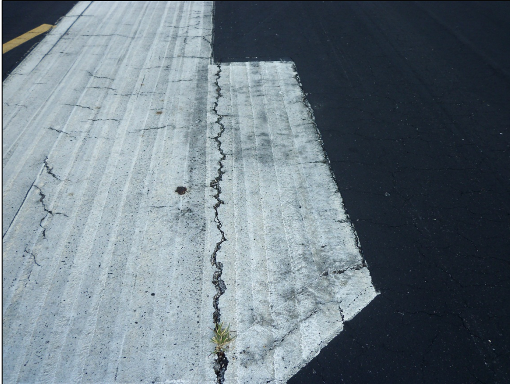
Runway 16-34, Section 6110, Sample Unit 158 – Low severity (48) Longitudinal and Transverse Cracking, (52) Weathering and Raveling
