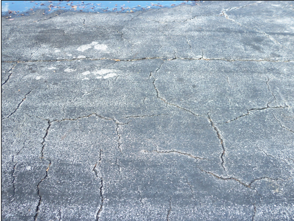
Apron Center, Section 4405, Sample Unit 200 – Medium severity (43) Block Cracking, Low severity (52) Raveling and Weathering
