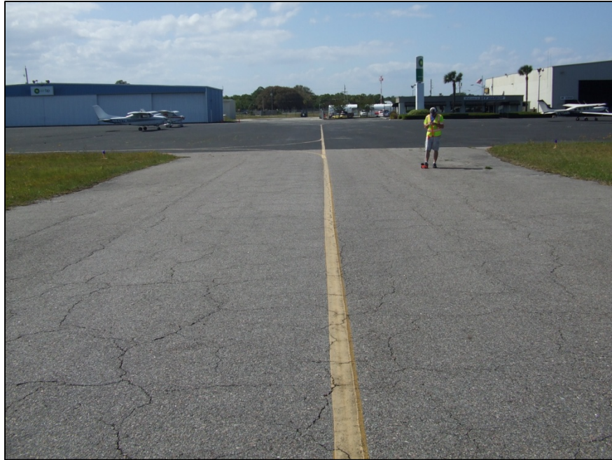
Taxiway B-4, Section 405, Sample Unit 407 – Low severity (43) Block Cracking, low severity (52) Weathering and Raveling.
