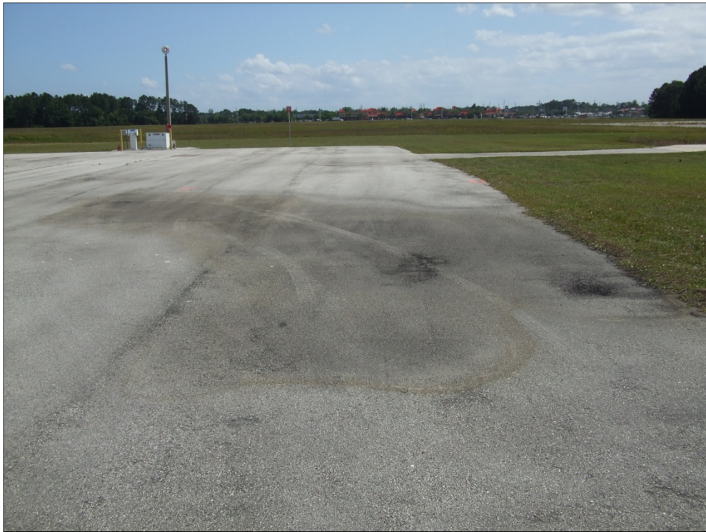
Southwest Apron, Section 4430, Sample Unit 200 – Low severity (45) Depression and low to medium severity (52) Weathering and Raveling.
