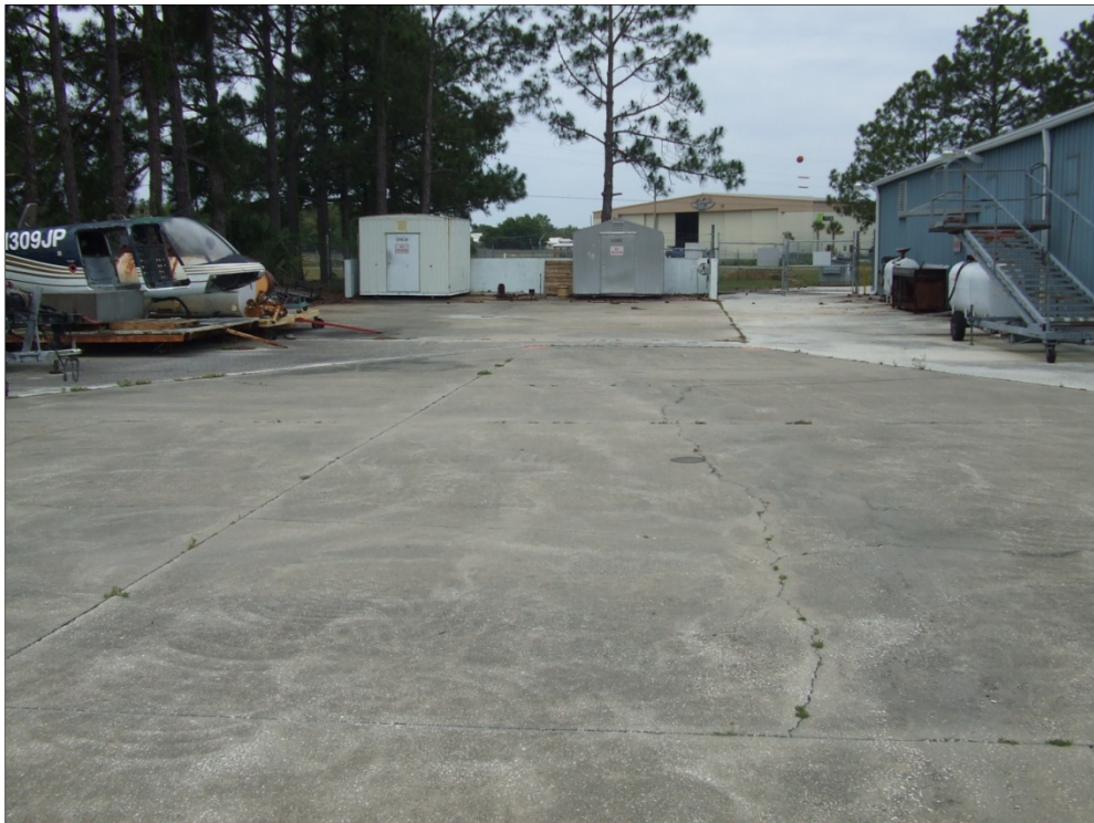
Southwest Apron, Section 4405, Sample Unit 101 – Low severity (63) Linear Cracking, high severity (65) Joint Seal Damage.
