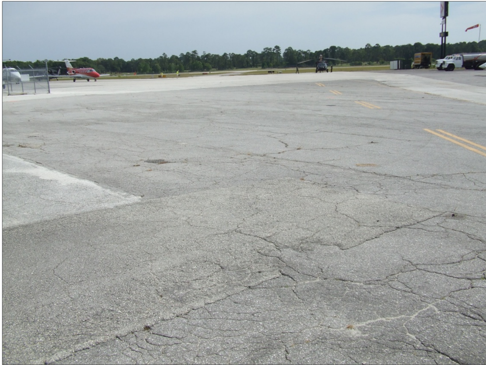
Northwest Apron, Section 4310, Sample Unit 204 – Low to high severity (43) Block Cracking, low severity (50) Patching, and low to medium severity (52) Weathering and Raveling.
