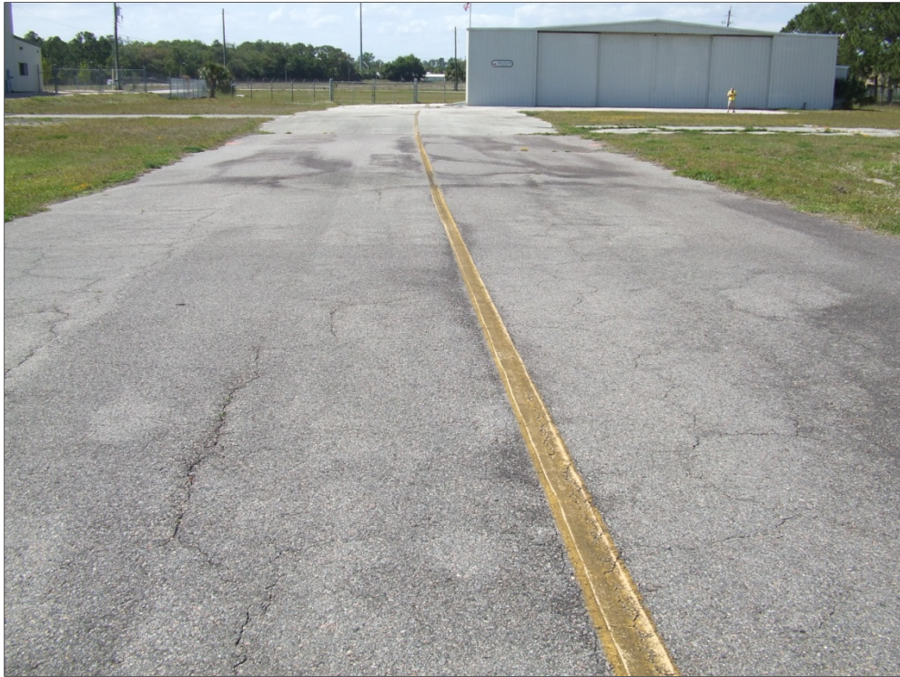
Southwest Apron, Section 4411, Sample Unit 99 – Low severity (43) Block Cracking and low severity (52) Weathering and Raveling.
