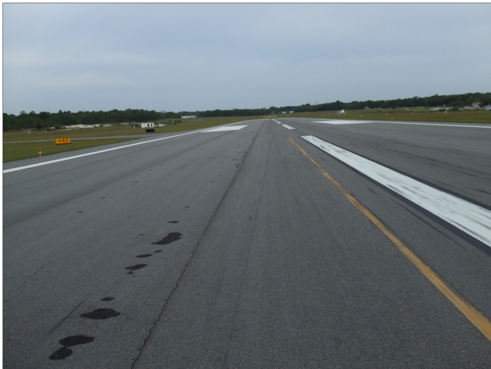
Runway 14-32, Section 6210, Sample Unit 151 – (42) Bleeding and low severity (48) Longitudinal and Transverse Cracking.
