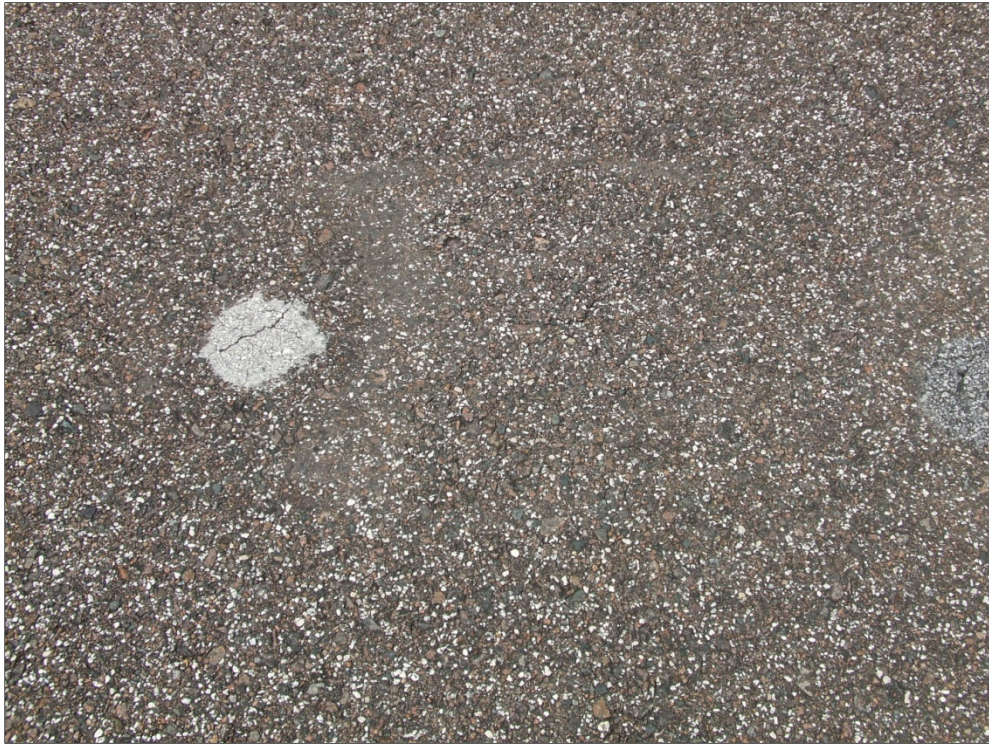
Taxiway Golf, Section 165, Sample Unit 314 – Low severity (50) Patching and low severity (52) Weathering and Raveling.
