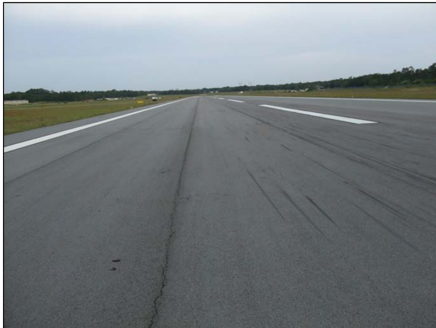
Runway 14-32, Section 6210, Sample Unit 125 – Low severity (48) Longitudinal / Transverse Cracking.
