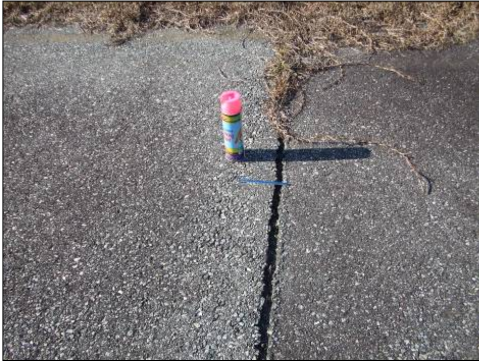
Taxiway Charlie, Section 220, Sample Unit 102 – Low, medium, and high severity (48) Longitudinal and Transverse Cracking, and low severity (52) Weathering and Raveling.
