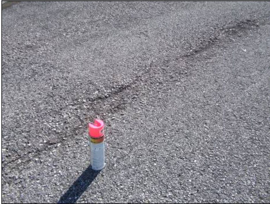
Runway 4-22, Section 6205, Sample Unit 100 – Low and medium severity (48) Longitudinal and Transverse Cracking; low, medium, and high severity (52) Weathering and Raveling; low severity (56) Swell.
