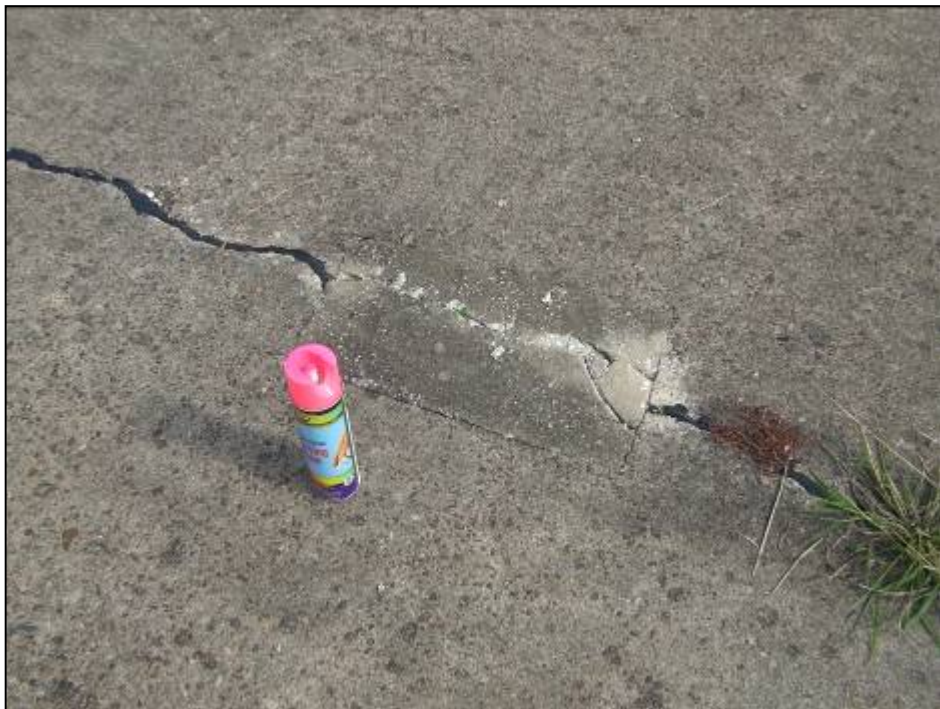
Runway 13-31, Section 6110, Sample Unit 194 – Low and medium severity (63) Linear Cracking; medium severity (65) Joint Seal Damage; medium severity (66) Small Patch; low severity (70) Scaling; low severity (73) Shrinkage Cracking; low severity (74) Joint Spall; low severity (75) Corner Spall.
