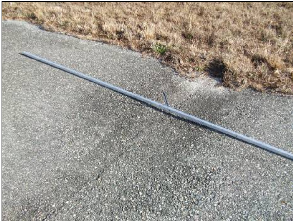
Runway 4-22, Section 6210, Sample Unit 205 – Low severity (45) Depression, low severity (48) Longitudinal and Transverse Cracking, low severity (50) Patching, and low severity (52) Weathering and Raveling.
