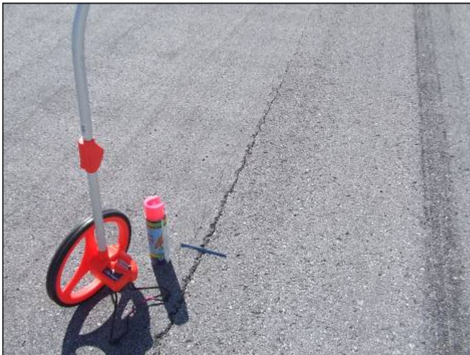
Runway 9-27, Section 6110, Sample Unit 161 –Low severity (48) Longitudinal and Transverse Cracking, low and medium severity (52) Weathering and Raveling.
