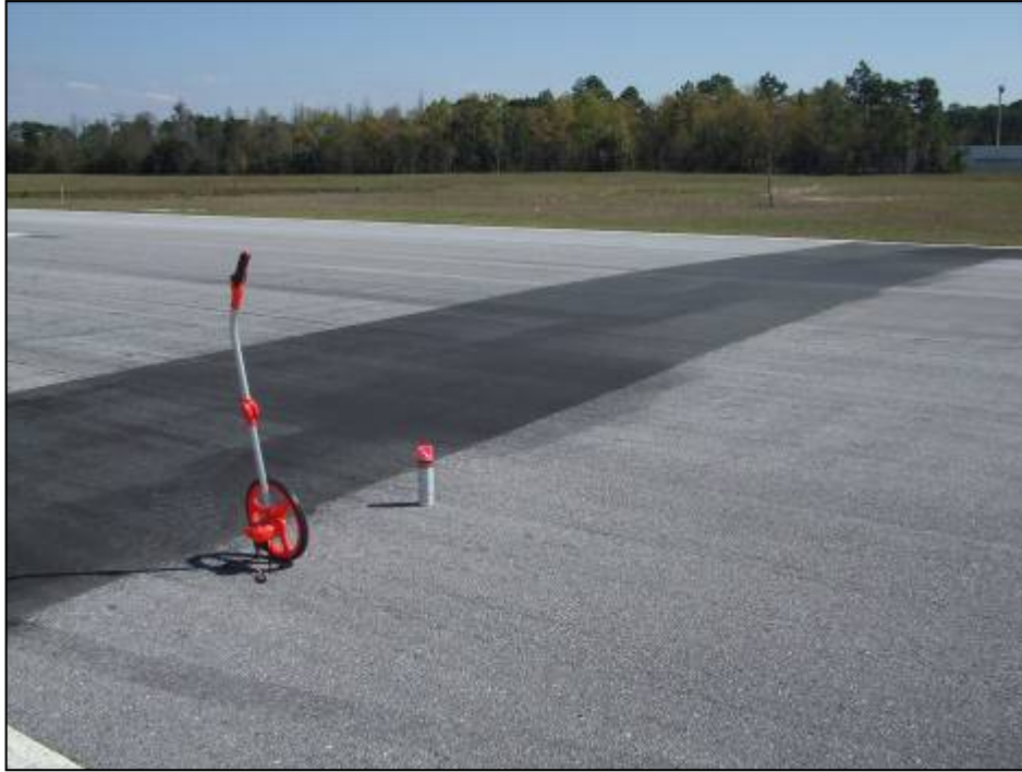
Runway 9-27, Section 6105, Sample Unit 146 – Low severity (48) Longitudinal and Transverse Cracking, low severity (50) Patching, low and medium severity (52) Weathering and Raveling.
