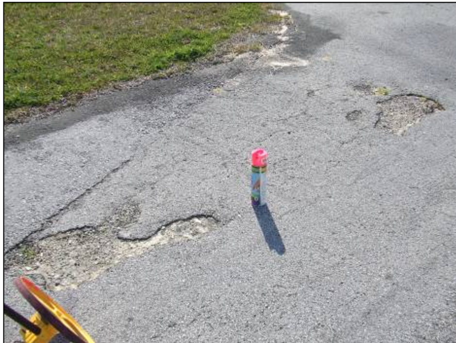
Connector Taxiway to AP, Section 205, Sample Unit 103 – Low severity (45) Depression, low severity (48) Longitudinal and Transverse Cracking, medium severity (50) Patching, medium and high severity (52) Weathering and Raveling.
