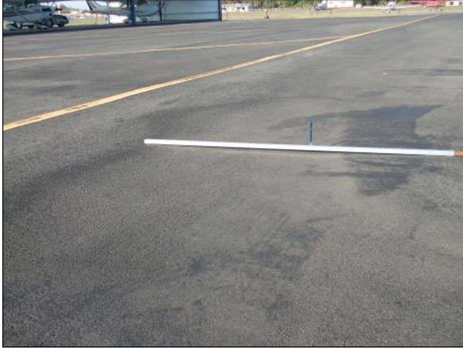
Main Apron, Section 4110, Sample Unit 198 – Low severity (45) Depression; low severity (49) Oil Spillage; low severity (50) Patching; low, medium and high severity (52) Weathering and Raveling.
