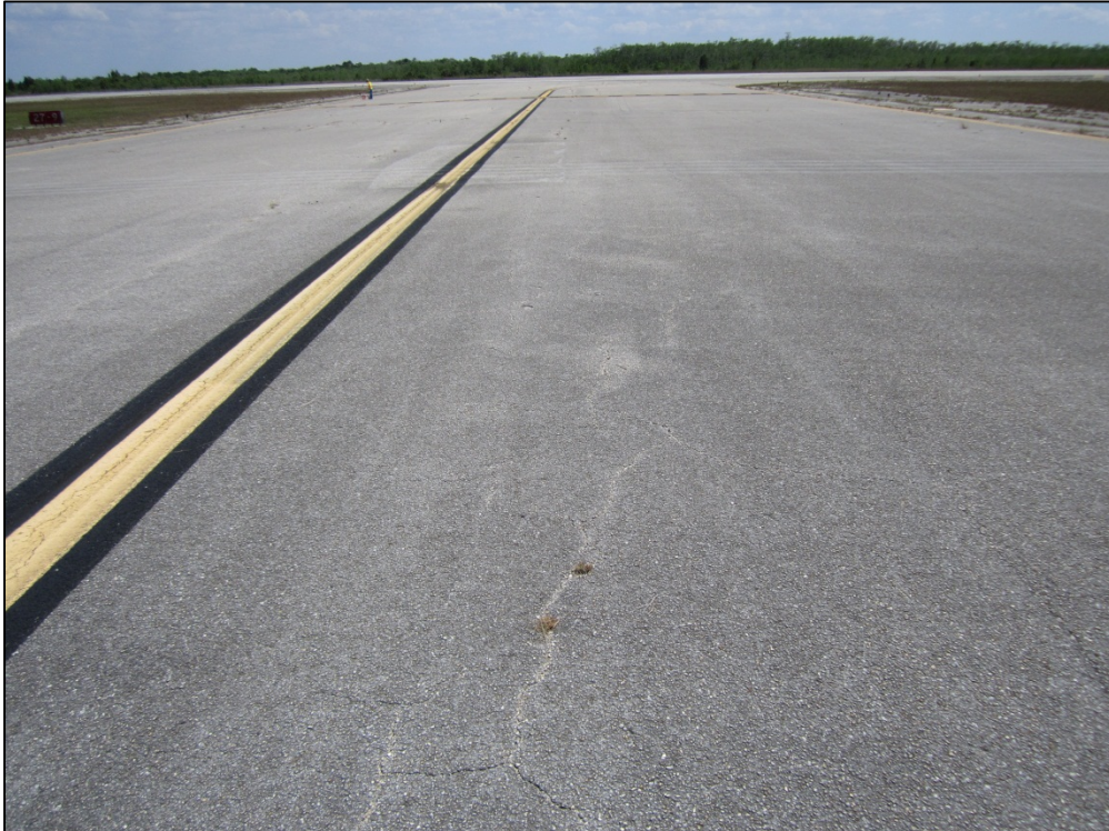
Taxiway A-6, Section 170, Sample Unit 608 – Low severity (52) Weathering and Raveling; low severity (48) Longitudinal and Transverse Cracking
