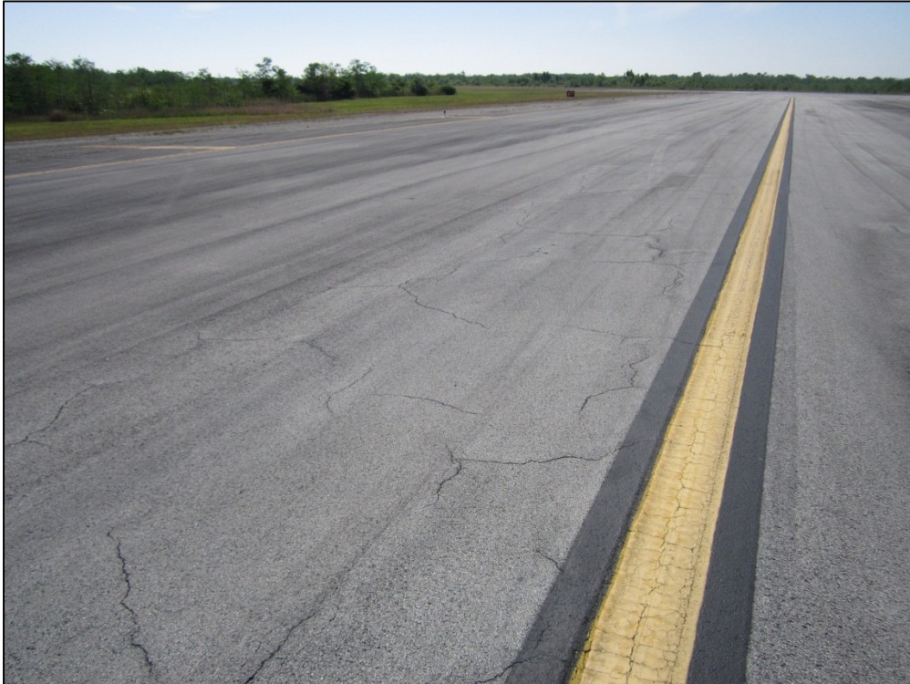
Taxiway Alpha, Section 180, Sample Unit 111 – Low severity (52) Weathering and Raveling; low severity (48) Longitudinal and Transverse Cracking; low severity (56) Swelling
