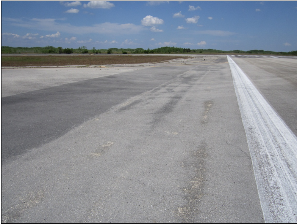
Taxiway A-6, Section 176, Sample Unit 600 – Low severity (52) Weathering and Raveling; low severity (48) Longitudinal and Transverse Cracking; low severity (56) Swelling
