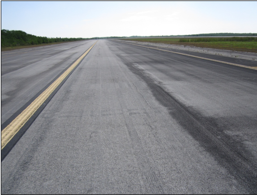
Taxiway Alpha, Section 105, Sample Unit 237 – Low severity (52) Weathering and Raveling; low severity (48) Longitudinal and Transverse Cracking; low severity (56) Swelling; low severity (53) Rutting
