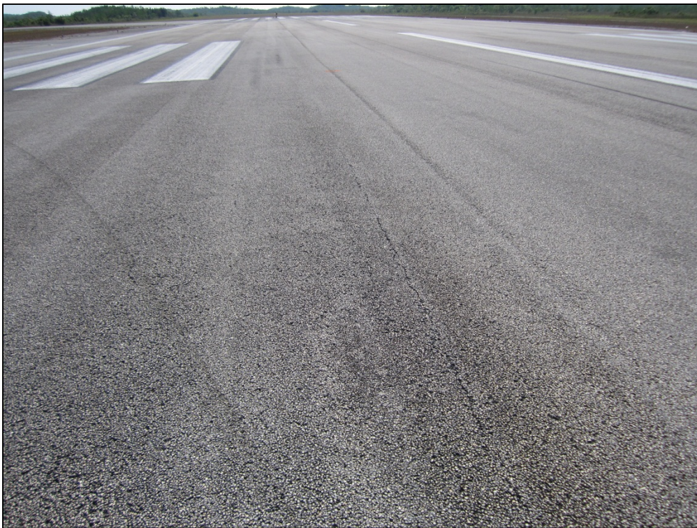
Runway 9-27, Section 6110, Sample Unit 198 – Low to medium severity (52) Weathering and Raveling; low severity (48) Longitudinal and Transverse Cracking; low severity (56) Swelling
