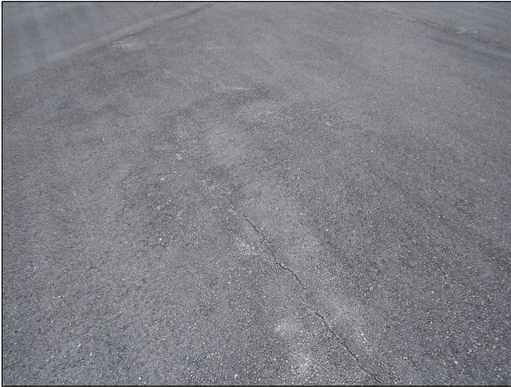
Taxiway A-4, Section 150, Sample Unit 417 – Low severity (52) Weathering and Raveling; low severity (48) Longitudinal and Transverse Cracking; low severity (56) Swelling
