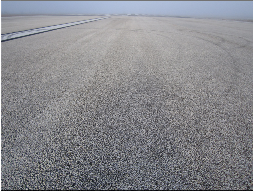
Runway 9-27, Section 6105, Sample Unit 304 – Low severity (52) Weathering and Raveling
