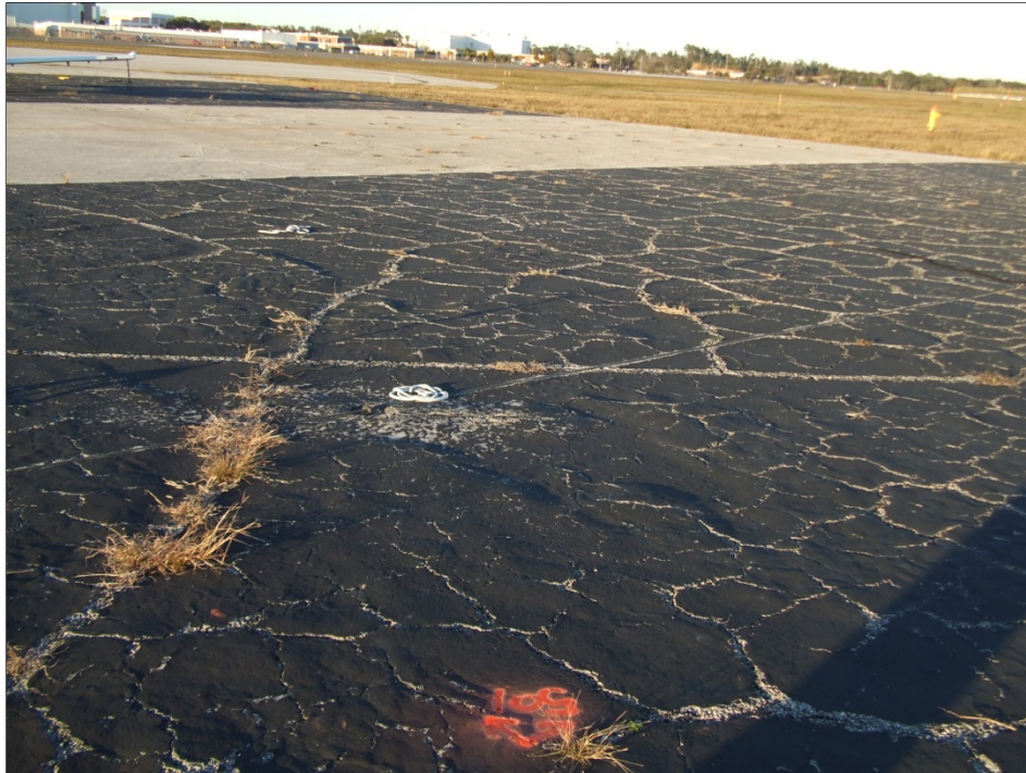
Nova Apron, Section 4305, Sample Unit 501 –Medium to high severity (43) Block Cracking; and low to medium severity (52) Weathering and Raveling.
