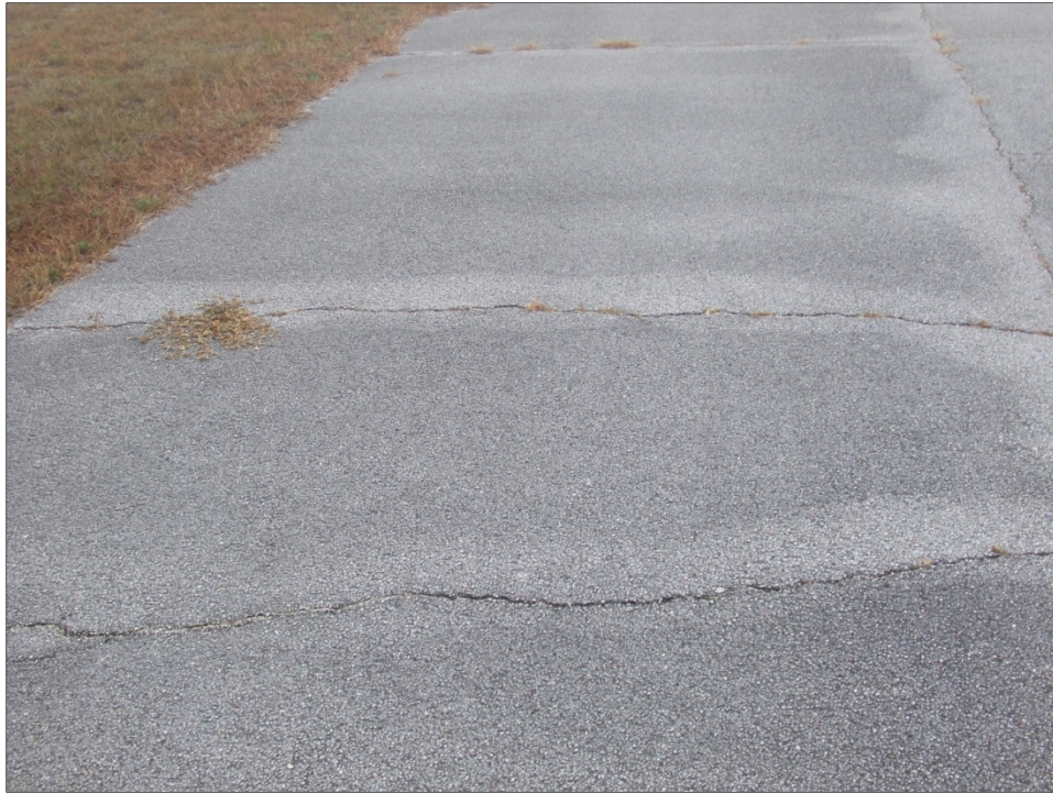
Taxiway Sierra, Section 1932, Sample Unit 205 – Medium severity (43) Block Cracking; and low severity (52) Weathering and Raveling.
