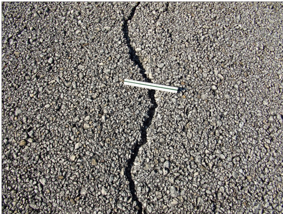
Taxiway November, Section 1408, Sample Unit 250 – Medium severity (48) Longitudinal / Transverse Cracking; and low severity (52) Weathering and Raveling.
