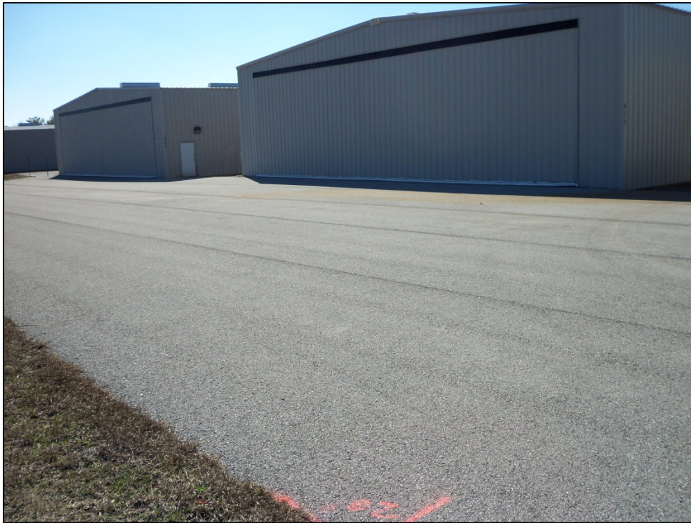
Apron, Section 4310, Sample Unit 208 – Low severity (48) Longitudinal and Transverse Cracking, low severity (52) Weathering and Raveling
