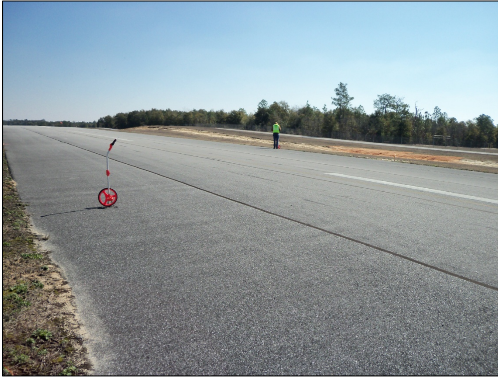
Runway 9-27, Section 6120, Sample Unit 95 – Low severity (48) Longitudinal and Transverse Cracking, low severity (52) Weathering and Raveling
