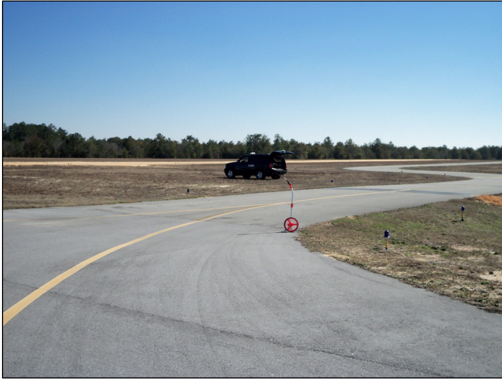
Taxiway Sierra, Section 710, Sample Unit 116 – Low severity (48) Longitudinal and Transverse Cracking, low and medium severity (52) Weathering and Raveling
