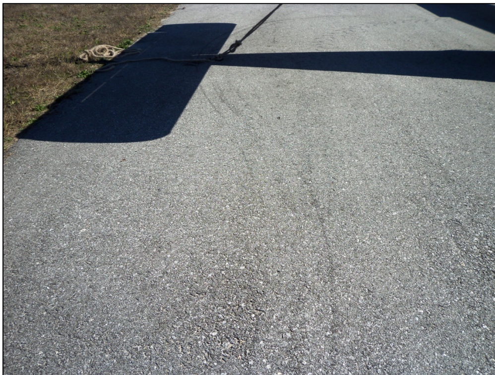
Apron, Section 4110, Sample Unit 303 – Low severity (52) Weathering and Raveling
