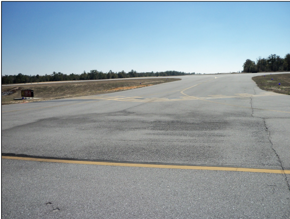
Taxiway Connector RW 9, Section 605, Sample Unit 101 – Low severity (48) Longitudinal and Transverse Cracking, low severity (52) Weathering and Raveling
