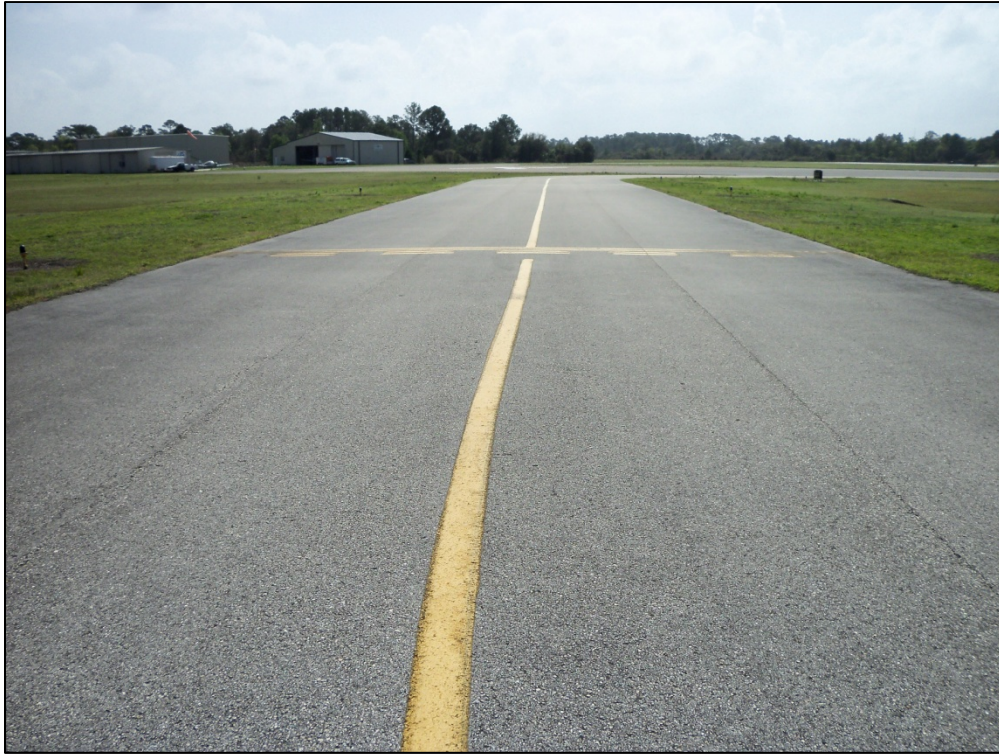
Taxiway Foxtrot, Section 115, Sample Unit 101 – Low severity (48) Longitudinal and Transverse Cracking, low severity (52) Weathering and Raveling
