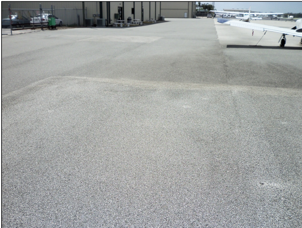
Apron, Section 4125, Sample Unit 201 – Low severity (48) Longitudinal and Transverse Cracking, low and medium severity (50) Patch, low severity (52) Weathering and Raveling
