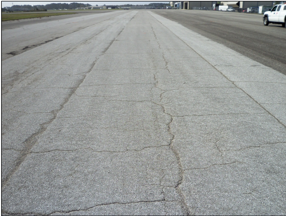
Taxiway Alpha, Section 150, Sample Unit 121 – Medium severity (43) Block Cracking, medium severity (52) Weathering and Raveling
