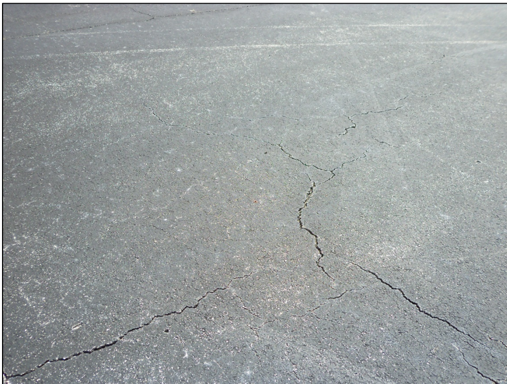
Apron, Section 4115, Sample Unit 302 – Low severity (43) Block Cracking, low and medium severity (48) Longitudinal and Transverse Cracking, medium severity (52) Weathering and Raveling
