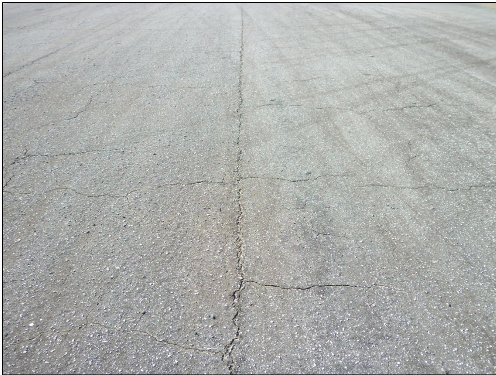
Taxiway Alpha, Section 162, Sample Unit 226 – Low severity (43) Block Cracking, medium severity (52) Weathering and Raveling
