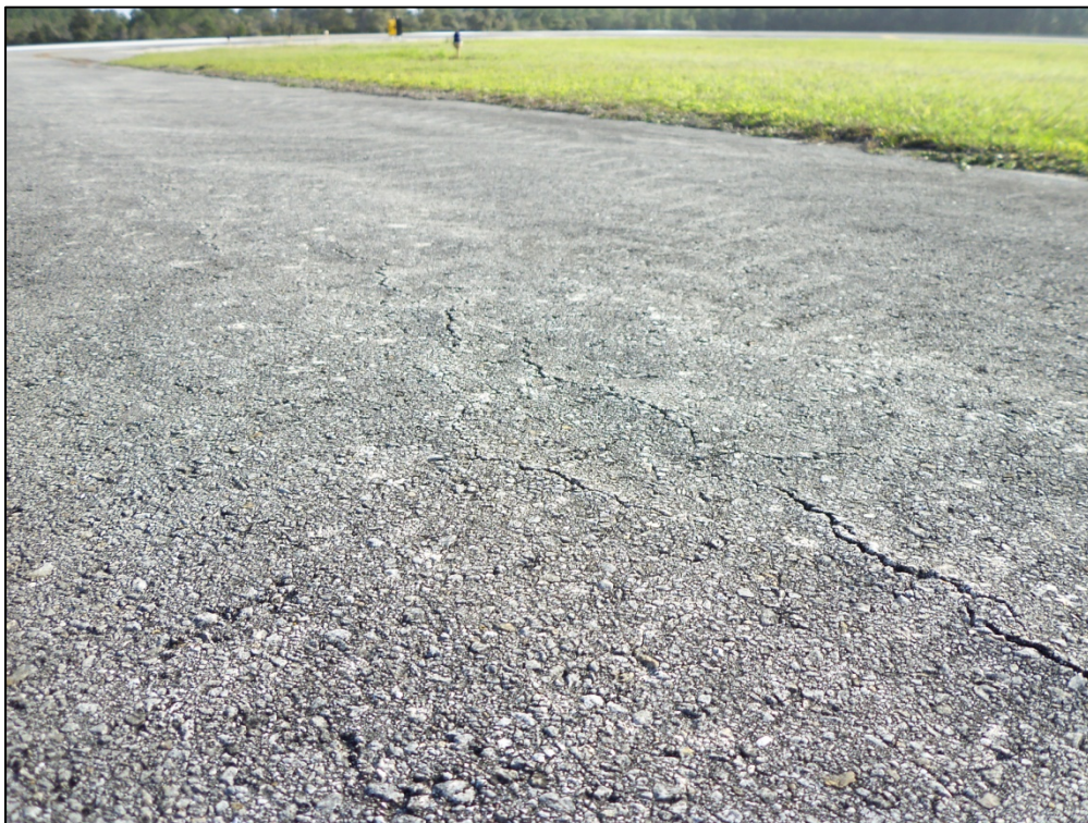
Taxiway Delta, Section 450, Sample Unit 401 – Low and medium severity (48) Longitudinal and Transverse Cracking, low severity (52) Weathering and Raveling, low severity (56) Swell
