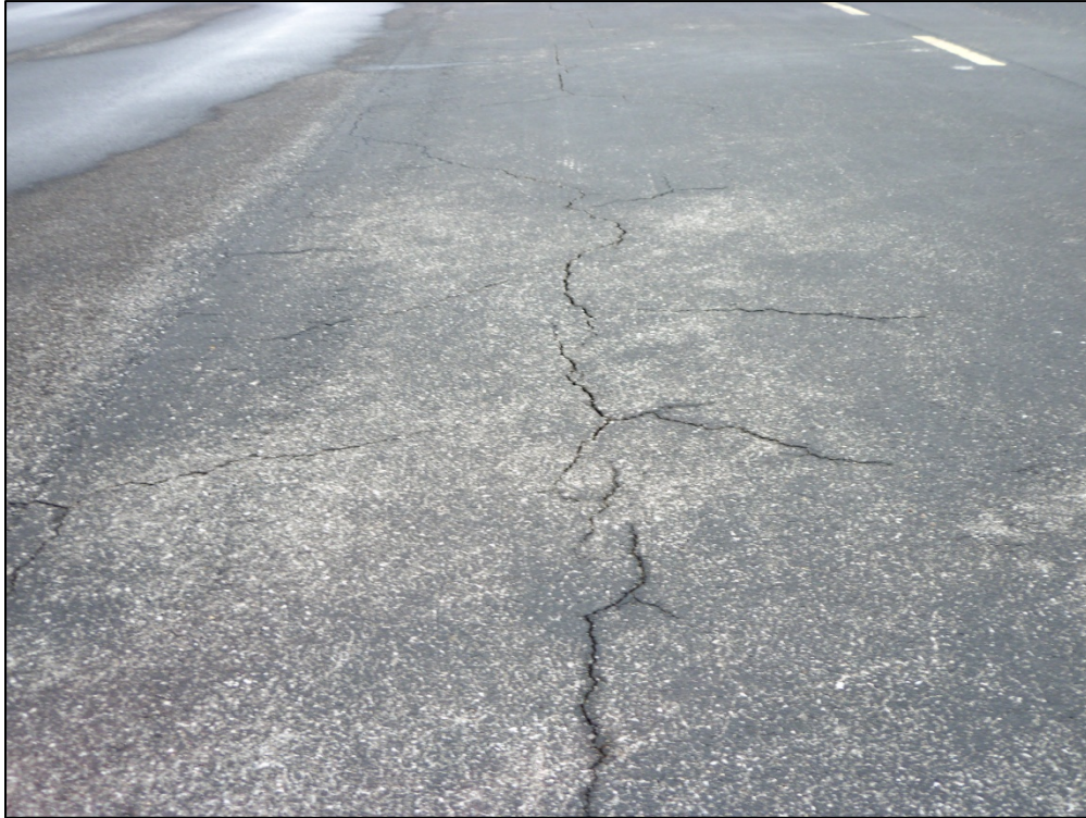
Apron, Section 4112, Sample Unit 307 – Medium severity (43) Block Cracking, low severity (52) Weathering and Raveling
