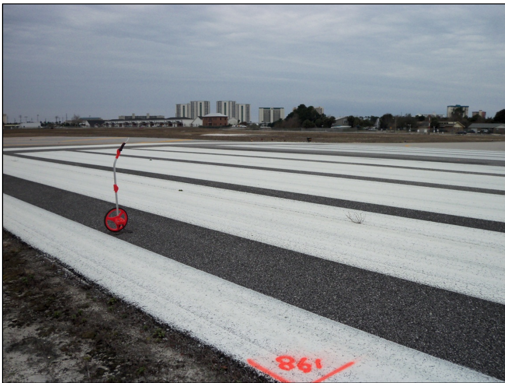
Runway 14-32, Section 6120, Sample Unit 198 – Low and medium severity (48) Longitudinal and Transverse Cracking, low severity (52) Weathering and Raveling
