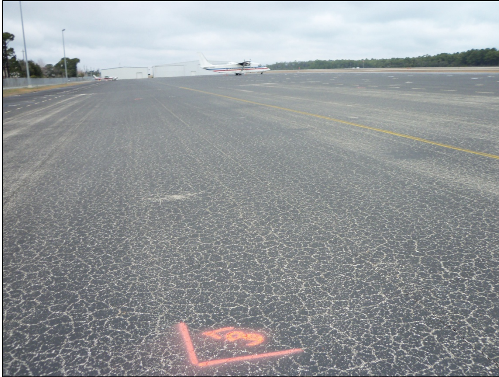
Apron, Section 4125, Sample Unit 607 – Low severity (43) Block Cracking, medium severity (48) Longitudinal and Transverse Cracking, medium severity (52) Weathering and Raveling
