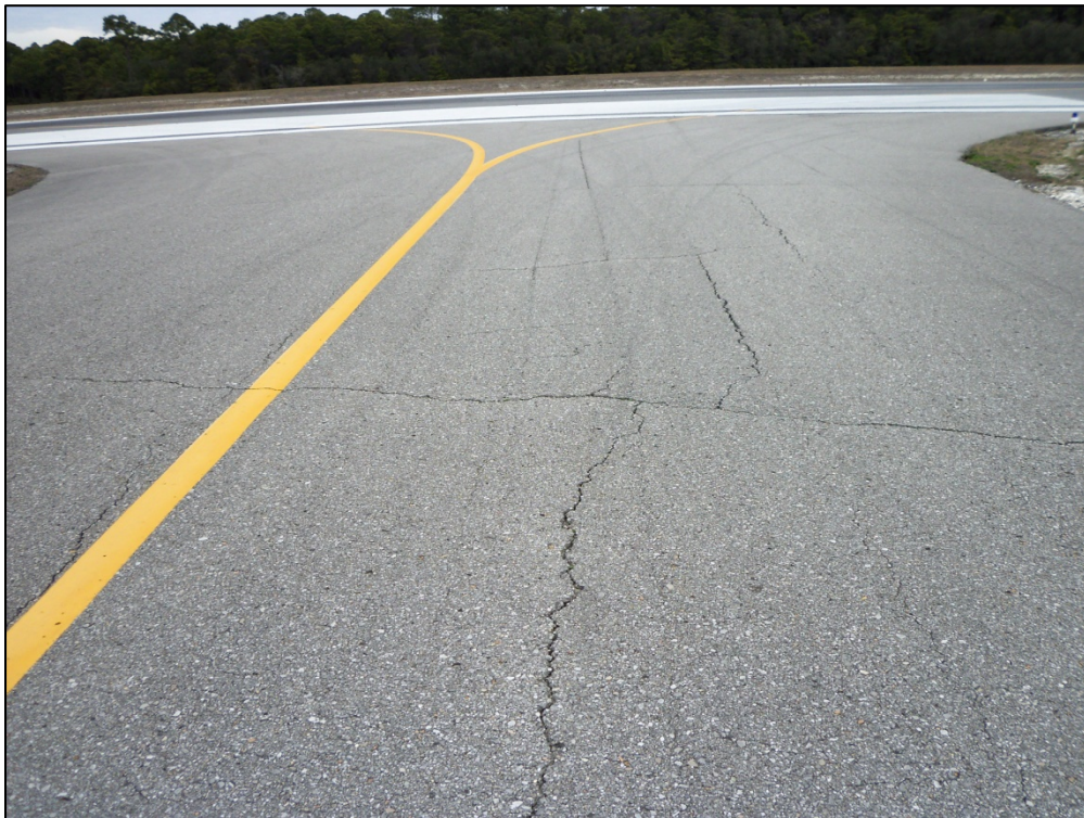
Taxiway A2, Section 110, Sample Unit 200 – Low severity (43) Block Cracking, medium severity (48) Longitudinal and Transverse Cracking, low severity (52) Weathering and Raveling
