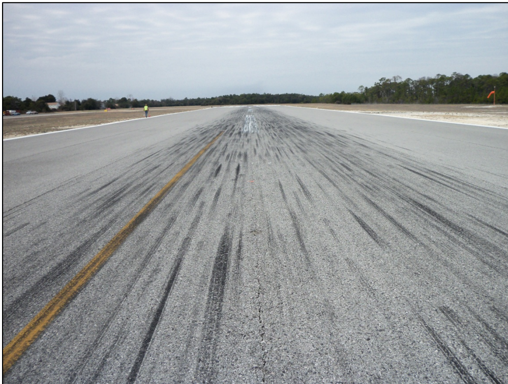
Runway 14-32, Section 6115, Sample Unit 117 – Low and medium severity (48) Longitudinal and Transverse Cracking, medium severity (52) Weathering and Raveling
