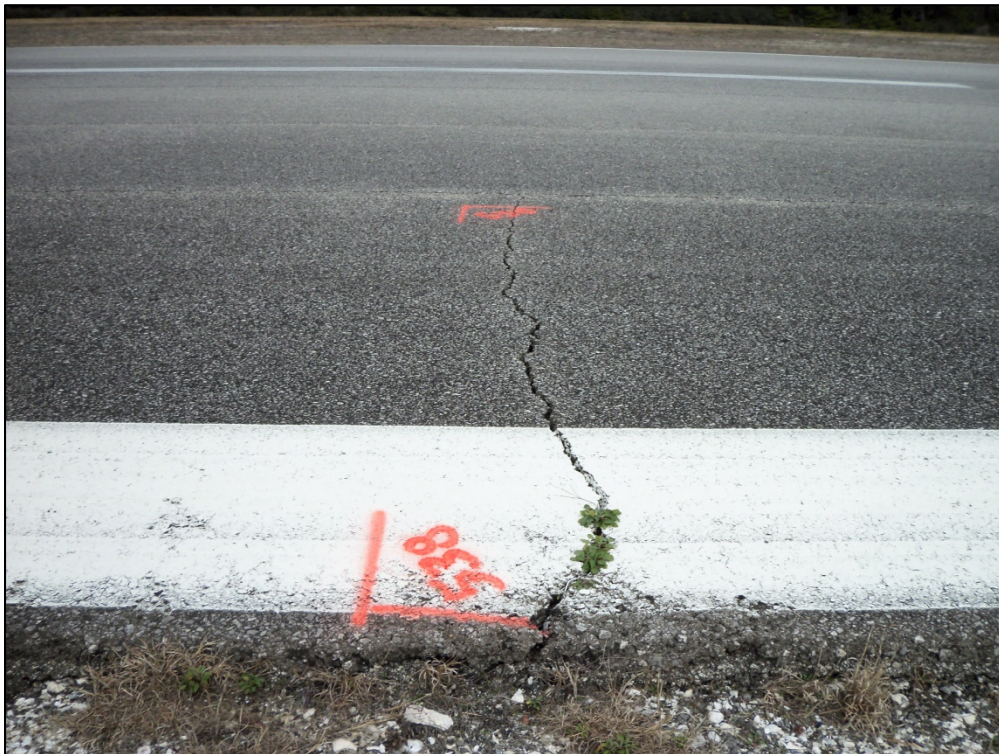
Runway 14-32 Shoulder, Section 6110, Sample Unit 538 – Medium severity (48) Longitudinal and Transverse Cracking, low severity (52) Weathering and Raveling
