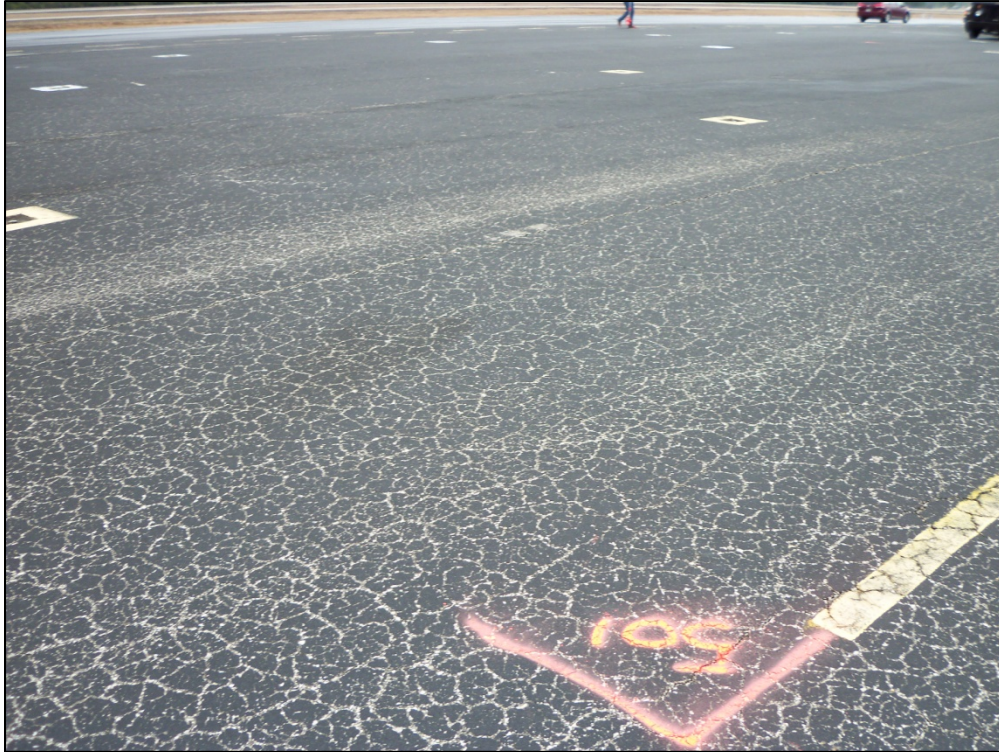
Apron, Section 4125, Sample Unit 501 – Low severity (43) Block Cracking, medium severity (48) Longitudinal and Transverse Cracking, medium severity (52) Weathering and Raveling
