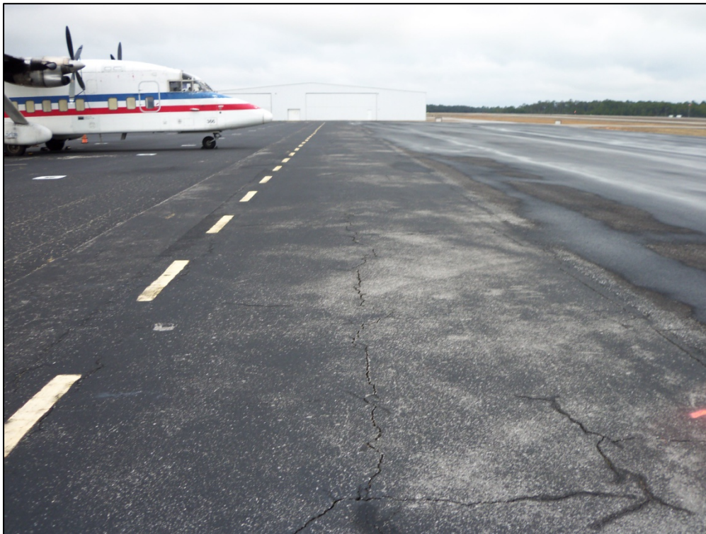
Apron, Section 4107, Sample Unit 302 – Medium severity (43) Block Cracking, medium severity (52) Weathering and Raveling
