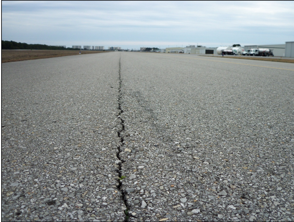
Taxiway Alpha, Section 150, Sample Unit 103 – Medium severity (48) Longitudinal and Transverse Cracking, low severity (52) Weathering and Raveling
