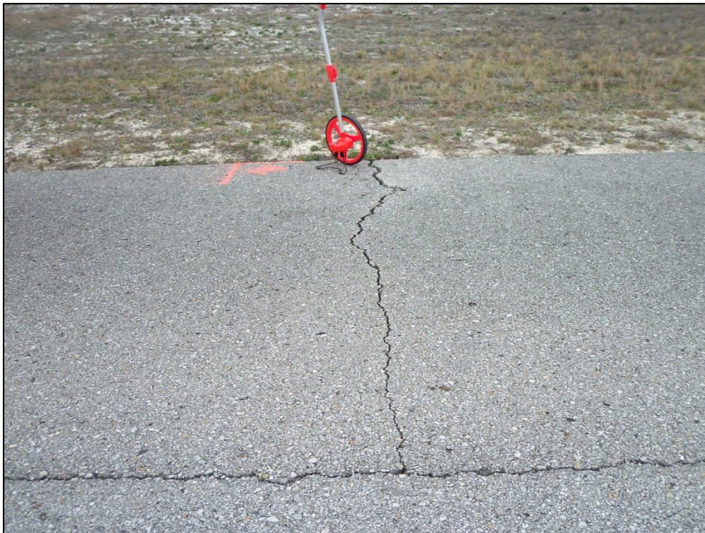
Taxiway Alpha, Section 115, Sample Unit 111 – Low and medium severity (48) Longitudinal and Transverse Cracking, low severity (52) Weathering and Raveling
