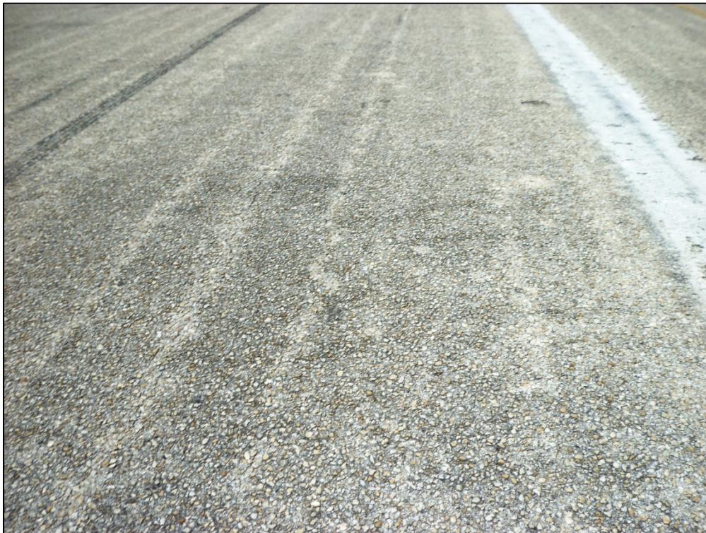
Runway 15-33, Section 6105, Sample Unit 101 – Low severity (48) Longitudinal and Transverse Cracking, low and medium severity (52) Weathering and Raveling
