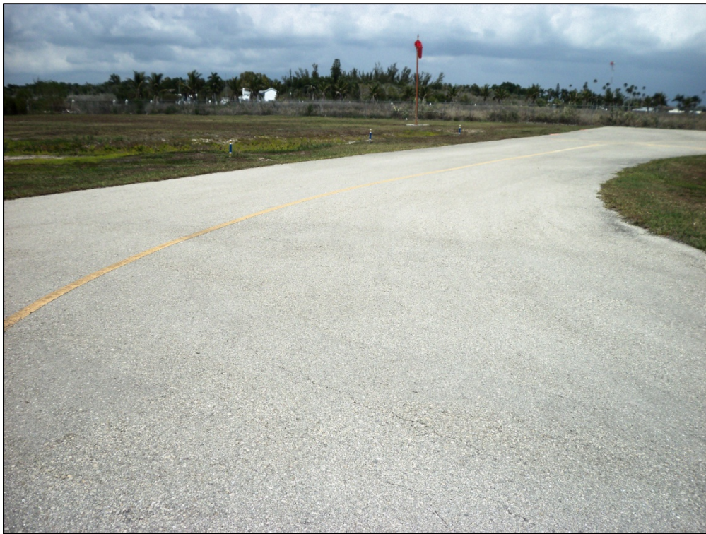
Taxiway Connector, Section 115, Sample Unit 214 – Low severity (48) Longitudinal and Transverse Cracking, low severity (52) Weathering and Raveling
