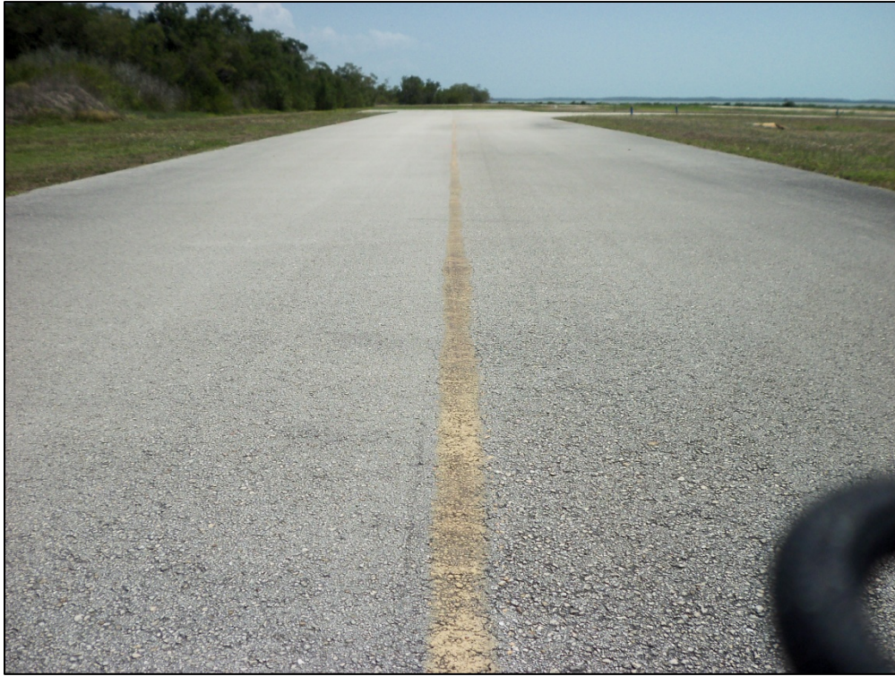
Taxiway Alpha, Section 105, Sample Unit 103 – Low severity (52) Weathering and Raveling
