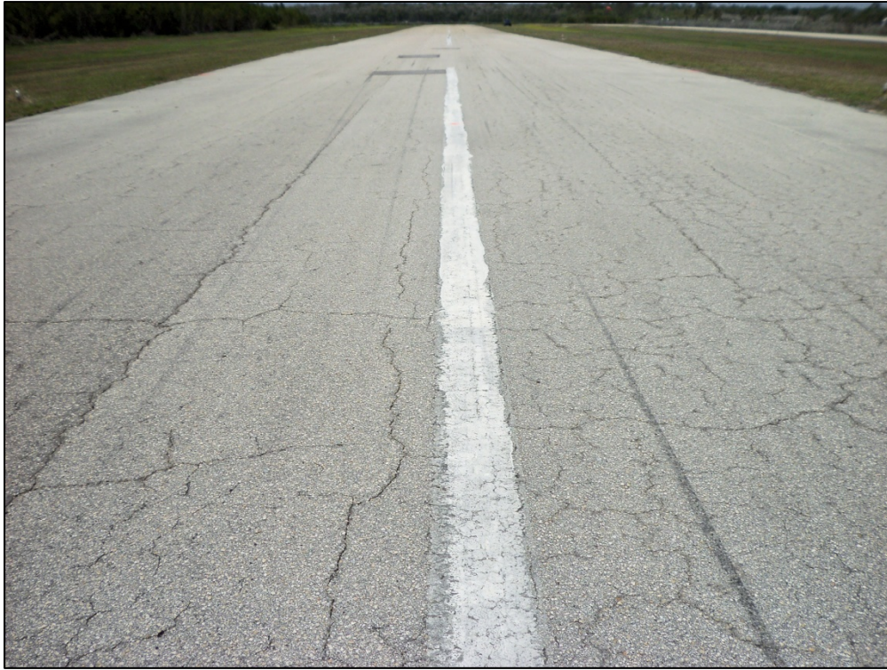
Runway 15-33, Section 6110, Sample Unit 109 – Medium severity (43) Block Cracking, low severity (45) Depression, medium severity (50) Patch, low and medium severity (52) Weathering and Raveling
