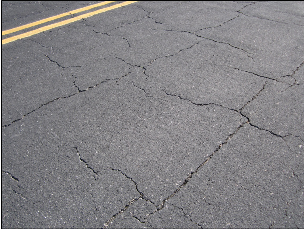
Taxiway Echo, Section 550, Sample Unit 146 – Medium severity (43) Block Cracking, low severity (52) Weathering and Raveling
