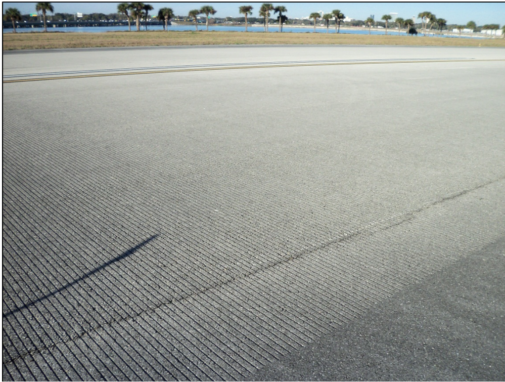
Runway 13-31, Section 6205, Sample Unit 115 – Low severity (48) Longitudinal and Transverse Cracking
