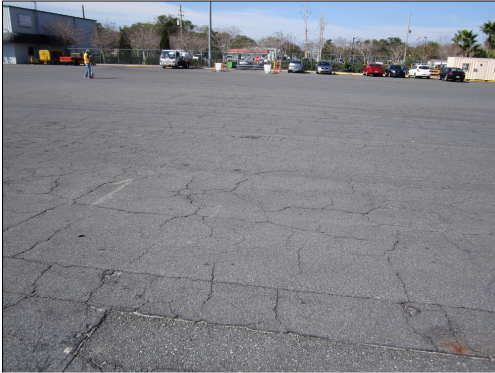
West Apron, Section 4610, Sample Unit 421 – Low severity (43) Block Cracking
