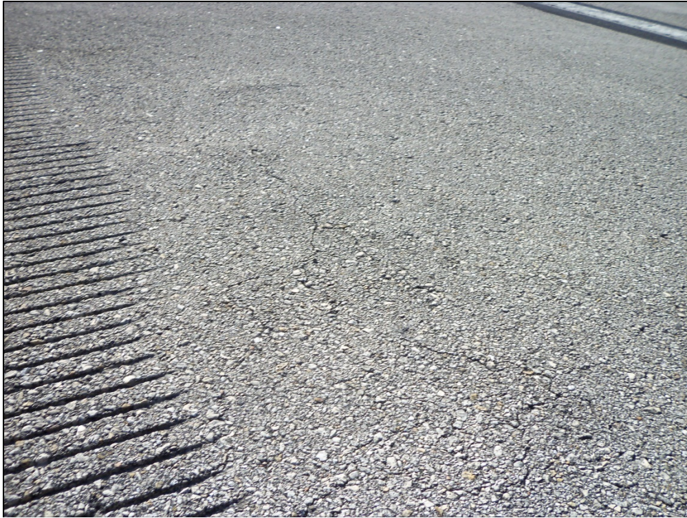
Runway 13-31, Section 6205, Sample Unit 198 – Low severity (48) Longitudinal and Transverse Cracking, low severity (56) Swelling, low severity (52) Weathering and Raveling
