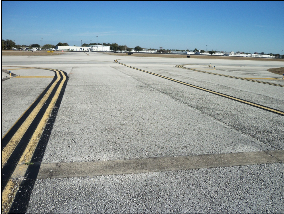
Taxiway E-3, Section 520, Sample Unit 412 – Low and medium severity (48) Longitudinal and Transverse Cracking, medium severity (52) Weathering and Raveling, medium severity (50) Patching
