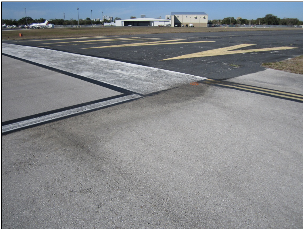
Taxiway Echo, Section 815, Sample Unit 103 – Low severity (45) Depression, low severity (52) Weathering and Raveling
