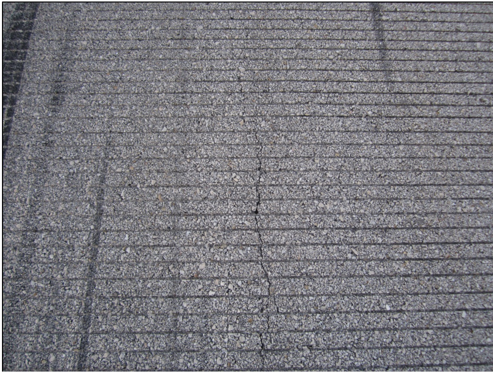
Runway 7-25, Section 6105, Sample Unit 391 – Low severity (48) Longitudinal and Transverse Cracking, low severity (52) Weathering and Raveling
