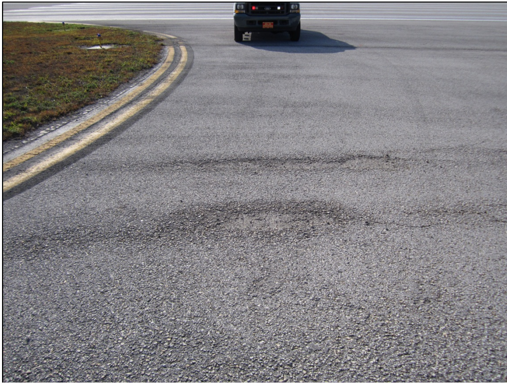
Taxiway E-4, Section 1085, Sample Unit 101 – Low severity (48) Longitudinal and Transverse Cracking; low, medium, and high severity (52) Weathering and Raveling
