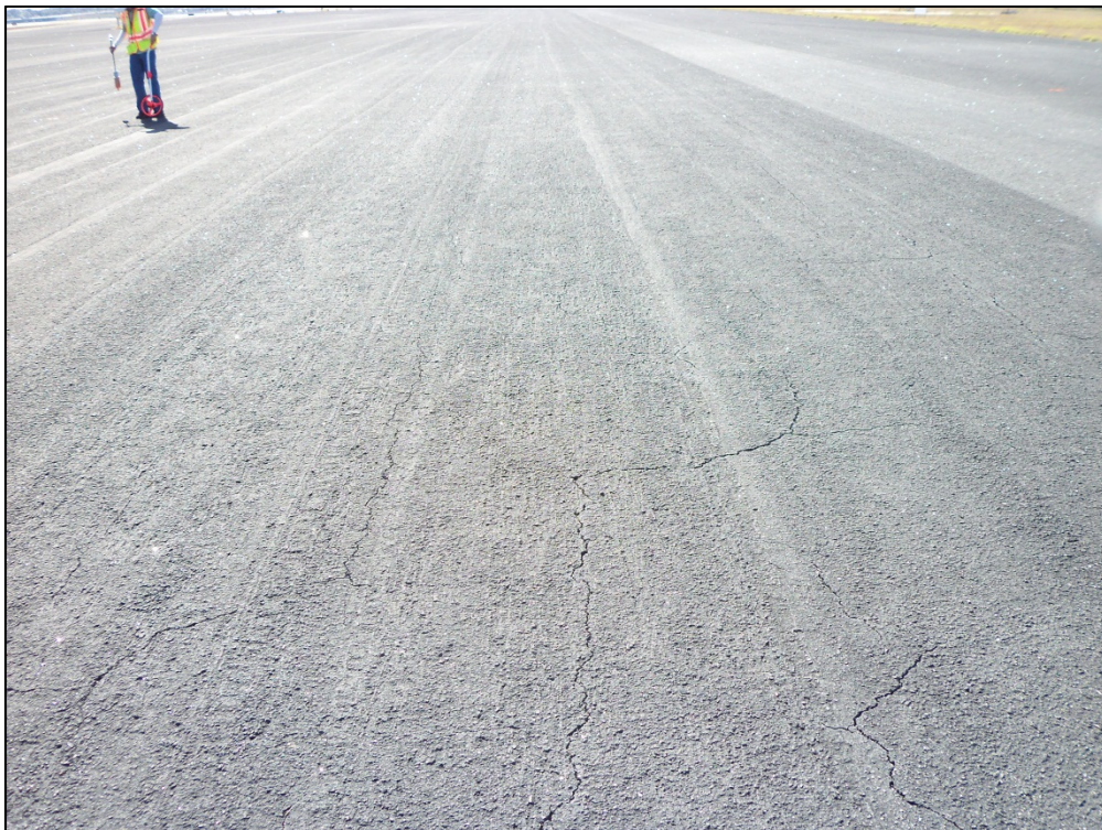
GA Apron, Section 4205, Sample Unit 165 – Low severity (48) Longitudinal and Transverse Cracking
