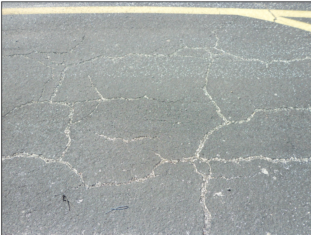
Northeast Apron, Section 4305, Sample Unit 404 – Medium severity (43) Block Cracking, medium severity (52) Weathering and Raveling
