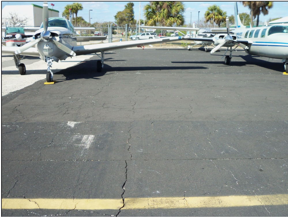
Northeast Apron, Section 4305, Sample Unit 350 – Low severity (43) Block Cracking
