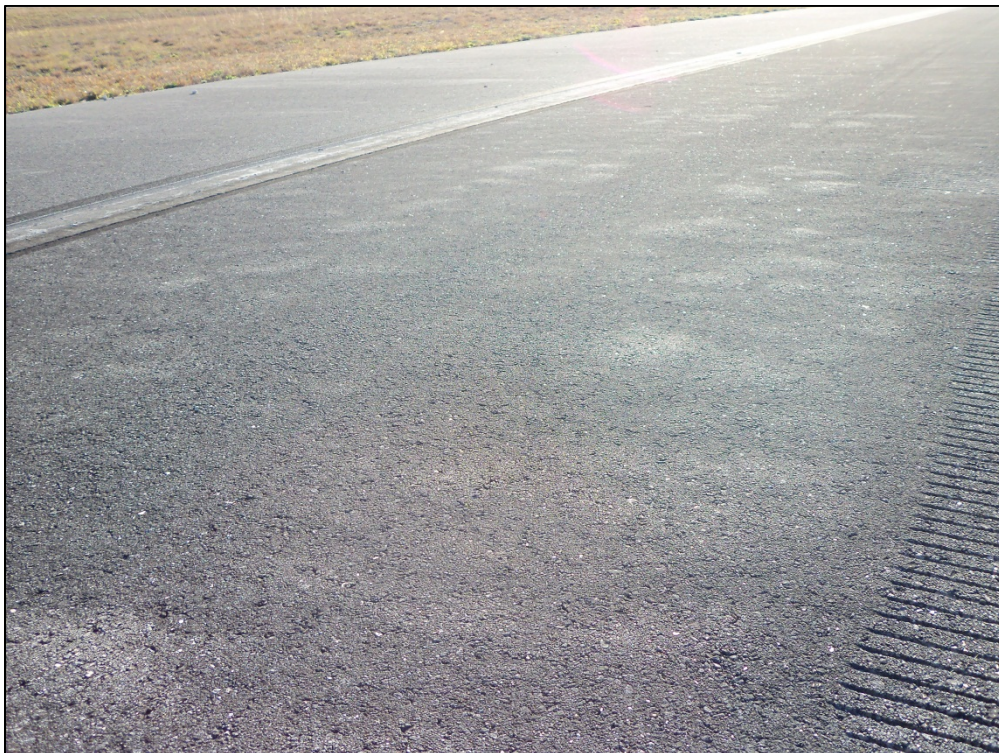
Runway 13-31, Section 6205, Sample Unit 122 – Low severity (56) Swelling
