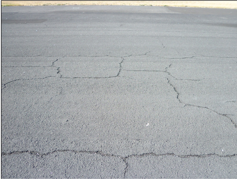
GA Apron, Section 4205, Sample Unit 154 – Low and medium severity (48) Longitudinal and Transverse Cracking
