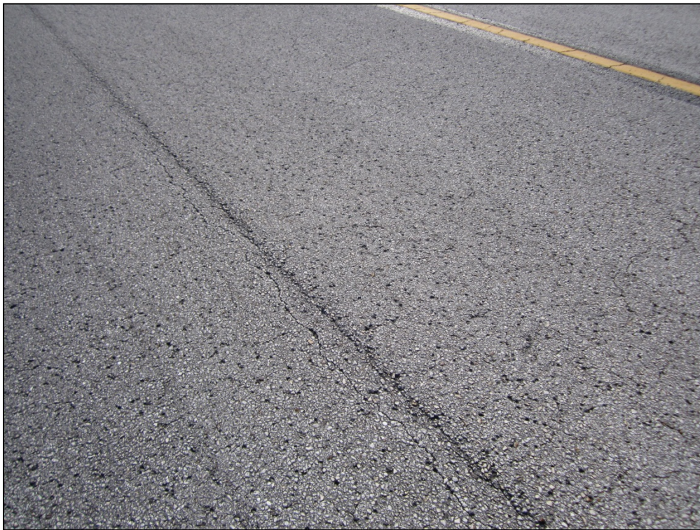
Taxiway Foxtrot, Section 605, Sample Unit 602 – Low severity (48) Longitudinal and Transverse Cracking, low severity (52) Weathering and Raveling
