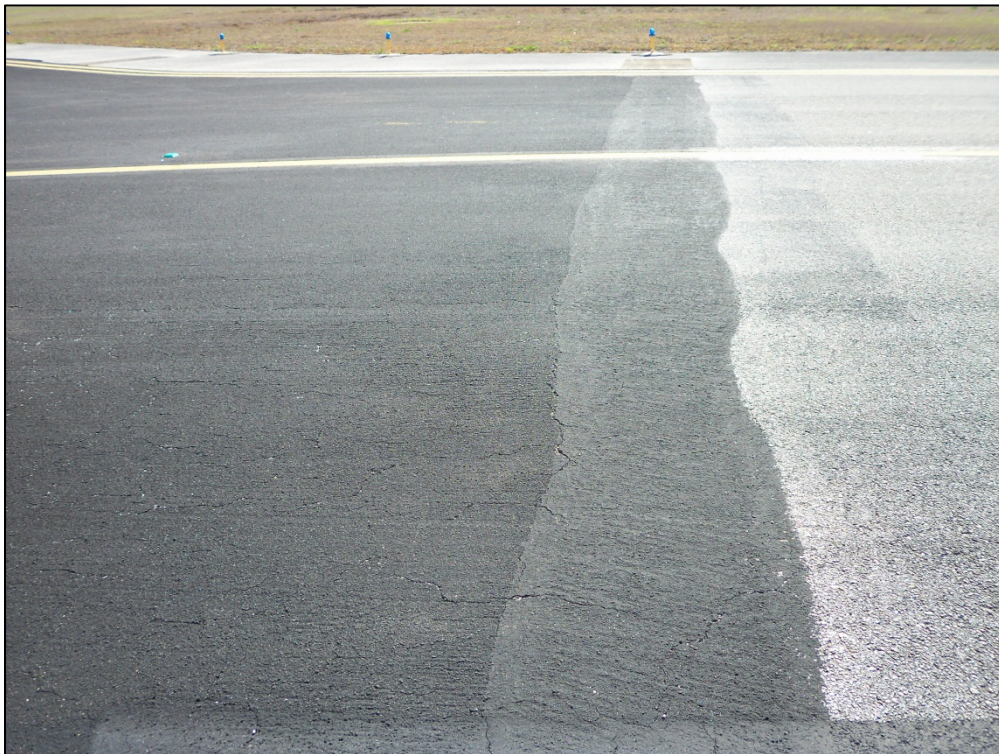
Taxiway E-4, Section 1105, Sample Unit 104 – Low severity (52) Weathering and Raveling, low severity (48) Longitudinal and Transverse Cracking
