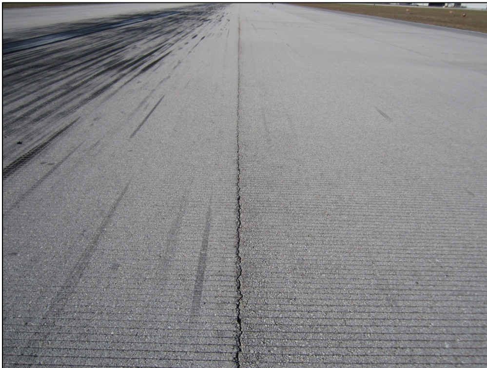
Runway 7-25, Section 6105, Sample Unit 321 – Low severity (48) Longitudinal and Transverse Cracking
