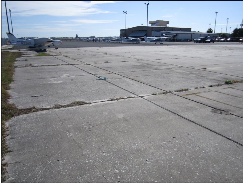
West Apron, Section 4665, Sample Unit 911 – Low severity (65) Joint Seal Damage, low severity (63) Longitudinal, Transverse, and Diagonal Cracking; low and medium severity (74) Joint Spalling, low and medium severity (75) Corner Spalling
