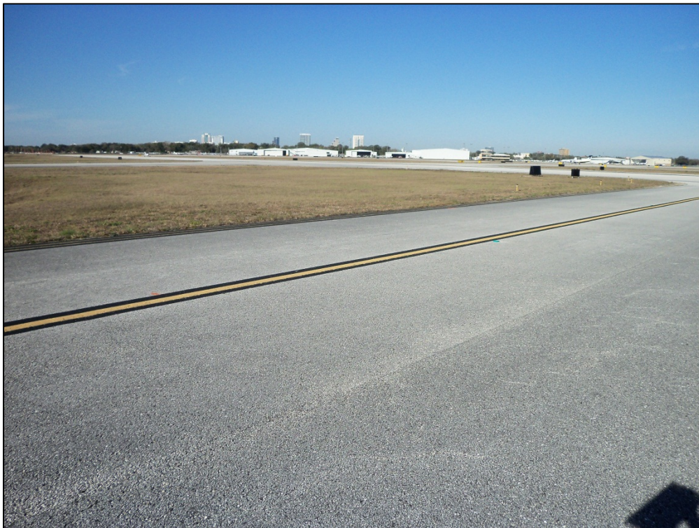
Taxiway Echo, Section 505, Sample Unit 118 – Low severity (48) Longitudinal and Transverse Cracking, low severity (52) Weathering and Raveling
