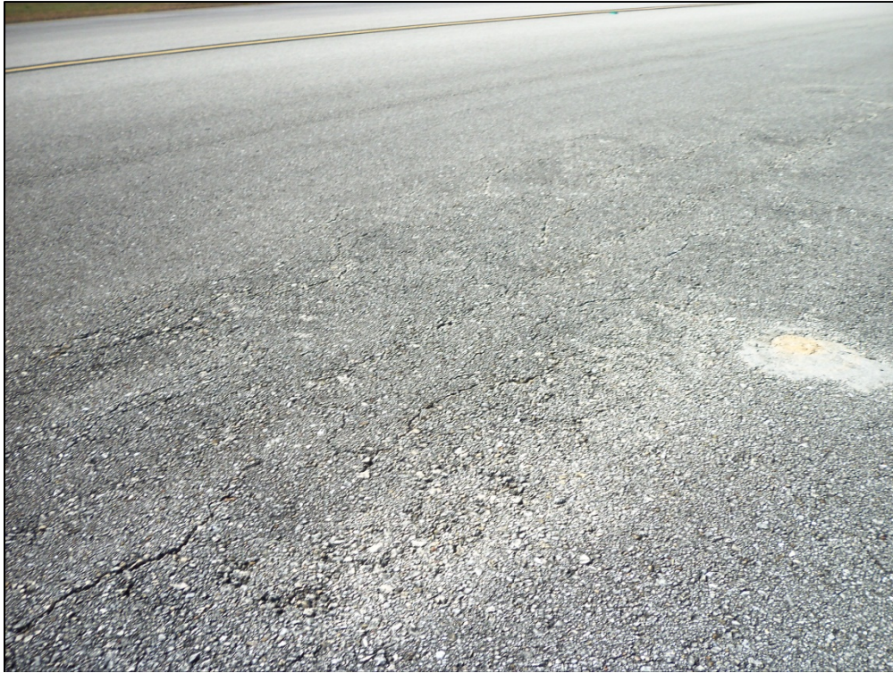
Taxiway Bravo, Section 103, Sample Unit 190 – Low severity (48) Longitudinal and Transverse Cracking, low severity (52) Weathering and Raveling, low severity (56) Swelling
