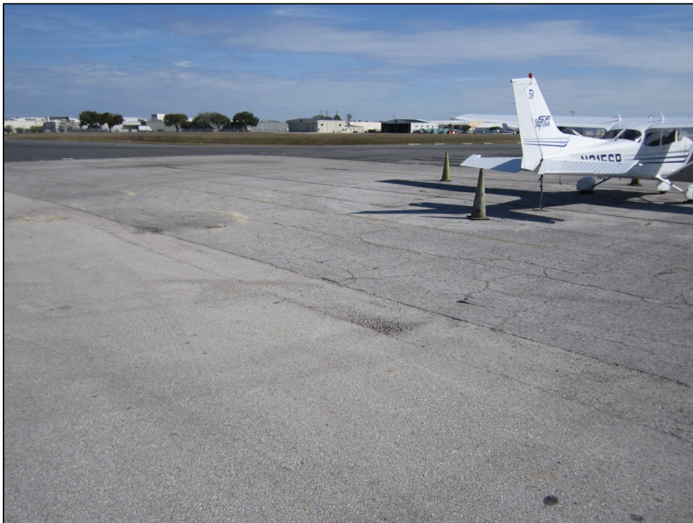
West Apron, Section 4660, Sample Unit 507 – Medium severity (43) Block Cracking; low and medium severity (52) Weathering and Raveling; low and medium severity (45) Depression
