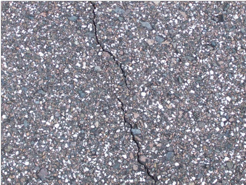
Taxiway Alpha, Section 335, Sample Unit 149 – Low severity (48) Longitudinal and Transverse Cracking.
