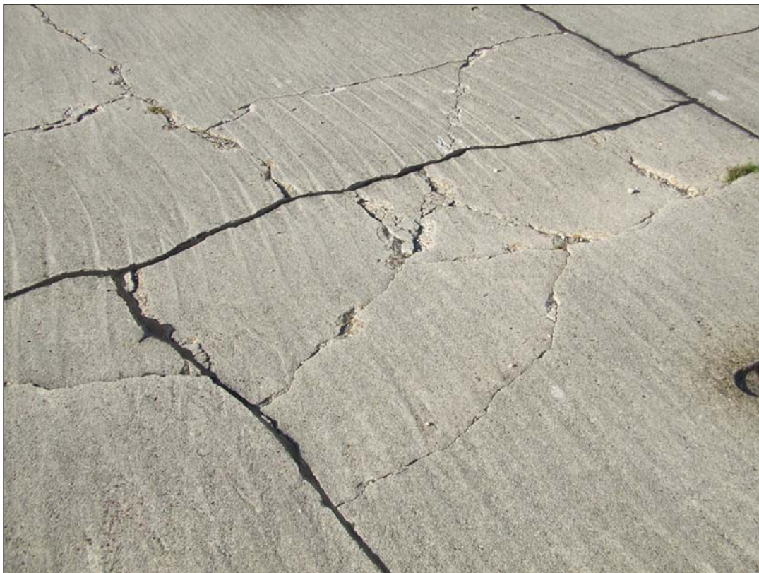
Apron North – Terminal, Section 4210, Sample Unit 219 – Low severity (65) Joint Seal Damage, low severity (70) Scaling, and high severity (72) Shattered Slab.
