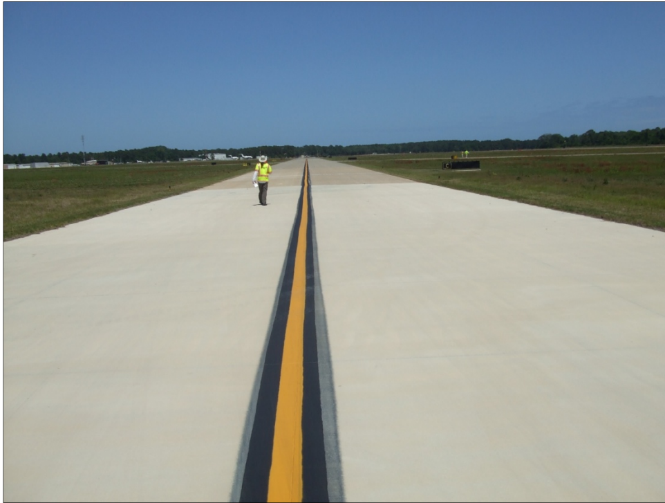
Taxiway Charlie, Section 125, Sample Unit 100 – New Pavement, No Distress.
