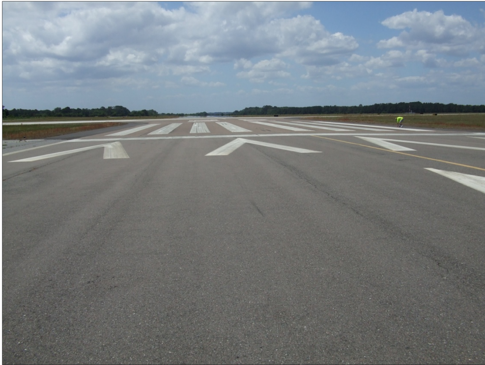
Runway 4-22, Section 6105, Sample Unit 199 – Low severity (48) Longitudinal and Transverse Cracking and low severity (52) Weathering and Raveling.
