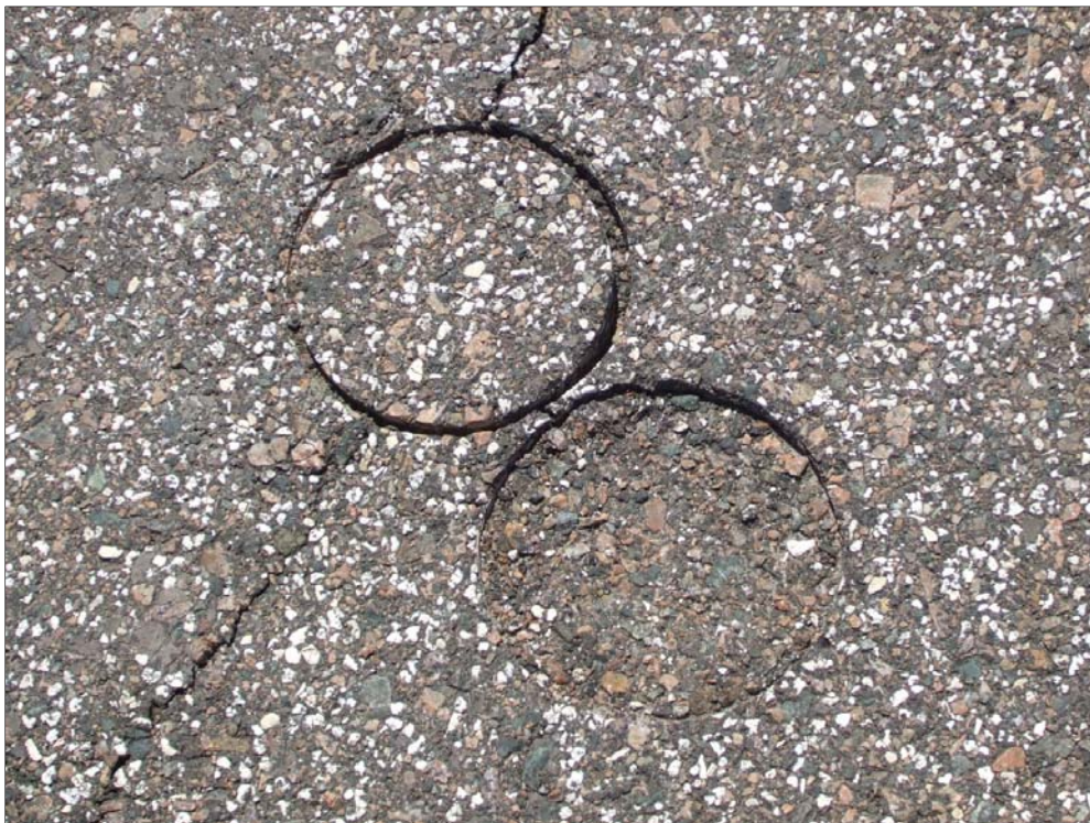
Runway 4-22, Section 6105, Sample Unit 136 – Low severity (48) Longitudinal / Transverse Cracking, low severity (50) Patching and low severity (52) Weathering and Raveling.
