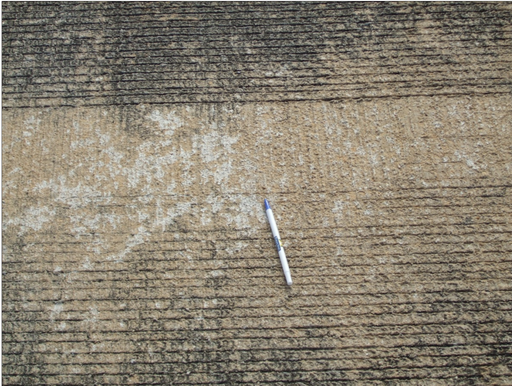
Runway 9-27, Section 6305, Sample Unit 304 – Medium severity (70) Scaling / Map Cracking / Crazing
