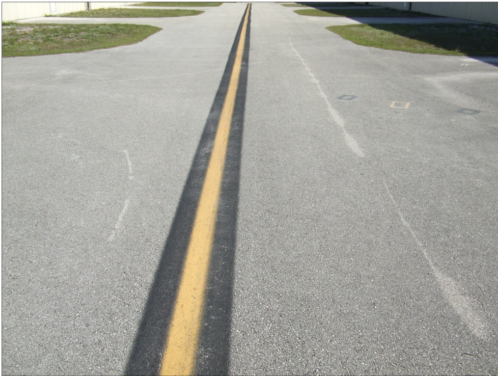
Apron T-Hangar, Section 4310, Sample Unit 302 – Low severity (52) Weathering and Raveling.
