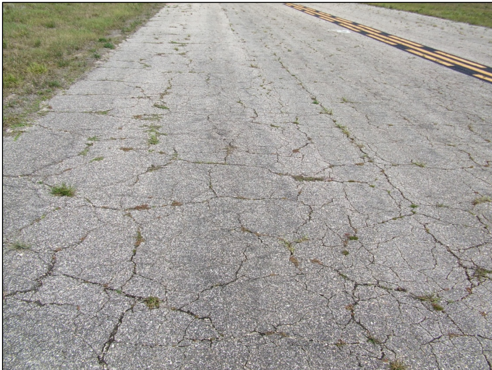
Taxiway Delta, Section 405, Sample Unit 103 – Medium to high severity (43) Block cracking and medium severity (52) Weathering / Raveling.
