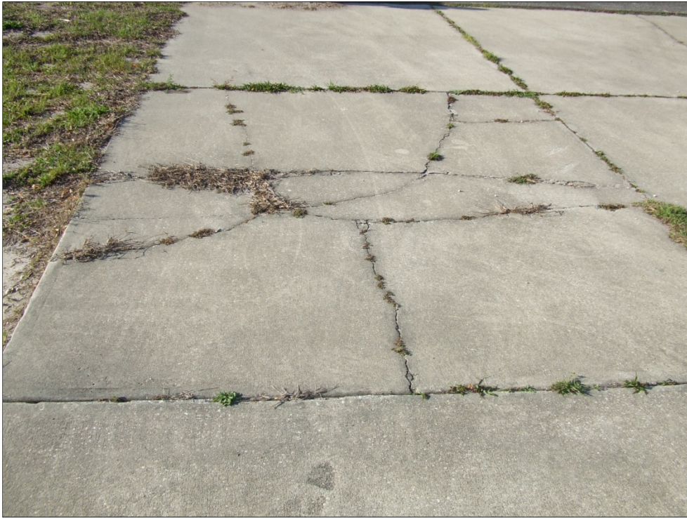
Apron, Section 4130, Sample Unit 101 – High severity (65) Joint Seal Damage and high severity (72) Shattered Slab.
