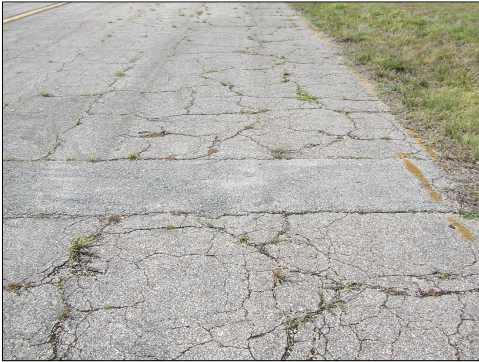
Taxiway Delta, Section 405, Sample Unit 101 – Low severity (41) Alligator Cracking, low to medium severity (43) Block cracking, low severity (50) Patching, and low to medium severity (52) Weathering and Raveling.
