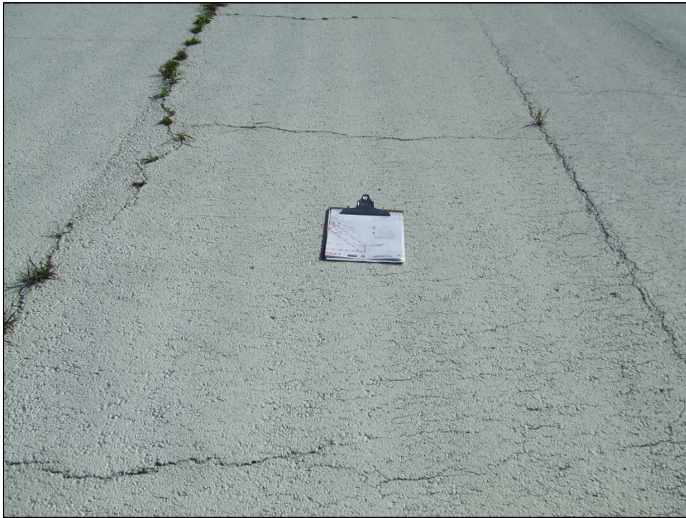
Runway 6-24, Section 6205, Sample Unit 177 – Low to medium severity (48) Longitudinal and Transverse Cracking and low severity (52) Weathering and Raveling.
