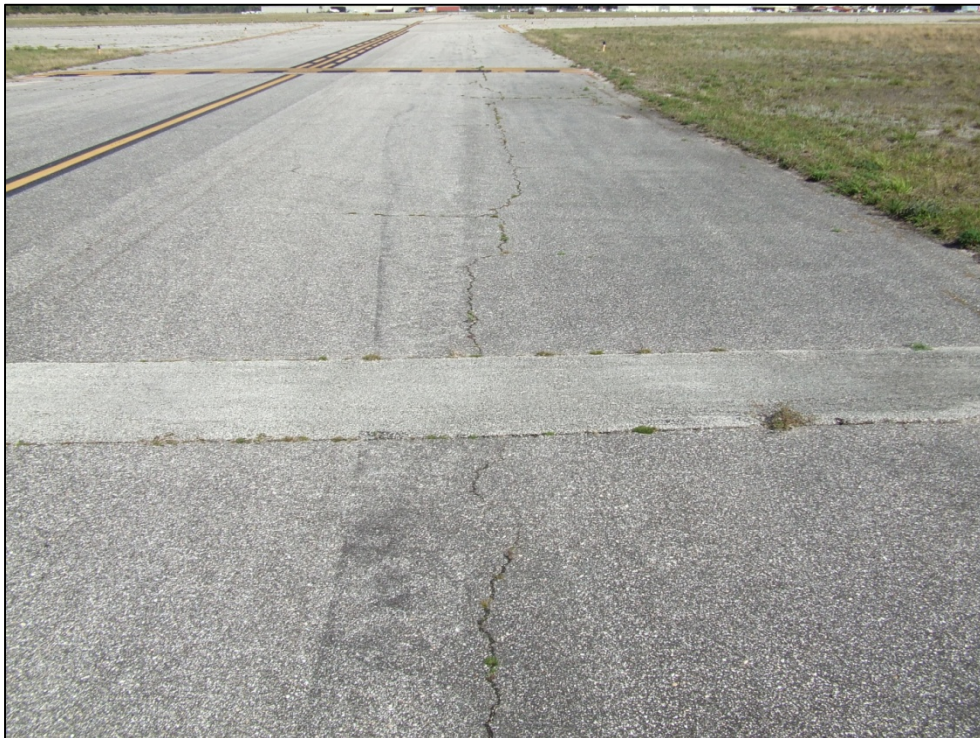
Taxiway Charlie, Section 310, Sample Unit 101 – Low to medium severity (48) Longitudinal and Transverse Cracking; medium severity (50) patching, low severity (52) Weathering and Raveling.
