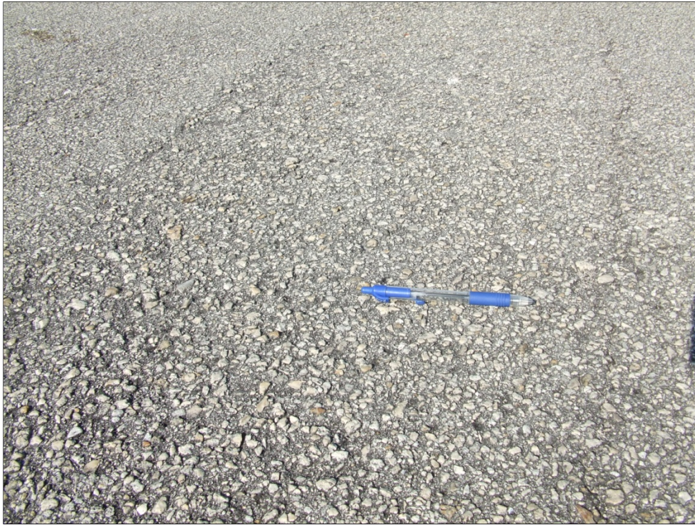
Taxiway Sierra, Section 1965, Sample Unit 5 – Low severity (48) Longitudinal and Transverse Cracking and medium severity (52) Weathering and Raveling.
