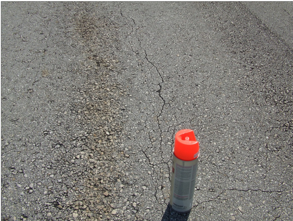
Taxiway Charlie, Section 305, Sample Unit 309 – Low severity (48) Longitudinal and Transverse Cracking and low severity (52) Weathering and Raveling.
