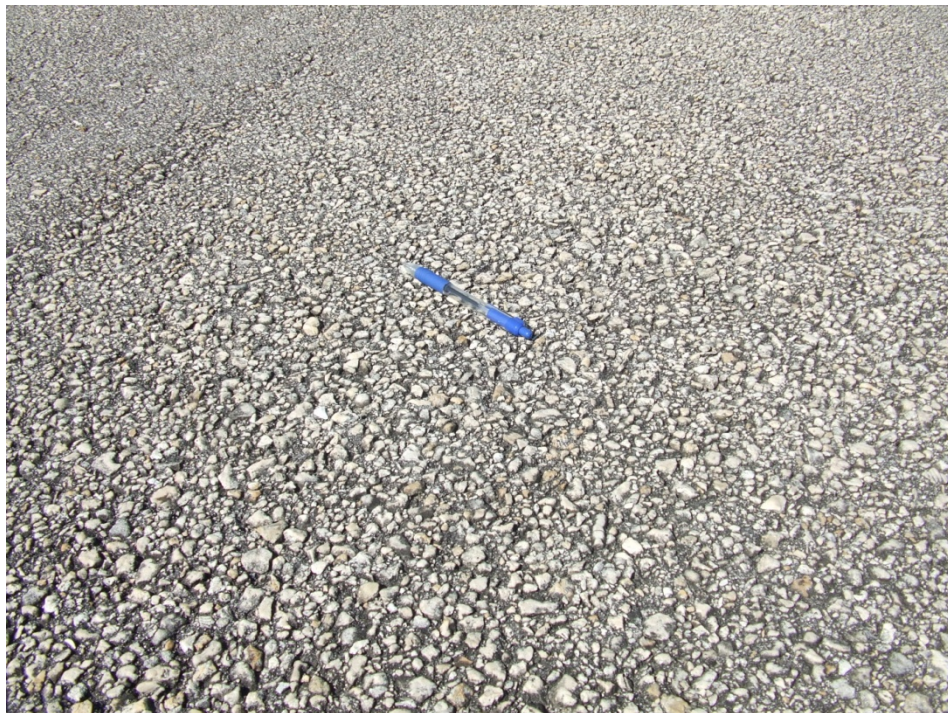
Taxiway Foxtrot, Section 607, Sample Unit 138 – Medium severity (52) Weathering and Raveling.
