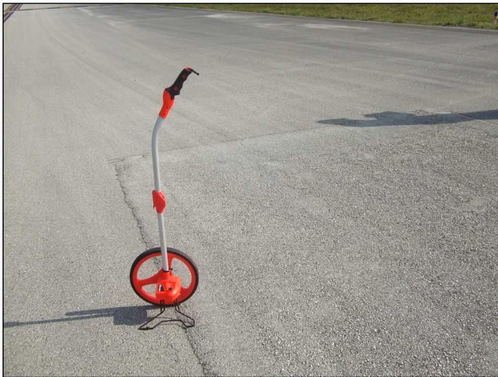
Taxiway Papa, Section 1610, Sample Unit 2 – Low severity (50) Patching and low severity (52) Weathering and Raveling.
