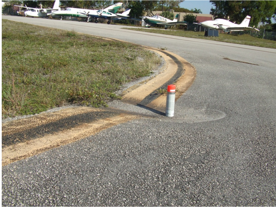
Taxiway S-1, Section 1950, Sample Unit 150 – High severity (45) Depression and low to high severity (52) Weathering and Raveling.
