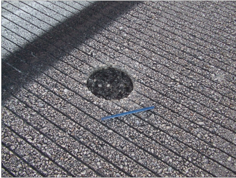
Runway 13-31, Section 6205, Sample Unit 175 – Medium severity (50) Patching and low severity (52) Weathering and Raveling.
