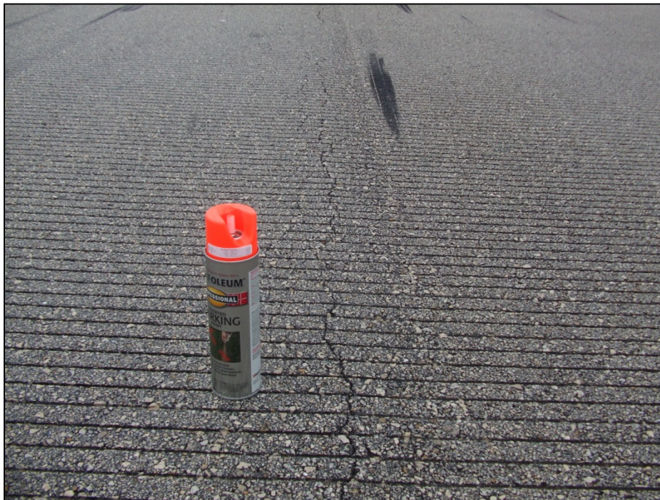
Runway 8-26, Section 6105, Sample Unit 303 – Low severity (48) Longitudinal and Transverse Cracking and low severity (52) Weathering and Raveling.
