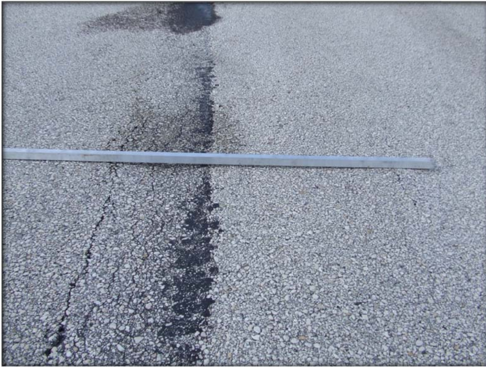
Taxiway A, Section 105, Sample Unit 302 – Low severity (52) Weathering and Raveling, Low severity (53) Rutting, (42) Bleeding
