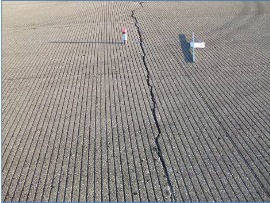
Runway 7-25, Section 6105, Sample Unit 534 – Low severity (42) Bleeding; low, medium and high severity (48) Longitudinal and Transverse Cracking; low and medium severity (52) Weathering and Raveling
