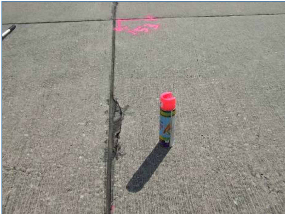
South Aprons, Section 4110, Sample Unit 153 – Low severity (65) Joint Seal Damage, low severity (73) Shrinkage Cracking, medium and high severity (74) Joint Spalling.
