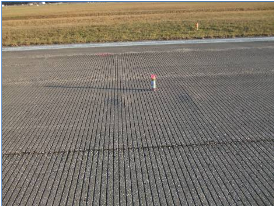
Runway 7-25, Section 6105, Sample Unit 525 – Low severity (42) Bleeding, low and medium severity (48) Longitudinal and Transverse Cracking, low severity (52) Weathering and Raveling
