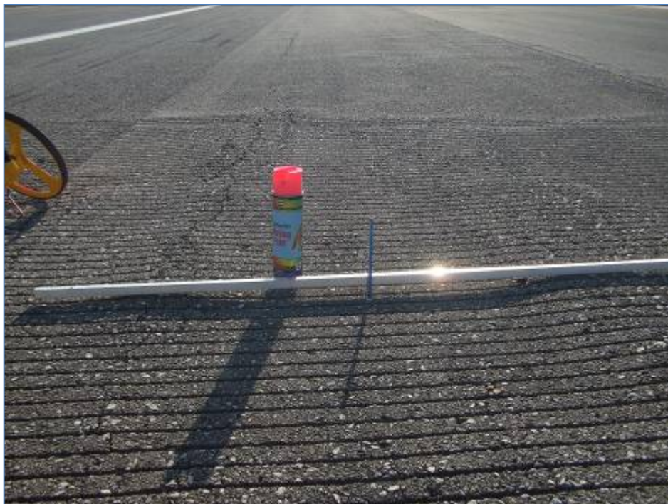
Runway 7-25, Section 6105, Sample Unit 567 – Low and medium severity (48) Longitudinal and Transverse Cracking, low and medium severity (52) Weathering and Raveling, medium severity (53) Rutting, low severity (56) Swelling
