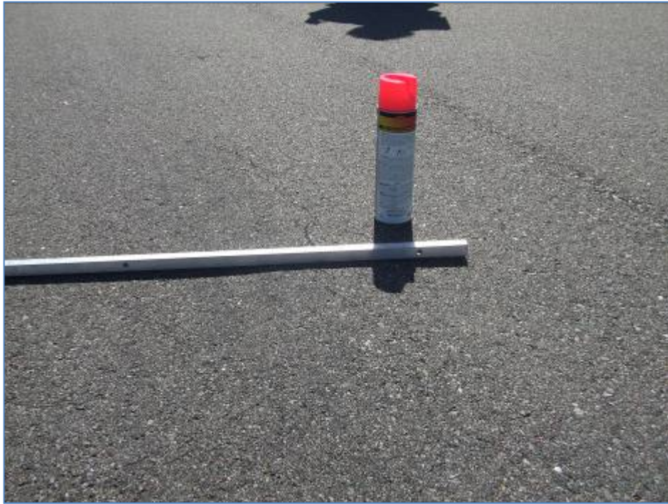
Taxiway Echo 1, Section 515, Sample Unit 102 – Low severity (48) Longitudinal and Transverse Cracking, low severity (50) Patching, low and medium severity (52) Weathering and Raveling, low severity (56) Swelling.
