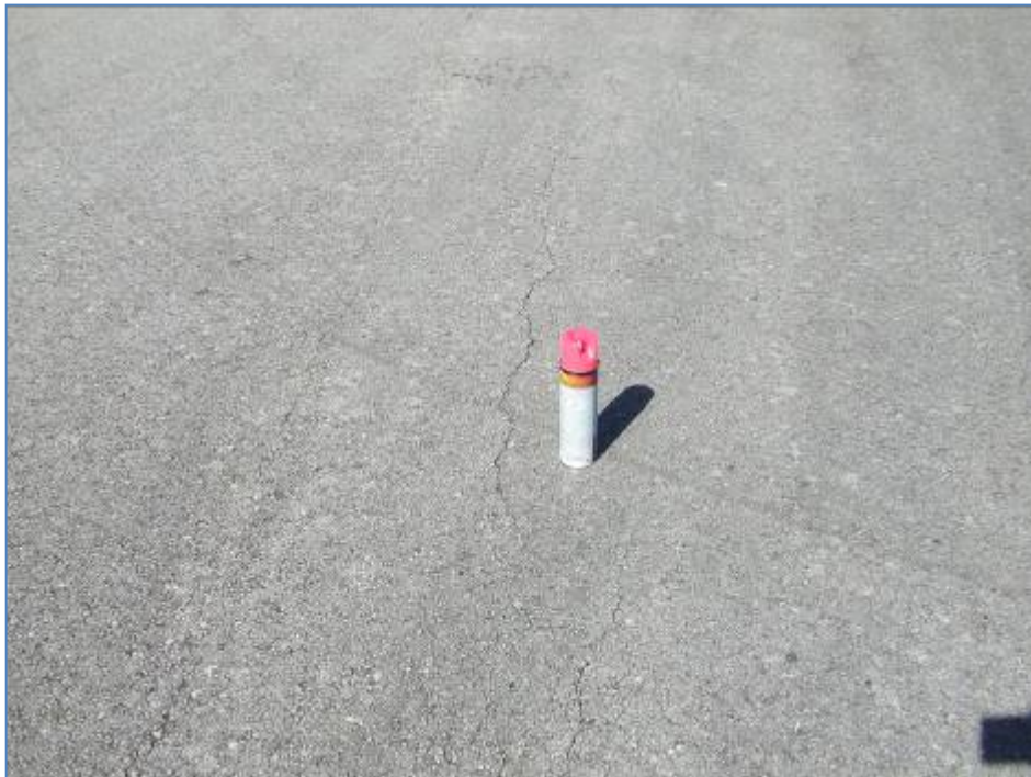
Taxiway Echo 1, Section 517, Sample Unit 104 – Low severity (48) Longitudinal and Transversal Cracking; low, medium and high severity (52) Weathering and Raveling; low severity (56) Swelling.
