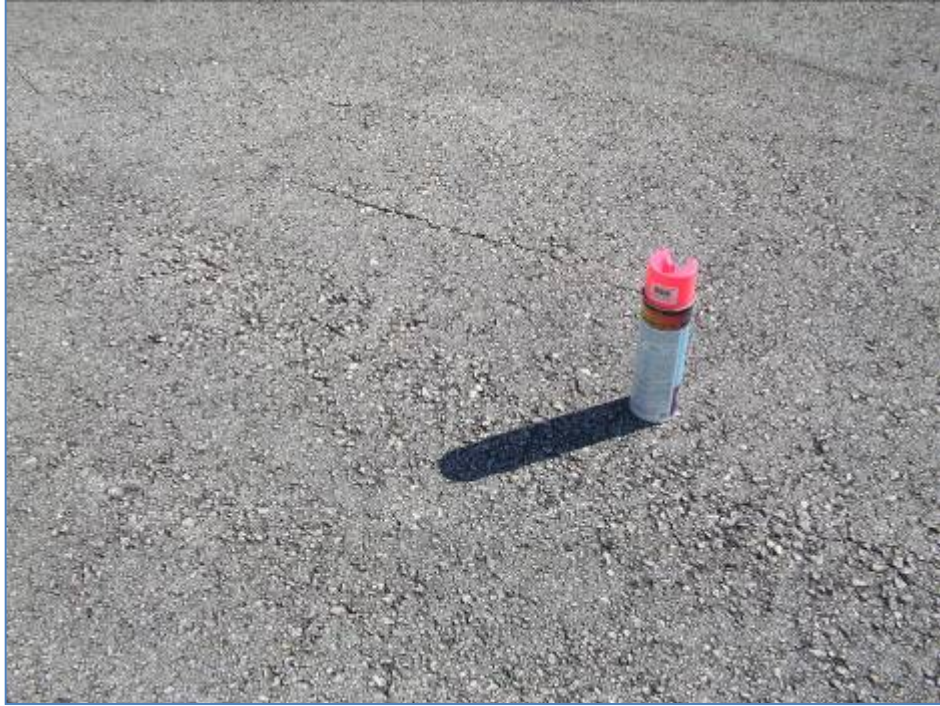
Taxiway Echo, Section 510, Sample Unit 648 – Low severity (48) Longitudinal and Transverse Cracking, low and medium severity (52) Weathering and Raveling, low severity (56) Swelling.
