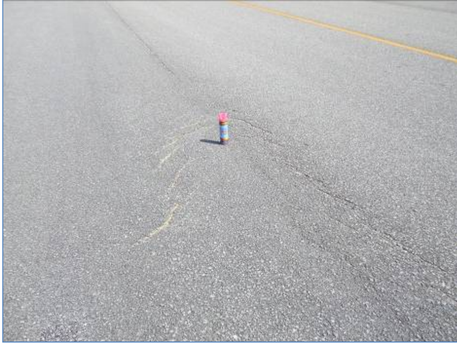
Taxiway Alpha, Section 110, Sample Unit 102 – Low severity (48) Longitudinal and Transverse Cracking, low and medium severity (52) Weathering and Raveling, low severity (55) Slippage Cracking
