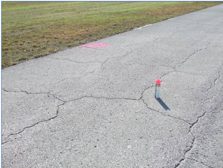
Taxiway Echo, Section 505, Sample Unit 622 – Medium severity (43) Block Cracking; low, medium, and high severity (48) Longitudinal and Transverse Cracking; low severity (52) Weathering and Raveling.
