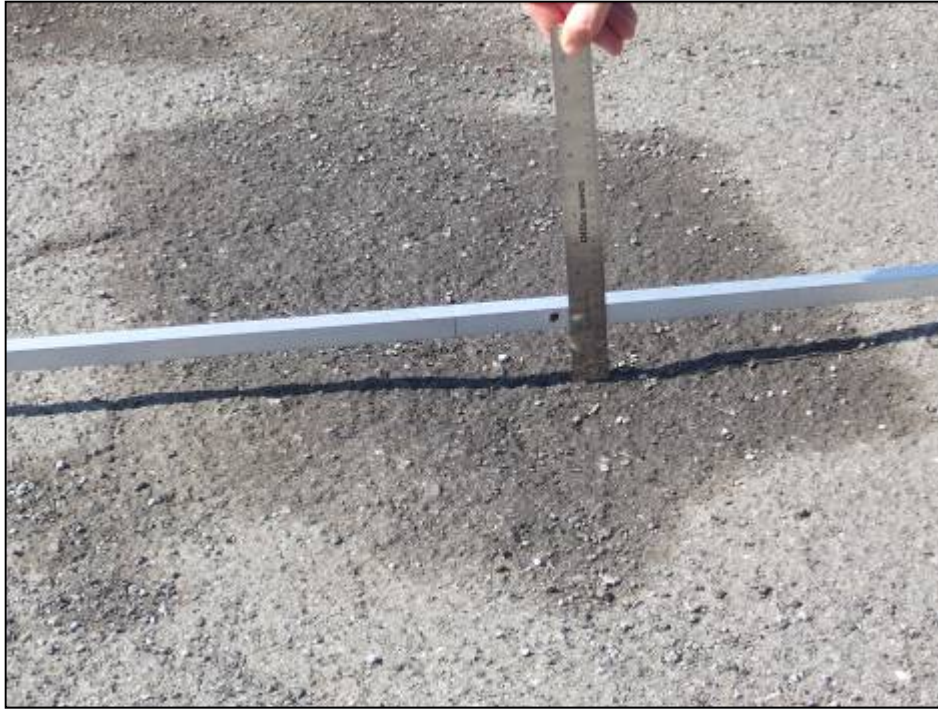
Apron, Section 4105, Sample Unit 100 – Low severity (43) Block Cracking, low and medium severity (45) Depression, medium severity (50) Patching, medium and high severity (52) Weathering and Raveling, low severity (56) Swelling.
