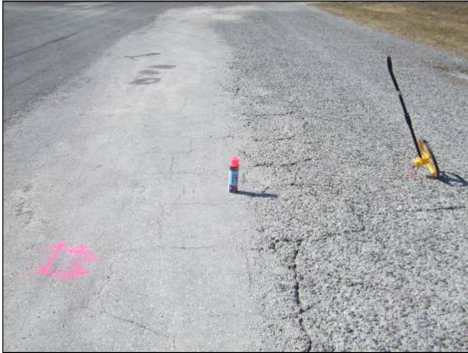
Taxiway Alpha, Section 105 Sample Unit 100 – Low severity (43) Block Cracking, low and medium severity (45) Depression, low severity (48) Longitudinal and Transverse Cracking, medium severity (50) Patching, high severity (52) Weathering and Raveling, low severity (56) Swelling.
