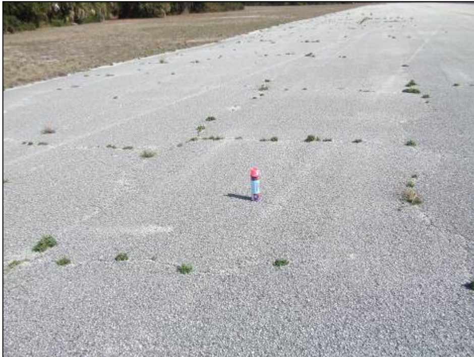
Runway 5-25, Section 6105, Sample Unit 105 – Low severity (43) Block Cracking, low severity (52) Weathering and Raveling, low severity (56) Swelling.
