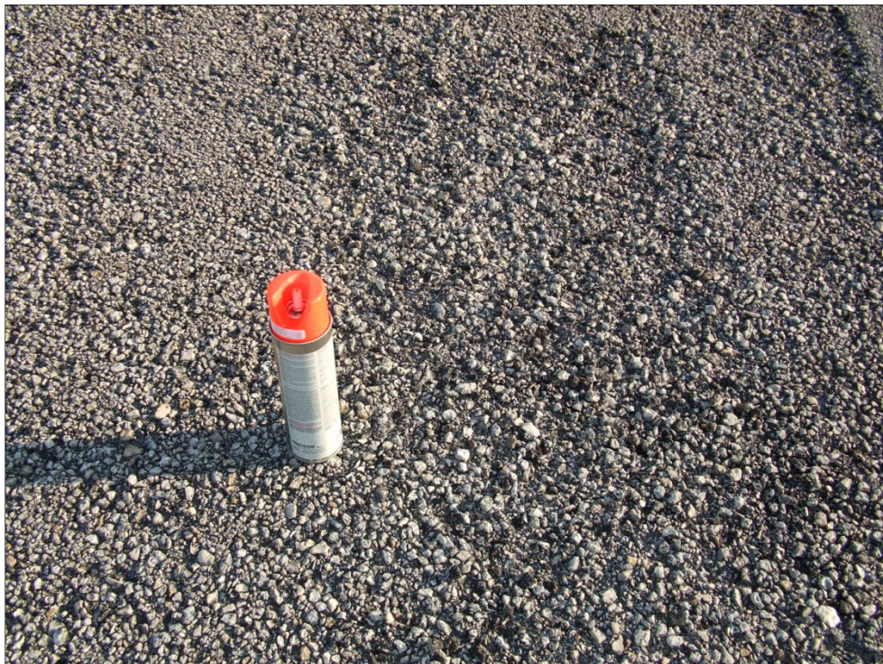
Run Up Apron on RWs 7, 25, Section 5110, Sample Unit 100 – High severity (52) Weathering and Raveling.
