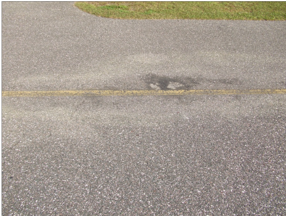
Taxiway T-Hangars, Section 925, Sample Unit 200 – Low severity (45) Depression and low severity (52) Weathering and Raveling
