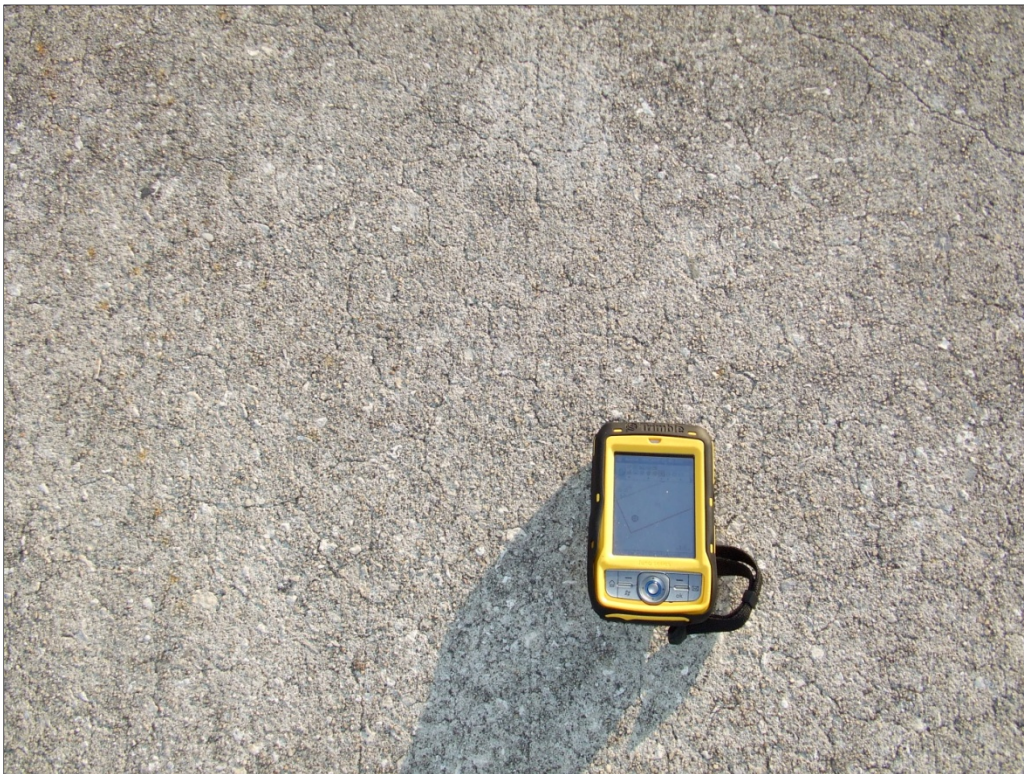
Northeast Apron, Section 4410, Sample Unit 201 –Low severity (70) Scaling.
