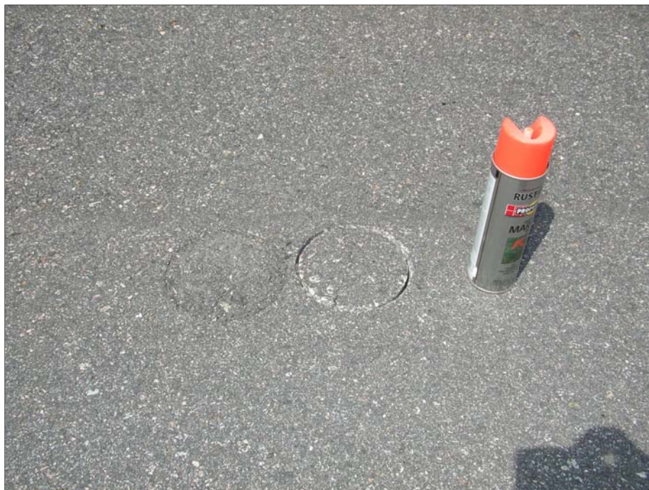
Runway 7-25, Section 6105, Sample Unit 106 – Low severity (50) Patching
