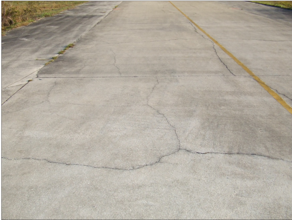
Taxiway to Northeast Apron, Section 1105, Sample Unit 500 – Low severity (63) Linear Cracking, low severity (65) Joint Seal Damage, medium severity (74) Joint Spalling, and low severity (72) Shattered Slab.
