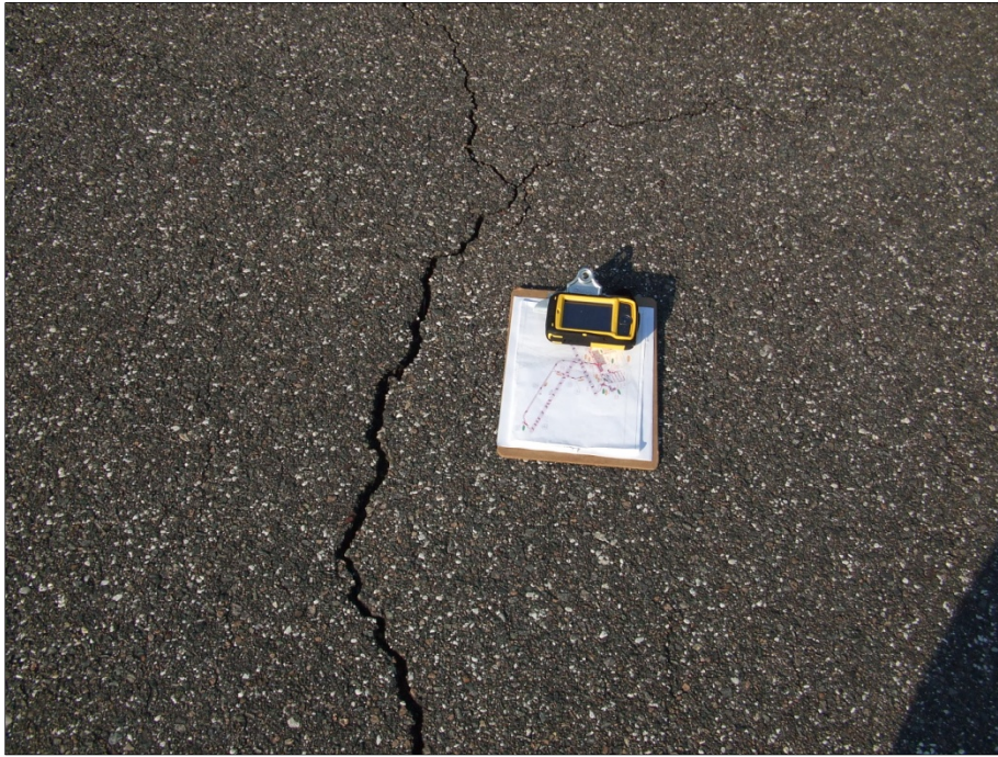
Taxiway T-Hangars, Section 920, Sample Unit 101 – Medium severity (48) Longitudinal / Transverse Cracking and low severity (52) Weathering and Raveling.
