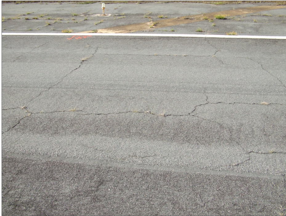
Runway 11-29, Section 6205, Sample Unit 149 – Low severity (43) Block Cracking and low severity (52) Weathering and Raveling
