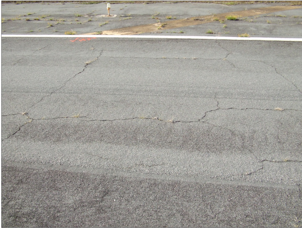
Runway 11-29, Section 6205, Sample Unit 149 – Low severity (43) Block Cracking, and low to medium severity (52) Weathering and Raveling.
