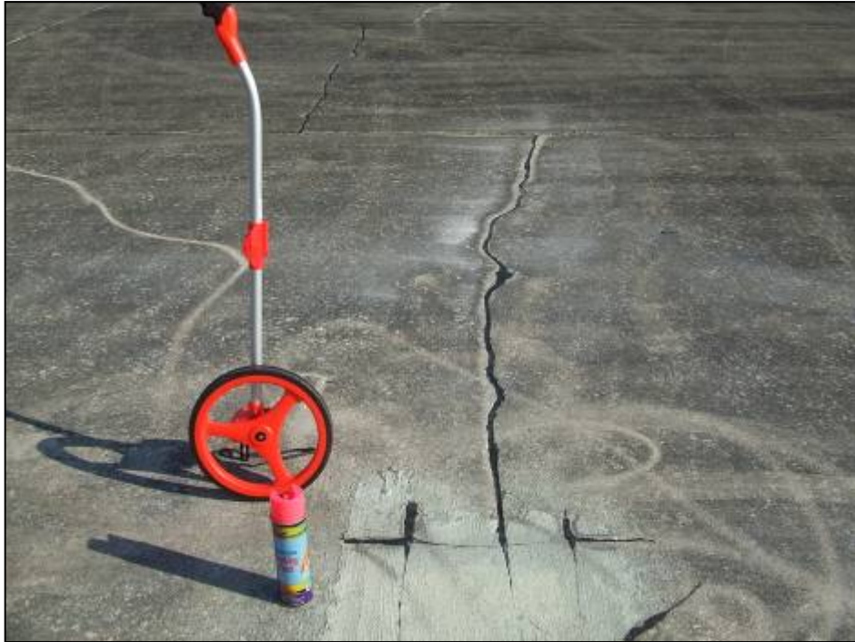
Runway 9-27, Section 6110, Sample Unit 306 – Low severity (63) Linear Cracking, low severity (65) Joint Seal Damage, low severity (66) Small Patch, low severity (70) Scaling.
