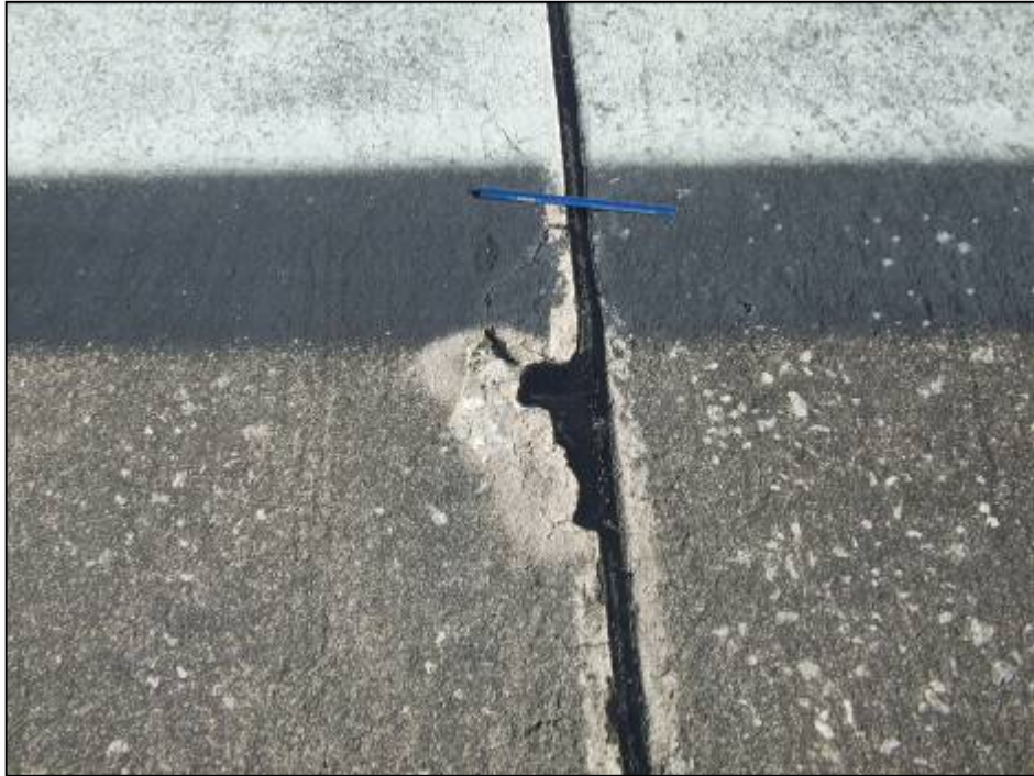
Runway 9-27, Section 6105, Sample Unit 520 – Low and medium severity (63) Linear Cracking, low severity (65) Joint Seal Damage, low severity (66) Small Patch, low severity (67) Large Patch, low severity (70) Scaling.
