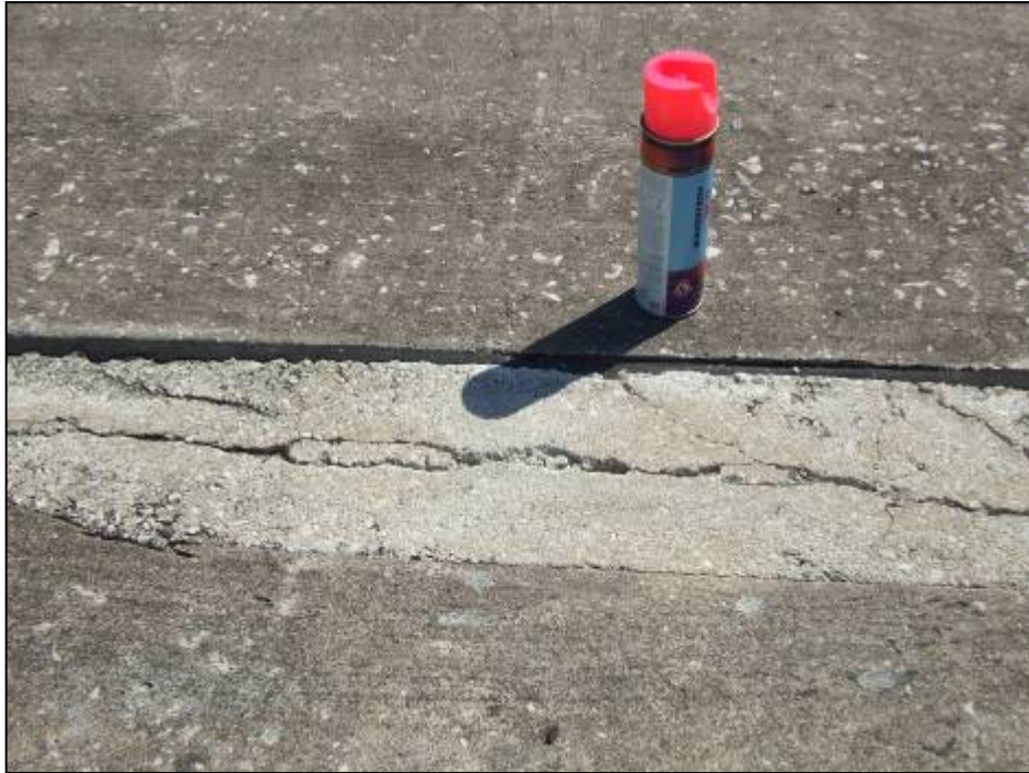
Taxiway Alpha, Section 105, Sample Unit 121 – Low severity (65) Joint Seal Damage, low and medium severity (66) Small Patch, low severity (70) Scaling, low severity (73) Shrinkage Cracking.
