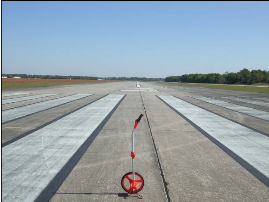
Runway 3-21, Section 6210, Sample Unit 301 – Low and medium severity (63) Linear Cracking, low severity (65) Joint Seal Damage, low and medium severity (66) Small Patch, low severity (70) Scaling, low severity (74) Joint Spalling.
