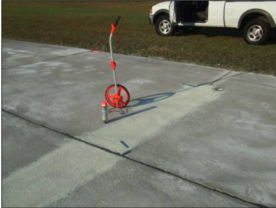
Taxiway Alpha, Section 140, Sample Unit 906 – Low severity (63) Linear Cracking, low severity (65) Joint Seal Damage, low severity (66) Small Patch, low severity (67) Large Patch, low severity (70) Scaling.
