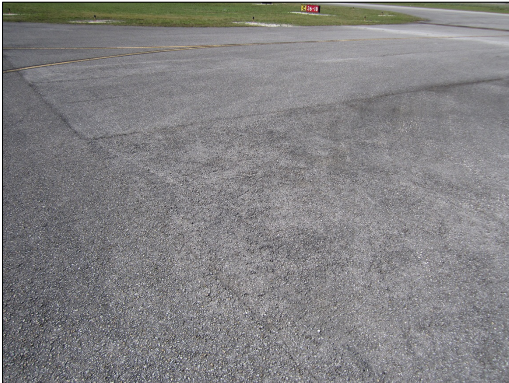
Taxiway B-4, Section 140, Sample Unit 402 – Low severity (48) Longitudinal and Transverse Cracking, low and medium severity (52) Weathering and Raveling
