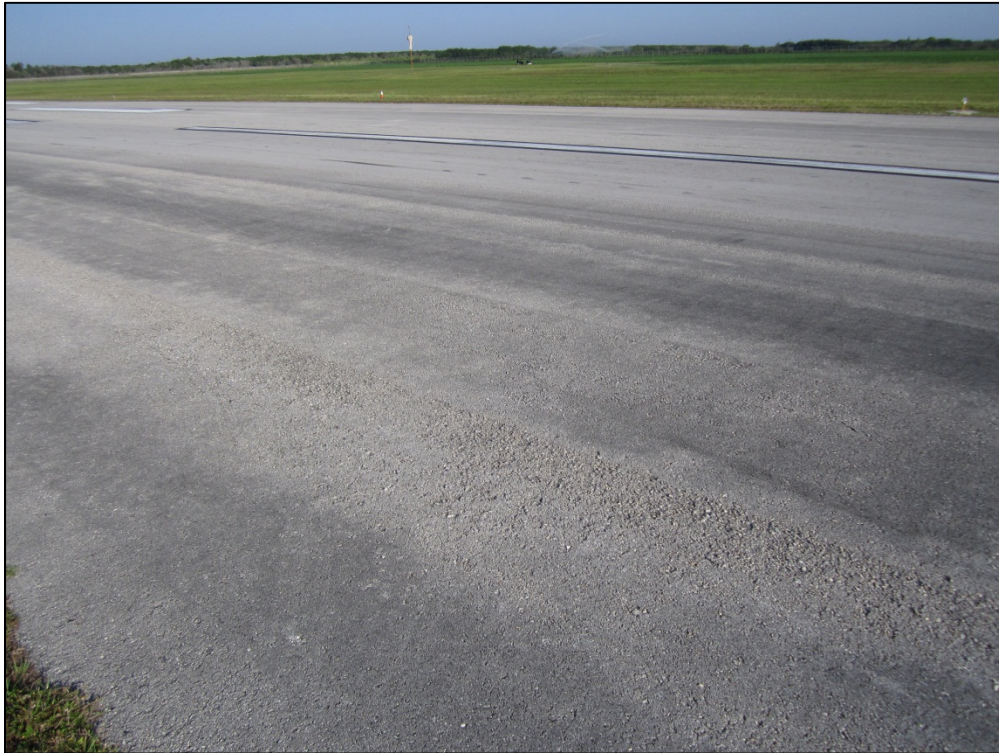
Runway 10-28, Section 6205, Sample Unit 107 – Low severity (48) Longitudinal and Transverse Cracking, low and medium severity (52) Weathering and Raveling
