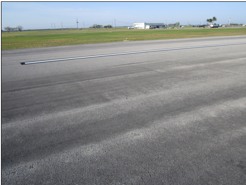
Runway 10-28, Section 6205, Sample Unit 149 – Low severity (48) Longitudinal and Transverse Cracking, low severity (52) Weathering and Raveling
