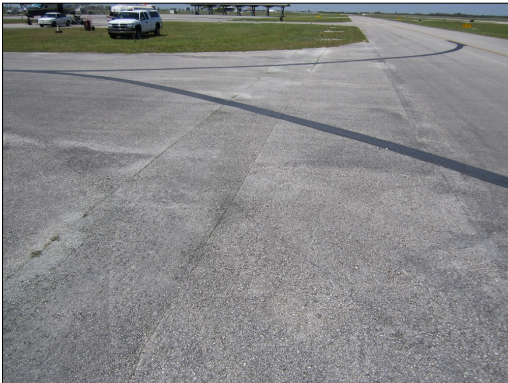
Taxiway Alpha, Section 295, Sample Unit 202 – Low severity (48) Longitudinal and Transverse Cracking, low and medium severity (52) Weathering and Raveling, medium severity (50) Patching
