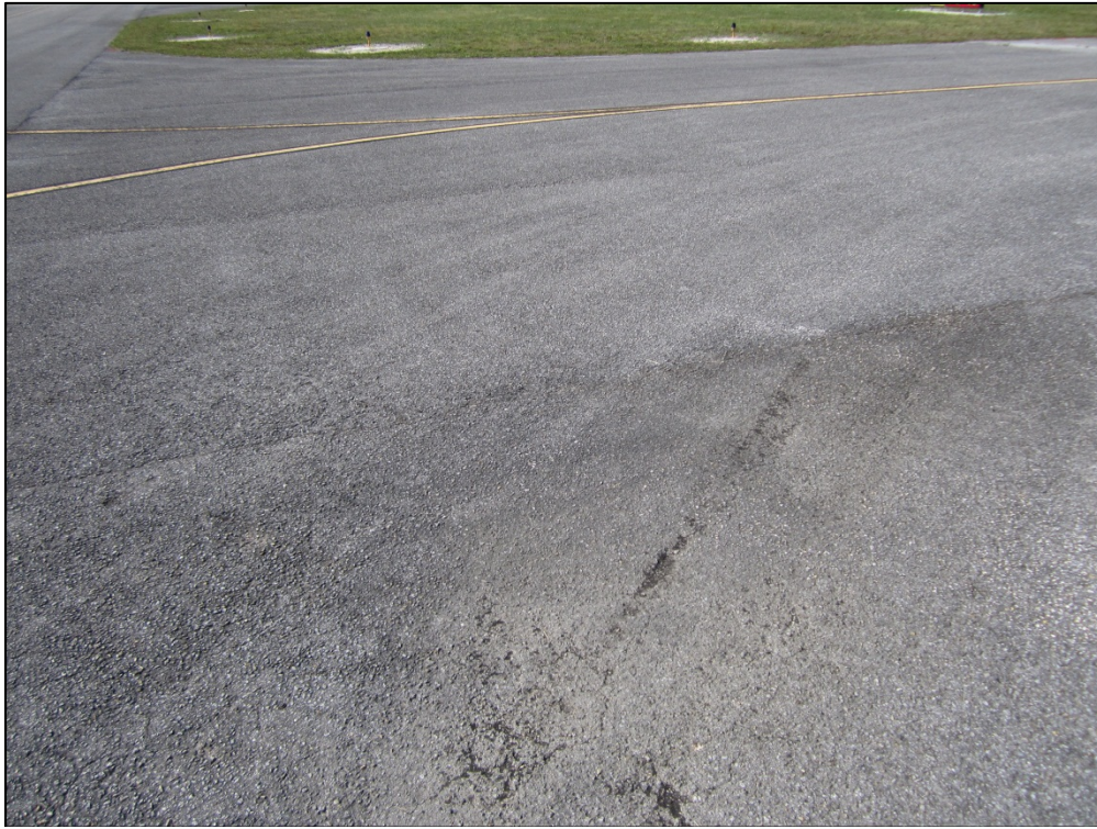
Taxiway B-3, Section 130, Sample Unit 302 – Low severity (48) Longitudinal and Transverse Cracking, low and medium severity (52) Weathering and Raveling
