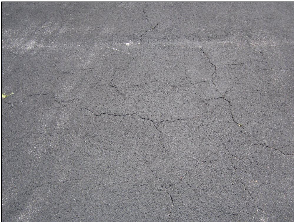
Northwest Apron, Section 4105, Sample Unit 454 – Low severity (48) Longitudinal and Transverse Cracking, low severity (43) Block Cracking, low severity (52) Weathering and Raveling
