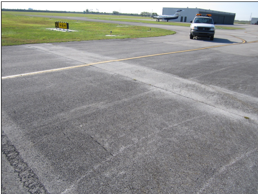
Taxiway A-3, Section 250, Sample Unit 301 – Low severity (48) Longitudinal and Transverse Cracking, low and medium severity (52) Weathering and Raveling, low severity (50) Patching
