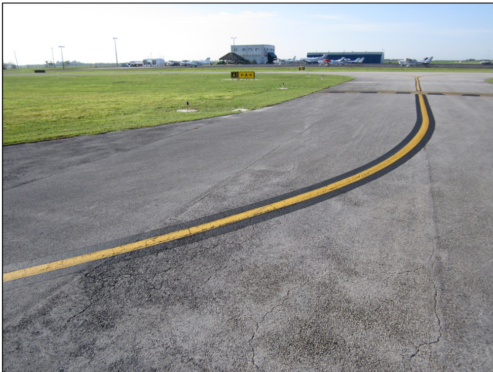
Taxiway A-1, Section 230, Sample Unit 100 – Low severity (48) Longitudinal and Transverse Cracking, low severity (52) Weathering and Raveling, low severity (41) Alligator Cracking
