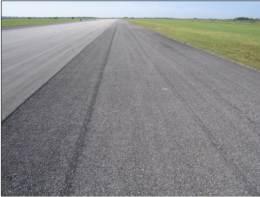
Runway 18-36, Section 6110, Sample Unit 164 – Low severity (48) Longitudinal and Transverse Cracking, low severity (52) Weathering and Raveling
