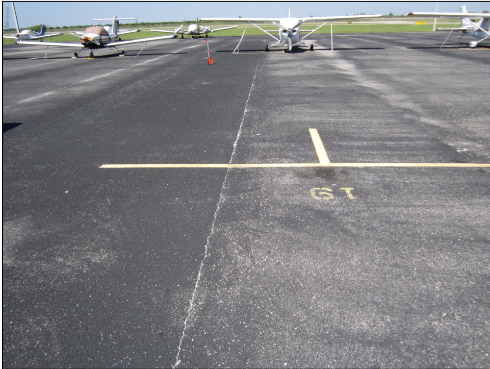
Northwest Apron, Section 4105, Sample Unit 153 – Low severity (48) Longitudinal and Transverse Cracking, low severity (52) Weathering and Raveling
