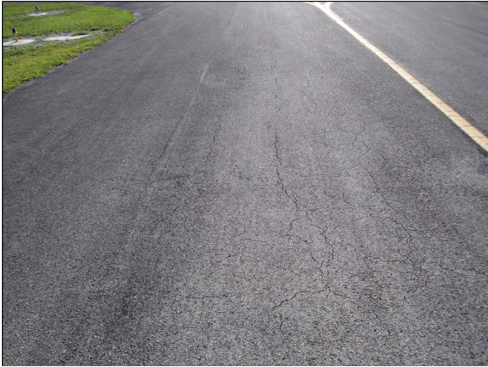
Taxiway Alpha, Section 215, Sample Unit 117 – Low severity (48) Longitudinal and Transverse Cracking, low severity (52) Weathering and Raveling, low severity (43) Block Cracking
