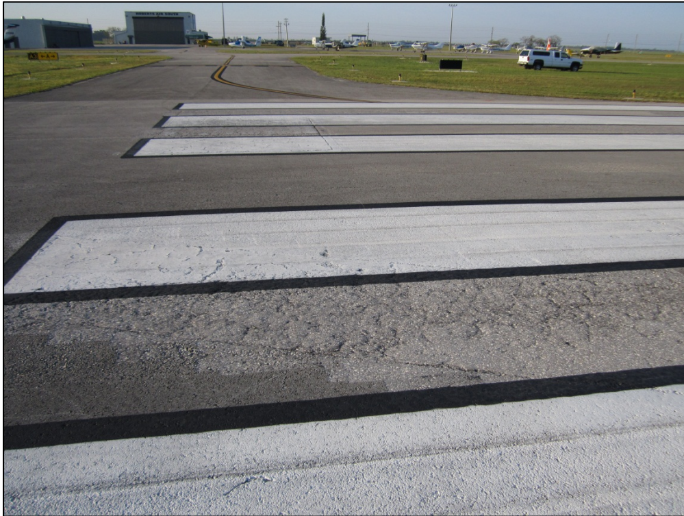
Runway 10-28, Section 6205, Sample Unit 159 – Low severity (48) Longitudinal and Transverse Cracking, low and medium severity (52) Weathering and Raveling
