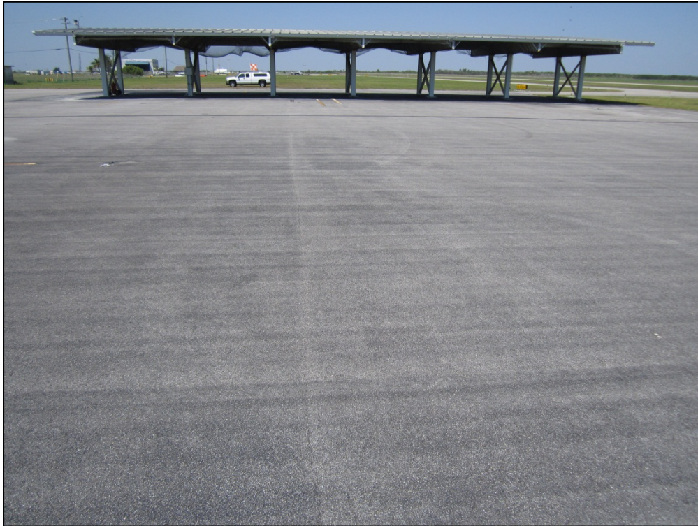
North Apron, Section 4205, Sample Unit 202 – Low severity (48) Longitudinal and Transverse Cracking, low severity (52) Weathering and Raveling
