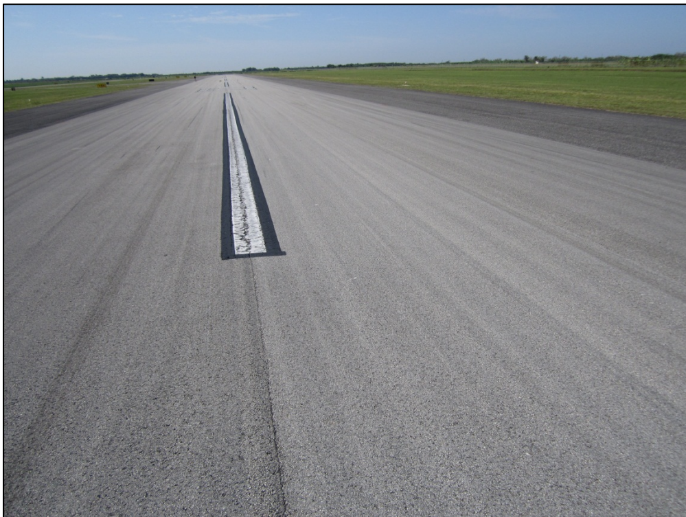
Runway 18-36, Section 6105, Sample Unit 320 – Low severity (48) Longitudinal and Transverse Cracking, low severity (52) Weathering and Raveling
