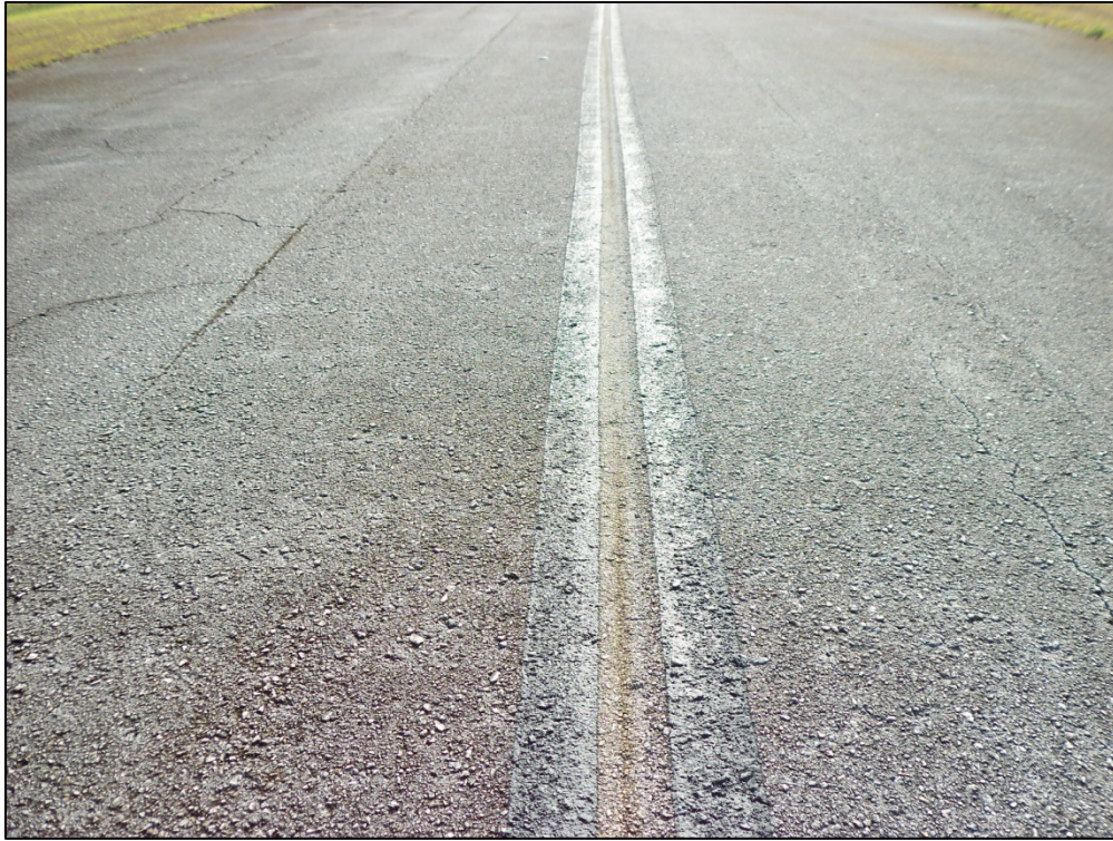
Taxiway Bravo, Section 105, Sample Unit 108 – Low and medium severity (43) Block Cracking, medium severity (52) Weathering and Raveling
