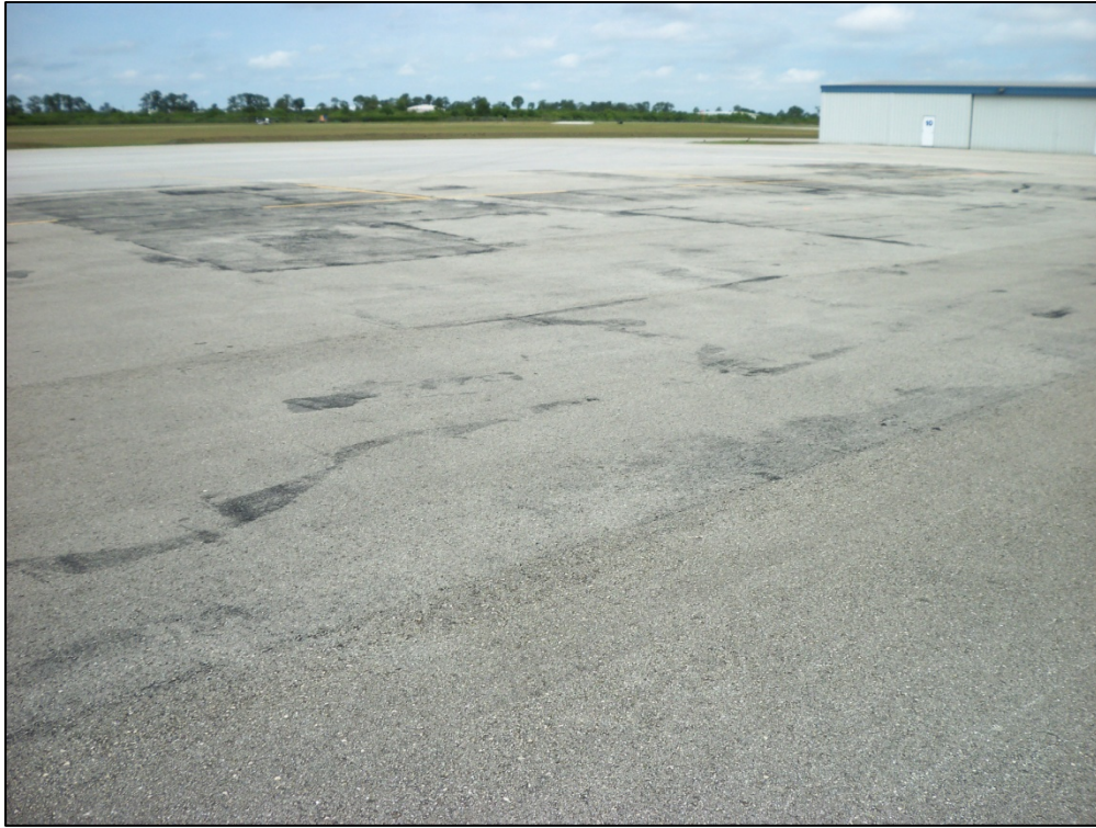
Apron, Section 4210, Sample Unit 203 – Low severity (48) Longitudinal and Transverse Cracking, low severity (50) Patch ,low severity (52) Weathering and Raveling
