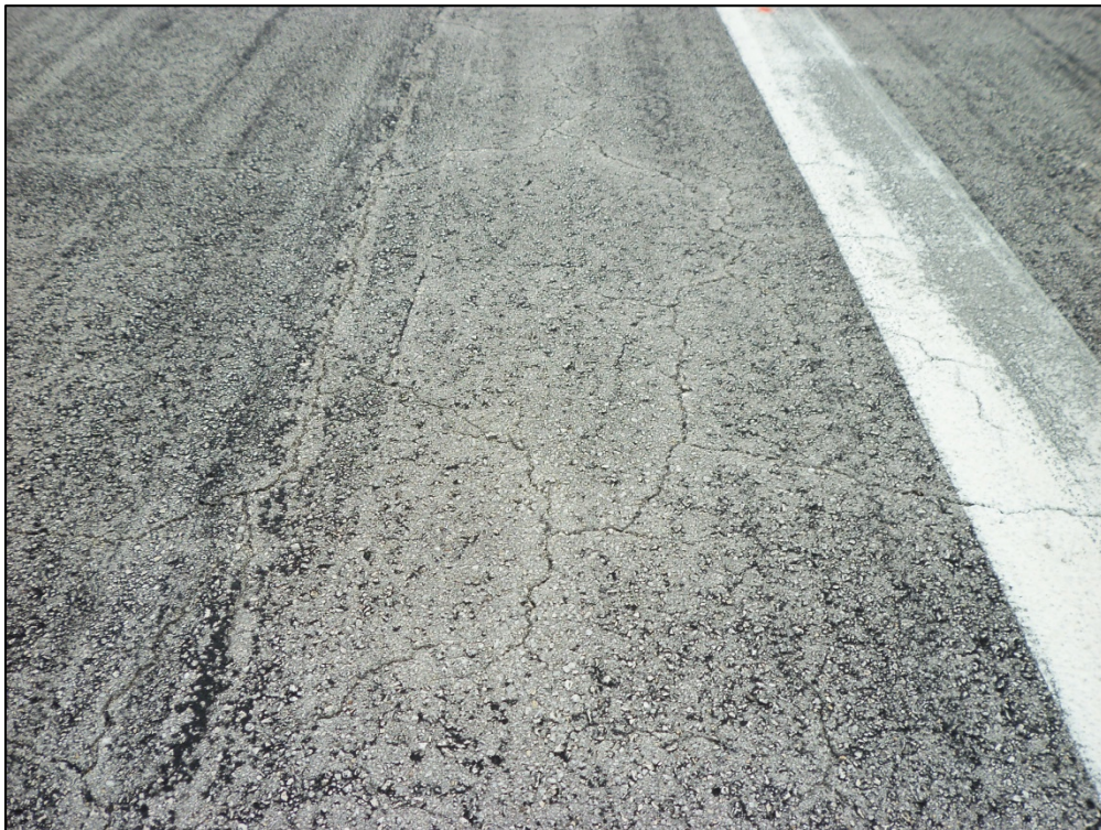
Runway 18-36, Section 6115, Sample Unit 383 – Medium severity (43) Block Cracking, medium severity (48) Longitudinal and Transverse Cracking, medium severity (52) Weathering and Raveling
