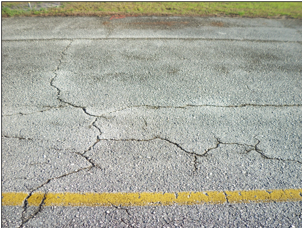
Taxiway A-1, Section 210, Sample Unit 201 – Medium severity (43) Block Cracking, medium severity (50) Patch, medium severity (52) Weathering and Raveling
