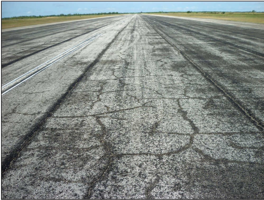
Runway 9-27, Section 6215, Sample Unit 380 – Low and medium severity (43) Block Cracking, medium severity (52) Weathering and Raveling
