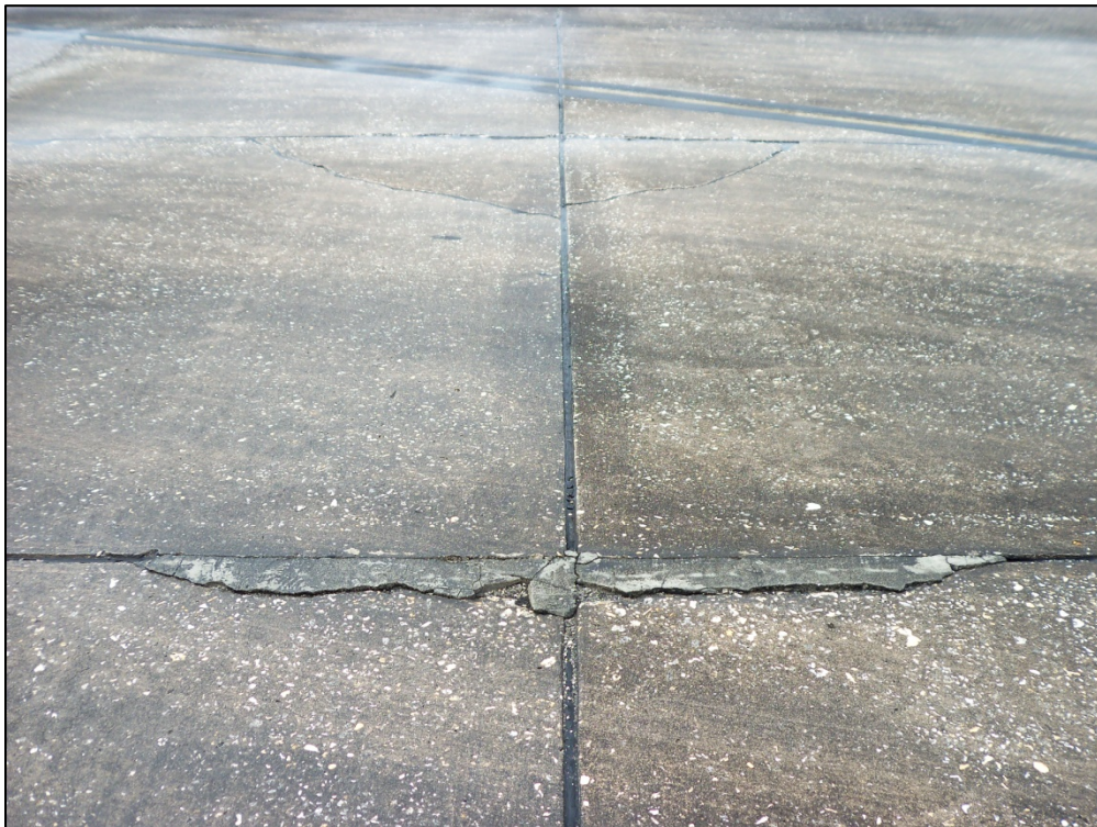
Runway 9-27, Section 6225, Sample Unit 388 – Low, medium and high severity (62) Corner Break, (63) LTD Cracking, (65) Joint Seal Damage, (70) Scaling/Map Cracking, (72) Shattered Slabs, (73) Shrinkage Cracks, (74) Joint Spalling, (75) Corner Spalling
