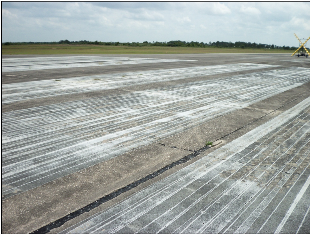
Runway 18-36, Section 6125, Sample Unit 392 – Low, medium and high severity (62) Corner Break, (63) LTD Cracking, (65) Joint Seal Damage, (70) Scaling/Map Cracking, (72) Shattered Slabs, (73) Shrinkage Cracks, (74) Joint Spalling, (75) Corner Spalling
