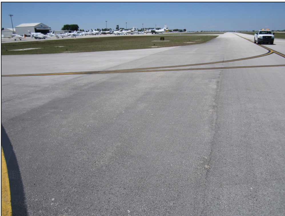
Taxiway Alpha, Section 108, Sample Unit 148 – Low severity (52) Weathering and Raveling; low severity (48) Longitudinal and Transverse Cracking
