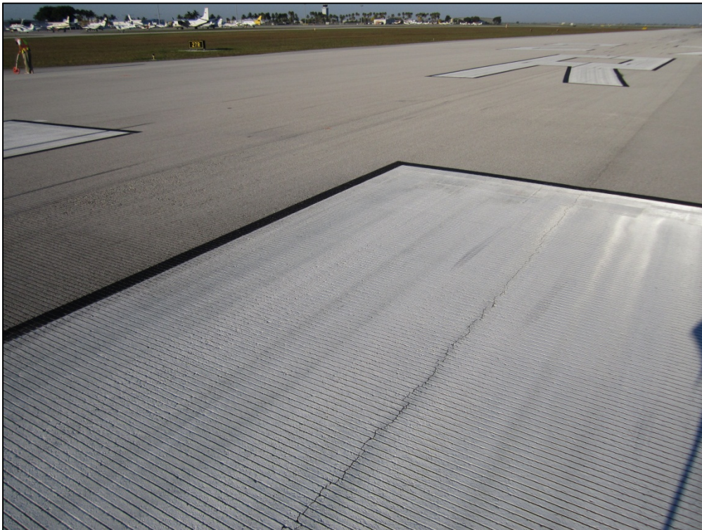
Runway 9L-27R, Section 6131, Sample Unit 396 – Low severity (52) Weathering and Raveling; low severity (48) Longitudinal and Transverse Cracking
