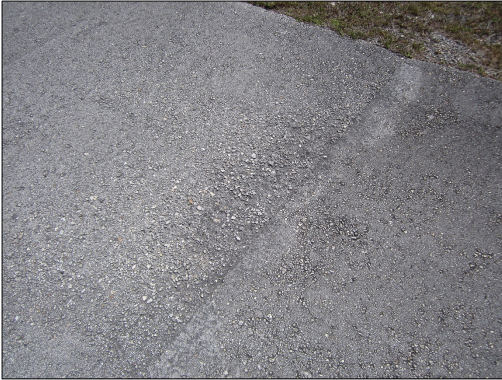
Taxiway Echo, Section 505, Sample Unit 159 – Medium severity (52) Weathering and Raveling
