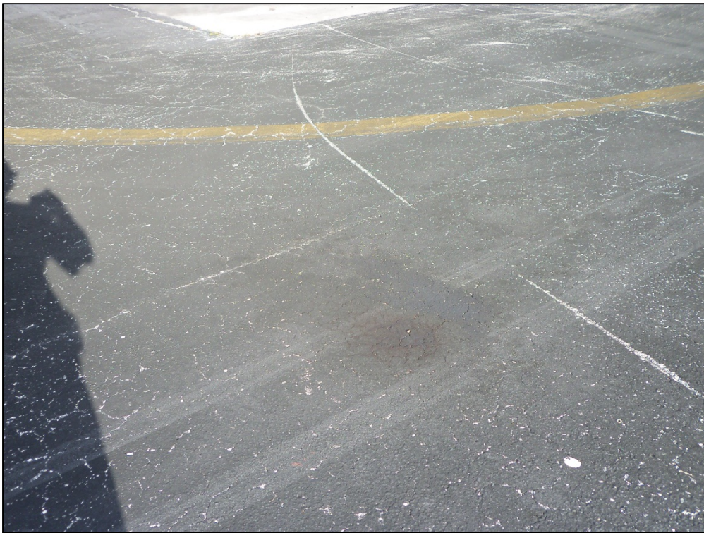
Southeast Apron, Section 4410, Sample Unit 501 – Low severity (52) Weathering and Raveling; low severity (48) Longitudinal and Transverse Cracking; (49) Oil Spillage
