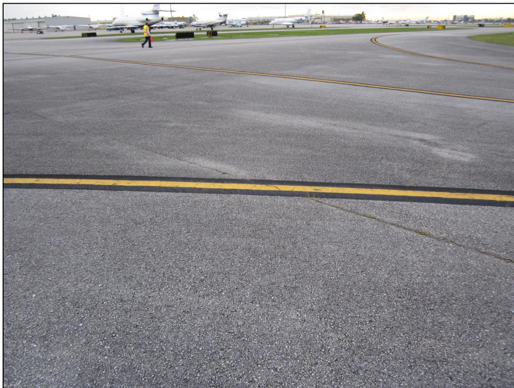
Taxiway D-2, Section 420, Sample Unit 205 – Low to medium severity (52) Weathering and Raveling; low severity (48) Longitudinal and Transverse Cracking
