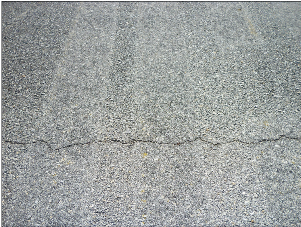
Taxiway D-1, Section 415, Sample Unit 101 – Low to medium severity (52) Weathering and Raveling; low severity (48) Longitudinal and Transverse Cracking
