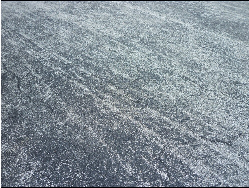
South Apron, Section 4140, Sample Unit 402 – Low severity (52) Weathering and Raveling; low severity (43) Block Cracking
