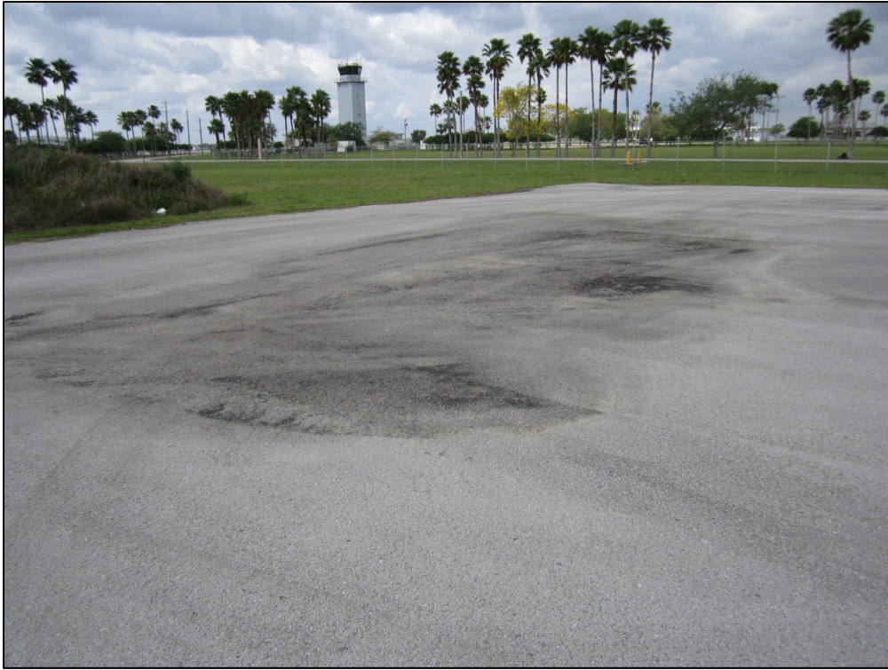
North Apron, Section 4230, Sample Unit 102 – Low severity (52) Weathering and Raveling; low severity (45) Depression
