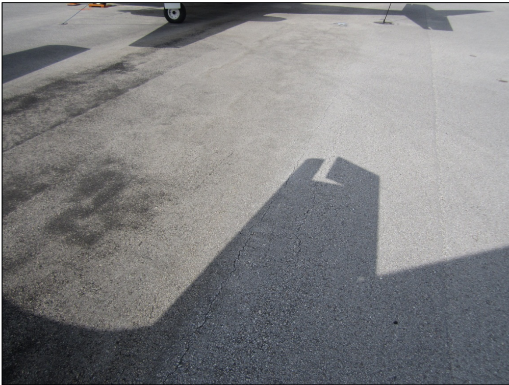
North Apron, Section 4205, Sample Unit 312 – Low severity (52) Weathering and Raveling; low severity (48) Longitudinal and Transverse Cracking; low severity (56) Swelling; (49) Oil Spillage
