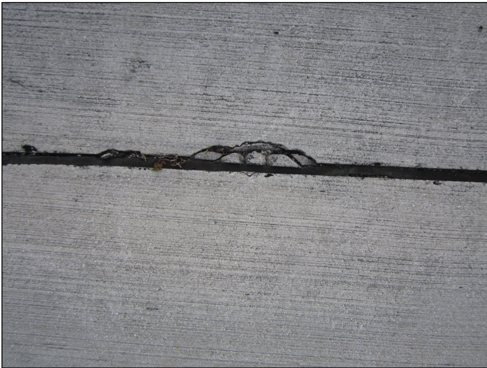
Northeast Apron, Section 4305, Sample Unit 201 – Low severity (74) Joint Spalling
