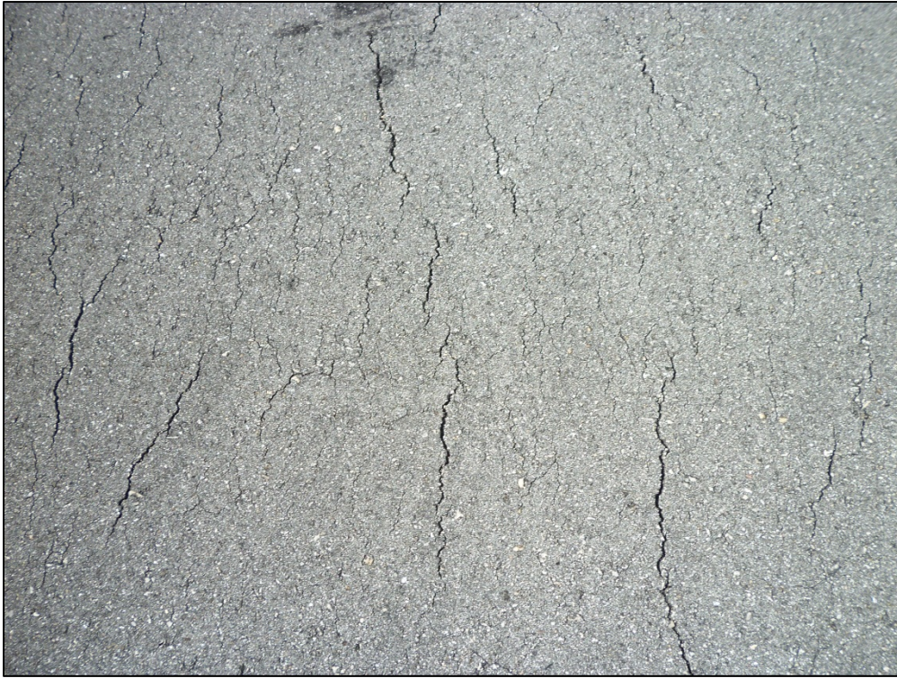
Runway 13-31, Section 6210, Sample Unit 508 – Low severity (52) Weathering and Raveling; low severity (48) Longitudinal and Transverse Cracking
