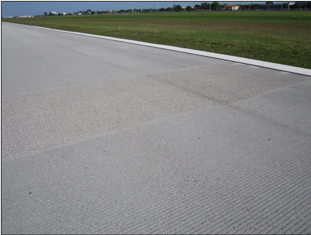
Runway 9R-27L, Section 6310, Sample Unit 544 – Low to medium severity (52) Weathering and Raveling
