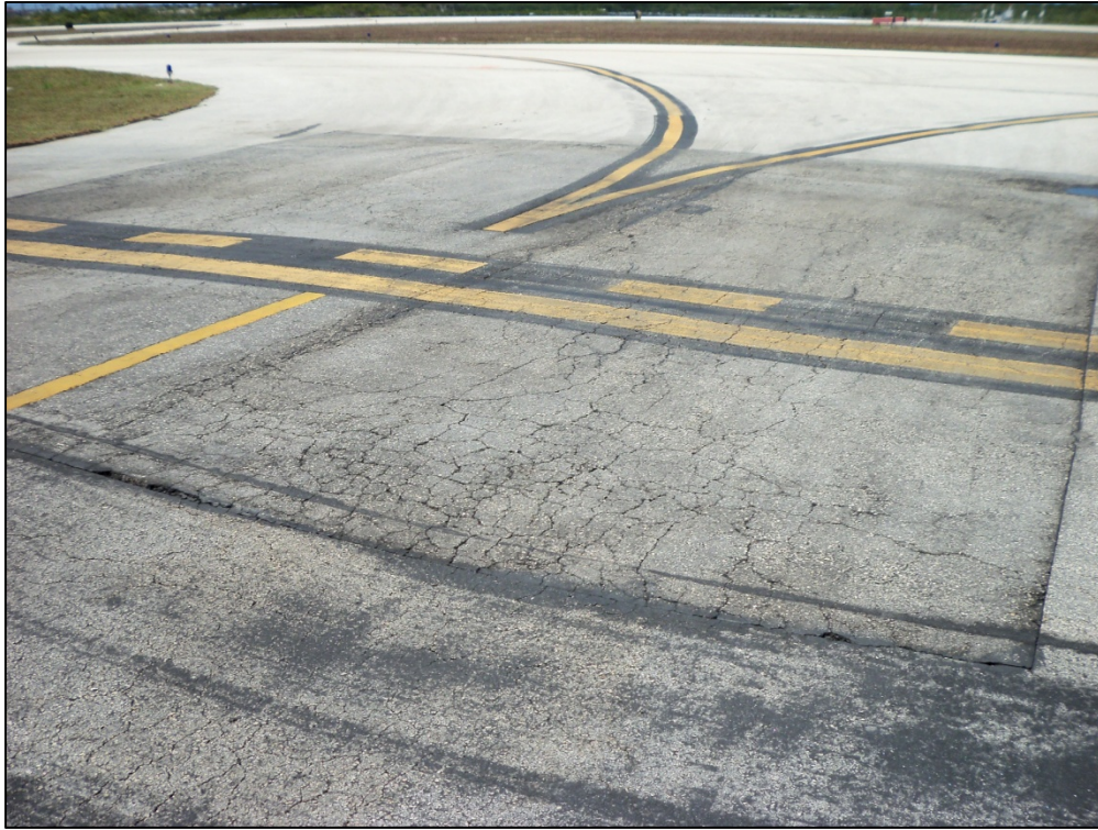
Taxiway Connector A9, Section 4150, Sample Unit 300 – Low and medium severity (43) Block Cracking, low severity (45) Depression, low and medium severity (48) Longitudinal and Transverse Cracking, high severity (50) Patch, low severity (52) Raveling and Weathering
