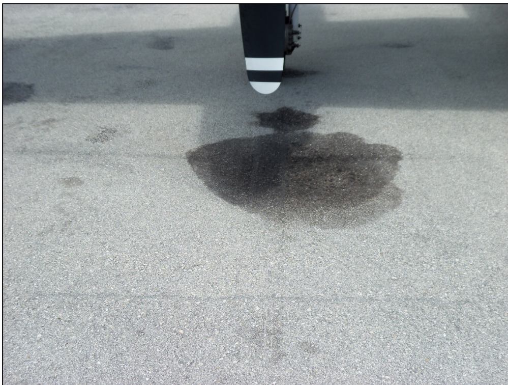
Hangars, Section 4215, Sample Unit 505 – (49) Oil Spillage, low severity (50) Patch, Medium severity (52) Raveling and Weathering
