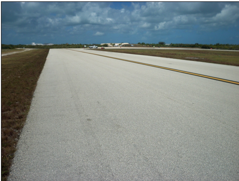
Taxiway Alpha, Section 105, Sample Unit 105 – Low severity (48) Longitudinal and Transverse Cracking, low severity (52) Raveling and Weathering
