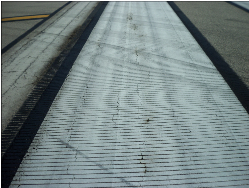
Runway 9-27, Section 6110, Sample Unit 100 – Low and Medium severity (48) Longitudinal and Transverse Cracking, low severity (52) Raveling and Weathering
