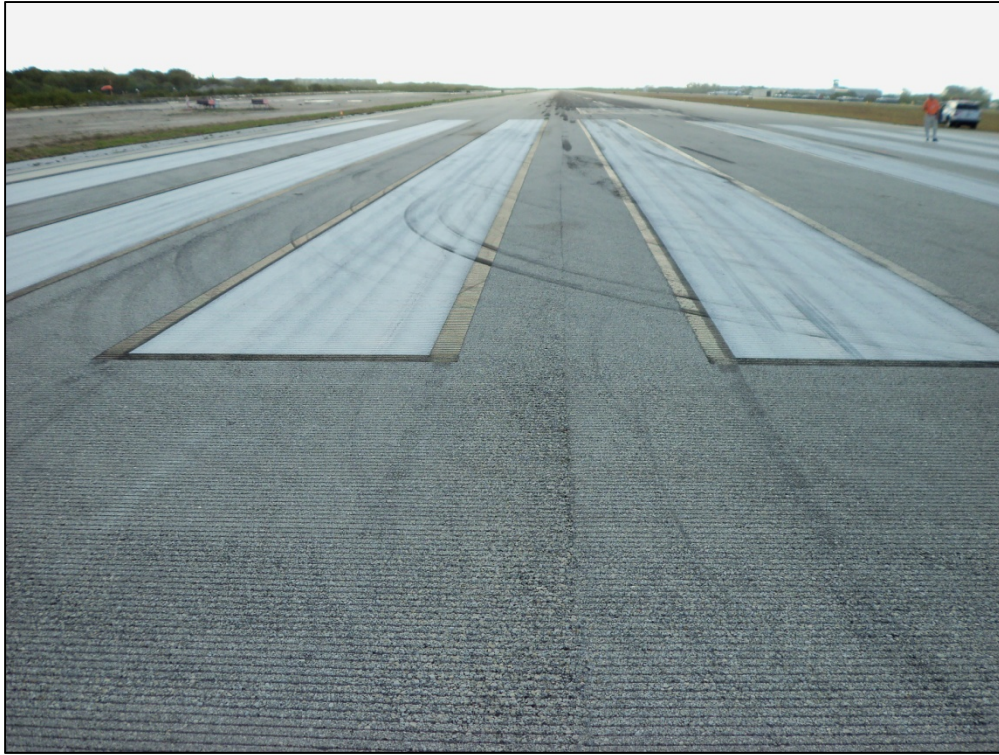
Runway 9-27, Section 6105, Sample Unit 100 – Low severity (48) Longitudinal and Transverse Cracking, low severity (52) Raveling and Weathering
