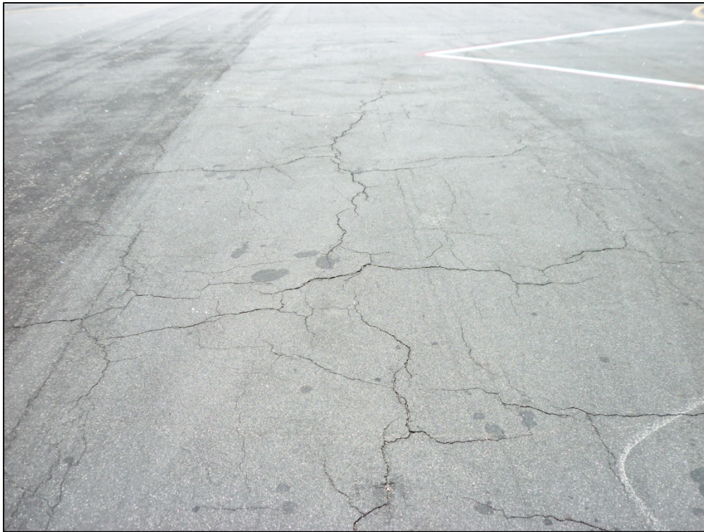
Commercial Apron, Section 4115, Sample Unit 605 – Low severity (50) Patch, medium severity (52) Raveling and Weathering
