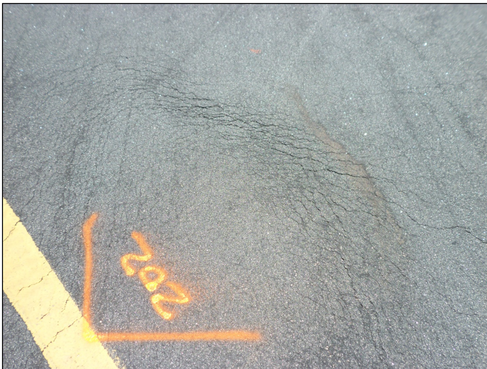
Commercial Apron, Section 510, Sample Unit 202 – Medium severity (52) Raveling and Weathering, medium severity (55) Slippage
