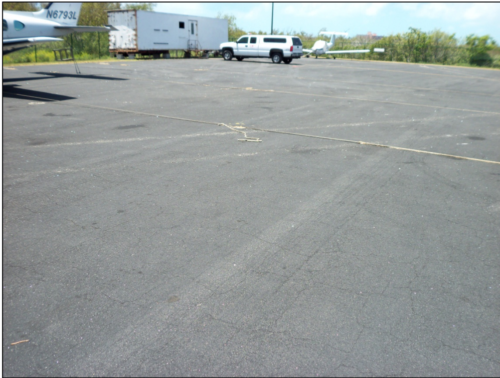
Apron (Overflow), Section 4210, Sample Unit 501 – Low severity (50) Patch, low severity (52) Raveling and Weathering
