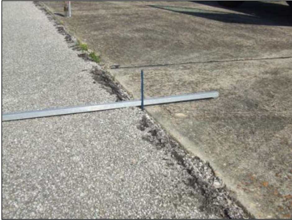
Apron, Section 4110, Sample Unit 200 – Low severity (48) Longitudinal and Transverse Cracking, low severity (54) Shoving, low and medium severity (52) Weathering and Raveling.
