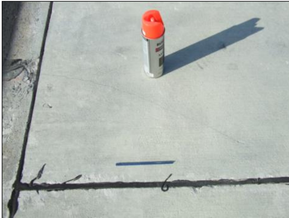
Runway 5-23, Section 6105, Sample Unit 301 – Low severity (62) Corner Break, low severity (63) Linear Cracking, low severity (65) Joint Seal Damage, low severity (67) Large Patch, low severity (70) Scaling, low severity (74) Joint Spalling.
