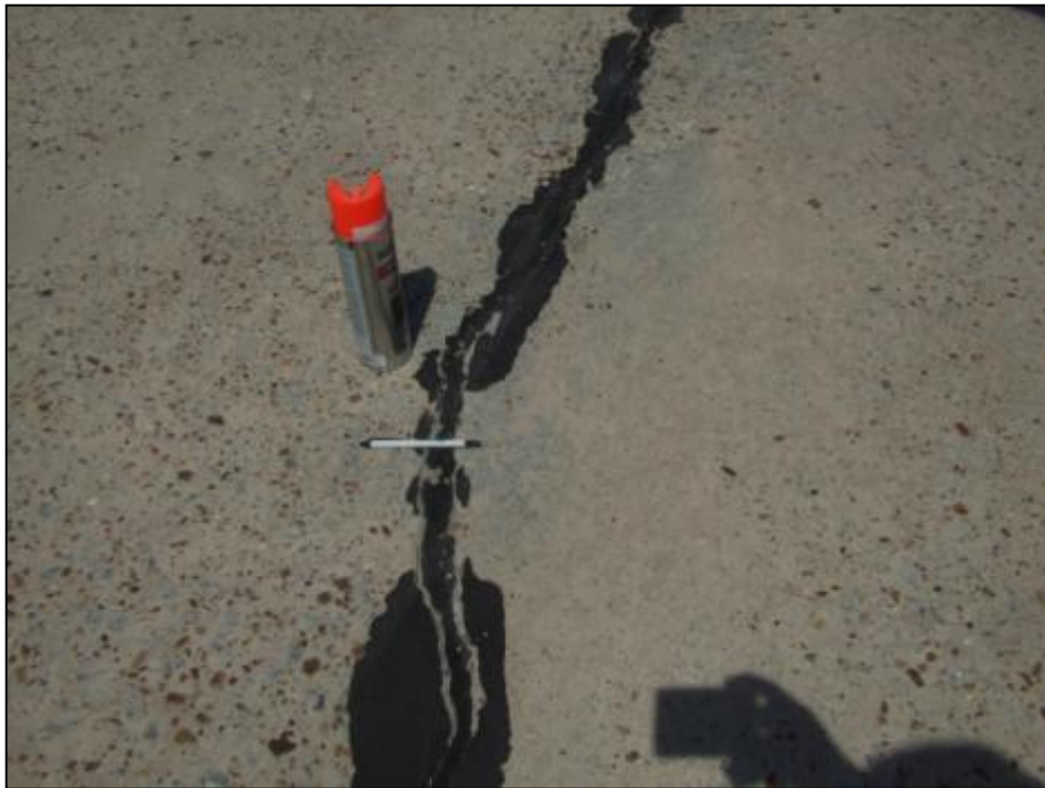
Runway 5-23, Section 6210, Sample Unit 500 – Low severity (62) Corner Break, low and medium severity (63) Linear Cracking, low severity (65) Joint Seal Damage, low severity (70) Scaling, low severity (72) Shattered Slabs, low severity (75) Corner Spall.
