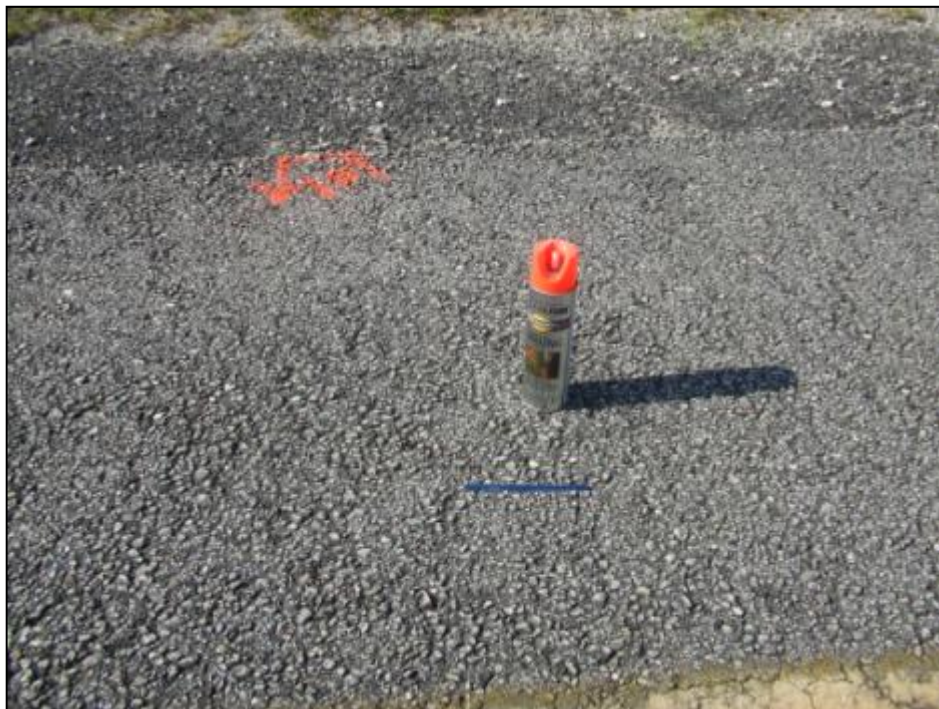
Taxiway Alpha, Section 105, Sample Unit 101 – Low and medium severity (48) Longitudinal and Transverse Cracking, low and medium severity (52) Weathering and Raveling.
