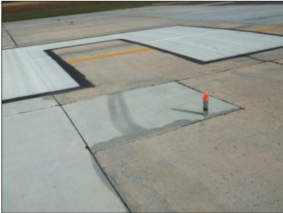
Runway 5-23, Section 6105, Sample Unit 305 – Low severity (62) Corner Break, low severity (63) Linear Cracking, low severity (65) Joint Seal Damage, low severity (67) Large Patch, low severity (70) Scaling.
