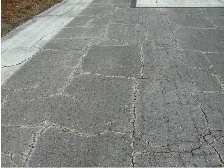
Runway 6-24, Section 6239, Sample Unit 576 – Low and medium severity (43) Block Cracking, low and medium severity (52) Weathering and Raveling.
