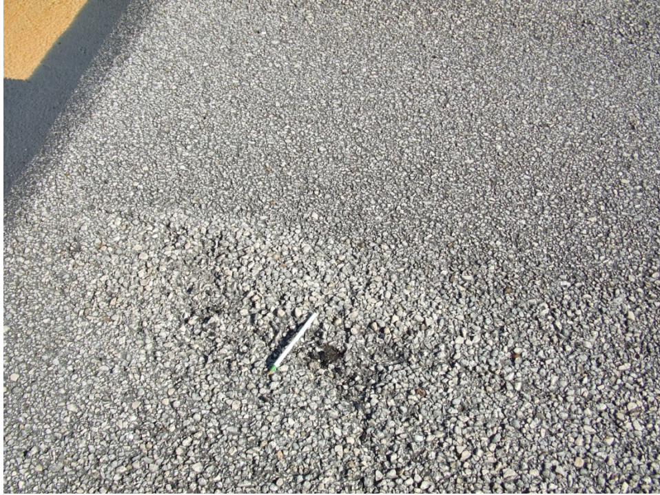
Taxiway Bravo, Section 205, Sample Unit 201 –High severity (52) Weathering and Raveling.
