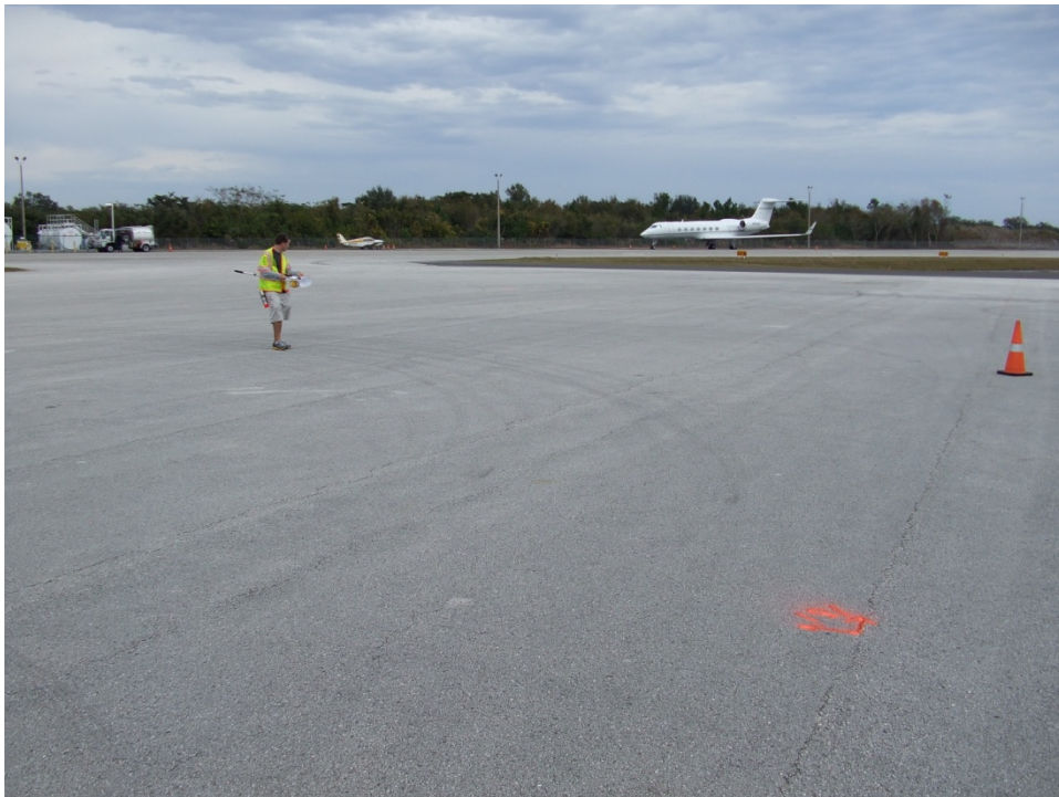
Center Apron, Section 4205, Sample Unit 151 – Low severity (48) Longitudinal and Transverse Cracking, low severity (52) Weathering and Raveling, and low severity (56) Swelling.
