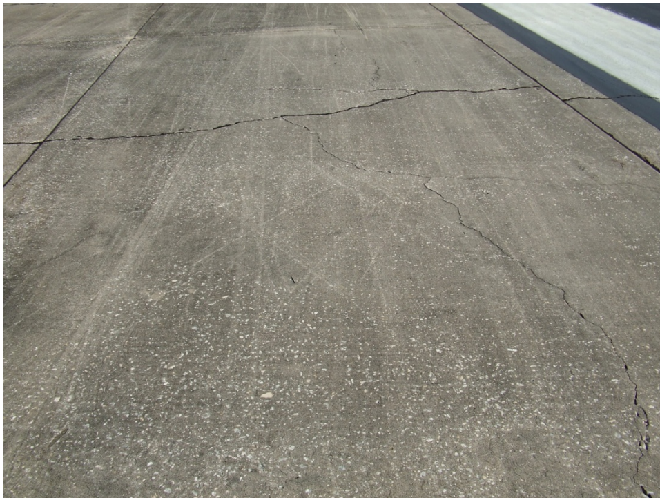
Runway 6-24, Section 6245, Sample Unit 395 – Low, moderate, and high severity (63) Linear Cracking, moderate severity (65) Joint Seal Damage, and low severity (70) Map Cracking / Scaling,.
