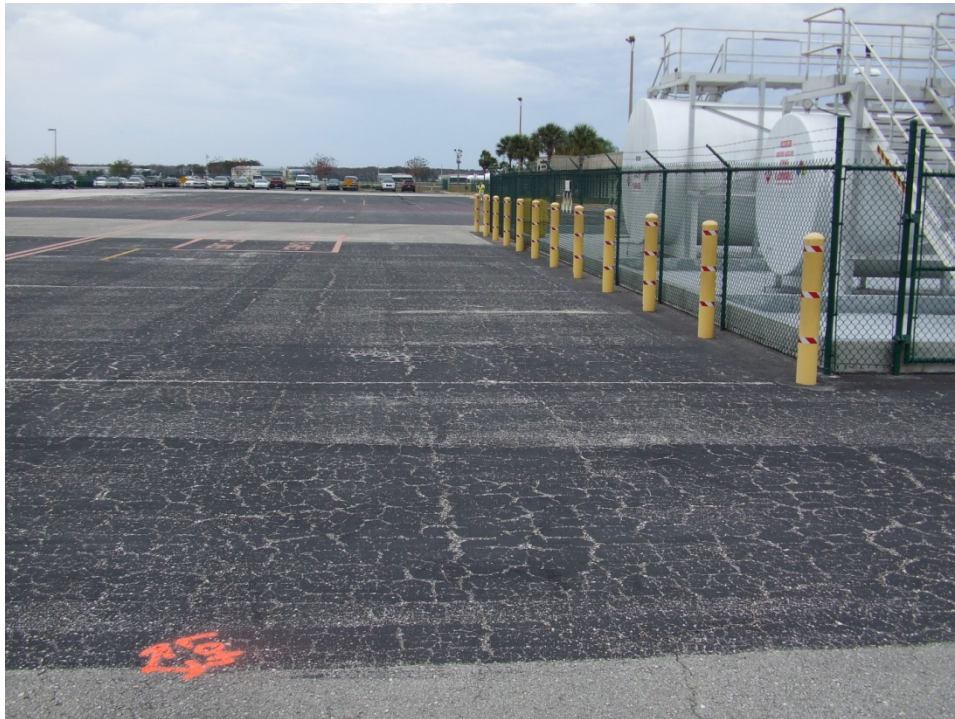
North Apron, Section 4112, Sample Unit 407 – Low severity (43) Block Cracking and medium severity (52) Weathering and Raveling.
