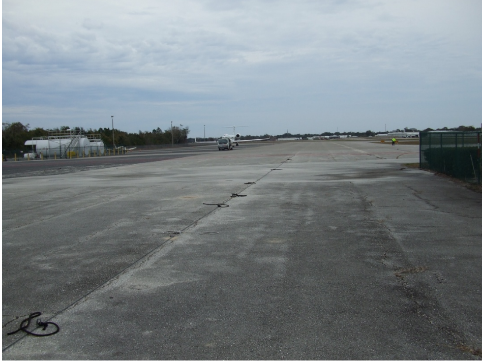
North Apron, Section 4105, Sample Unit 111 – Low and medium severity (48) Longitudinal and Transverse Cracking, and low severity (52) Weathering and Raveling.
