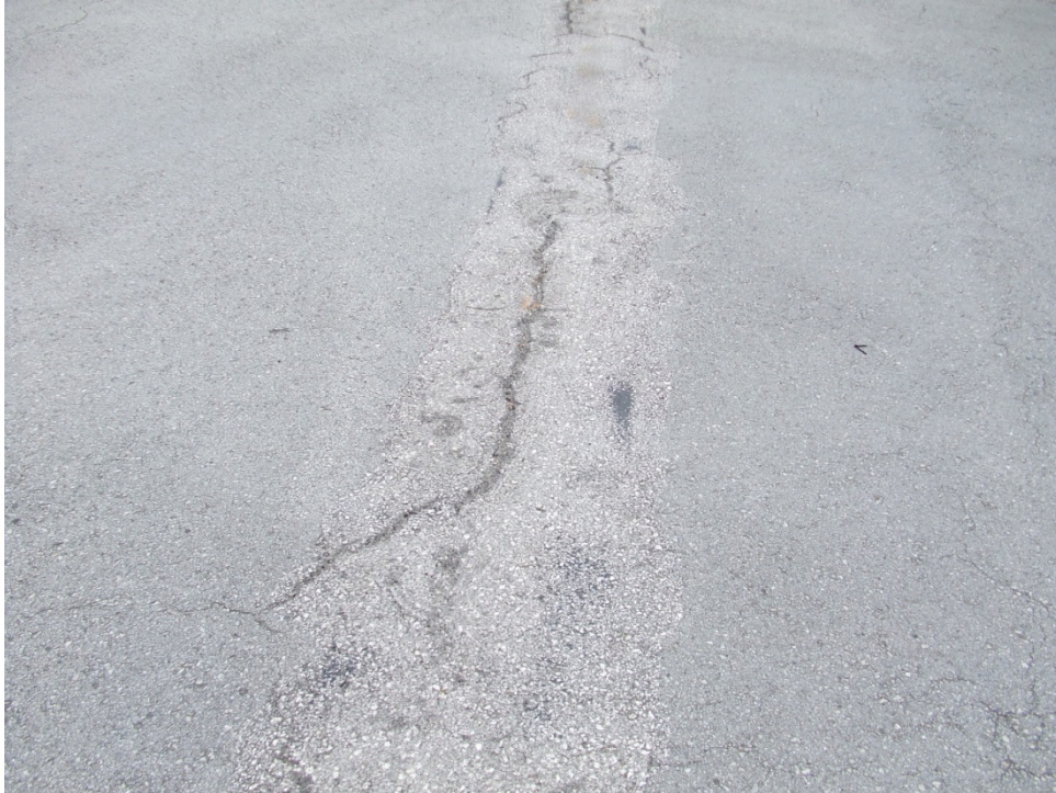
Center Apron, Section 4205, Sample Unit 151 – Low severity (48) Longitudinal and Transverse Cracking and low severity (52) Weathering and Raveling.
