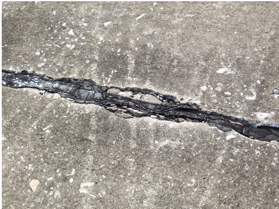
Runway 6-24, Section 6245, Sample Unit 395 – Medium severity (65) Joint Seal Damage, low severity (70) Map Cracking / Scaling, and Medium severity (74) Joint Spalling.
